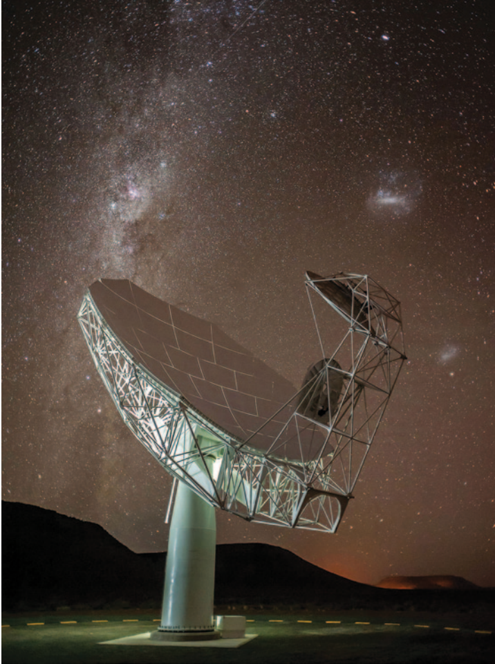
FIG. 15.3 An artist's rendering of a MeerKAT antenna poised to register radio signals from very, very far away. The first has just been constructed and in the next few years another 63 antennas like this will define the project. (Credit: SKA South Africa)
