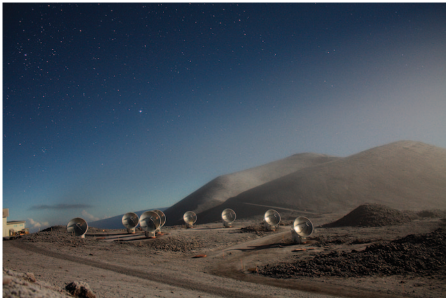
FIG. 14.9 Sentinels on a mountaintop in Hawaii, the Submillimeter Array (SMA) photographed in November 2010 when the array was in its compact configuration. All the antennas were in stow position because they were closed down due to a freezing fog, which had receded just before the photo was taken. The lighting is due to the setting Moon and the ground is still covered in frost. (Credit: Nimesh A. Patel)
