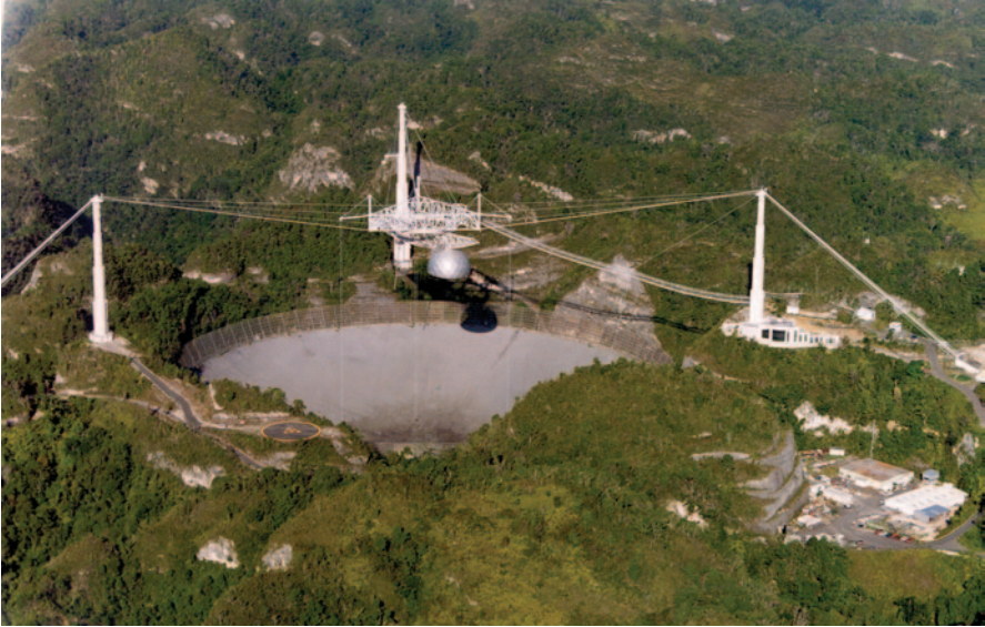
FIG. 18.4 The upgraded William E. Gordon 1000 ft (305 m) diameter radio dish near Arecibo in Puerto Rico. The antennas are housed in the bulbous structure at the focus suspended by cables from three support towers. It houses two other reflectors in what is known as a Gregorian system that then sends the radio waves to a receiver in that enclosure. The diameter of Chinese FAST instrument will be 60 % larger. (Credit: NAIC—Arecibo Observatory, a facility of the NSF)
