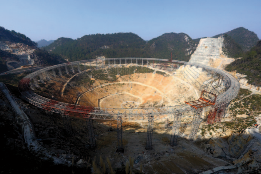
Fig. 16.1 The 500 m (1635 ft) diameter FAST radio telescope under construction in China. (Credit: The FAST group, National Astronomical Observatories of China)
