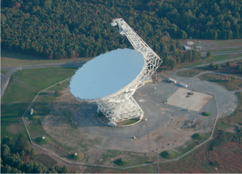
FIG. 18.2 The Robert C. Byrd Green Bank Telescope 100 m (330 ft.) radio telescope of the NRAO in Green Bank, West Virginia. The unusual location of the support structure above the dish reduces unwanted reflections of radio waves from the steel beams that hold up a secondary reflector that then reflects the radio waves to a focus behind the main dish. In most other radio telescopes the support structure has multiple legs located inside the dish. (Credit: NRAO/AUI/NSF)
