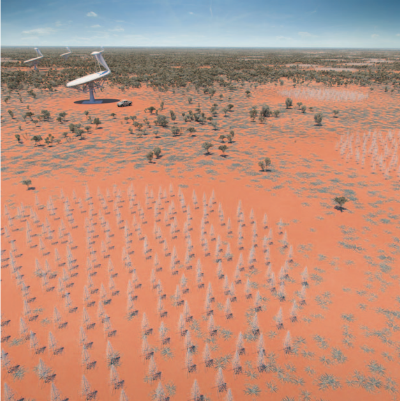
FIG. 15.1 Artist's impression of a small section of the low frequency segment of the SKA to be constructed in Australia's Murchison semi-desert region involving hundreds of thousands of strange-looking dipole antennas in clusters that stretch into the distance. Also shown are a number of survey telescopes being planned that will become part of the project as it moves into a subsequent phase. (Credit: SKA Organization)
