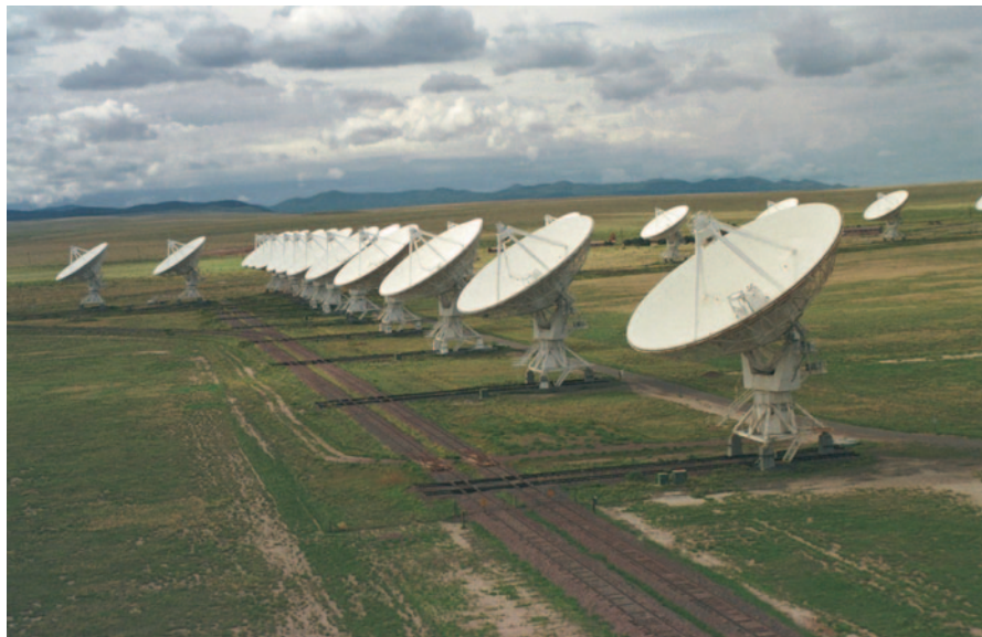
FIG. 1.2 The VLA radio telescope of the National Radio Astronomy Observatory located west of Socorro, NM, out in the middle of nowhere, which is what radio astronomers prefer in order to avoid unwanted radio interference. In this view the dishes are spaced in the so-called compact array. The railroad tracks on which the dishes can be moved for up to 11 miles along each of three arms of the array can be seen in the foreground. The VLA uses the principles of aperture synthesis to create images of radio sources and now is part of the even larger Expanded VLA, also known as the Jansky VLA. (Credit NRAO/AUI/NSF)
