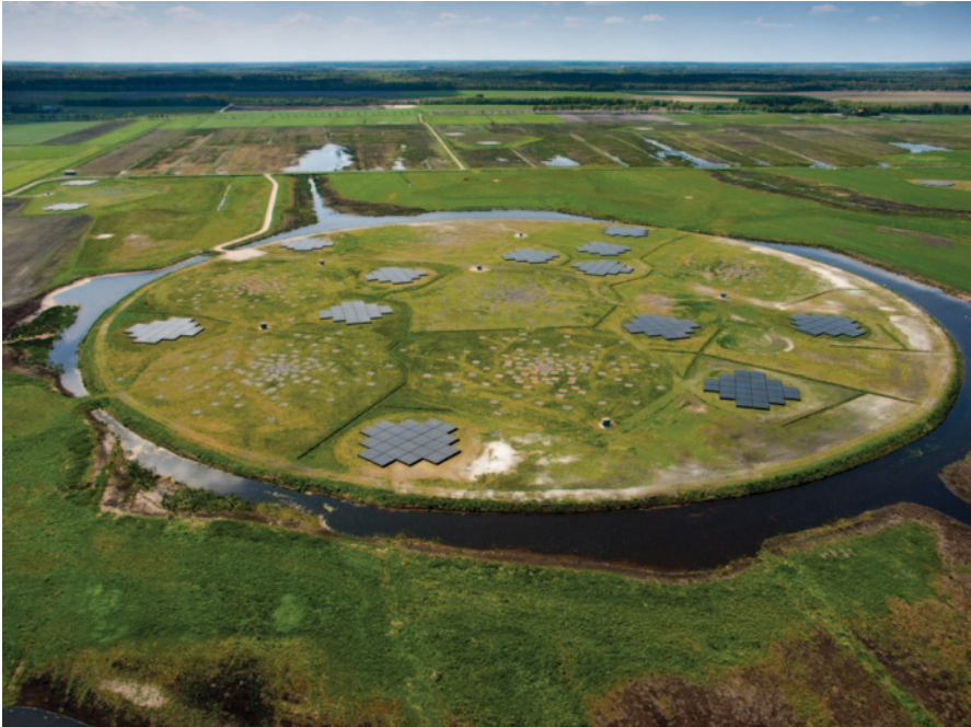
FIG. 15.9 A small section of the LOFAR radio telescope as constructed in the Netherlands. The tiles that define 6 of the separate antennas located on a raised segment of land called a super-terp, an artificial hill or raised area, to protect the equipment from possible flooding that may occur in this open countryside. (Credit: © Top-Foto, Assen)
