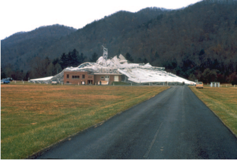
FIG. 18.1 R.I.P. The remains of the 300 ft radio telescope draped over its control building where the author had spent many enjoyable hours probing the nature of interstellar neutral hydrogen clouds in the ‘good old days’ when the dish was still functional. (Credit: NRAO/AUI/NSF and Richard Porcas)
