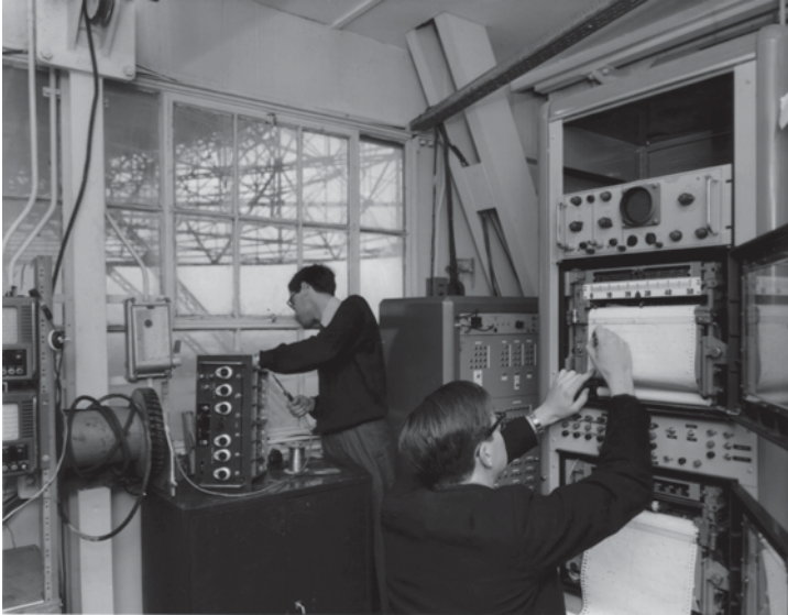
FIG. 19.1 Back in the early 1960s radio astronomical data were displayed on paper charts records. There were no computers to help you. In this carefully posed photo two earnest graduate students are in their lab 120 ft up in the Green Tower at of the 250 ft radio telescope at Jodrell Bank. On the left is Steve Gottesman examining a 6-channel unit used in studies of interstellar HI while on the right your author is earnestly marking paper charts. (Credit: Author)
