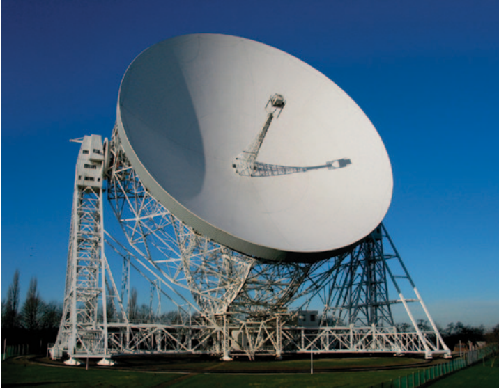
FIG. 1.1 The 250 ft diameter radio telescope at Jodrell Bank in Cheshire, England. This image shows the upgraded version known as the Lovell telescope. At the top of the tall mast in the center of the dish electronic amplifiers attached to a small antenna (or feed, as it is called) are housed in the box at the focal point of the dish. The amplified signal is fed down to a laboratory at ground level or, in the days that I was using the dish, to our lab in the tower at the right . (Photo courtesy of Nuffield Radio Astronomy Laboratories, University of Manchester)
