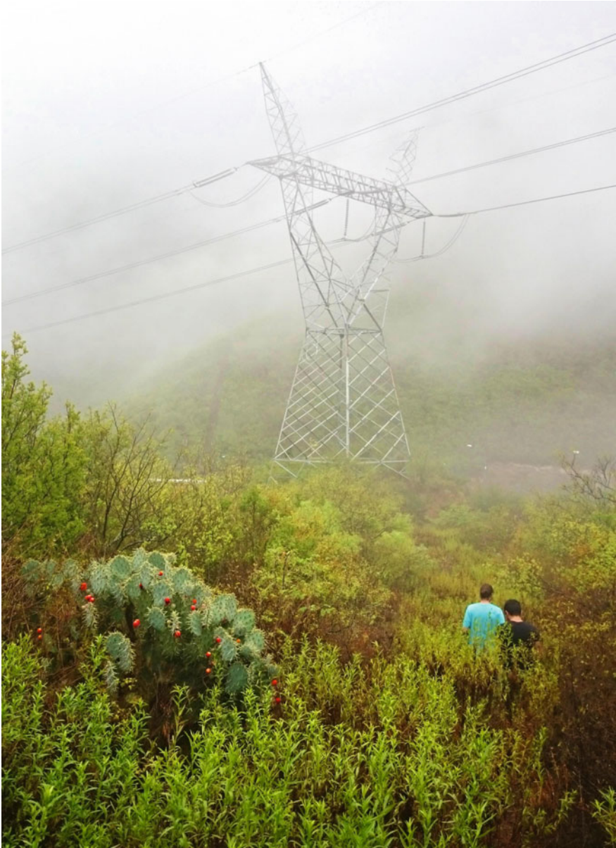
Fig. 8.1 Installation site of the tests for a Symbiotic Matorral project in the Sierra Madre Oriental: luxuriant matorral with large nopal laden with prickly pears, power-line pylon, and wanderers (photo rp)
