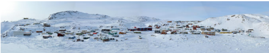
Fig. 4.8 Kimmirut, Canada, Arctic Adaptations: Nunavut at 15, Lateral Office 2014 (photo Billy Aakavak, courtesy of Lateral Office)
