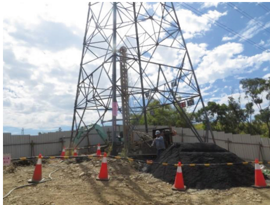
Fig. 8. Drilling machine positioning and drilling.
