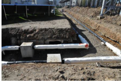
Fig. 3. Construction of the buried pre-insulated steel pipeline of sections 2 and 4
