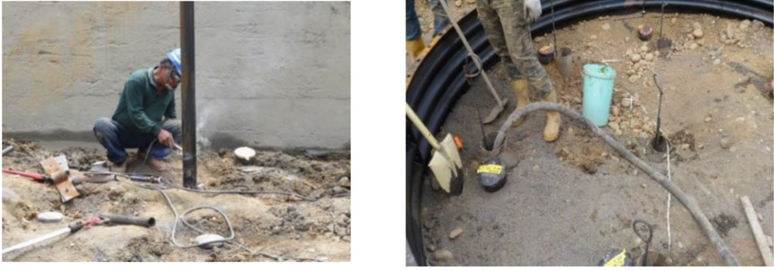
Fig. 9. Steel pipe spliced by welding and pile grouting
