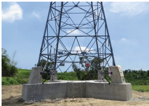
Fig. 11. Improvement of transmission tower foundation finished
