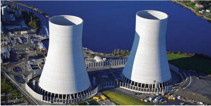
Fig. 2. Cooling Towers in Electric Industries
