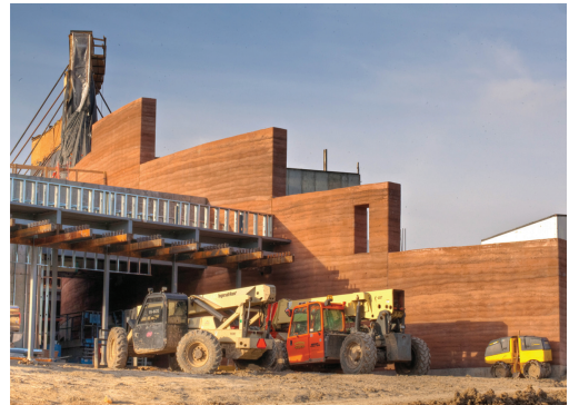
Figure 1. Loadbearing 51' tall SIREWALL.
