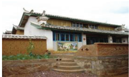
Figure 6. Demonstrate RE house in Yunnan.
