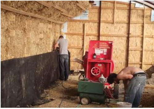
Figure 3. Rammed earth back wall.
