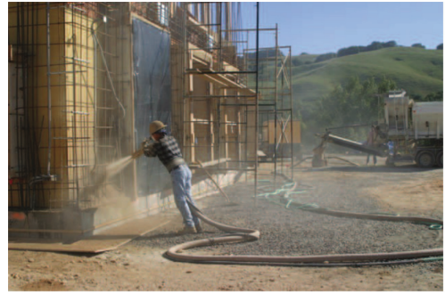
(a) work in progress
