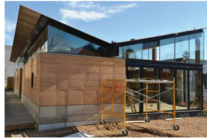
Figure 3. Photograph of Casa Sanitas under construction.
