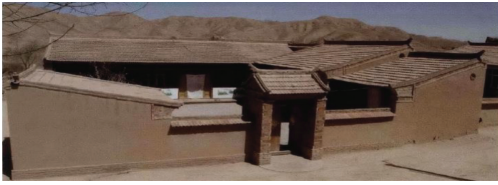
Figure 8. Demonstrate RE house in Gansu [10] .
