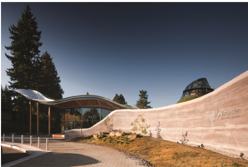
Figure 2. RE wall with 6670 psi (46 MPa) compressive strength.
