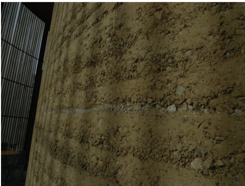
Figure 3. Berlin Chapel: unstabilised loadbearing rammed earth.
