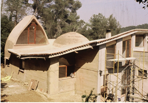
Figure 1. Rammed earth building in Collserola, Barcelona. Above: Prefabricated cement-cork stabilised earth ground floor slab undergoing laboratory testing.
