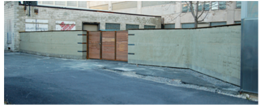
Figure 1. Raw rammed earth wall constructed on MIT campus (photo taken just after completion in 2005).
