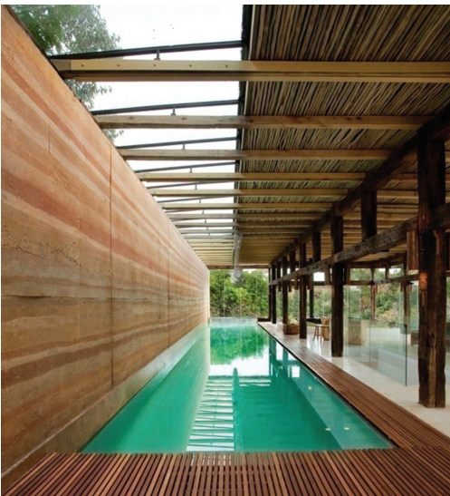
Figure 1. The Dalrymple pavilion under construction (Photo: Rech carstens architects).
