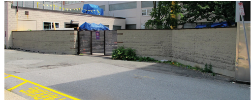
Figure 2. Rammed earth wall after 9 years of weathering (photo taken in 2014).
