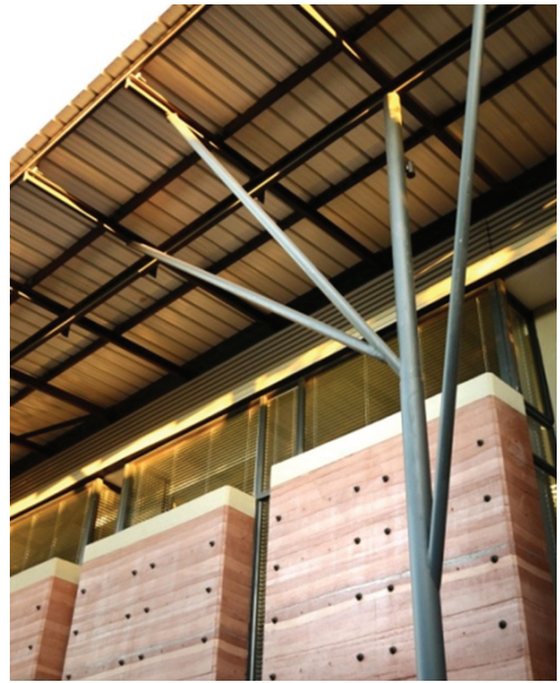
Figure 3. The roof and soil-cement walls of the SIOC-CDT office building. (Photo: Authors).
