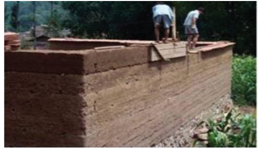
Figure 5. Rammed earth walls during construction.
