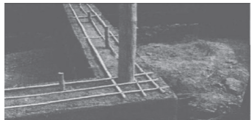
Figure 7. Traditional reinforcing in RE wall [11] .
