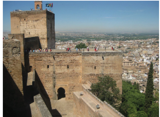
Figure 5. Rammed Earth Alhambra Palace in Spain.
