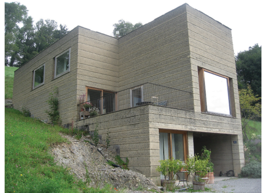
Figure 6. Rauch House: 3 storey loadbearing unstabilised RE.
