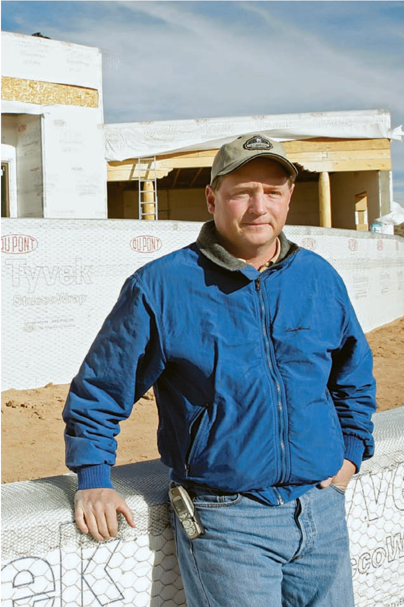
Home builder Norm Schreifels stands outside his green home that he is building in Corrales, New Mexico. Schreifels and other contractors are using better building techniques and environmentally friendly materials to create what industry insiders are describing as the future of homebuilding. AP Photo/Jake Schoellkopf
