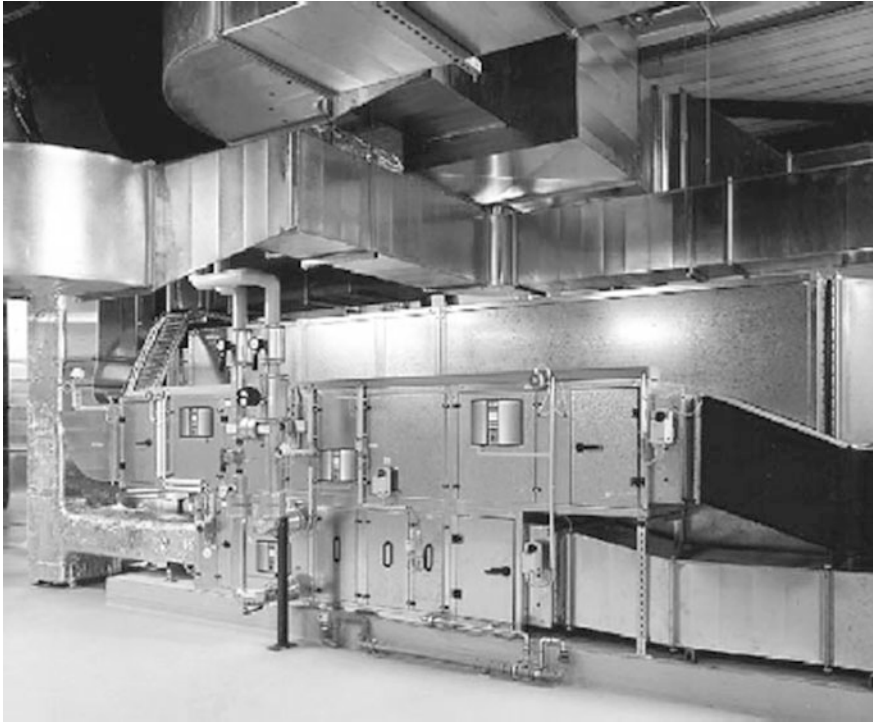
Fig. 1.1 A ventilation system in a commercial building [1]
