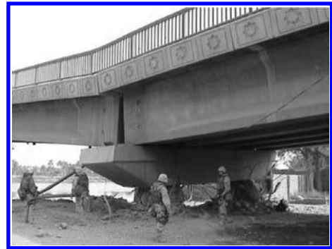
Figure 2. Bridge with piers destroyed by terrorists.
