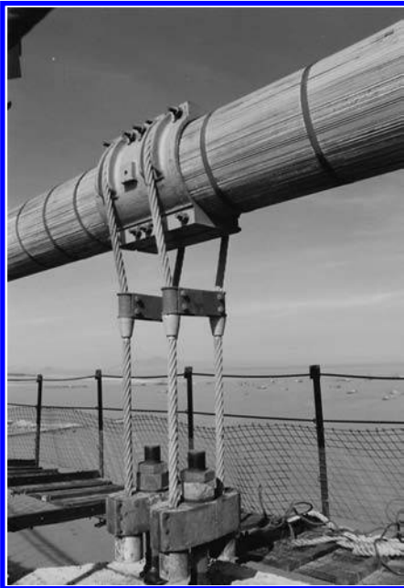
Figure 1. The Shantou Bay Bridge.
