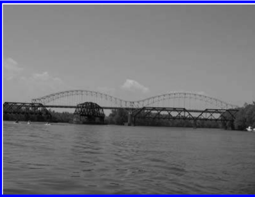
Figure 1. Arrigoni Bridge, Middletown, CT.
