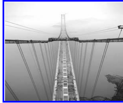
Figure 2. Xihoumen Bridge with 1650 m span.
