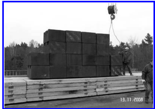
Figure 1. The technique of placing concrete slabs and steel blocks was used during test.
