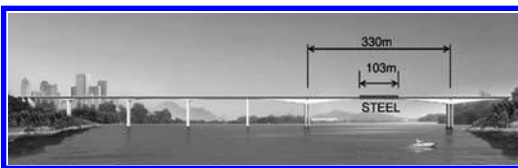
Figure 1. Shibanpo Bridge – Hybrid with concrete and steel box.
