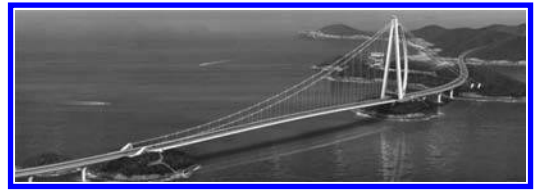
Figure 1. Aerial view of Dandeung bridge.
