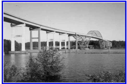
Figure 12. Port Mann Bridge, BC, Canada.
