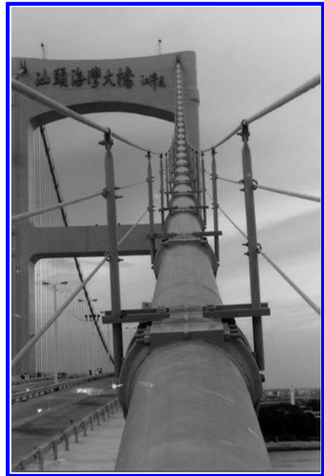
Figure 2. The Shantou Bay Bridge, China.
