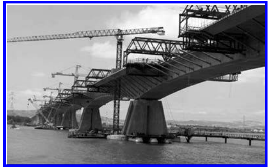
Figure 2. Bridge during construction.
