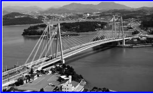
Figure 1. The 1st (right) and 2nd (left) Jindo Bridges.
