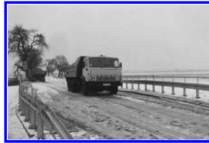
Figure 1. Wroclaw Bridge during passing the Kamaz vehicle on the object with speed of 30 km/h.
