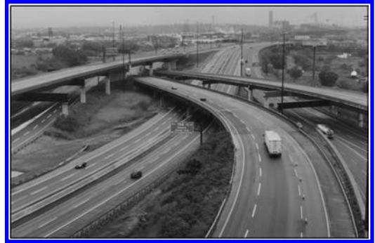
Figure 1. The New Jersey Turnpike varies from two 2-lane roadways to six 3-lane roadways by Newark Airport, with dual-dual roadways over a 32 mile length through the busiest zone.
