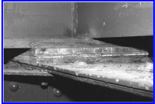
Figure 9. Shims between new floor beam and existing girder.
