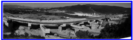
Figure 1. View of the bridge.
