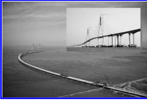
Figure 1. View of Incheon Bridge linking Youngjong Island and the mainland (total length: 12.3 km, central span: 800 m, design service life: 100 years).
