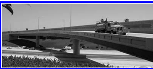
Figure 1. West street on-ramp.
