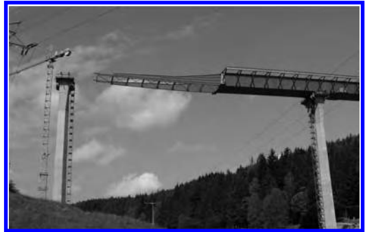
Figure 1. Composite bridge “Dambachtal”.
