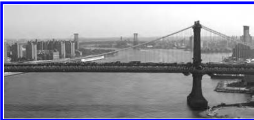
Figure 1. Manhattan (foreground) and Williamsburg (background) Bridges.
