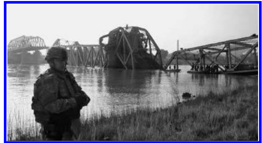
Figure 1. Bridge destroyed terrorists.
