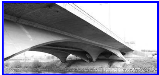
Figure 1. View of the Erdberger Bridge.
