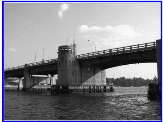
Figure 1. Oceanic Bridge Bascule Span.
