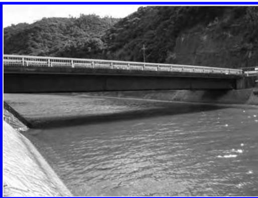
Photo 1. Panorama bridge (Okinawa in Japan).
