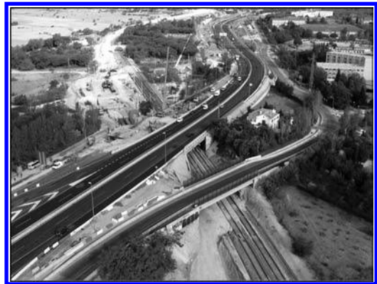
Figure 3. The new bridge E-2 and to the bridge E-3A/3B in construction.
