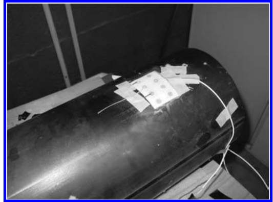
Figure 1. Flexible piezoelectric paint sensor mounted on a circular hollow section (CHS) steel member.
