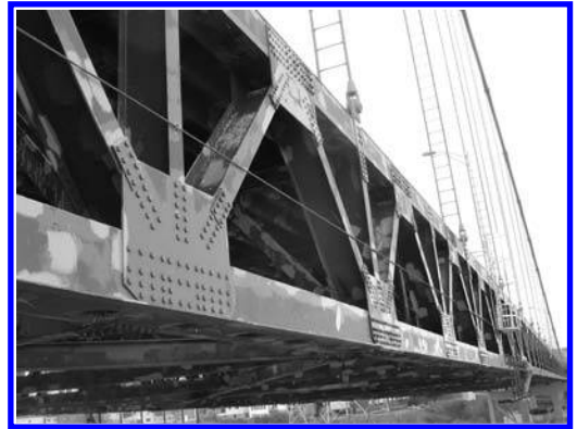
Figure 3. Stiffening truss, MacKay Bridge.
