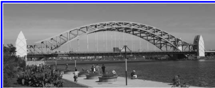
Figure 1. Guotai Bridge in Tianjin.
