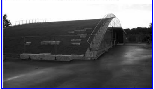
A new gymnasium (Reisenfeld, Austria)
