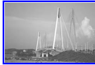
Figure 1. The 1st (right) and 2nd (left) Jindo Bridges.
