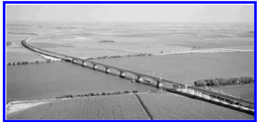
Figure 1. Aerial view of the bridge.
