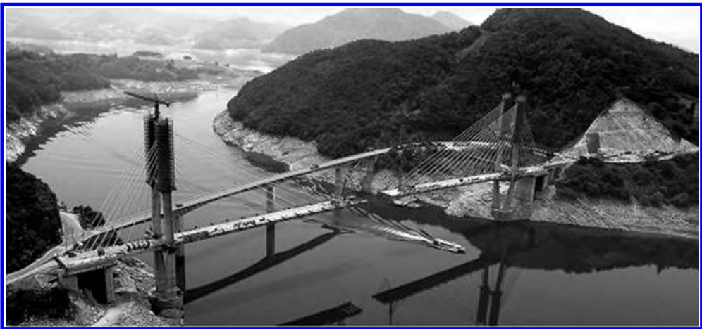
Figure 1. A view of Cheong Poong Bridge.
