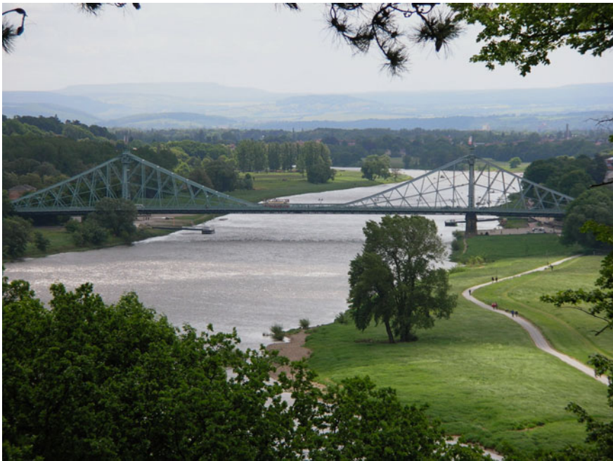
Fig. 7.2 Blue wonder bridge in Dresden (Picture D. Proske)
