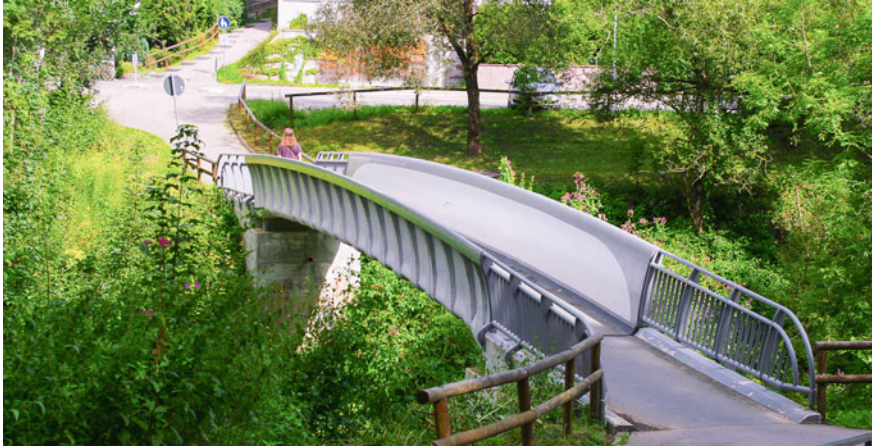
Fig. 6.46 Textile reinforced concrete bridge in Germany (Picture H. Michler)
