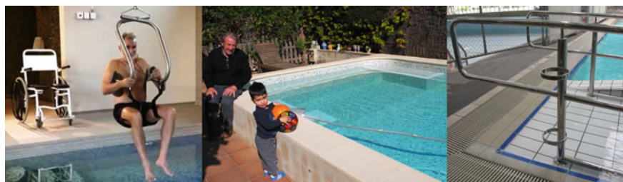
Fig. 1 Ceiling-mounted pool lift (left); Private pool in Spain with transfer bed (centre); Public pool in Australia with cane holder (right) (credits: 1. H.-M.; 2. M. B.-E.; 3. F. D.)
