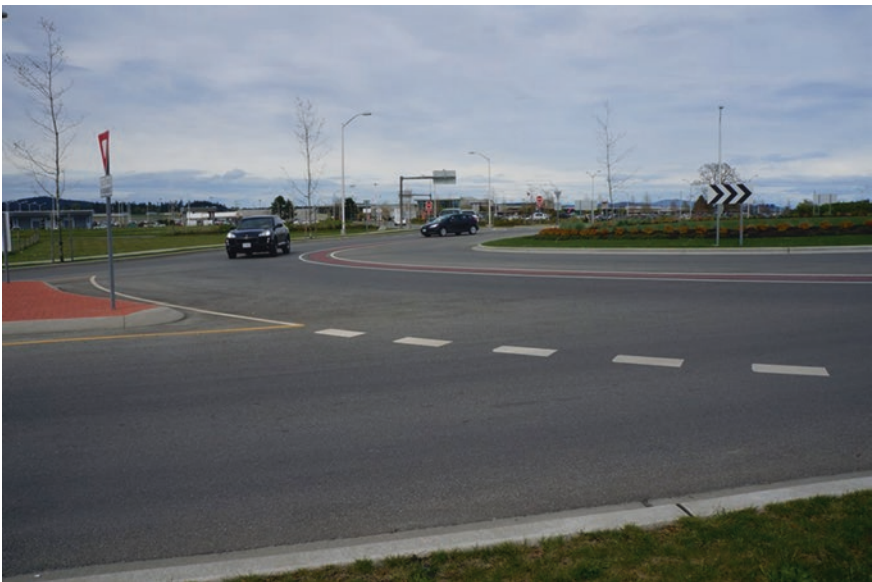
Fig. 3.53 Circulatory carriageway at the first Canadian turbo-roundabout
