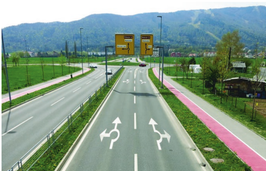
Fig. 4.21 Special form of signposts and arrow-markings at a turbo-roundabout; Slovenia
