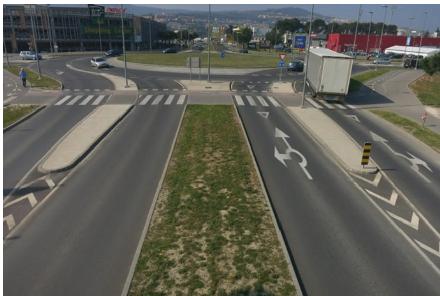
Fig. 7.5 Separation of entry and exit lanes with separating islands at pedestrians' and cyclists crossings; Koper, Slovenia
