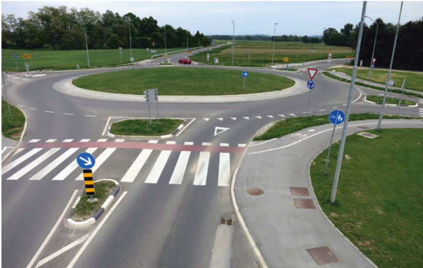
Fig. 2.8 Typical Slovenian one-lane roundabout
