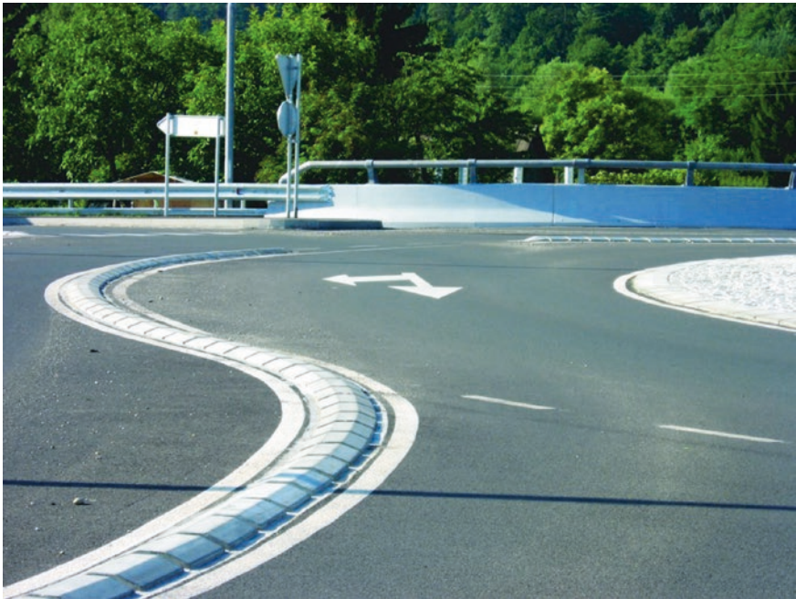
Fig. 4.20 Divided curbs (delineators) on a turbo-roundabout's circulatory carriageway
