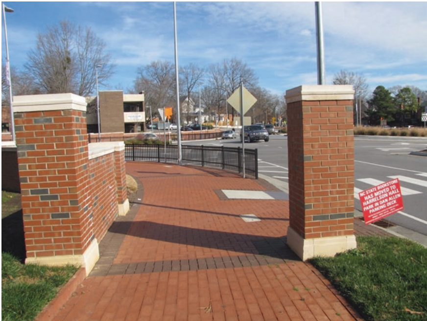
Fig. 7.14 Tactile ground surface indicators; Raleigh, North Carolina, USA
