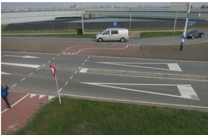
Fig. 7.6 Deviated position of the cycle crossing at the entry and exit; near Den Haag, The Netherlands
