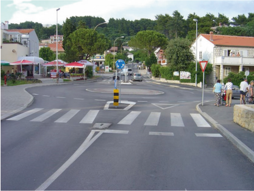
Fig. 2.40 Three arm double mini-roundabout with short central link road; island Rab, Croatia
