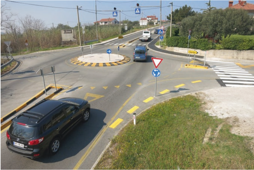
Fig. 4.4 An assembly roundabout constructed from prefabricated rubber curbs, Izola, Slovenia
