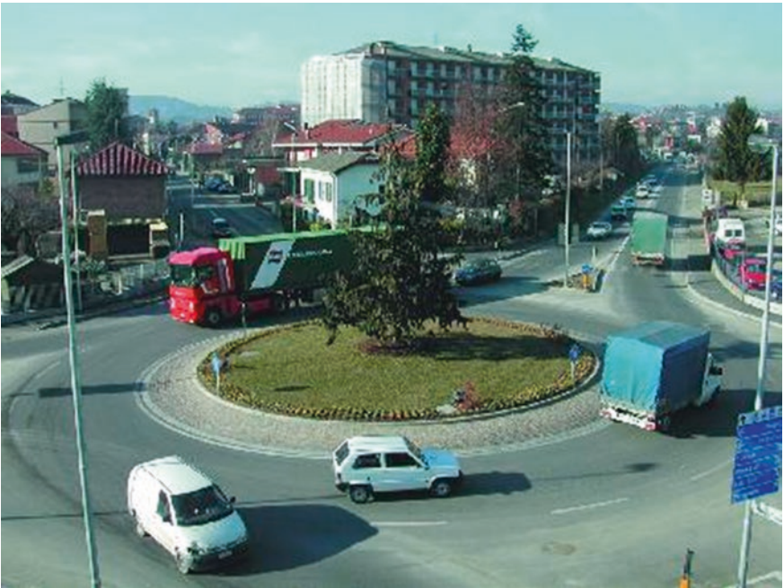
Fig. 3.30 Actual example of Italian compact roundabout
