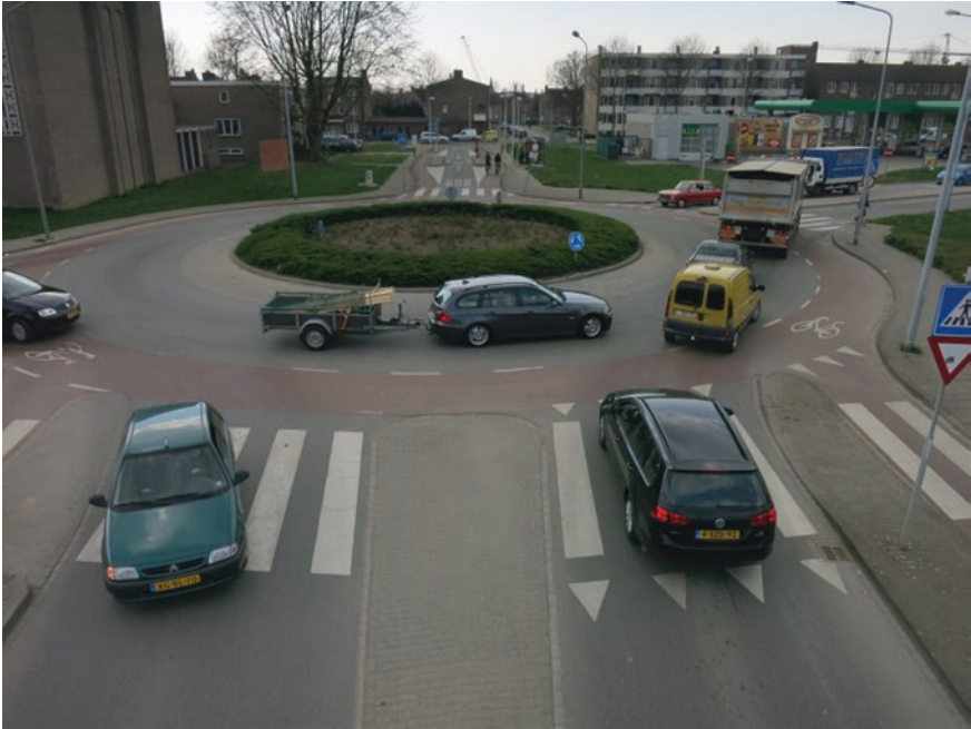
Fig. 3.13 Parallel cycling traffic management along the outer roundabout edge; Maastricht, The Netherlands
