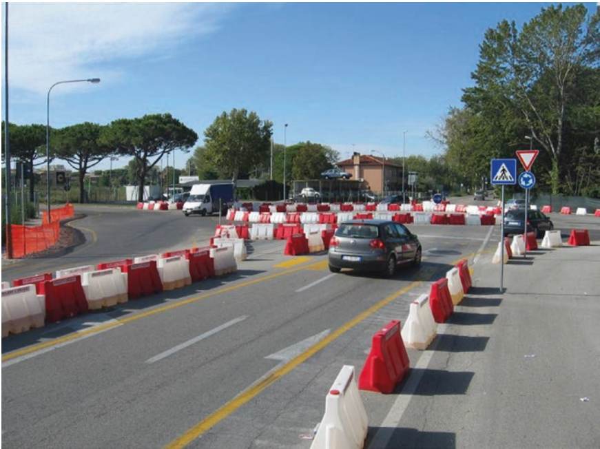
Fig. 4.5 Assembly roundabout, constructed from plastic protective barriers, San Donà di Piave, Italy
