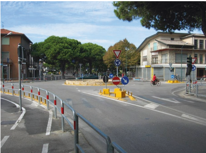
Fig. 4.2 Turned off traffic lights at an assembly roundabout on an existing traffic lighted intersection; Jesolo–Punta Sabbioni, Italy
