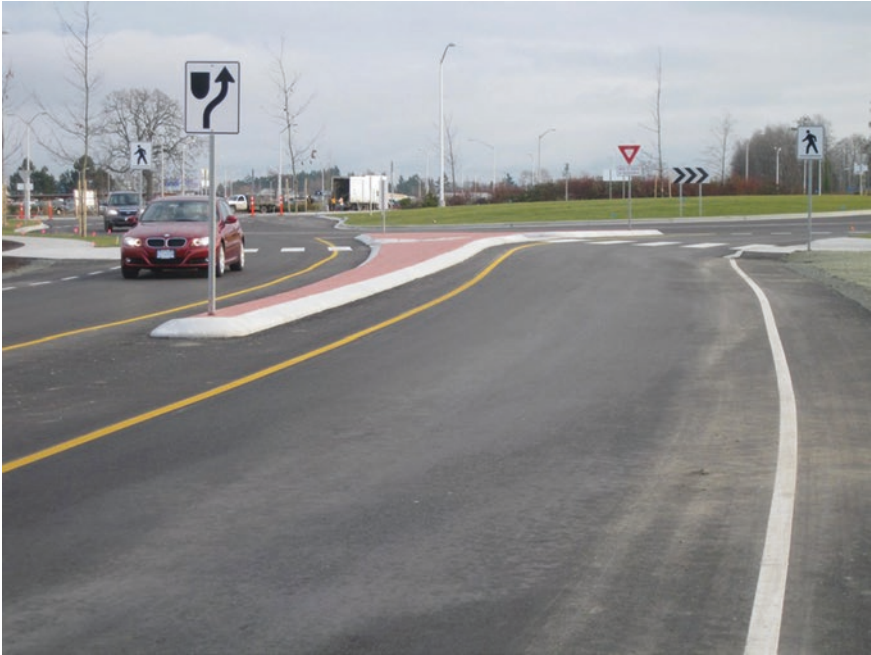
Fig. 3.54 Splitter island and traffic signs
