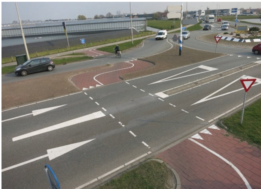
Fig. 7.7 Design of deviated position of the crossing; near Den Haag, The Netherlands
