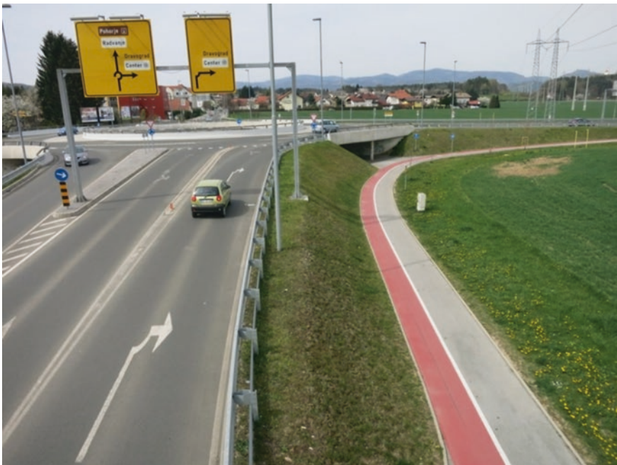
Fig. 7.11 An underpass at a turbo-roundabout on a main town arterial; Maribor, Slovenia
