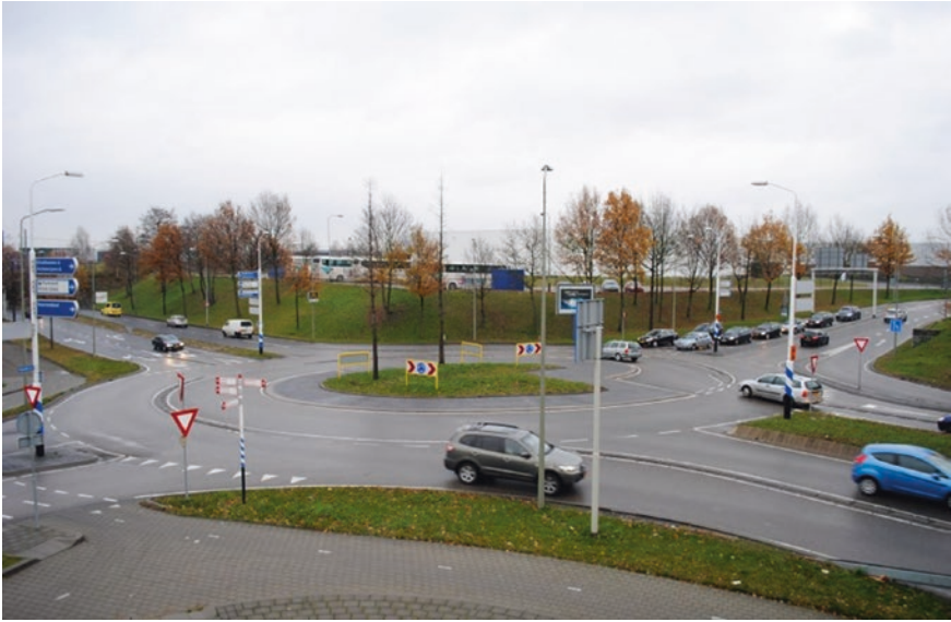
Fig. 4.18 The Netherlands' typical turbo roundabout
