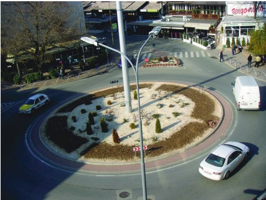
Fig. 3.37 Small roundabout, Skopje
