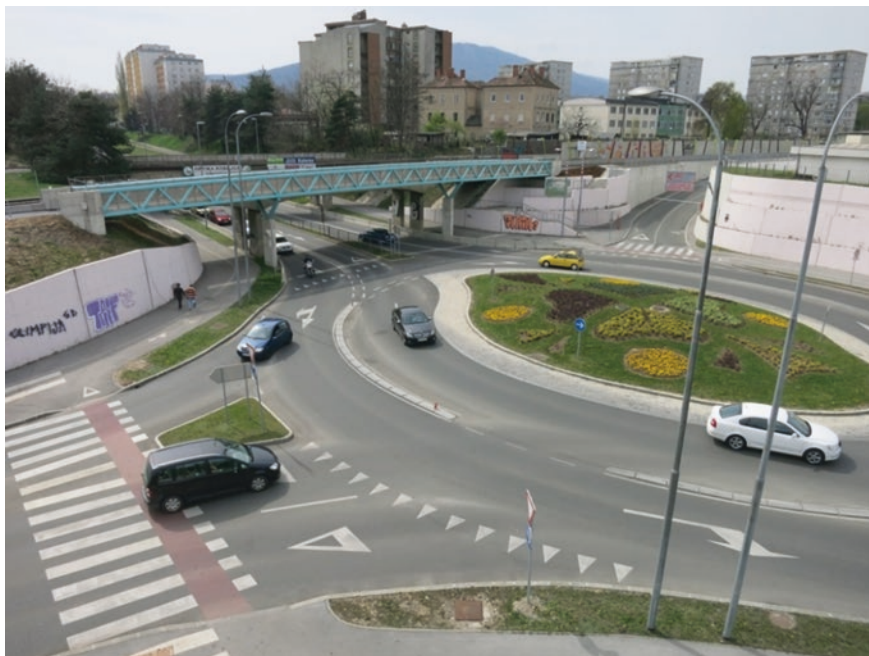
Fig. 7.12 An overpass at a turbo-roundabout on a main town arterial; Maribor, Slovenia
