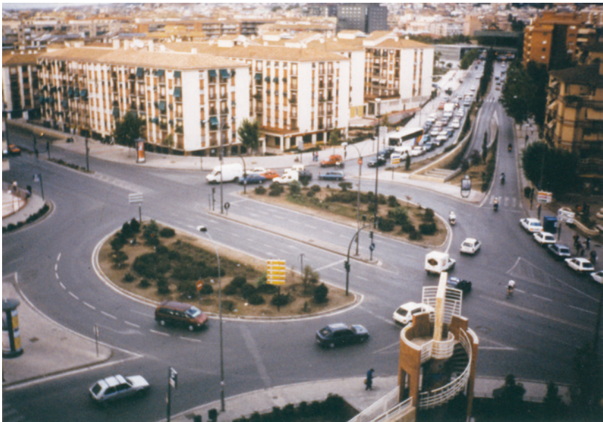
Fig. 2.51 Two-level hamburger roundabout; Barcelona, Spain
