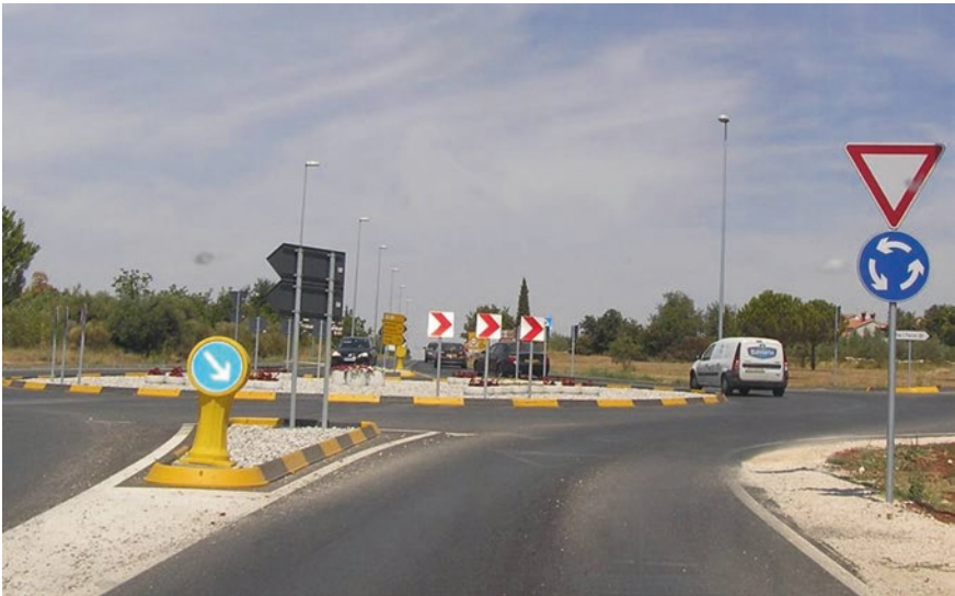
Fig. 3.35 Assembled roundabout, Tar-Vabriga, Croatia
