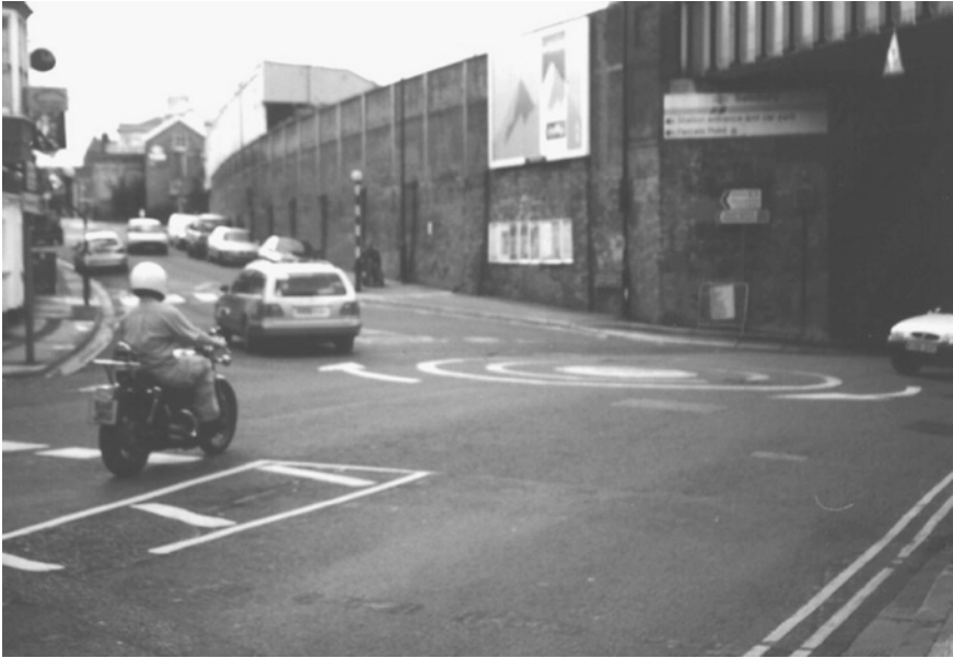
Fig. 2.27 The origin of the mini roundabout, still widely used; Salisbury, the UK
