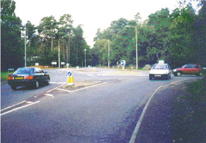
Fig. 2.38 Double mini-roundabout with short central link road; suburb of Coventry, the UK
