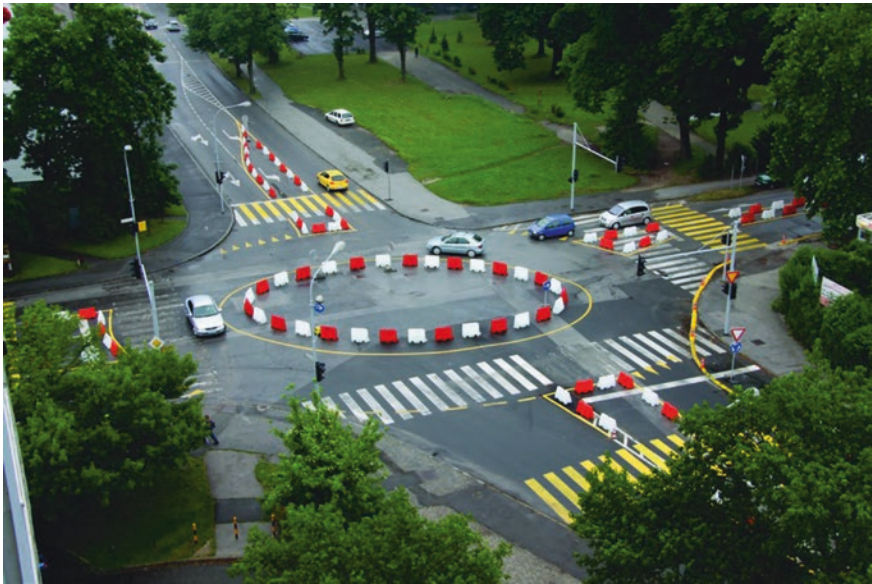
Fig. 4.1 An assembly roundabout—under construction; Maribor, Slovenia
