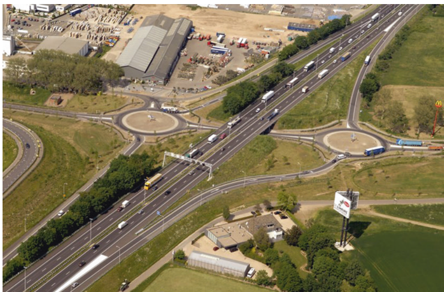
Fig. 2.43 Dumb-bell roundabout on motorway; The Netherlands
