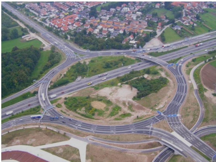
Fig. 4.28 Traffic-lighted turbo-roundabout; Ljubljana
