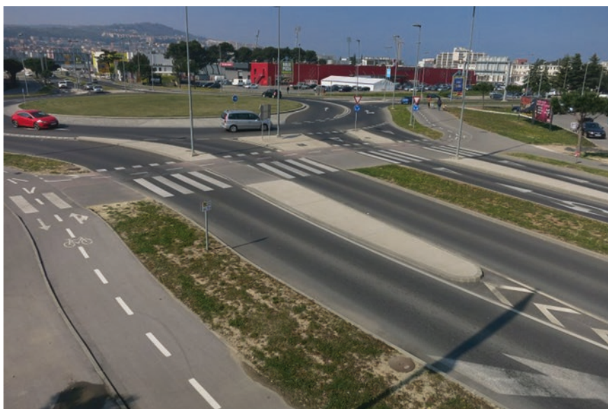
Fig. 4.30 Intermediate splitter lane between two driving lanes on entrance and exit on Slovenian turbo-roundabout in urban area
