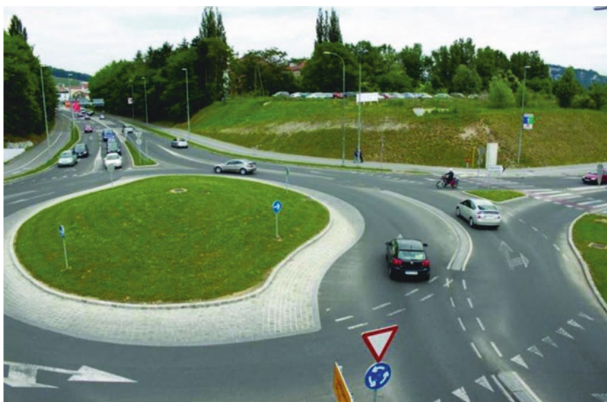
Fig. 4.29 Divided element (delineator) without a “peak” on Slovenian turbo-roundabout
