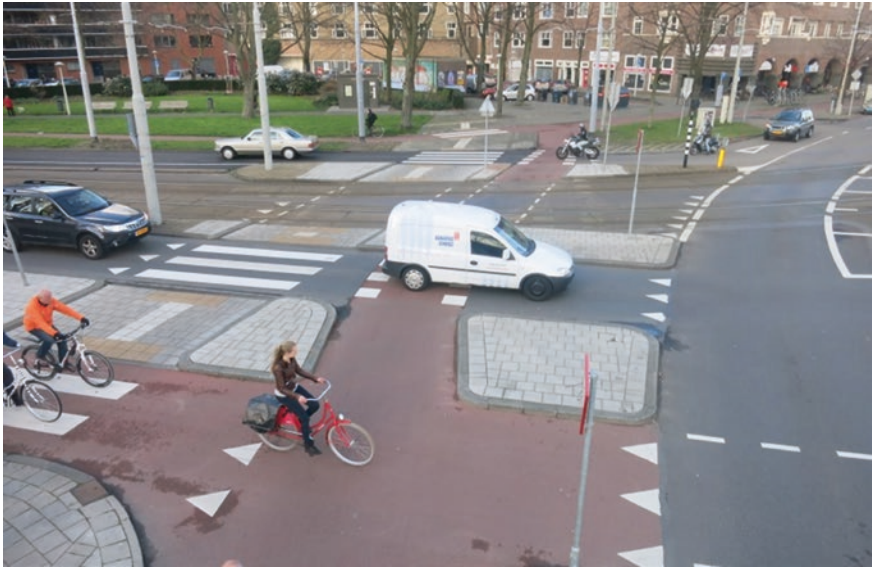
Fig. 7.13 Tactile ground surface indicators or detectable warning surfaces are installed along the curb and splitter island at a pedestrian crossing; Amsterdam, The Netherlands
