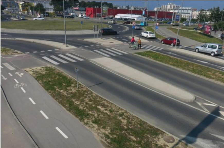
Fig. 7.3 Separation of entry and exit lanes with separating islands at pedestrians' and cyclists crossing; Koper, Slovenia
