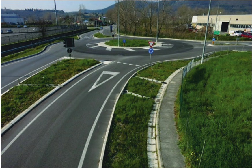
Fig. 3.29 Actual example of Italian one-lane roundabout, Trieste
