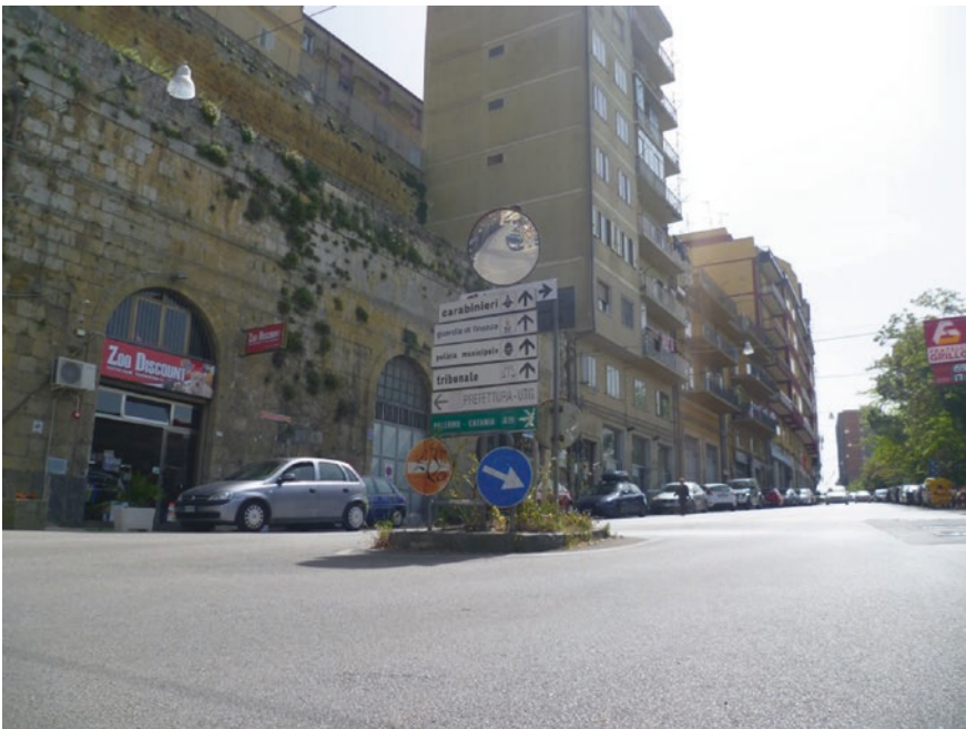
Fig. 4.13 Traffic calming circle; Enna, Italy
