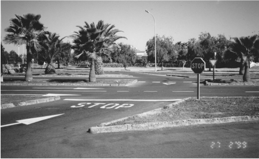
Fig. 2.48 Stop and yield signs on the crossing with a straight-through section of carriageway
