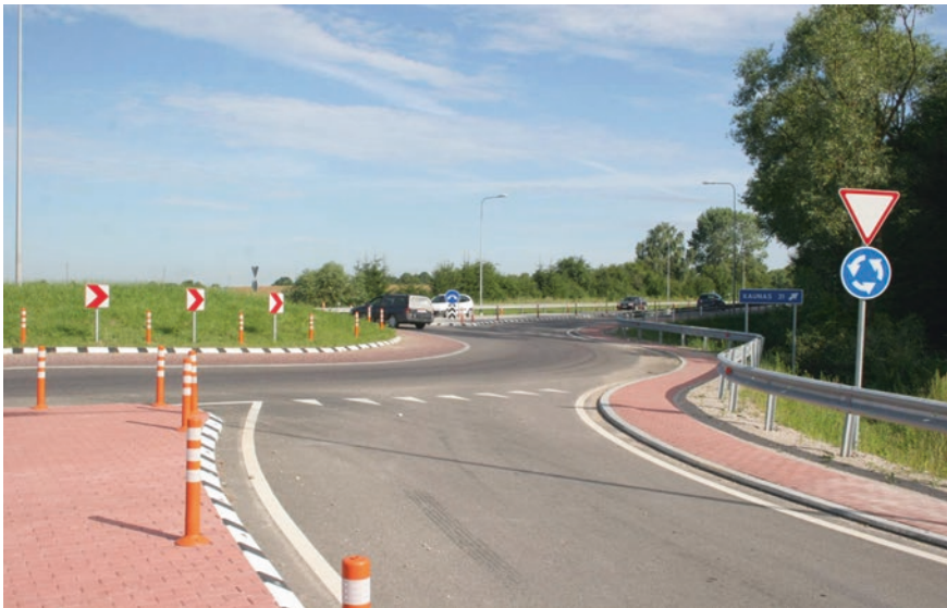
Fig. 3.40 One of the first Lithuanian one-lane roundabout, City of Prienai
