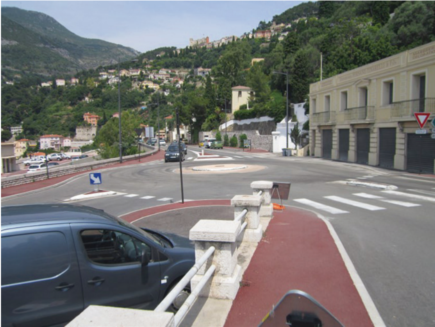
Fig. 2.33 Domed circle and curbed splitter islands; suburb of Nice
