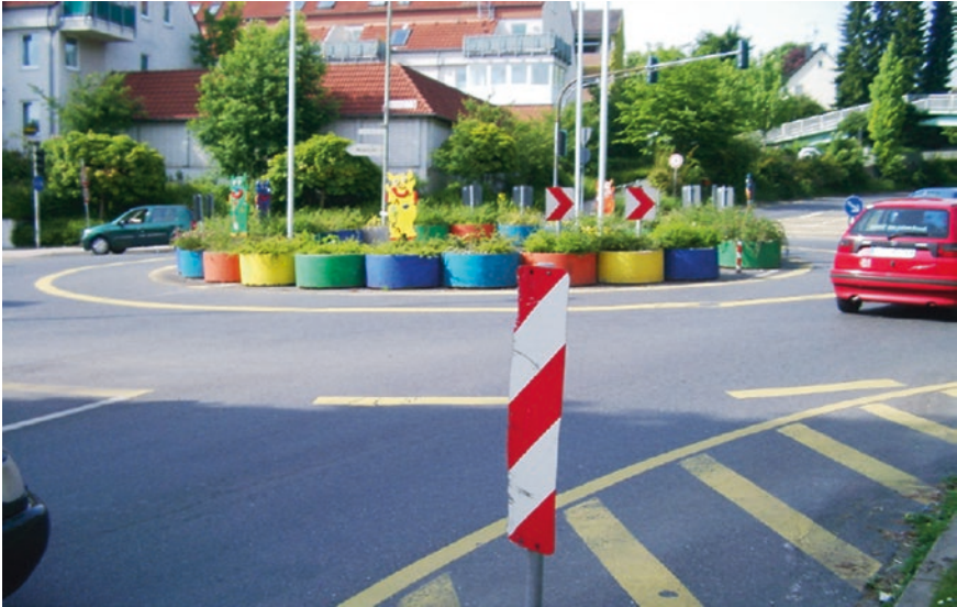
Fig. 4.6 Central island of an assembly roundabout, constructed from concrete sewage pipes, Wülfrath, Germany [2]
