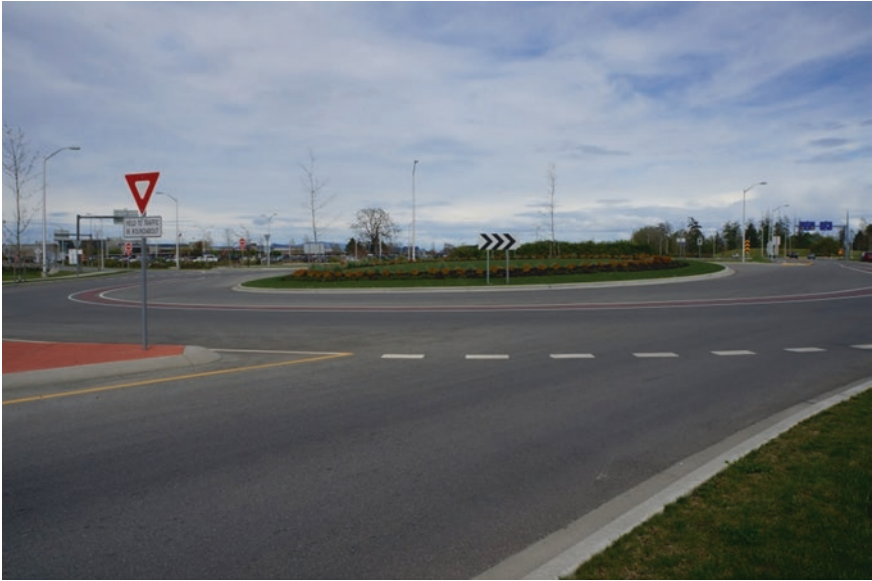
Fig. 3.52 The first Canadian turbo-roundabout, approach; Victoria international airport, Victoria, British Columbia
