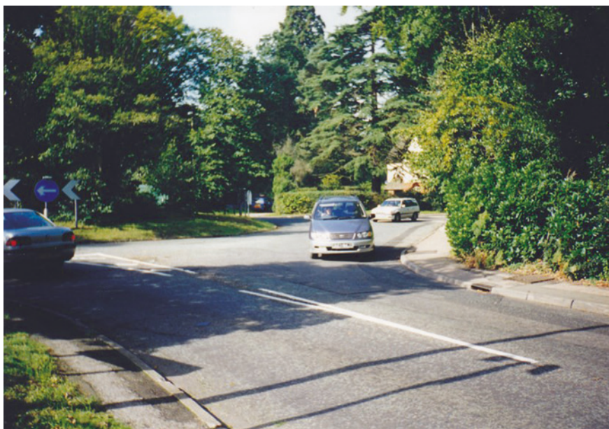
Fig. 2.6 Square roundabout with square island; Coventry
