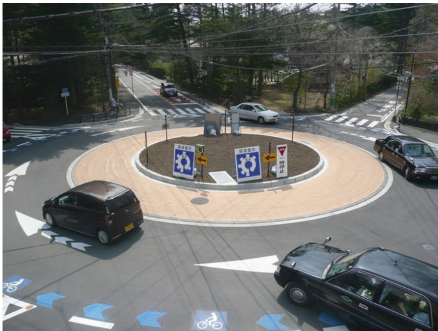
Fig. 3.56 A six-leg roundabout improved from non-signalized intersection through a pilot study; Karuizawa Town
