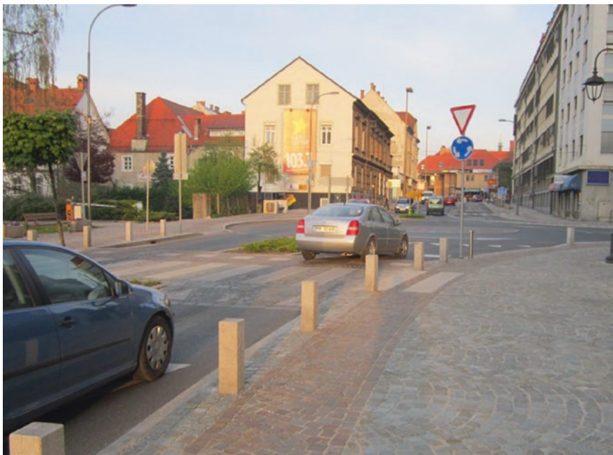
Fig. 7.10 Raised platform with a crosswalk and LED lights in front of a mini-roundabout; Maribor, Slovenia
