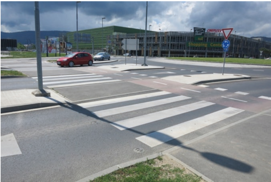
Fig. 7.4 Separation of entry and exit lanes with separating islands at pedestrians' and cyclists crossing; Koper, Slovenia
