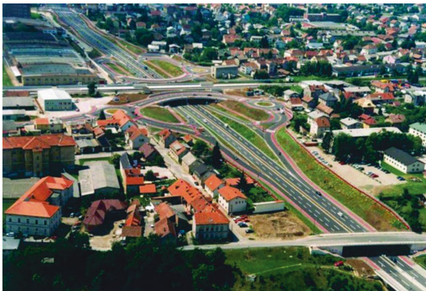
Fig. 2.44 Dumb-bell roundabouts on motorway; Slovenia
