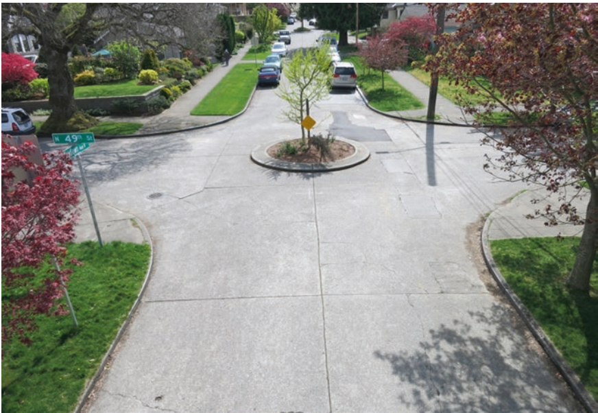
Fig. 3.45 Landscaped traffic calming circle (neighborhood traffic circle); Seattle, Washington
