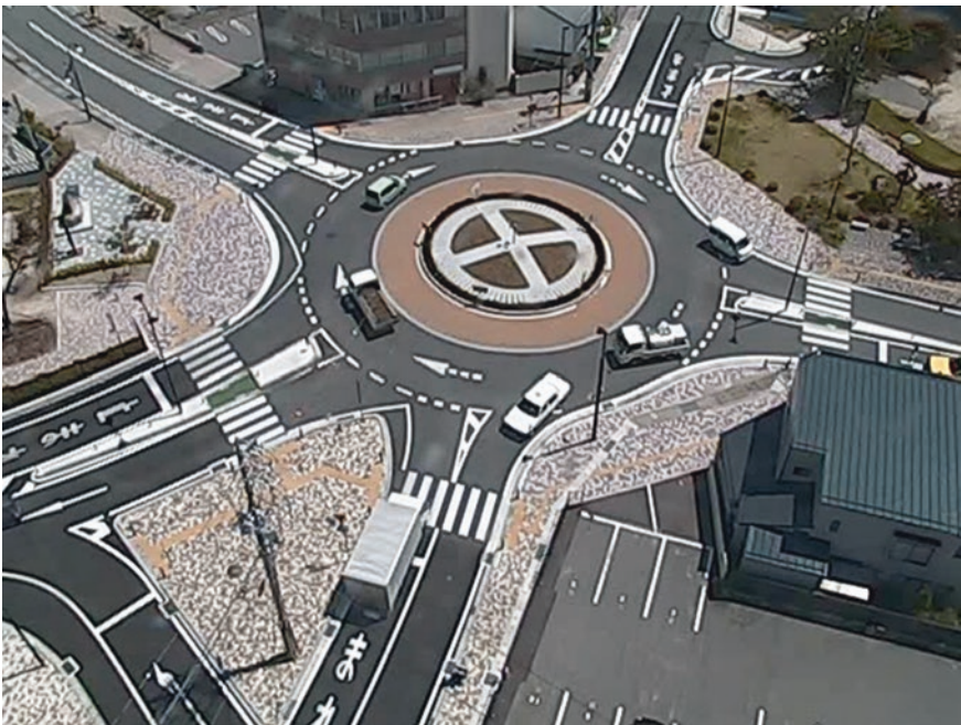
Fig. 3.55 The first Japanese example of roundabout improved from signalized intersection; Iida City, 2013
