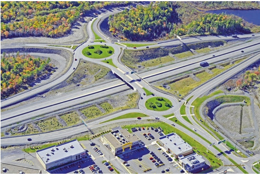
Fig. 3.51 Well landscaped Canadian dumb-bell roundabout
