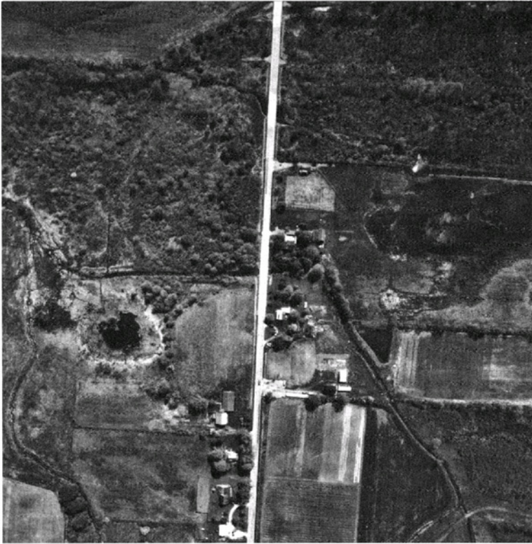
Figure 5.19. Low altitude aerial photographs are acquired to make large-scale topographic maps for engineering of highways. The state department of transportation or like agency archives these photos, which supplied fine detail on wetlands such as these in Trumbull County, Ohio.
