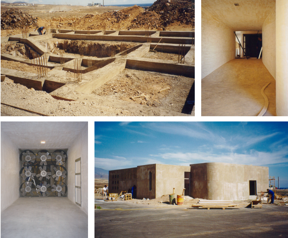
Figure 15. Photographic sequence of the construction of the ITER Low Speed Wind Tunnel. The top left picture shows the foundations, the top right the contraction, the bottom left the power plant and the bottom right a view from the outside almost at the end of the construction.
