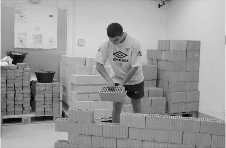
Fig. 4 – Standardised workstation for bricklaying.
