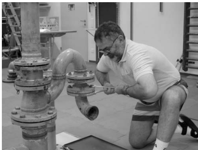
Fig. 8 – For work simulation training, inexpensive devices can be used (assembly system of old tubes).
