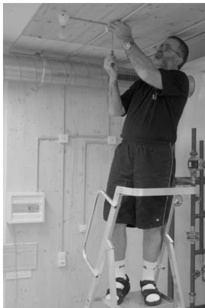
Fig. 9 – Work station for electro-installation.
