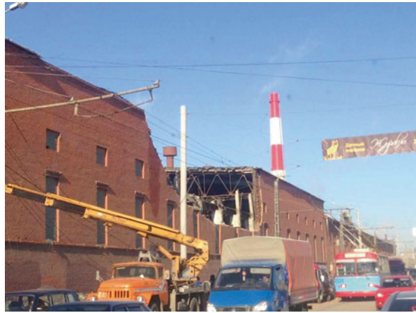
Fig. 1 Asteroid explosion collapses Chelyabinsk warehouse (Posper A. Creative Commons License via Wikimedia Commons)
