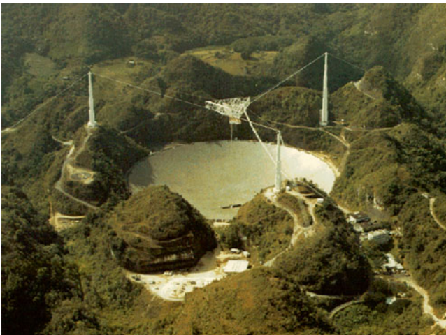
Fig. 17 Arecibo radio telescope, 1 km diameter. It mainly points via the Earth's rotation, but the receiver suspended over it can be moved back and forth a few degrees (National Astronomy and Ionosphere Center, Cornell U., NSF [Public domain], via Wikimedia Commons)
