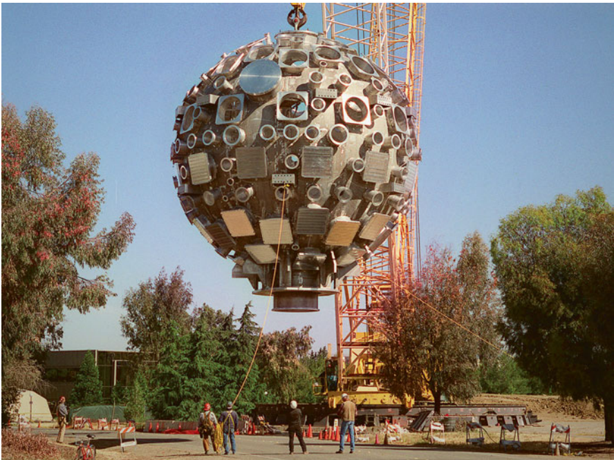
Fig. 22 NIF target chamber being delivered (US Department of Energy—Public Domain)
