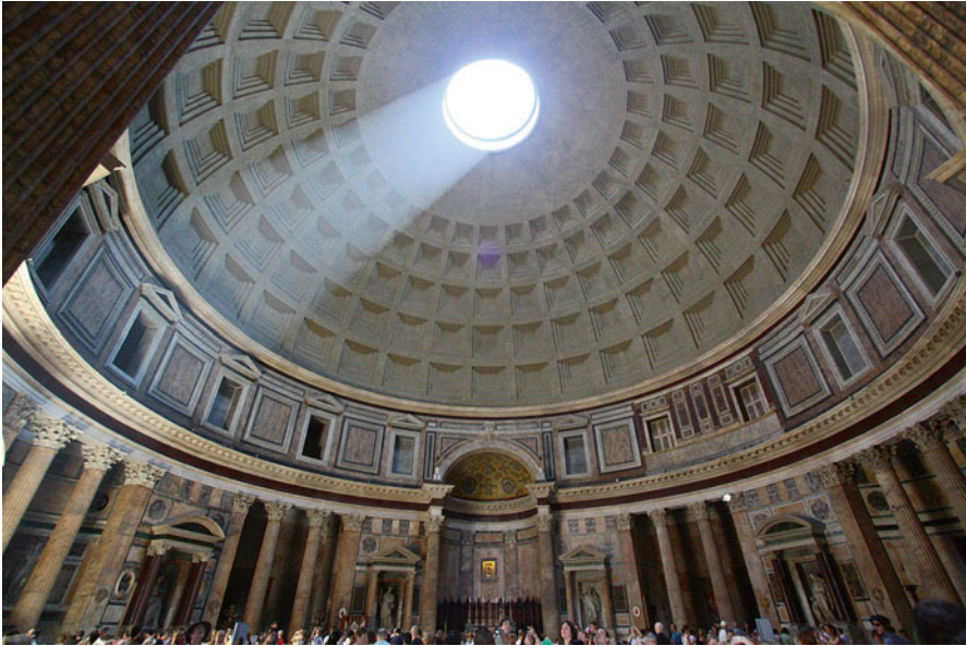
Fig. 1 Roman concrete 1900 years later: The Pantheon (125 A.D.), the largest unreinforced concrete dome in the world (Rich J. Heath, public domain)
