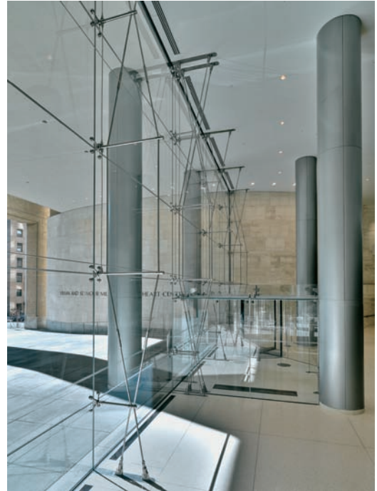
FIGURE 11.3 The entry wall cable truss system establishes the vocabulary for the truss system used for the climate wall. Note the glass box vestibule in the middle ground.
