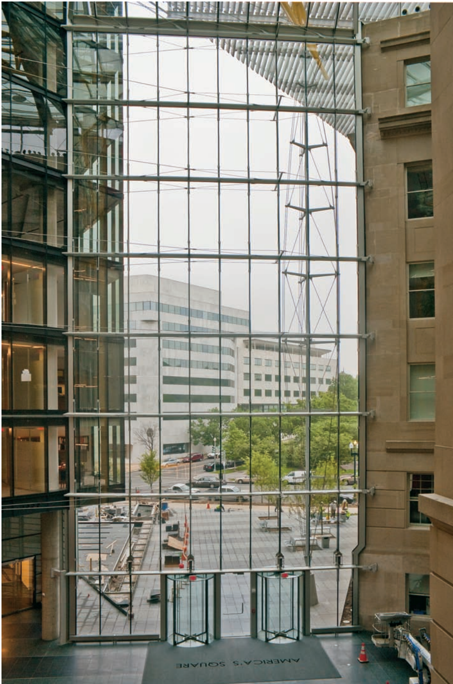
FIGURE 10.4 The glass entry wall is suspended from an overhead beam that is cantilevered from the new building structure on the left, so that it applies only minimal loads to the older building on the right.
