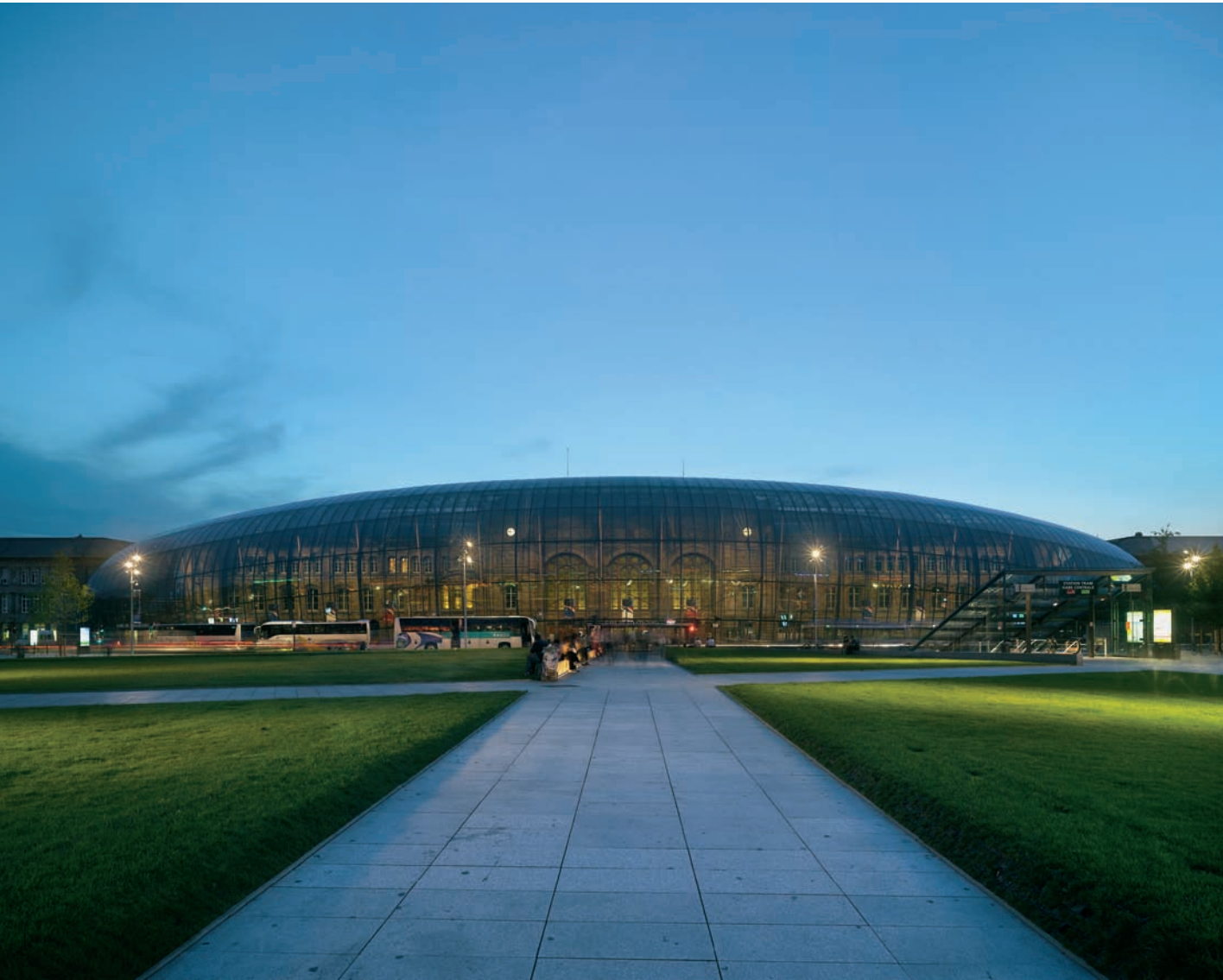
FIGURE 12.1 The stone facade of the old station glows behind the transparent glass shell of the new entrance enclosure.
