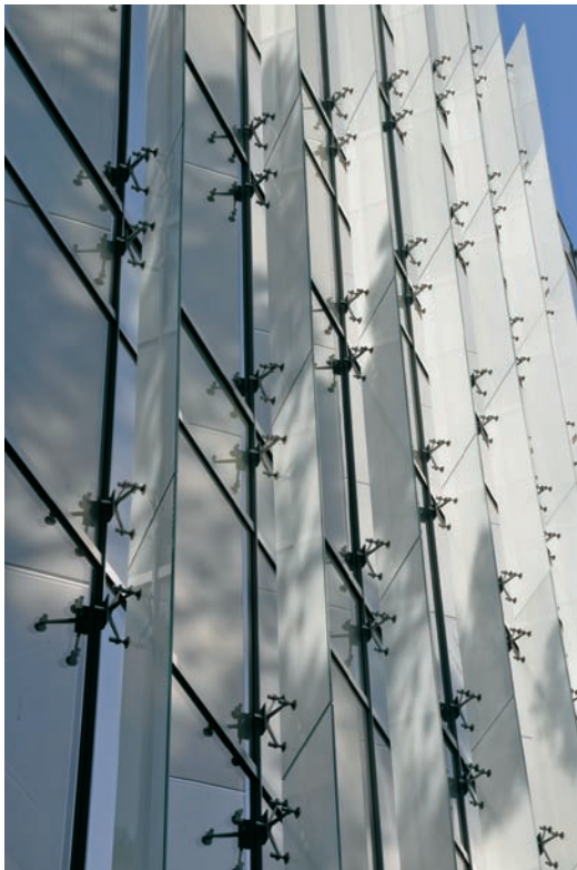
FIGURE 13.7 The laminated fins are point-fixed from cast spiders supported from the curtain wall framing.
