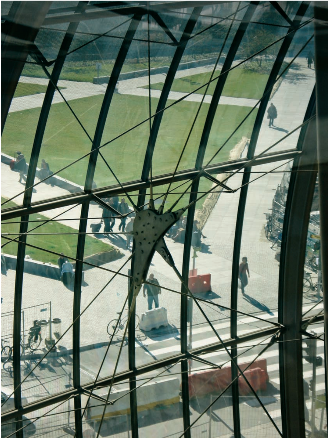
FIGURE 12.5 All elements of the structure can be seen in this view except the columns just outside the old facade.
