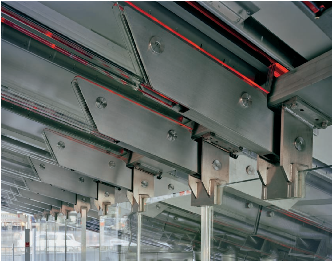
FIGURE 6.5 Finished photograph of the midwall connection.
