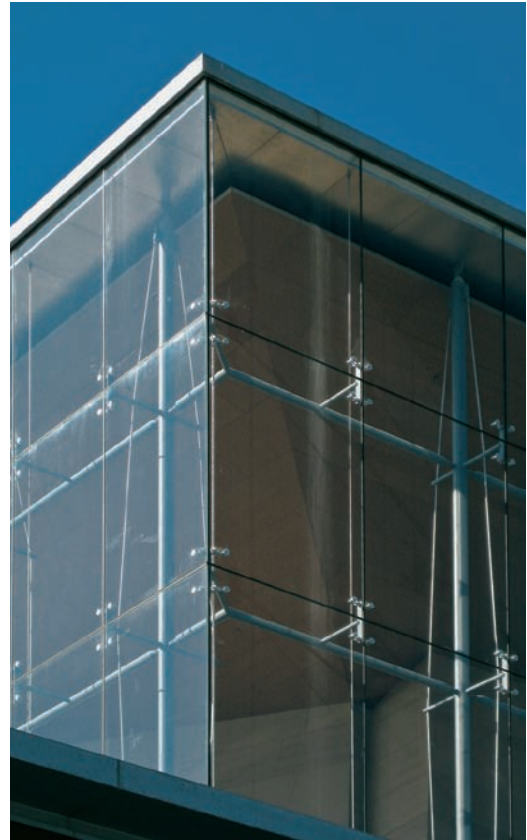
FIGURE 9.6 This exterior view of the corner condition reveals the minimal structure.
