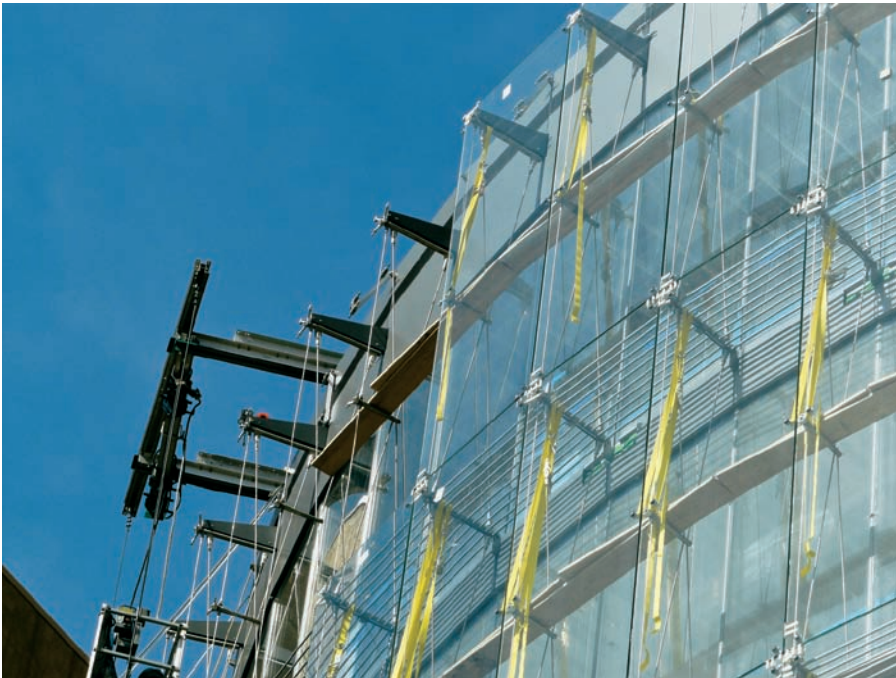
FIGURE 11.18 Glass installation in progress on the climate wall.
