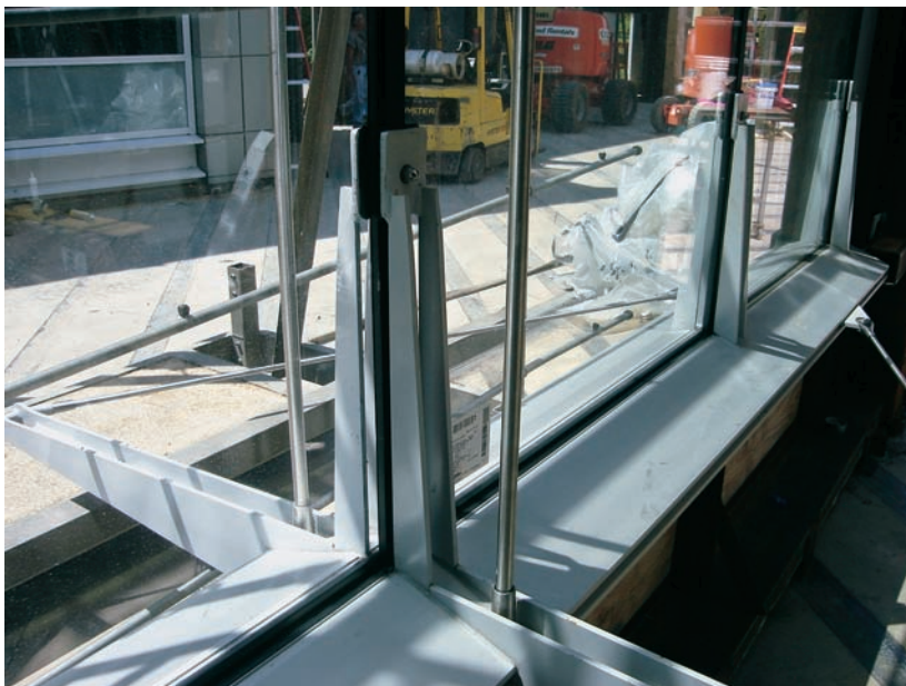
FIGURE 10.14 A kipper truss forms part of the mockup.
