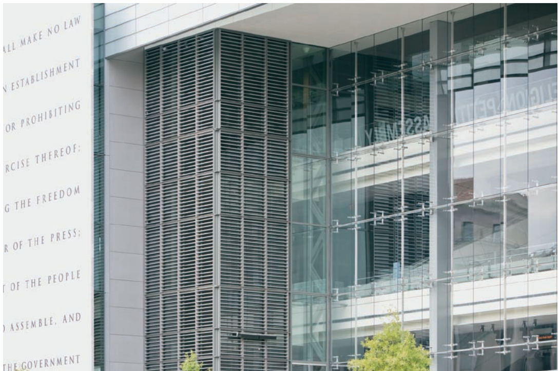
FIGURE 15.2 The highly transparent cable wall is a predominant architectural feature.
