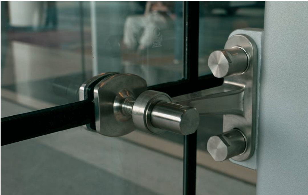
FIGURE 2.10 A point-fixed clamped glass system requires no perforation in the glass. A blade penetrates through the silicone joint to support the glass dead load. An exterior cap plate secures to the blade to fix the glass.
