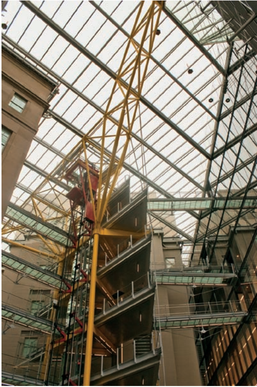
FIGURE 10.8 The skylight framing is supported by perimeter building structure and the dramatic yellow tree truss that houses the central circulation.
