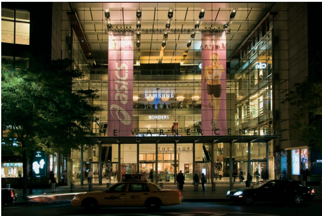
FIGURE 5.5 Time Warner Center, New York, 2004, Skidmore Owings & Merrill. This flat cable net is 150 ft (46 m) tall and 90 ft (27 m) wide.
