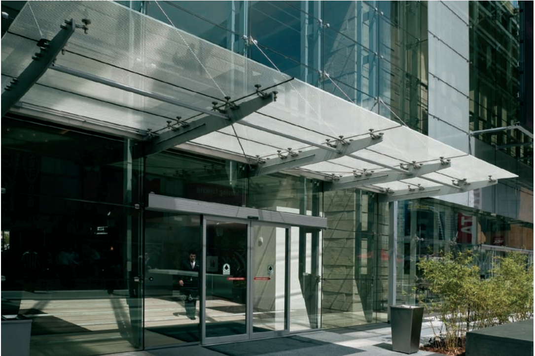
FIGURE 7.9 A 20 ft (6.1 m) canopy is supported by the south facade truss system, with cable tiebacks penetrating through slots in the glass membrane.
