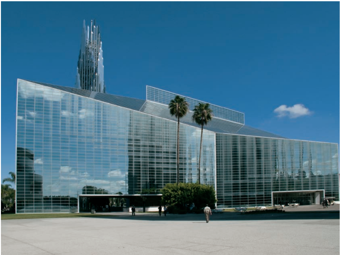
FIGURE 4.2 The Crystal Cathedral (1980), Garden Grove, California, is a space frame structure clad in a curtain wall system incorporating reflective glass. Operable vents provide natural ventilation.
