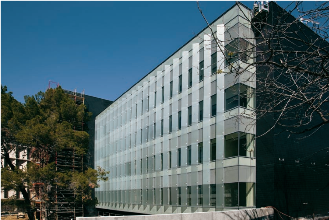
FIGURE 13.2 The west facade is glazed with a simple curtain wall system but incorporates a novel glass fin shading element.
