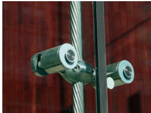
FIGURE 16.9 Exterior view of the intermediary point fixing.
