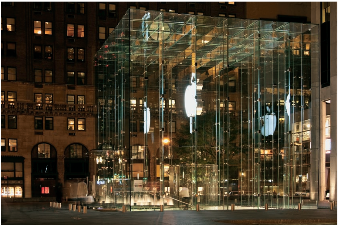
FIGURE 6.1 Apple Store, Fifth Avenue, New York City, 2006, Bohlin Cywinski Jackson architect with Eckersley O'Callaghan as the glass engineer. The Apple Cube broke new ground in glass structure design.
