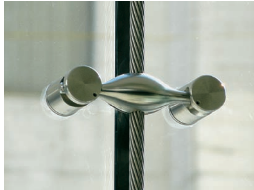
FIGURE 16.8 Interior view of the intermediary point fixing.
