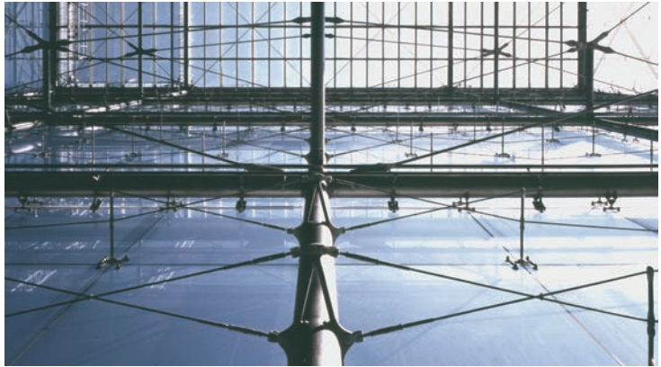
FIGURE 1.6 Glass Walls (Les Serres), Parc de la Villette, Paris, 1986, Adrien Fainsilber, architect, with Rice Francis Ritchie (RFR). Peter Rice conceived the cable mullion as a means of optimizing transparency.
