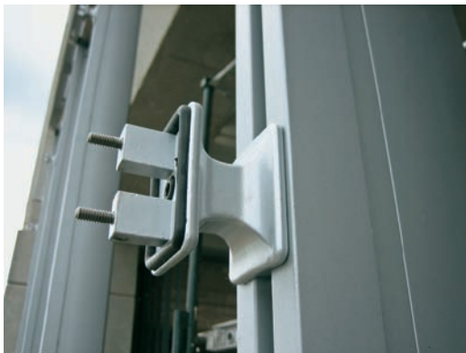
FIGURE 14.11 The VS-1 System before glass installation.
