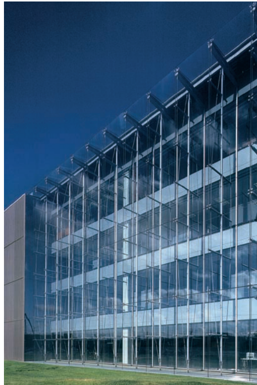
FIGURE 3.8 Yasaki North America, Canton, Michigan, 1998, Skidmore Owings & Merrill. The mast trusses support the outer skin of one of the first double-skin walls.
