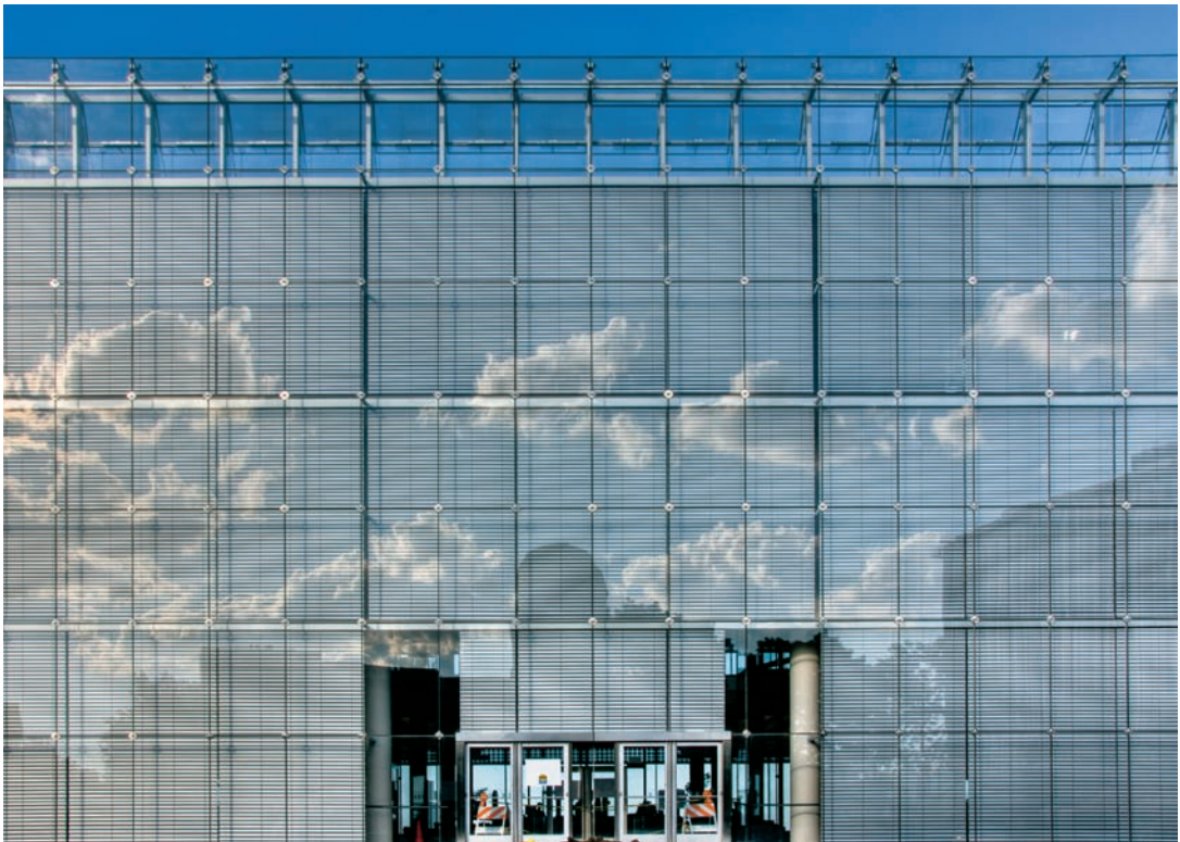
FIGURE 14.17 The main entry through the west facade on a summer afternoon, with the automated blinds fully closed.
