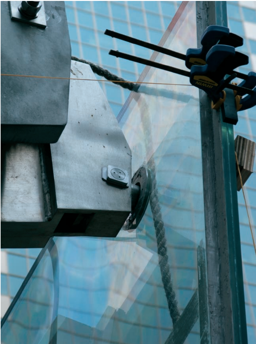
FIGURE 6.7 Construction detail at the rotule connection.
