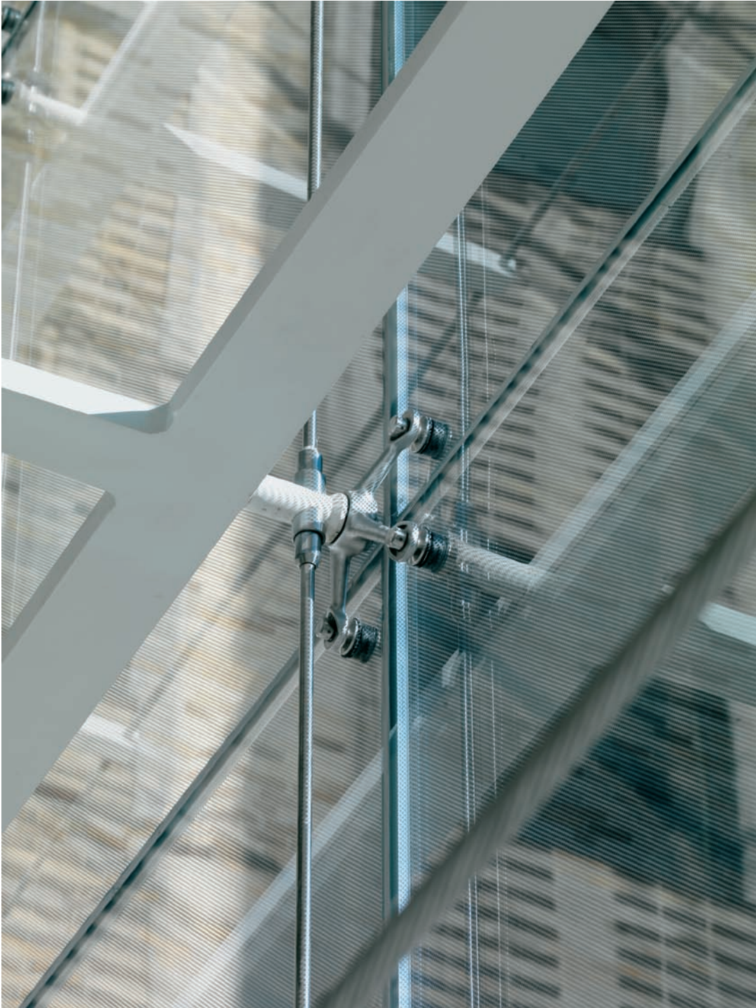
FIGURE 11.11 Detail of glass fixing on the atrium wall. Note the dead load rods.
