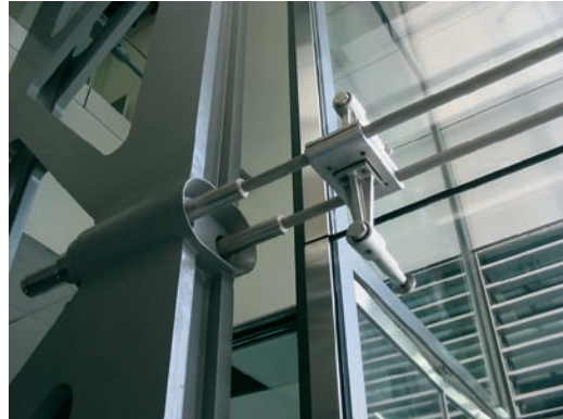
FIGURE 15.15 The truss and cable termination are exposed at the perimeter of the facade.
