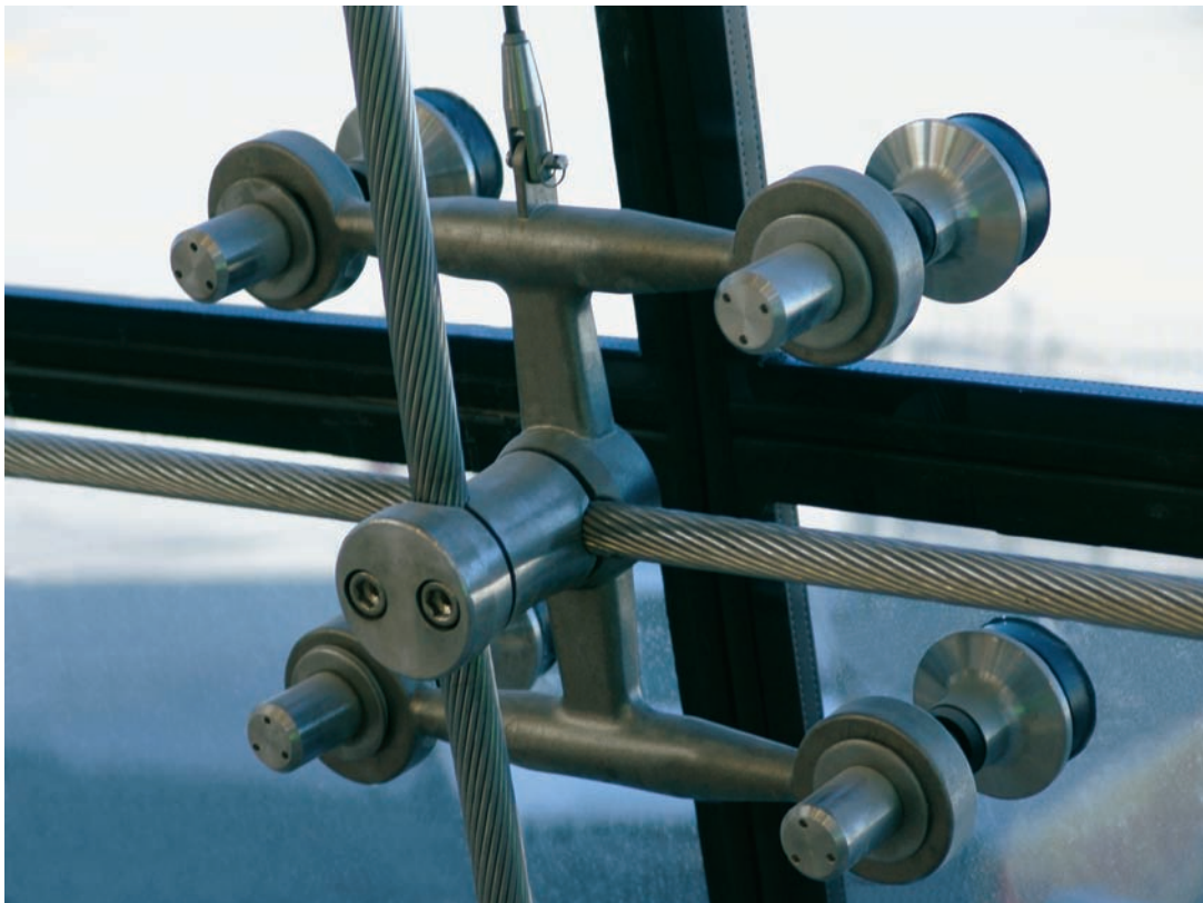
FIGURE 5.10 An H-type spider fitting supported by a double-curved cable net. Note the large silicone joint between the insulating glass units (IGUs).
