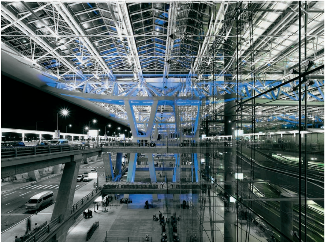
FIGURE 8.11 The large roof overhangs are intended to shade the facades from the tropical sun. The facades comprise a minimal membrane between inside and outside environments.
