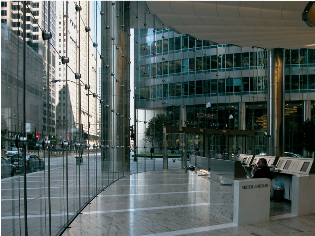
FIGURE 5.2 This cable mullion system enclosing the lobby of a 53-story tower at 111 South Wacker in Chicago by Lohan Caprile Goettsch Architects (2005) is curved in plan and encloses the lobby of a downtown Chicago high-rise.
