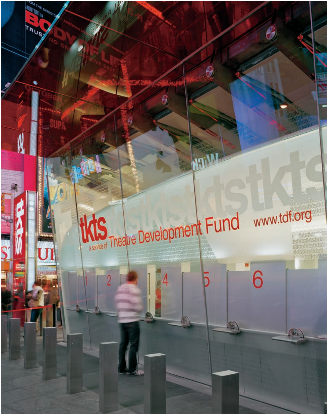
FIGURE 17.8 The ticket wall glass panels are 6 ft (1.8 m) wide and nearly 17 ft (5.1 m) tall, and weigh nearly 3000 lb (1361 kg). The glass stringer beams are supported from a rotule connection at the top of the panel.
