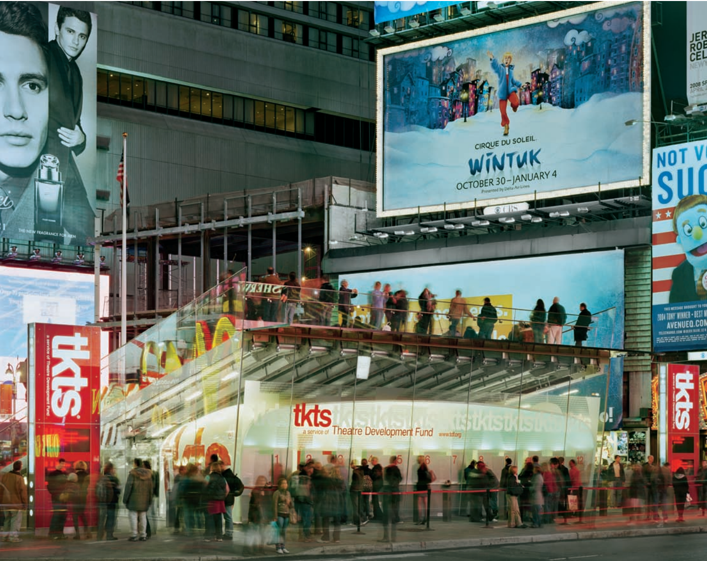
FIGURE 17.1 Show tickets are sold from a white fiber-glass shell located within the glass enclosure.
