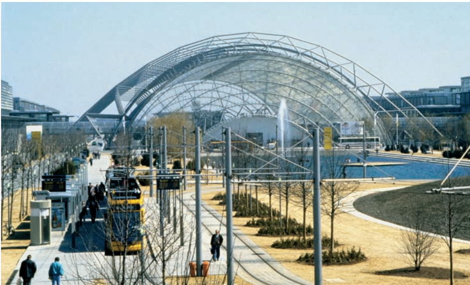
FIGURE 1.11 Messe-Leipzig Glass Hall, Leipzig, Germany, 1995, Gerkan Marg & Partners and Ian Ritchie Architects. The monumental glass vault is another milestone in the evolution of SGFs, widely publicized and influencing future applications.
