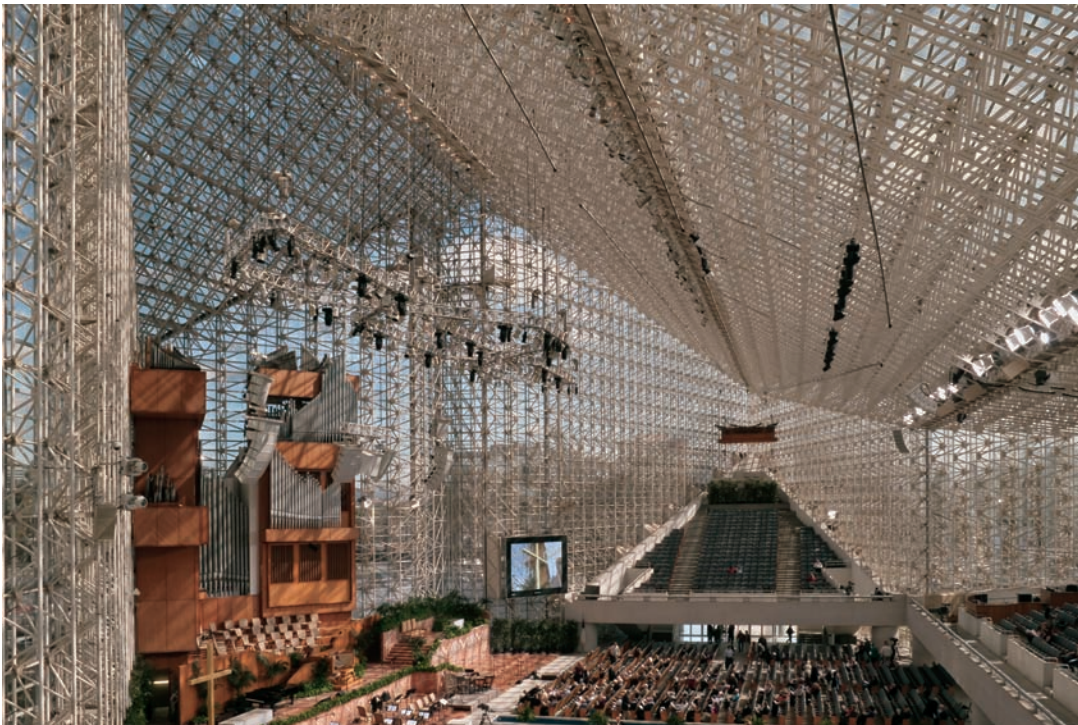
FIGURE 1.5 Crystal Cathedral, Garden Grove, California, 1980, Johnson/Burgee Architects. A reflective glass-clad space frame provides the enclosure for the Garden Grove Church.
