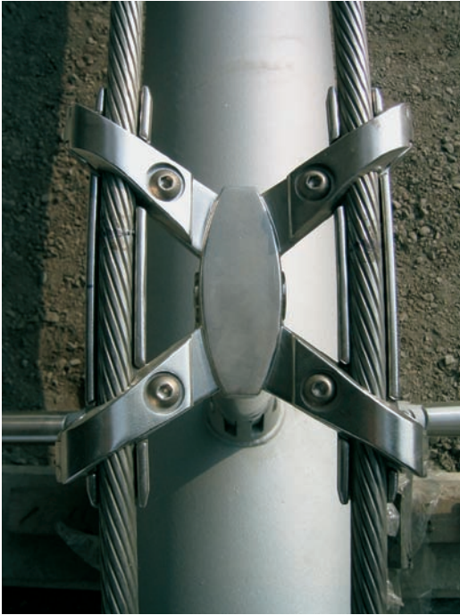
FIGURE 8.12 A butterfly cable guide, one of the cast fittings developed for the MTB facade structural system.
