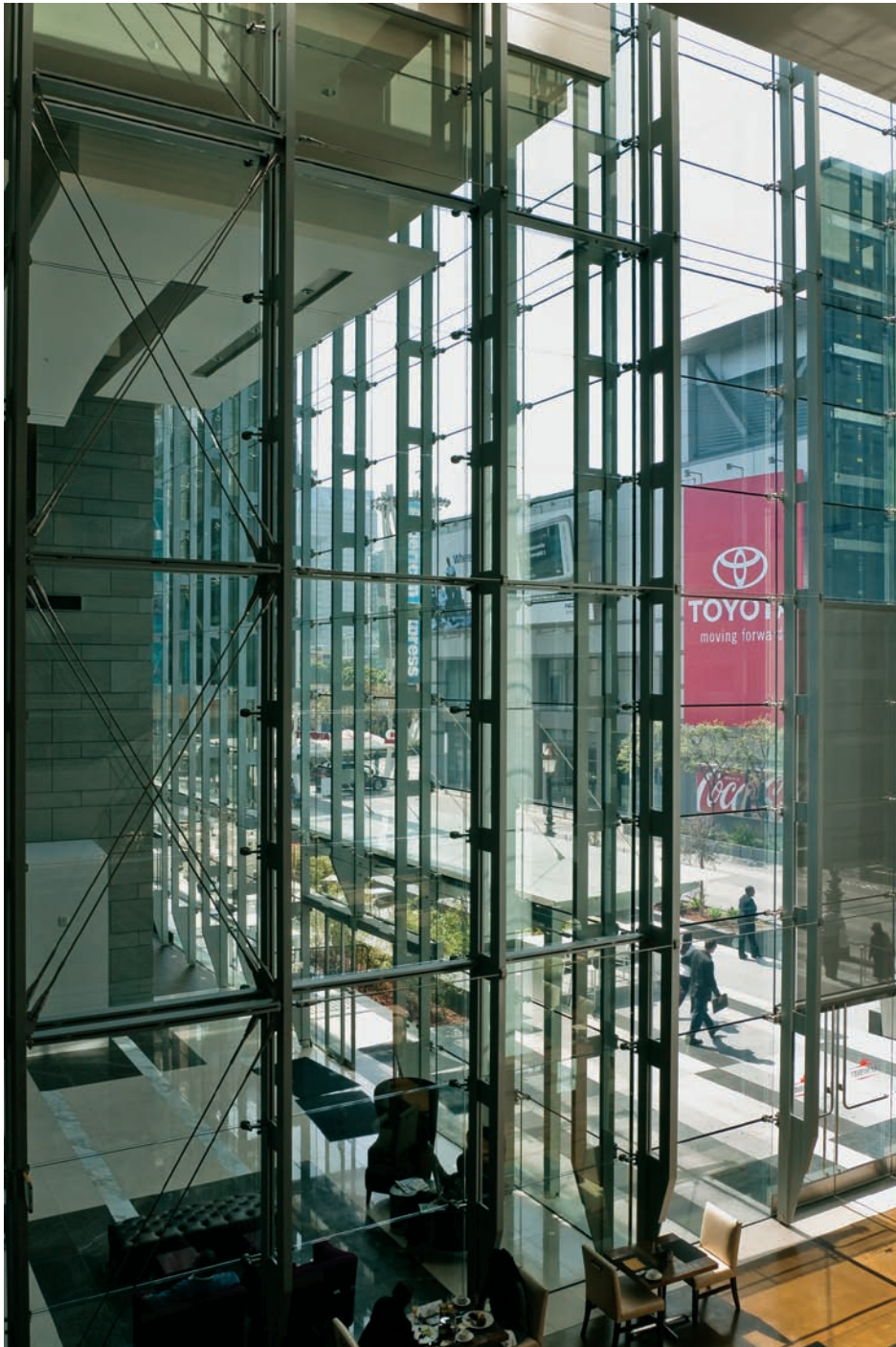
FIGURE 7.16 Rather than pursue maximum transparency, the designers chose to express the trusses as strong visual elements in the facade.
