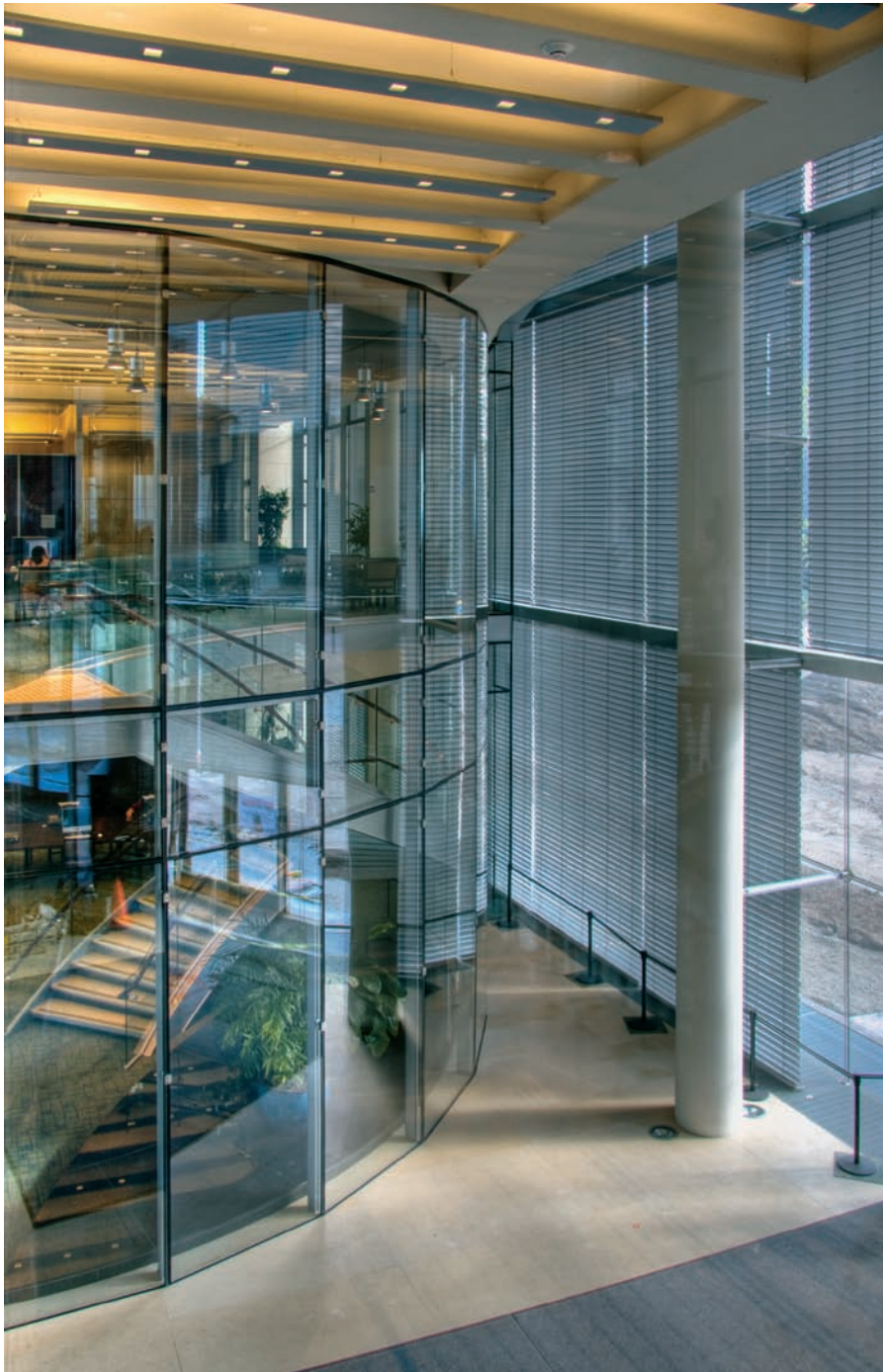
FIGURE 14.16 A vestibule located inside the main entry of the west facade is actually part of the double-skin cavity. The opening through the inboard skin is just to the left of the picture frame.
