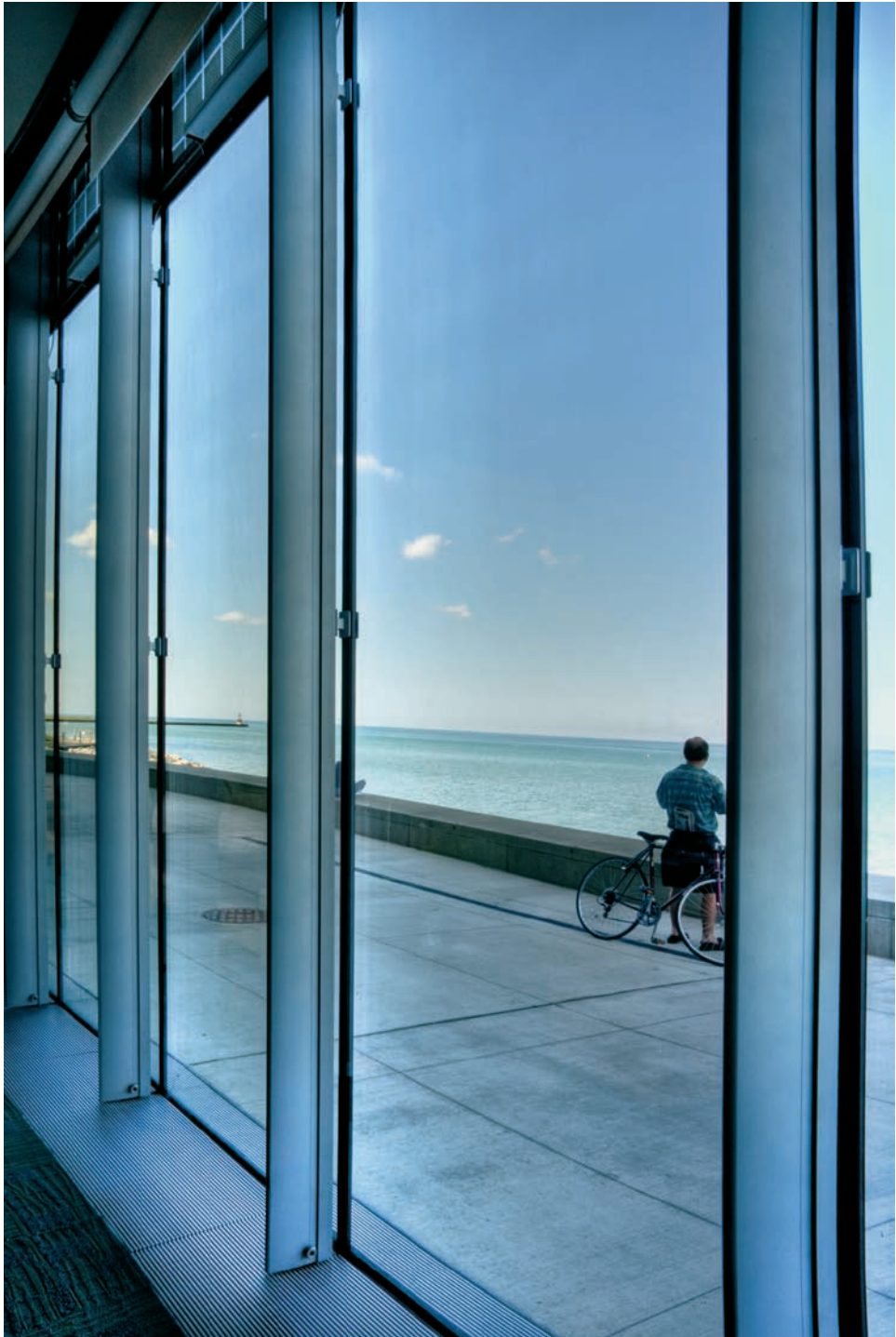
FIGURE 14.5 A view through the ground floor of the east facade. Note the automated roller shades at the top.
