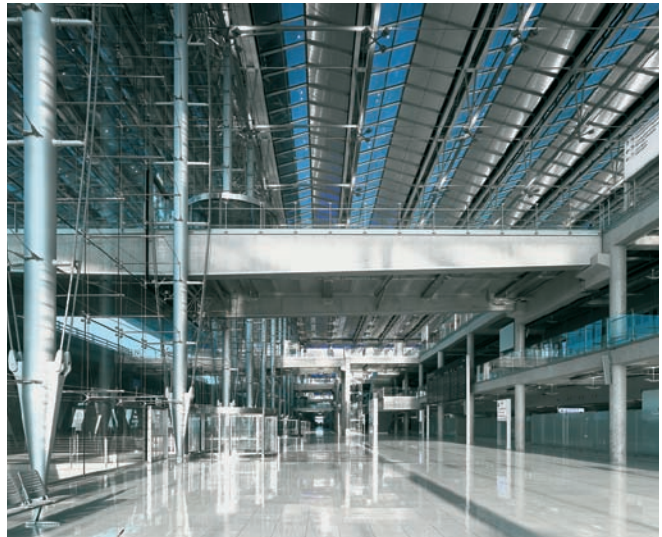
FIGURE 8.7 The masthead and footing are large castings. The footing tapers to a pin connection.
