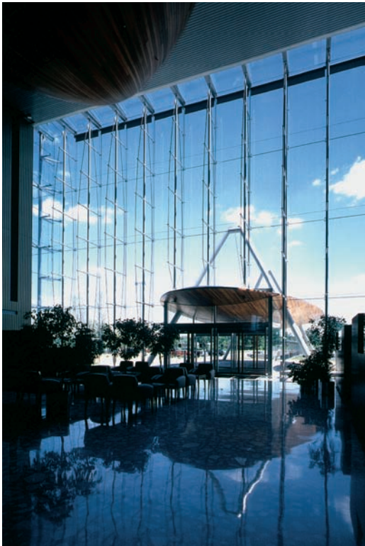
FIGURE 3.9 The mast trusses are left exposed in the lobby area of the office building.
