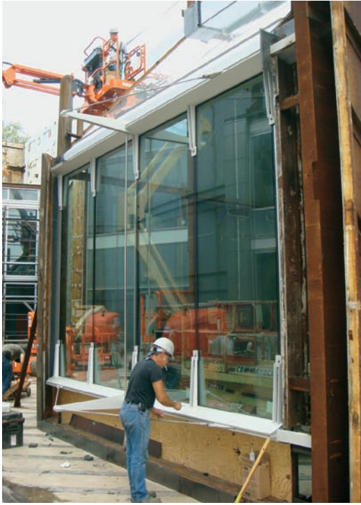
FIGURE 10.13 A full-scale test mockup includes wall, transition, and roof sections.
