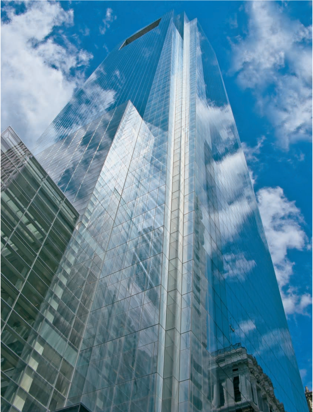
FIGURE 1.1 Comcast Center, Philadelphia, 2008, Robert A.M. Stern architect.
