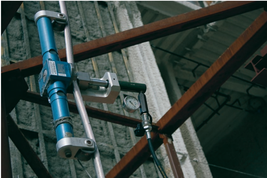
FIGURE 5.11 A tension meter is being used here to measure the prestress levels in a cable.
