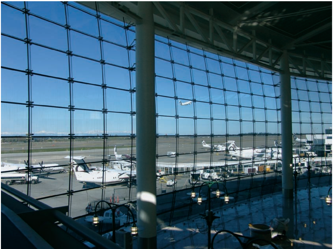
FIGURE 5.8 Sea-Tac International Airport Central Terminal, 2005, Fentress Bradburn Architects. The double-curved cable net facade supports a point-fixed drilled glass system.
