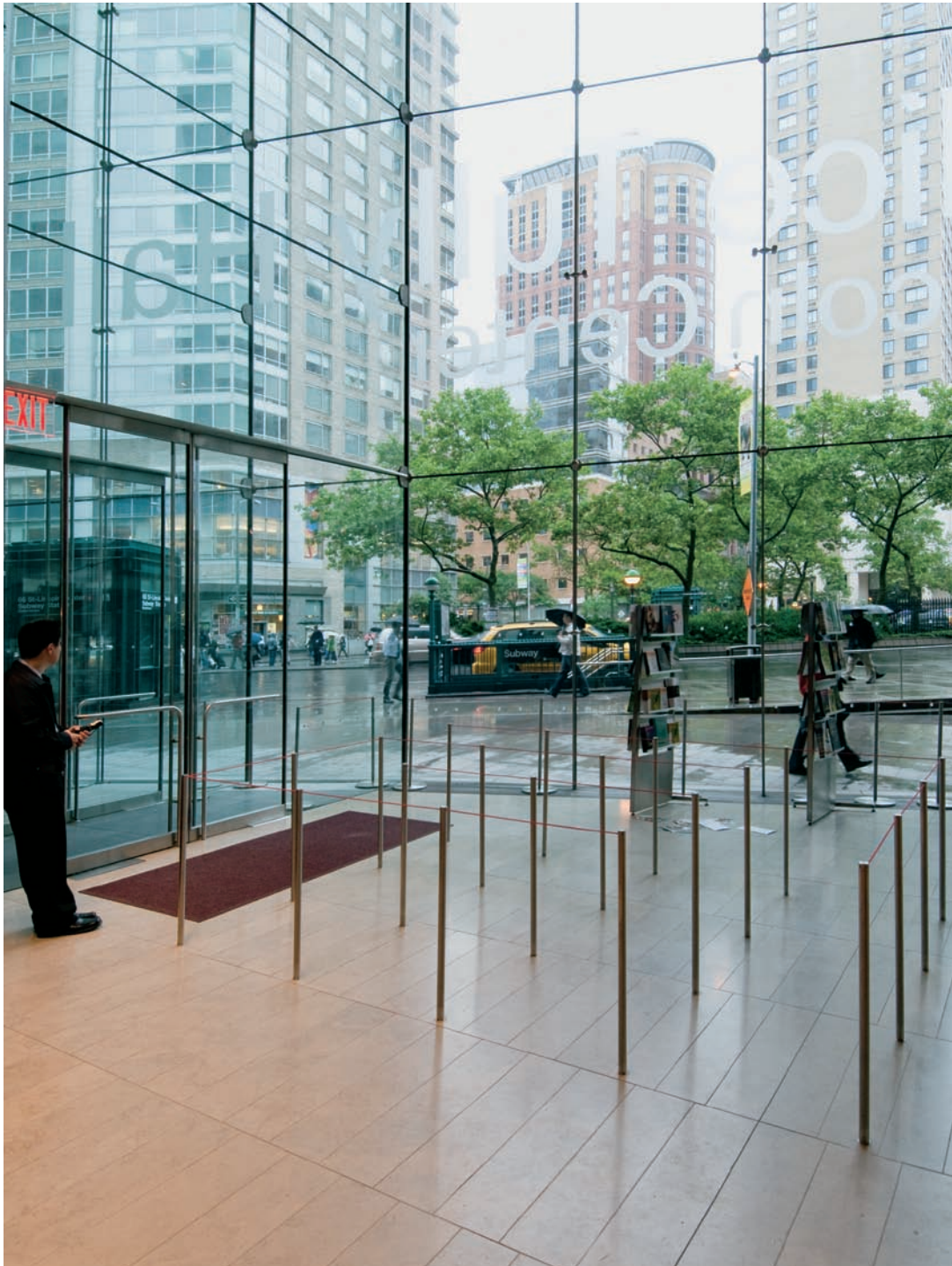
FIGURE 16.5 A double vestibule is located near the intersection of the two walls.
