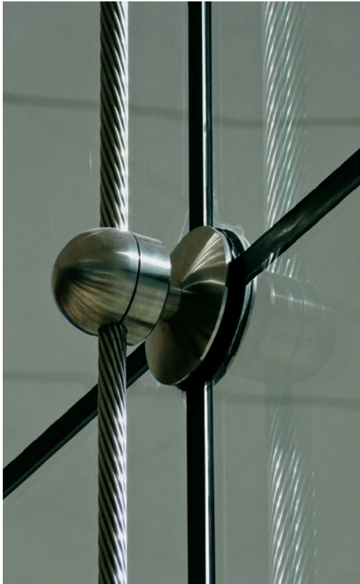
FIGURE 16.7 Clamp fitting at the glass grid vertex.
