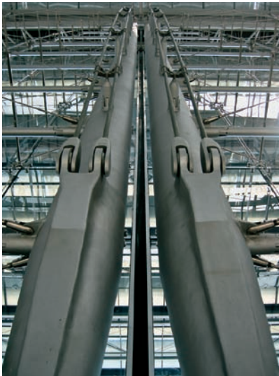
FIGURE 8.6 Cast cable ties at base of mast trusses at expansion joint.
