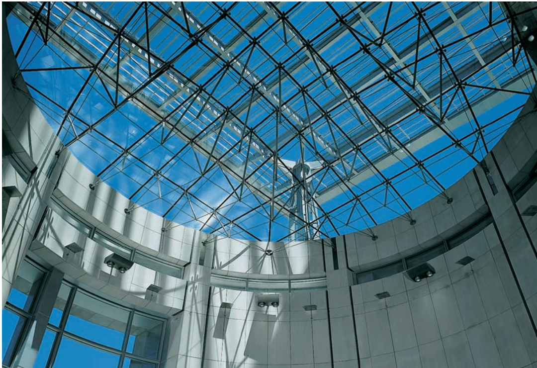
FIGURE 4.9 Lloyd D. George United States Courthouse, Las Vegas, 2002, Dworsky Associates. A cable-strut skylight encloses the entry lobby to the courthouse.
