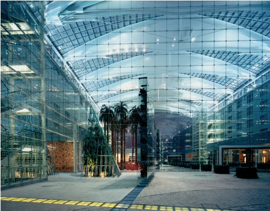
FIGURE 1.10 Cable net facades at the Kempinski Hotel, Munich, 1993, Murphy/Jahn Architects. This is the first application of a flat cable net as a glazed facade structure.
