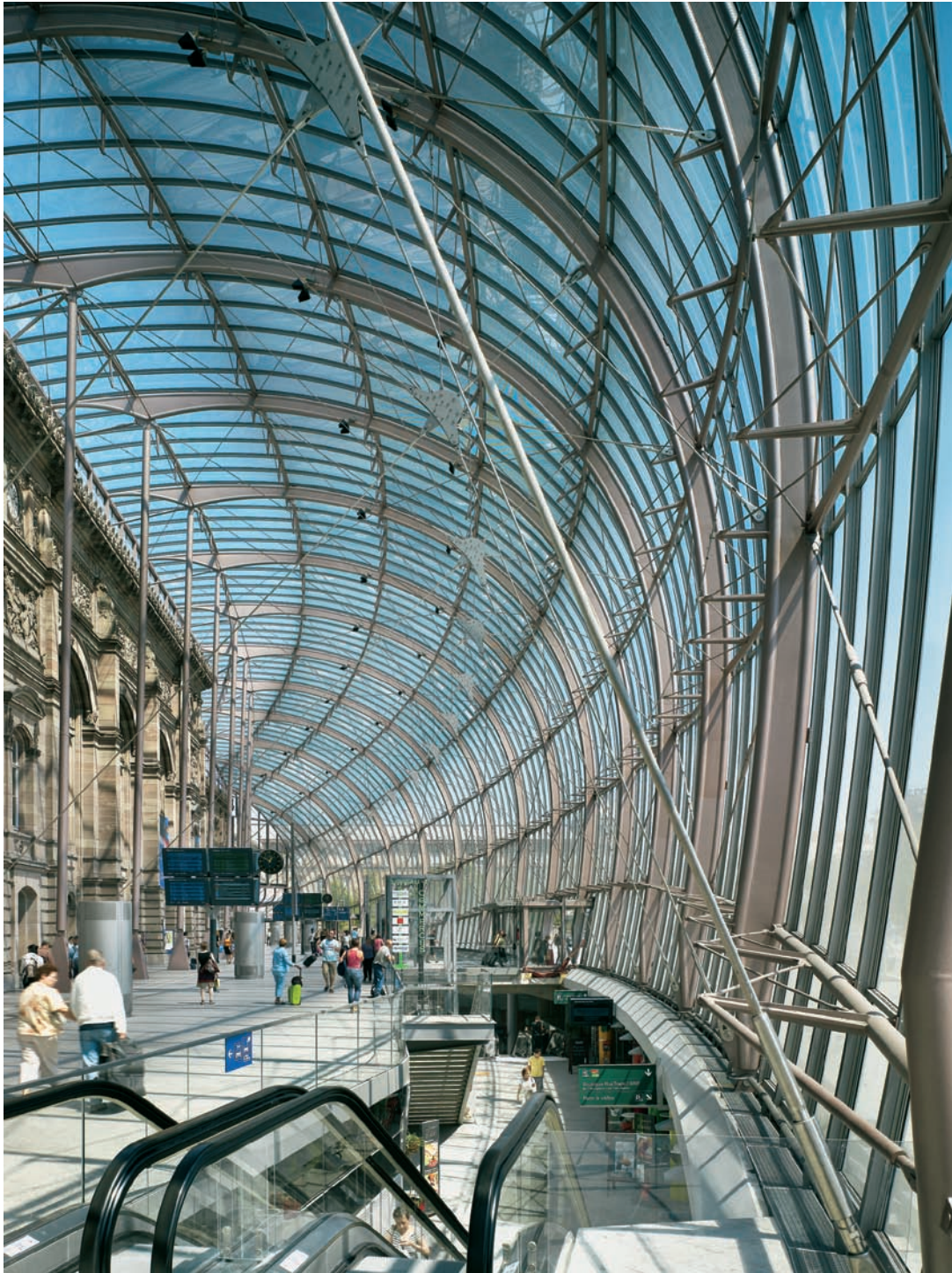
FIGURE 12.2 The new glass enclosure curves along the face of the old station, creating a climate-moderated public space that provides access to the various transport options.
