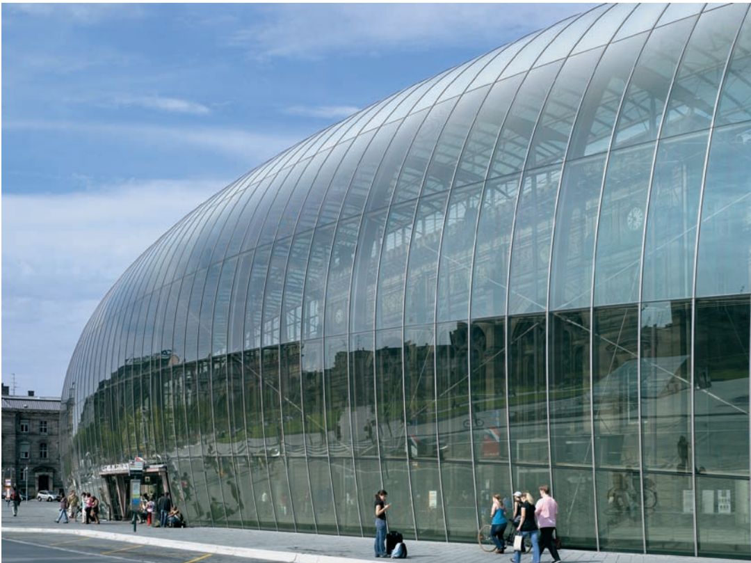
FIGURE 12.7 The glass is cold-formed in the absence of the heat characteristic of the conventional glass-bending process. The glass module has a slender aspect ratio with the short axis perpendicular to the curvature of the glass, facilitating the cold-bending process. The optical quality of the glass resulting from the cold forming is apparent from the reflections.
