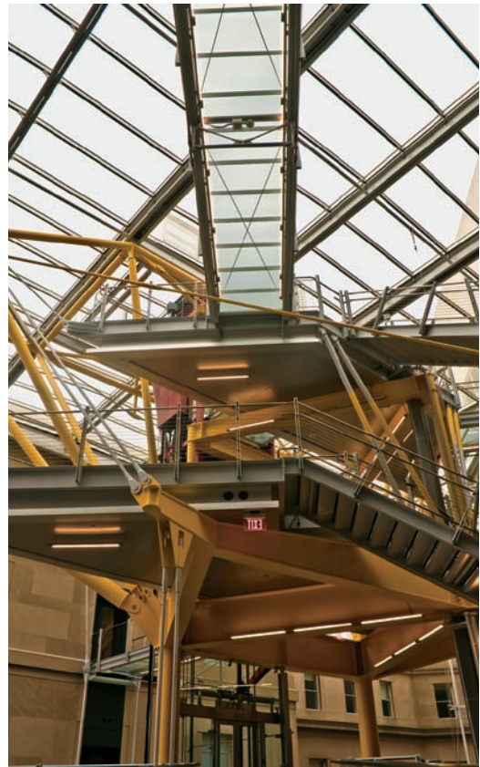
FIGURE 10.2 The atrium ties three buildings together at multiple levels using 16 glass bridges spanning to a central elevator/utility core.
