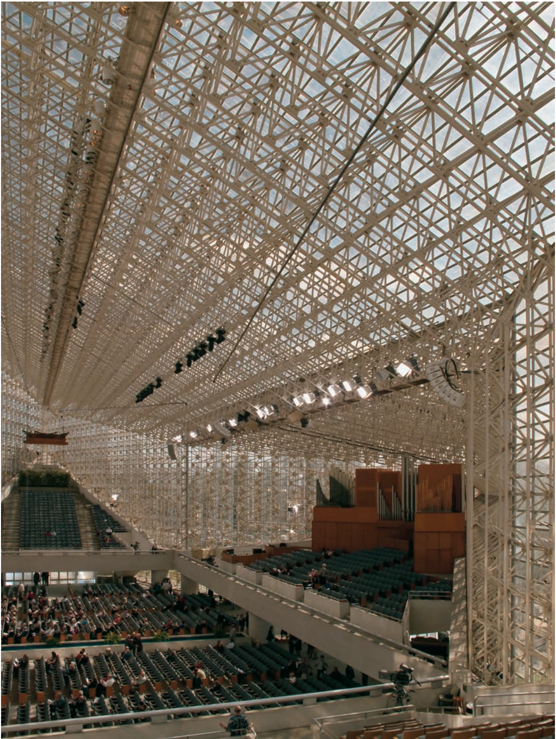
FIGURE 4.3 An interior view of the Crystal Cathedral clearly shows that space frames are not the most transparent structure type.
