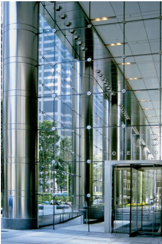
FIGURE 5.4 UBS Tower, Chicago, 2001, Lohan Caprile Goettsch Architects. A series of flat nets enclose the lobby of this high-rise tower, among the first to be completed in the United States.
