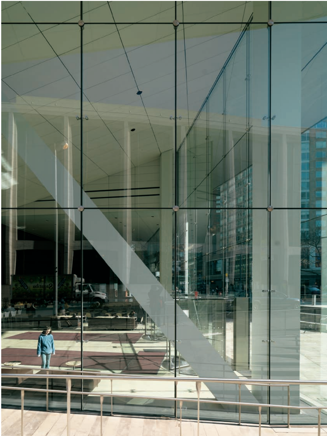
FIGURE 16.3 From the street, the building's structural system becomes sculpture behind glass.
