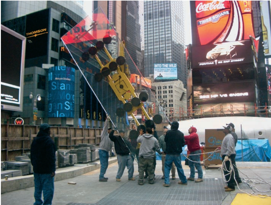
FIGURE 17.13 The first ticket wall panels arrive at the site.
