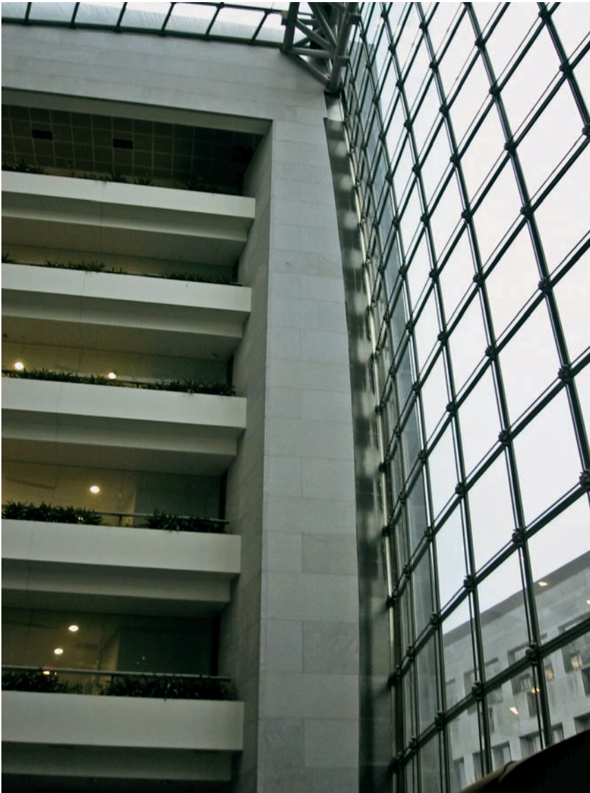
FIGURE 5.7 The slight curvature in the placement of the perimeter anchors is key to providing form to the cable net.
