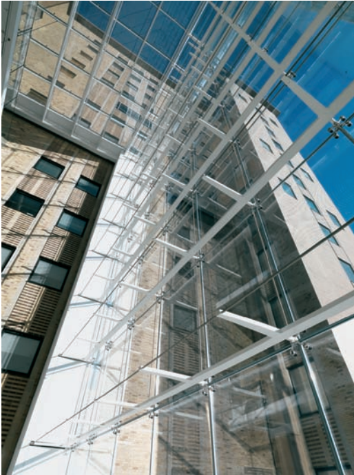
FIGURE 11.8 The atrium wall is supported by horizontal cable trusses.
