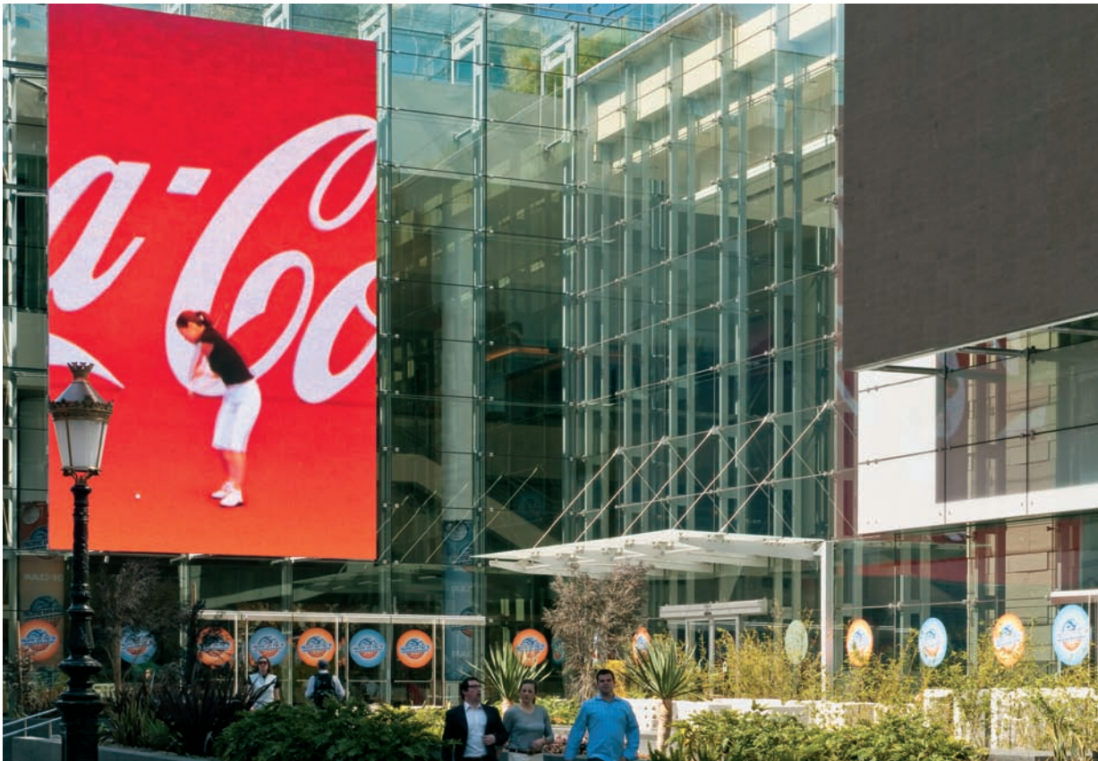
FIGURE 7.15 The south facade experiences considerable solar exposure despite the presence of nearby buildings. A solar control glazing was used to provide an improved SHGC.
