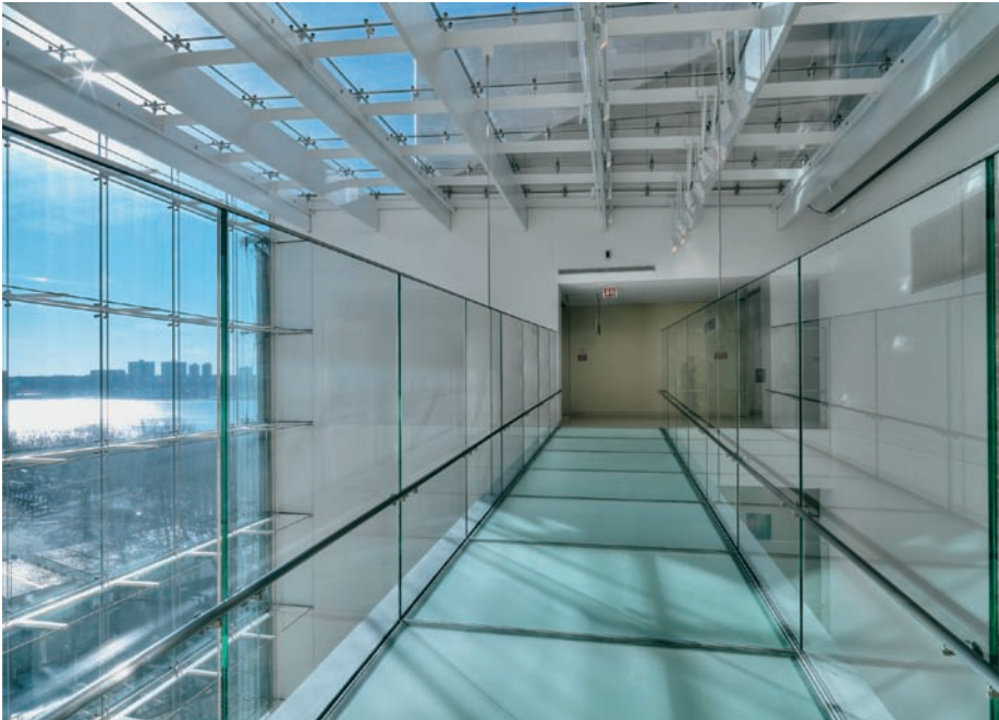
FIGURE 11.9 The atrium wall intersects with a glass skylight roof.
