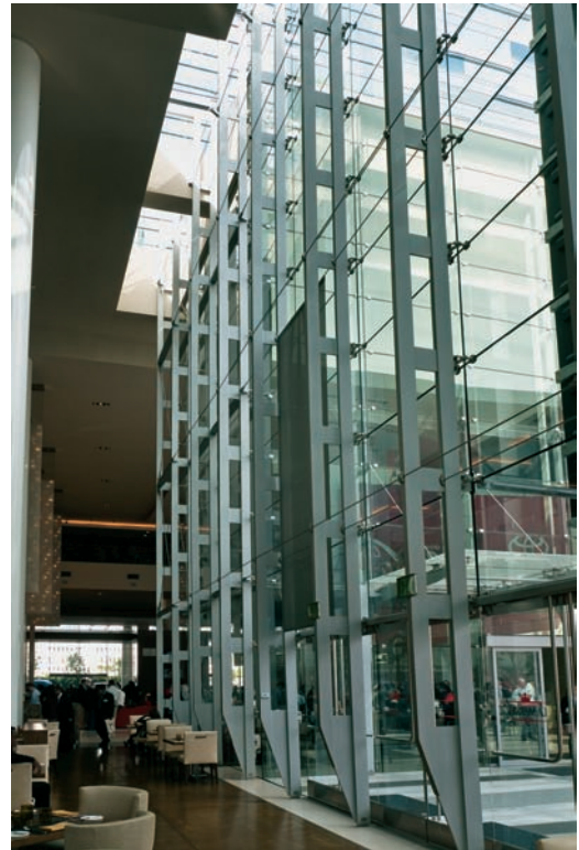
FIGURE 7.2 Plate trusses spanning 52 ft (15.8 m) define the south facade.
