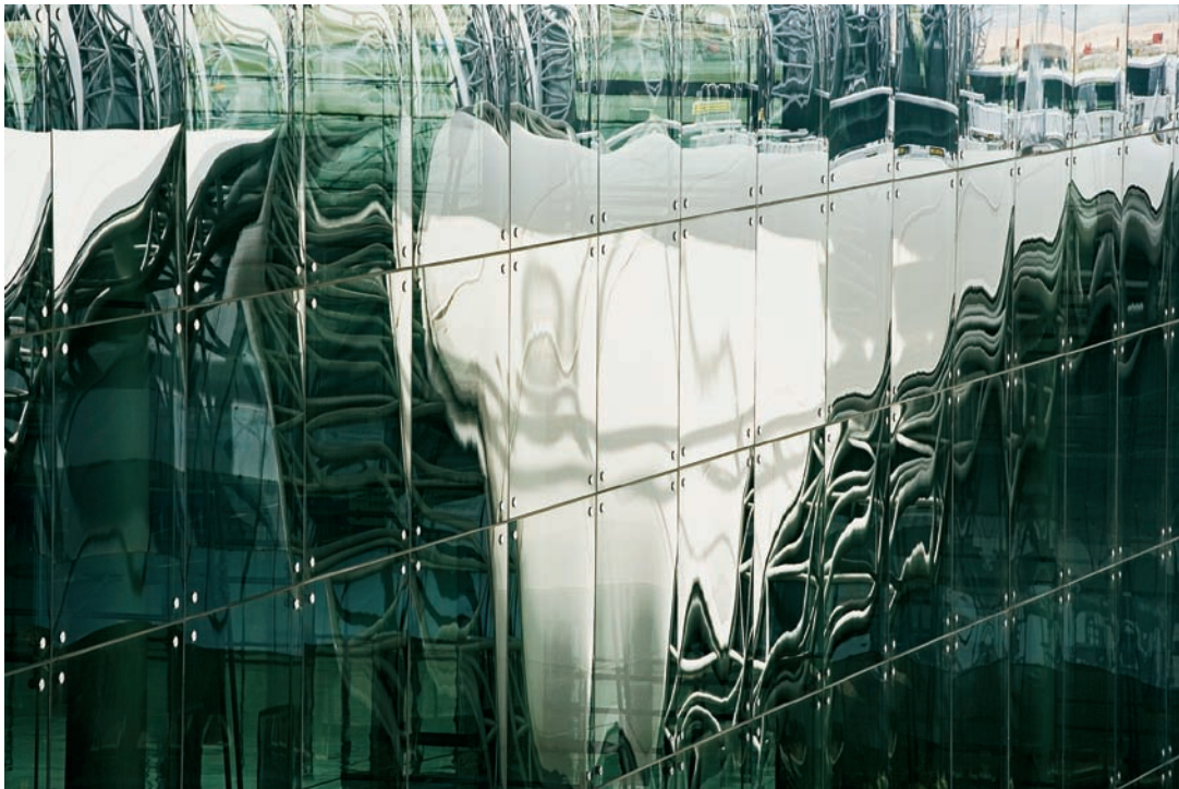
FIGURE 8.10 A solar-control interlayer makes the glass reflective from the exterior. Reflections reveal optical distortion resulting from heat treatment of the glass.
