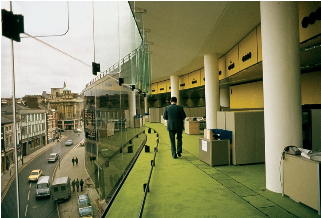
FIGURE 1.4 The Willis Faber & Dumas Building, Ipswich, England, Foster Architects, 1975. The glass facade marks the birth of SGF technology.
