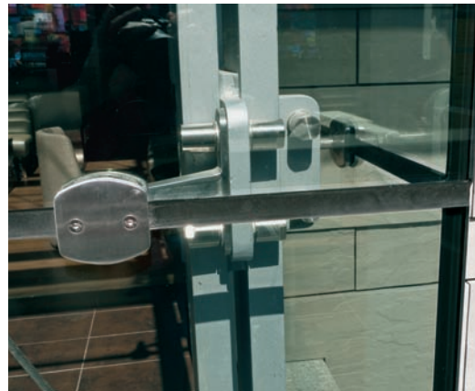
FIGURE 7.13 Glass system connection detail: corner condition.
