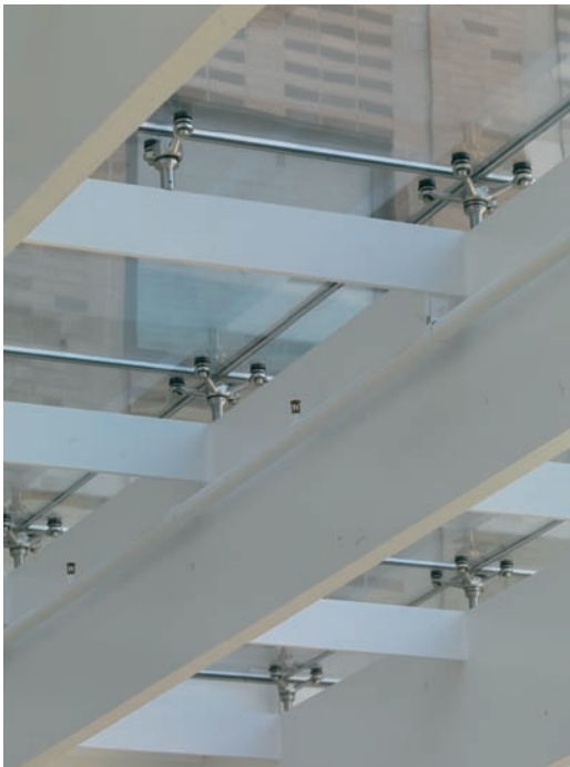
FIGURE 11.12 Plate beams support the point-fixed roof glass.
