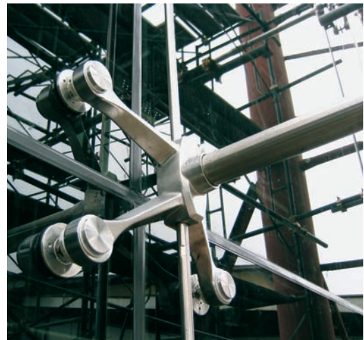
FIGURE 8.9 Cast stainless steel spider fitting.
