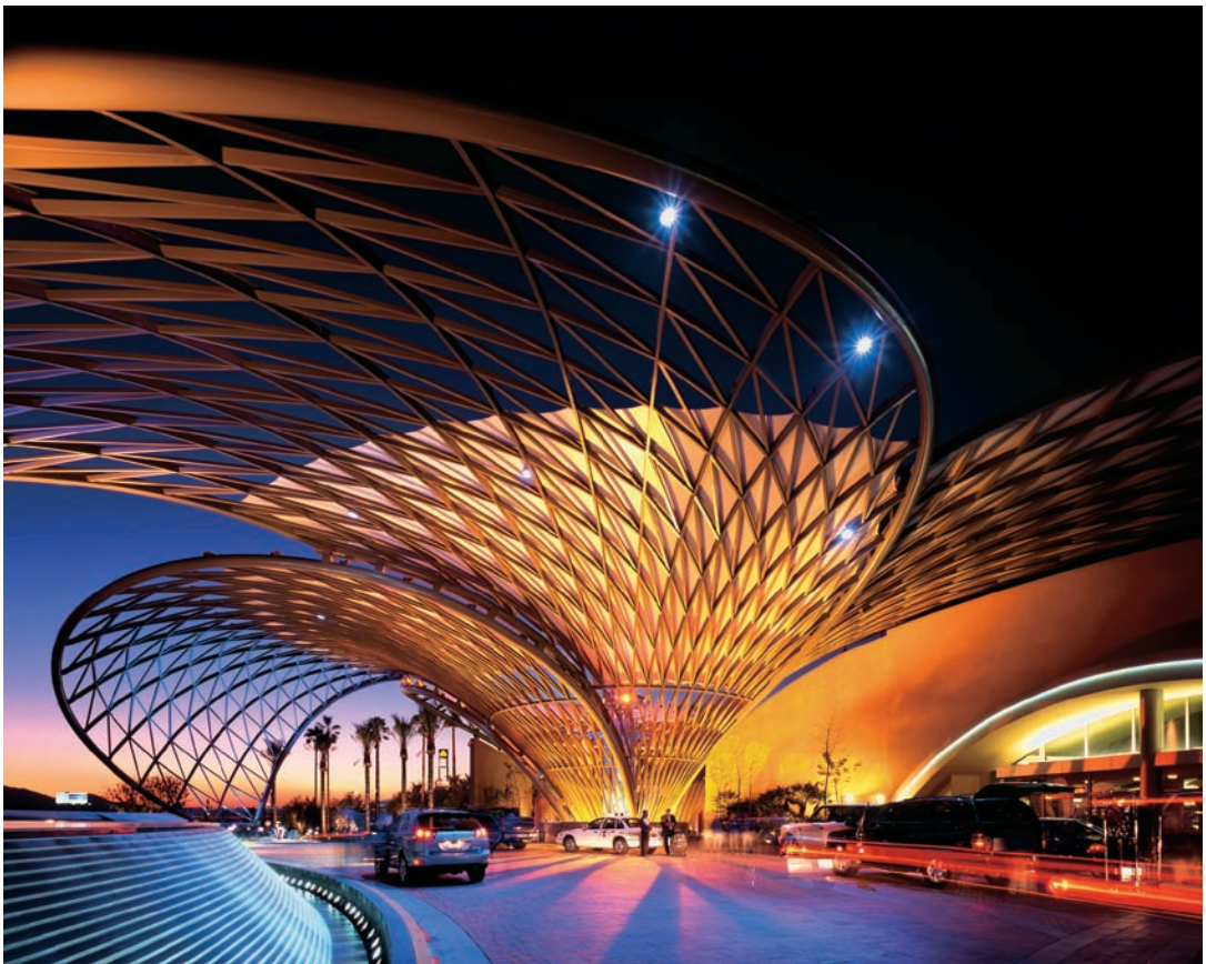
FIGURE 4.7 Desert Bloom, Casino Morongo, Cabazon, California, 2004, Jerde Partnership. The leaves of this triangulated gridshell span 90 ft (27m).
