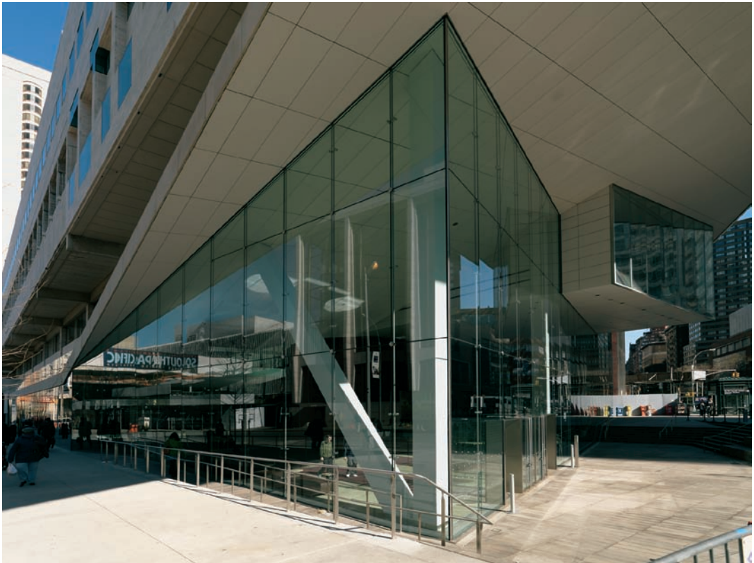
FIGURE 16.4 The two facade faces slope upward to meet at a corner with an elevation of approximately 45 ft (13.7 m).
