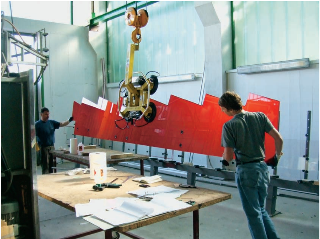
FIGURE 17.12 The perimeter stringer beams are prepared for assembly at the fabricator's plant.
