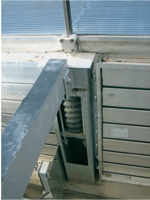
FIGURE 14.6 The base connection detail of the cable net structure during installation.
