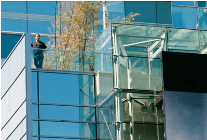
FIGURE 7.5 The trusses step back at their tops to create a 7 ft (2.1 m) skylight that also acts as a perimeter partition to an upper-level entertainment area.
