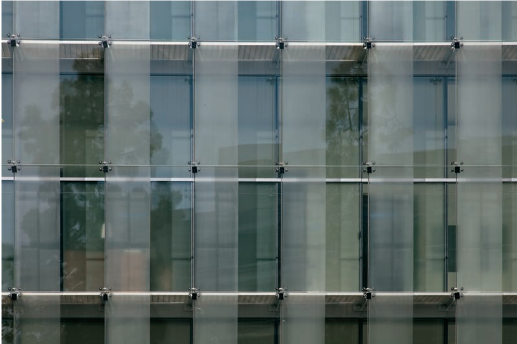
FIGURE 13.5 Exterior of the double-skin facade showing the visual effect of the offset vertical banding in the interior and exterior skins.
