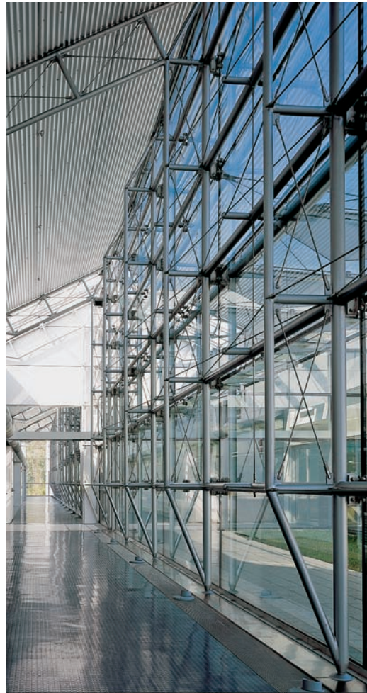
FIGURE 3.5 A simple truss system combining vertical truss elements with horizontal cable trusses.
