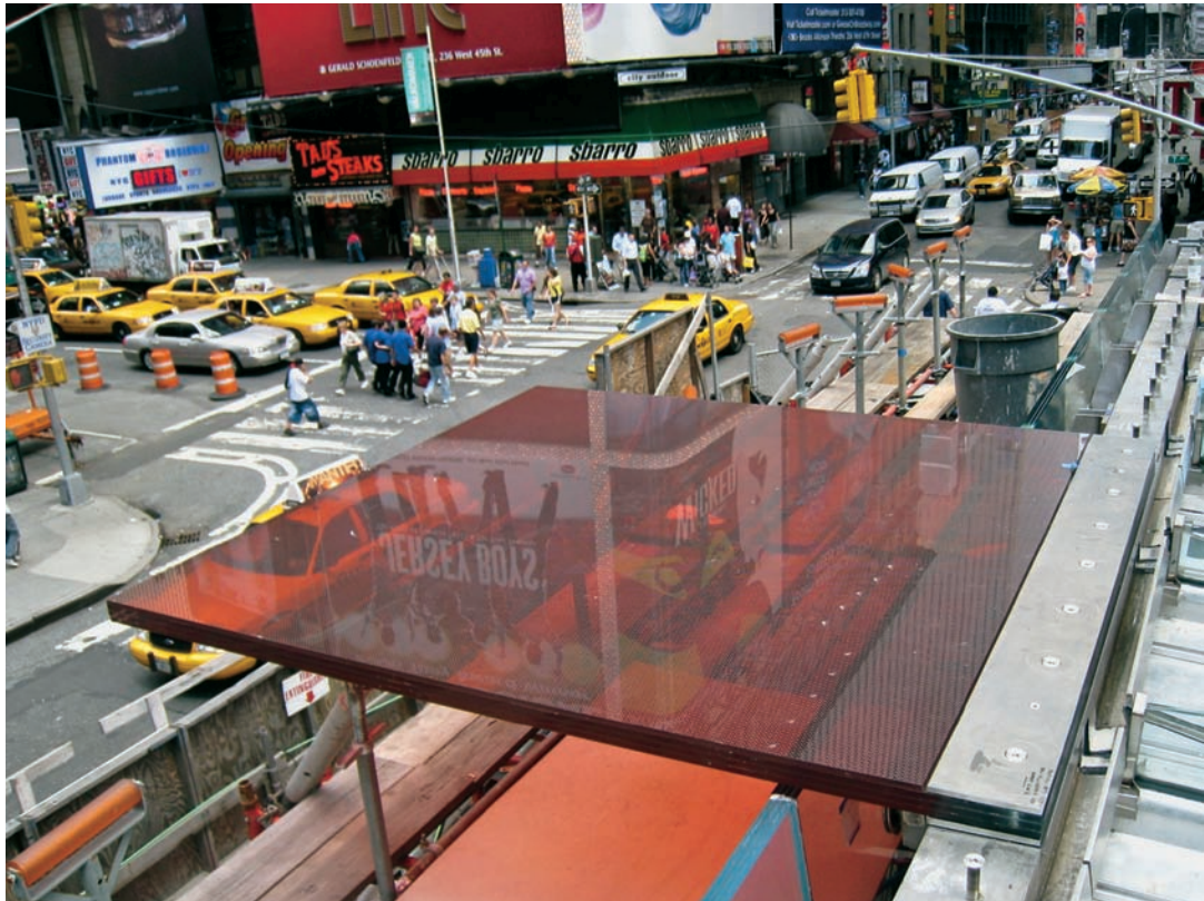
FIGURE 17.10 The first canopy panel is installed. Note the connection detail.
