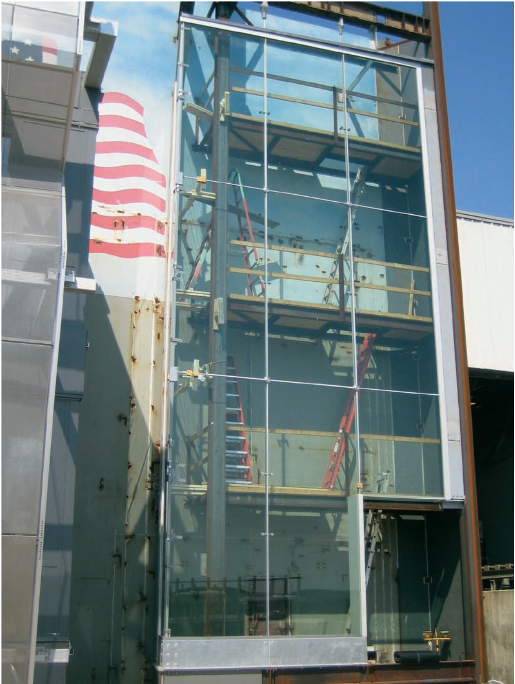
FIGURE 16.10 The performance testing mockup nearing completion.
