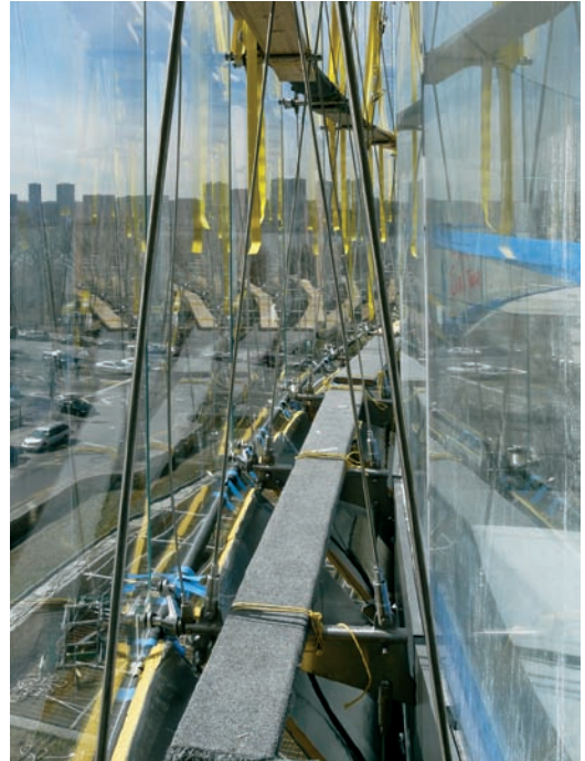
FIGURE 11.10 Inside the cavity of the climate wall during construction.
