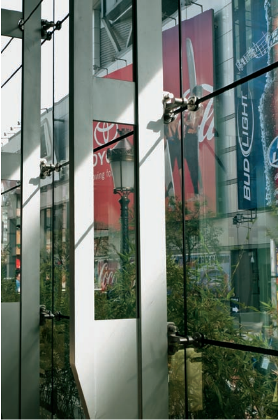
FIGURE 7.4 The plate trusses are fabricated to Architecturally Exposed Structural Steel (AESS) standards and include a bracket at the front face to attach the glass-fixing components.
