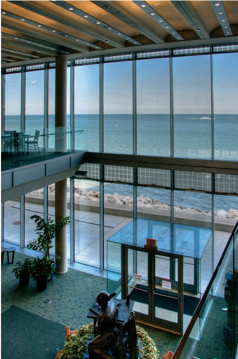
FIGURE 14.4 The VS-1 system spans two floors in the atrium area of the east facade.
