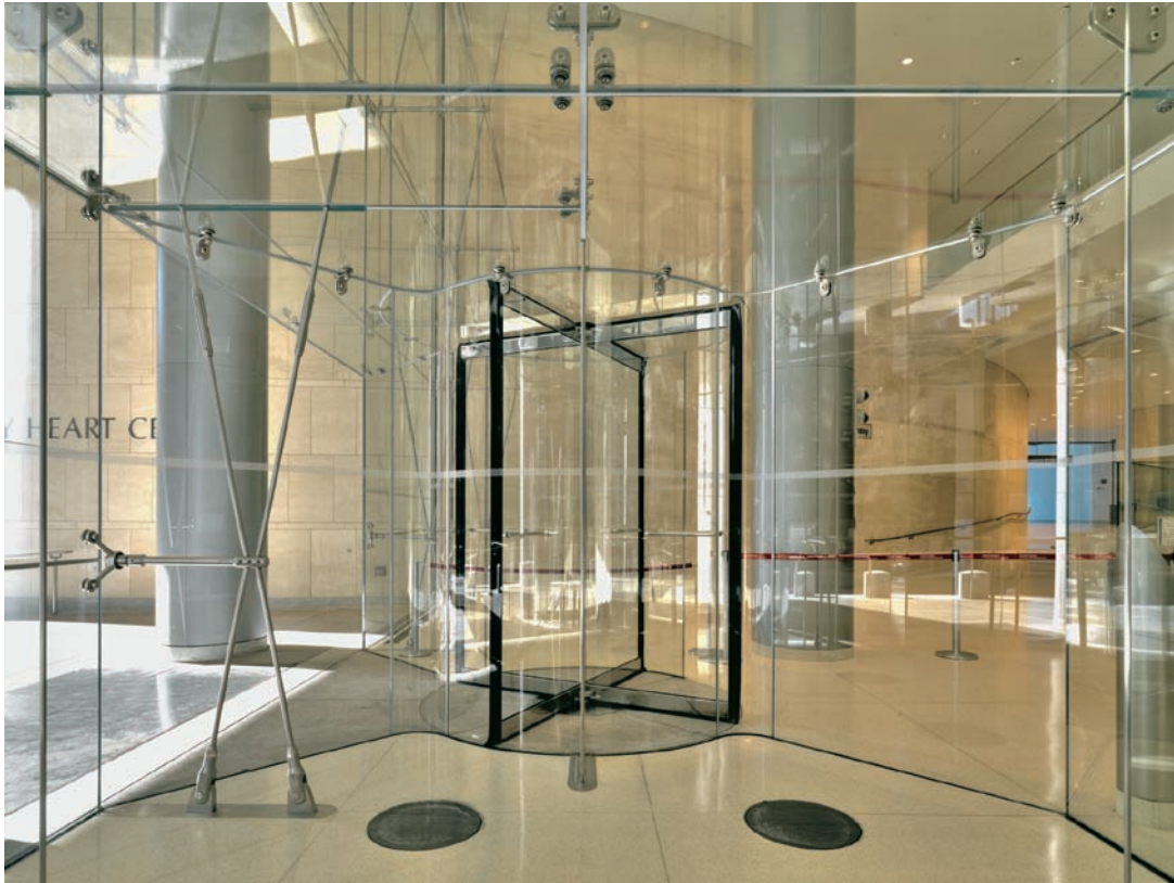
FIGURE 11.20 The entry vestibule combines glass, glass fins, and cable trusses.
