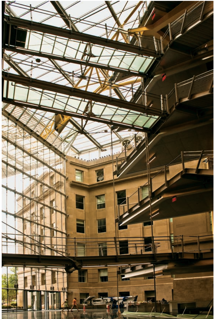
FIGURE 10.1 The atrium enclosure is a 10-story glass wall and skylight roof.
