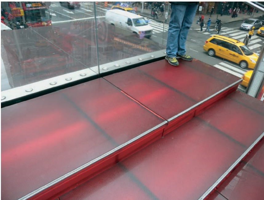
FIGURE 17.7 The top tread. Note the metal nosing.
