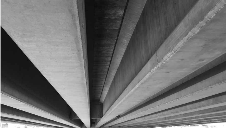
Figure 8.1 Underside of a bridge constructed using precast and pre-tensioned concrete beams.
