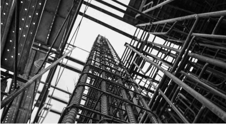
Figure 7.10 A RC column prior to casting.
