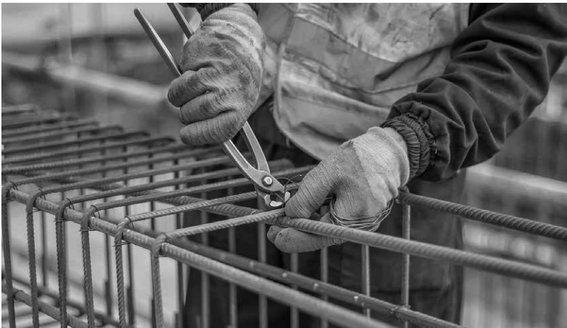
Figure 7.9 A steel fixer attaching a shear link to a beam.
