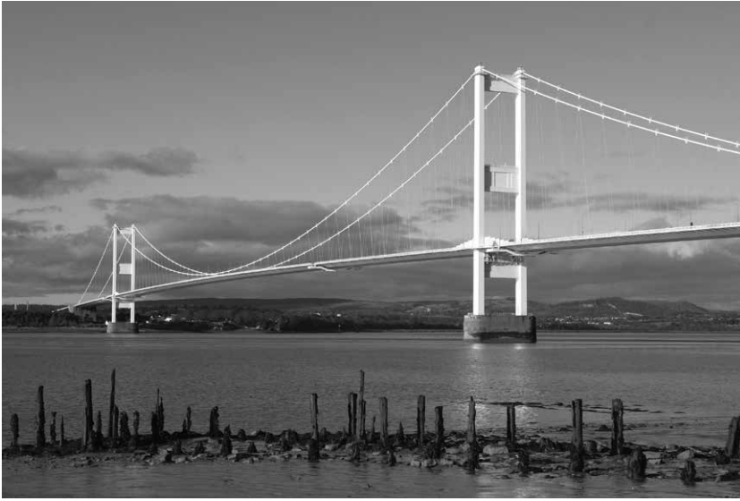
Figure 5.22 This bridge over the River Severn in the United Kingdom uses box-shaped stiffeners, similar to those shown in Figure 5.18.
