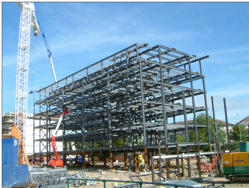
Figure 1.5 Primary steel frame in a major residential project in Southampton
