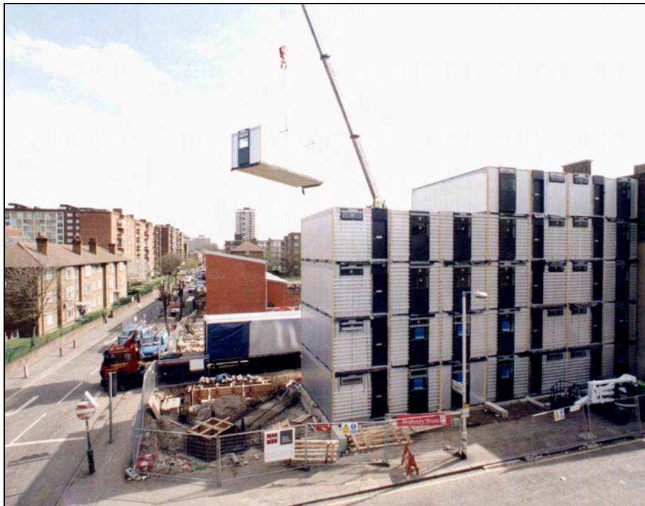
Figure 4.13 Modular units used in multi-storey social housing project in London
