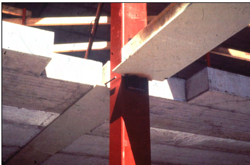
Figure 4.7 Slimflor beams supporting precast concrete slabs
