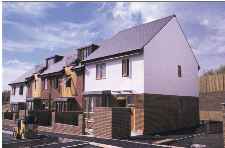
Figure 4.11 Light steel infill walls in a major housing development in Basingstoke
