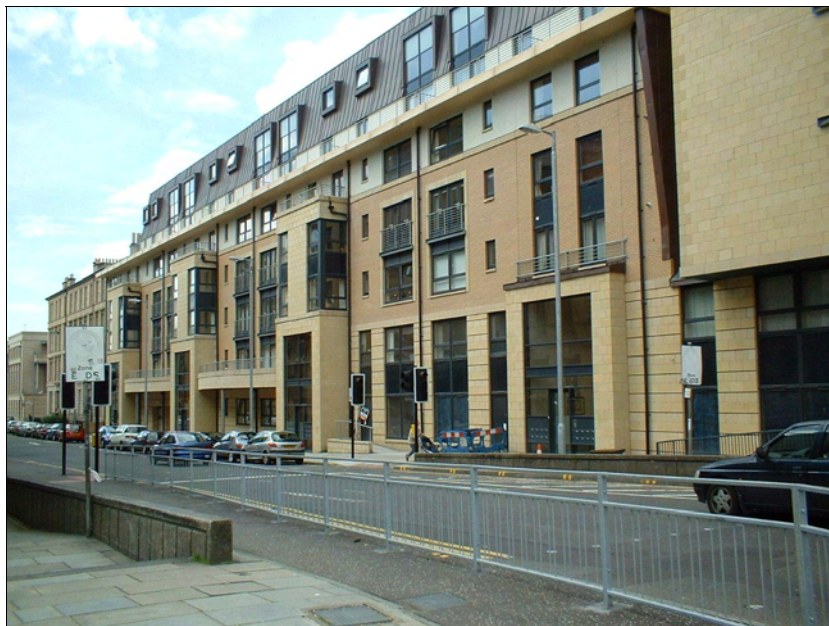
Figure 1.2 Variety of façade treatments in a steel framed residential building in Glasgow
