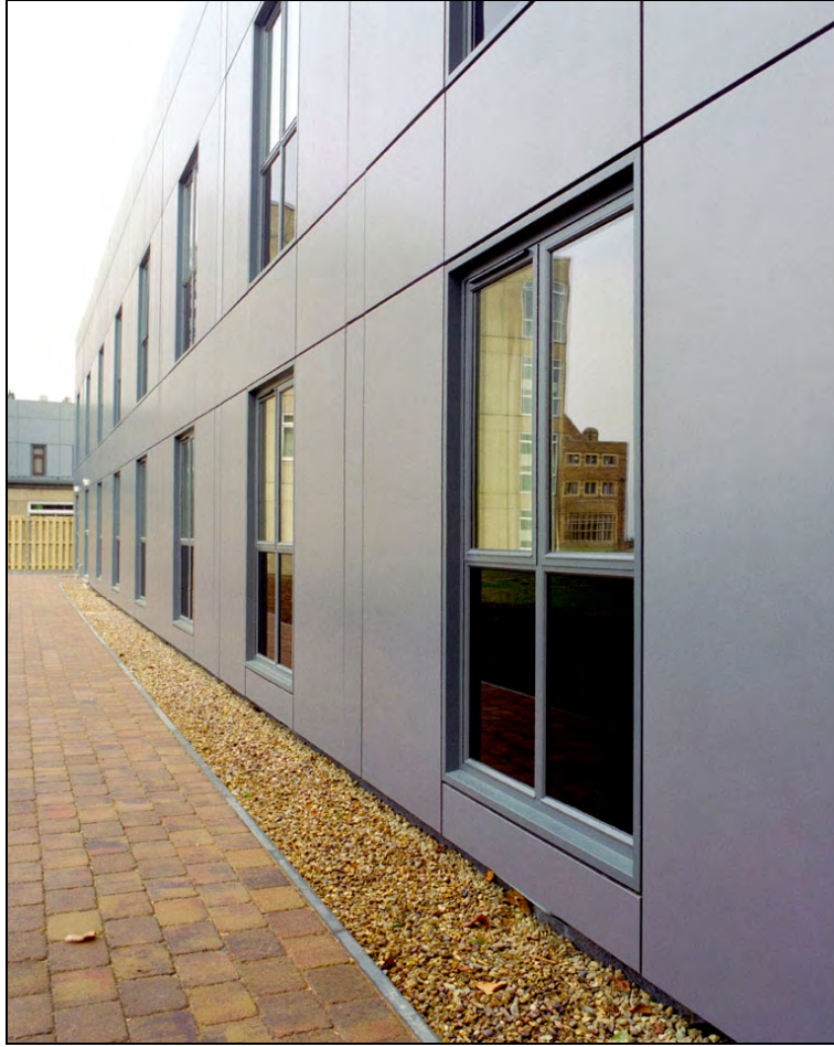
Figure 5.4 Large cassette panels used at the Ashorne Hill Management College
