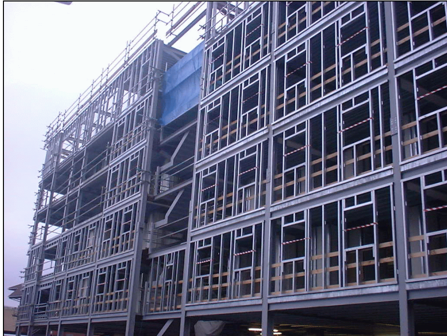
Figure 4.16 Light steel infill walls in a residential building in Southampton
