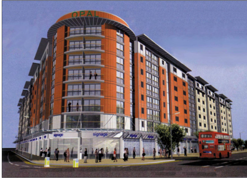
Figure 1.4 Eight-storey modular building in Manchester, supported on a composite frame at podium level
