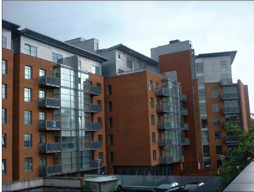
Figure 1.1 Steel framed apartments with pre-fabricated balconies in Manchester
