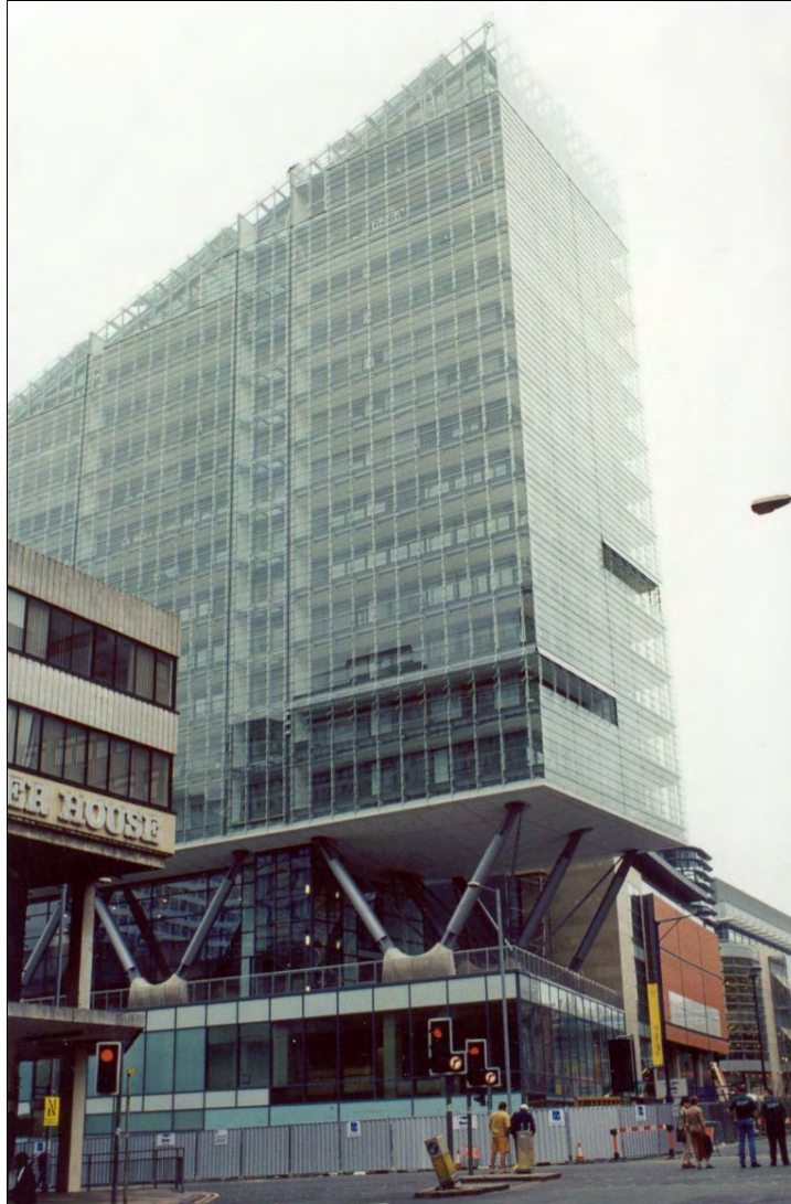
Figure 1.3 16-storey composite steel framed building in Manchester
