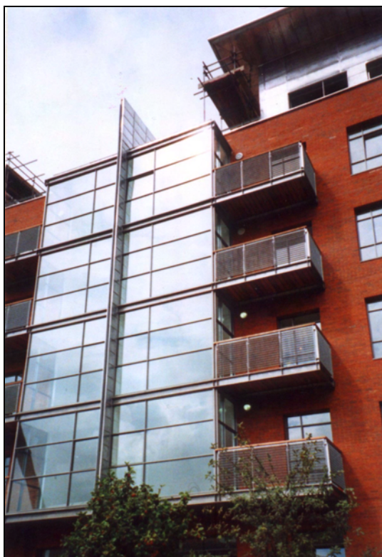
Figure 6.3 Cantilever balconies in a composite structure, Deansgate Quay, Manchester (Courtesy of Stephenson Bell)
