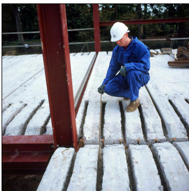
Figure 4.8 Installation of tying reinforcement in precast hollow core units
