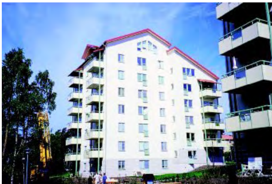
Figure 6.1 Stacked modular balconies (project in Sweden)
