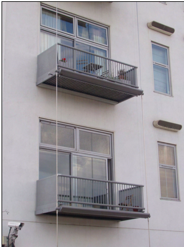
Figure 6.7 Suspended balconies (Piper Building, Fulham)
