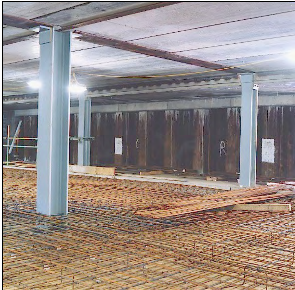
Figure 7.3 Use of Slimflor beams in basement construction
