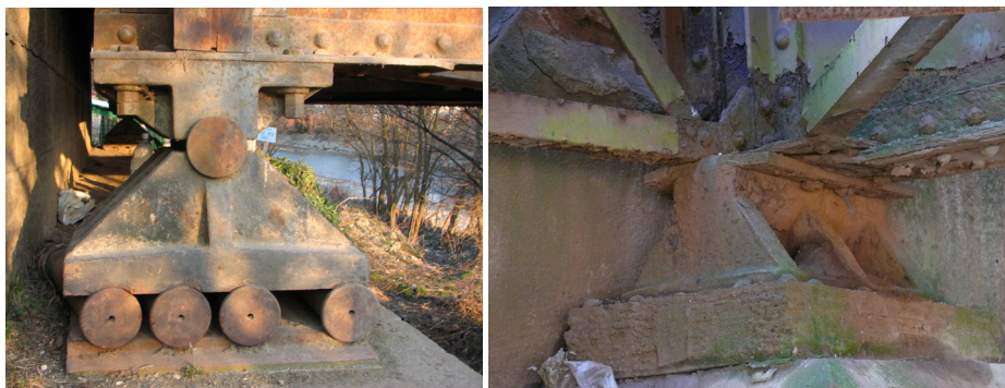
Fig. 5. Defects on bearings
