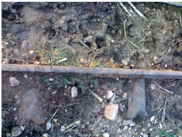
Fig. 16. Balastless narrow rail track showing intensive rust of sleepers buried in the clay soil
