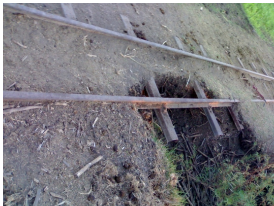
Fig. 17. Soil Erosion under the railroad.
