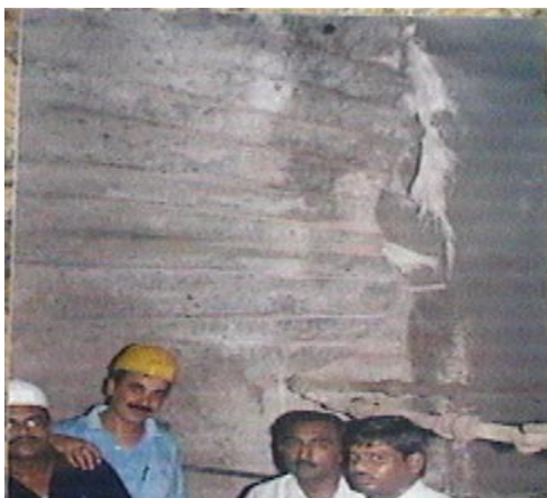
Fig. 5(b). Pier nose wall after pre-split blasting
