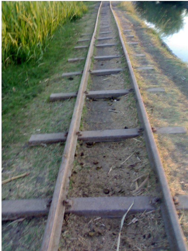
Fig. 5. A ballastless narrow railway expanded on a bank of an irrigation channel
