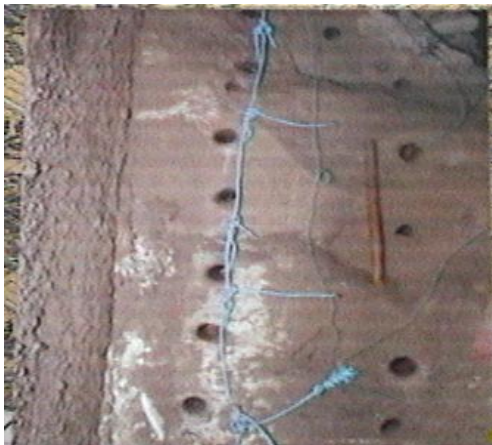
Fig. 5(a). Connections for pre-split blasting
