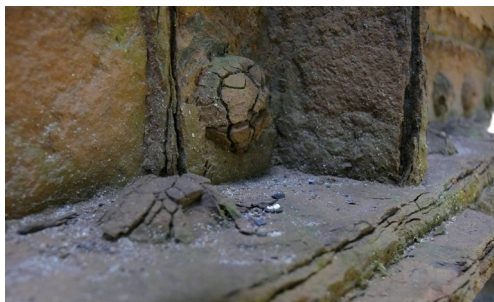
Fig. 6. Strong corrosion at the lower flange – railway bridge on a main line
