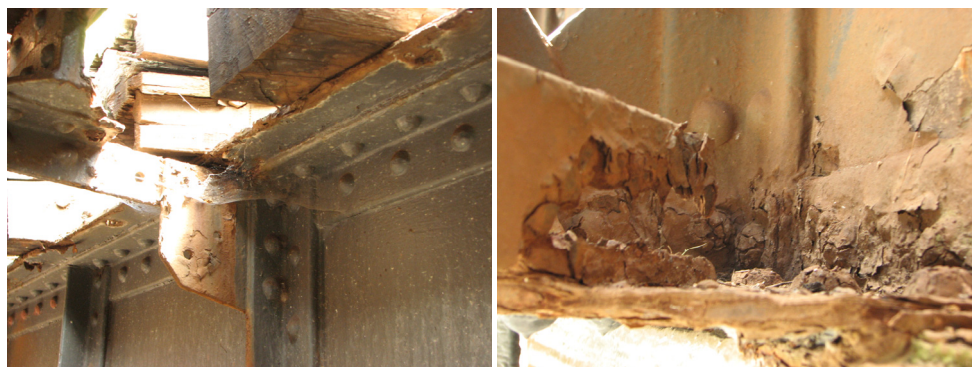
Fig. 34. Corrosion attack details
