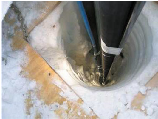
Fig. 10.12 The hot water hose and support cables disappear down one of the many boreholes drilled into the Antarctic ice to construct the IceCube Neutrino Observatory. Credit: Jim Haugen, IceCube/NSF
