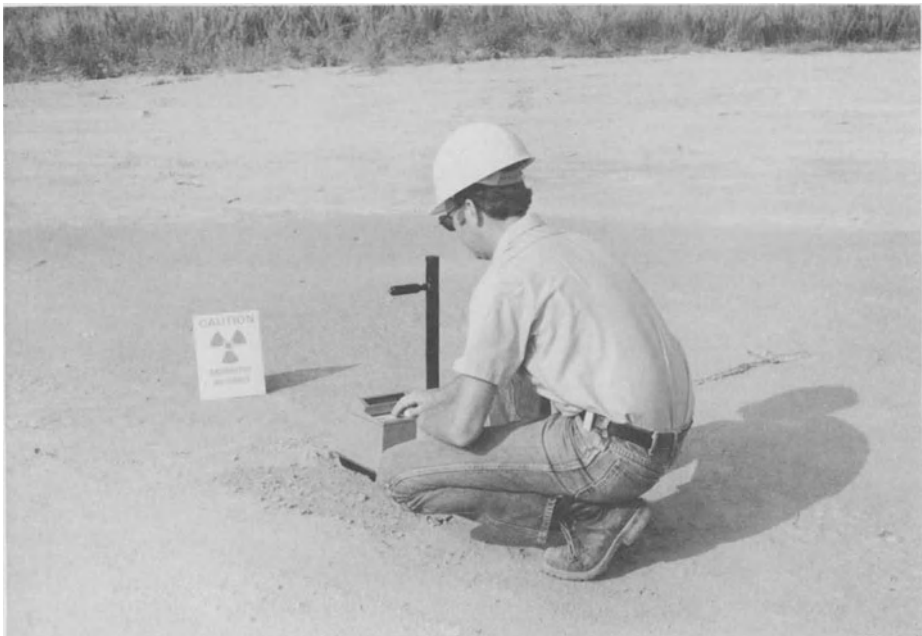
FIGURE 10-9. Soil density using nuclear methods. [Ref. 4]
