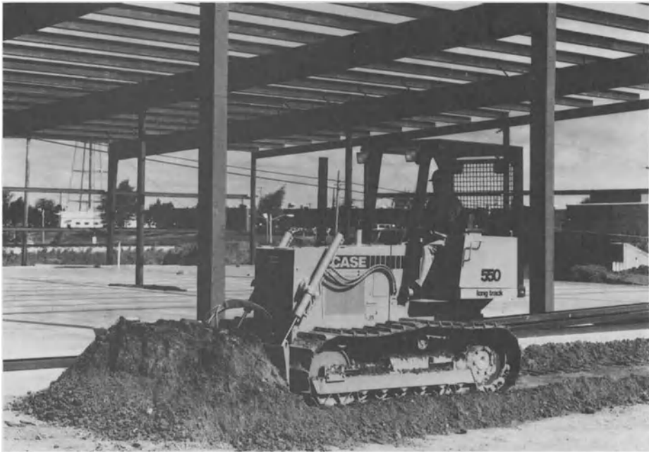
FIGURE 10-2. Spreading soil before compaction. [Ref. 7]
