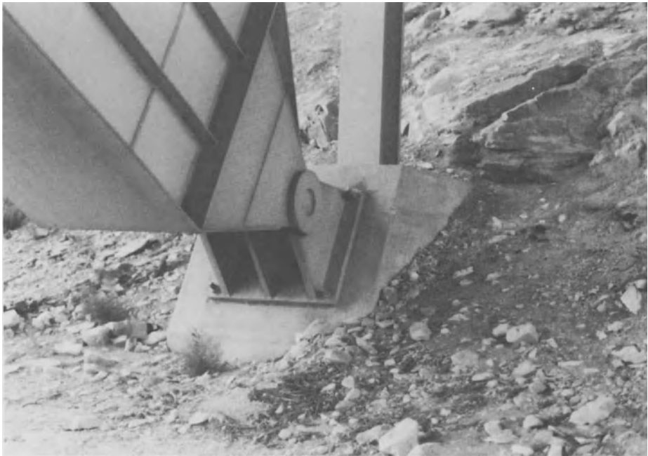
FIGURE 12-2. Arch base bearing on bedrock: (a) overview; (b) close up. [Ref. 21]
