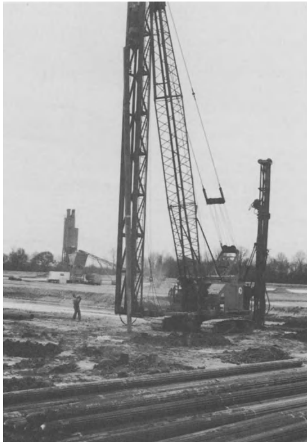
FIGURE 6-3. Installation of steel shell piles. [Ref. 15]
