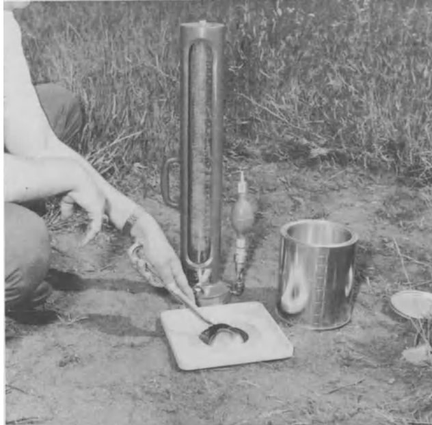
FIGURE 10-8. Soil density by the rubber balloon method. [Ref. 17]
