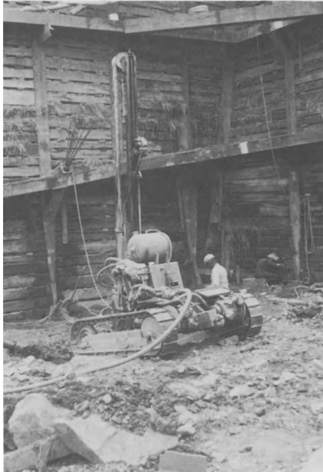
FIGURE 8-19. Rock anchor hole being drilled. [Refs. 9 and 12]
