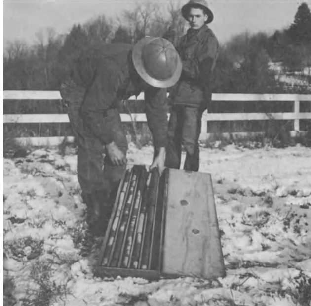
FIGURE 12-1. A typical core box, used to transport rock cores. [Ref. 1]
