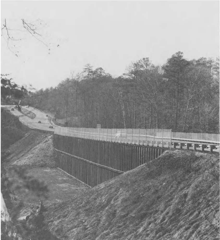
FIGURE 8-4. Bethlehem PZ27 sheet piling stabilizes this busy roadway in a marshy location near Williamsburg, Va. [Ref. 3]
