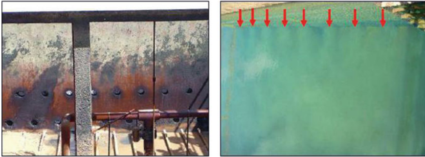
Fig. 4 Clarifier with perforated inlet baffle wall [5]
