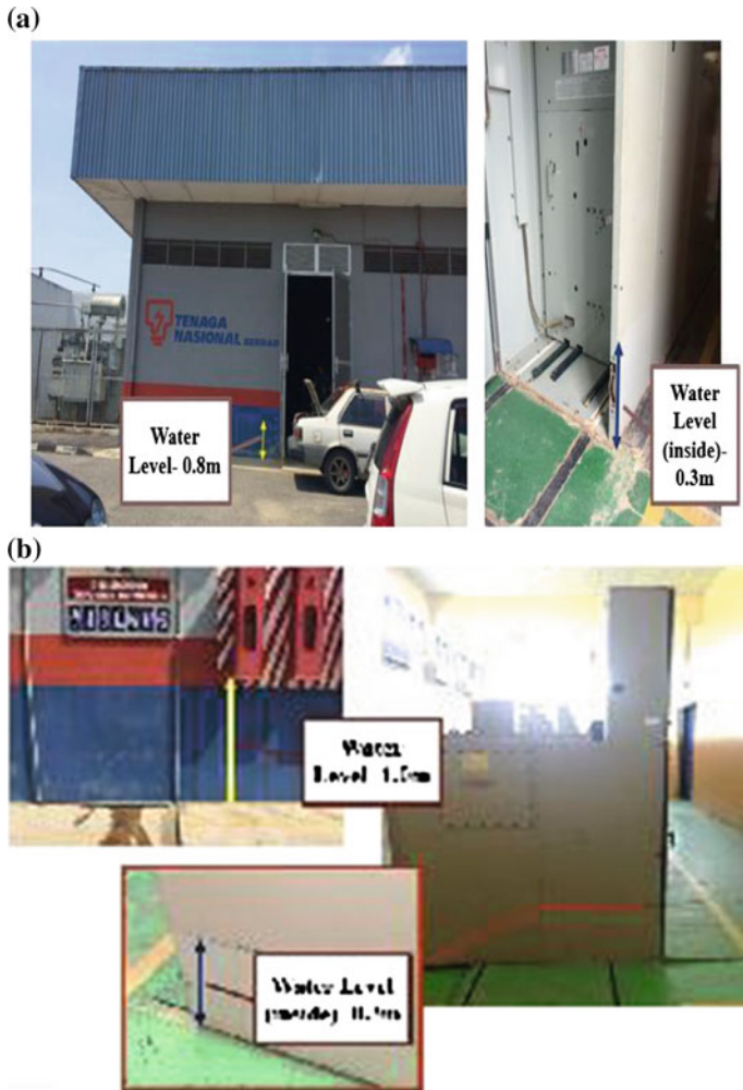
Fig. 1 a Flood mark located in PMU Tanah Merah. b Flood mark located at PMU LMAL located in Pasir Mas
