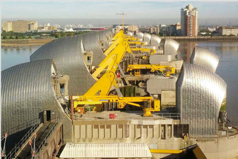
Fig. 11.8 The Thames Barrier (Environment Agency 2015, © Crown Copyright 2015. Contains public sector information licensed under the Open Government Licence v3.0)
