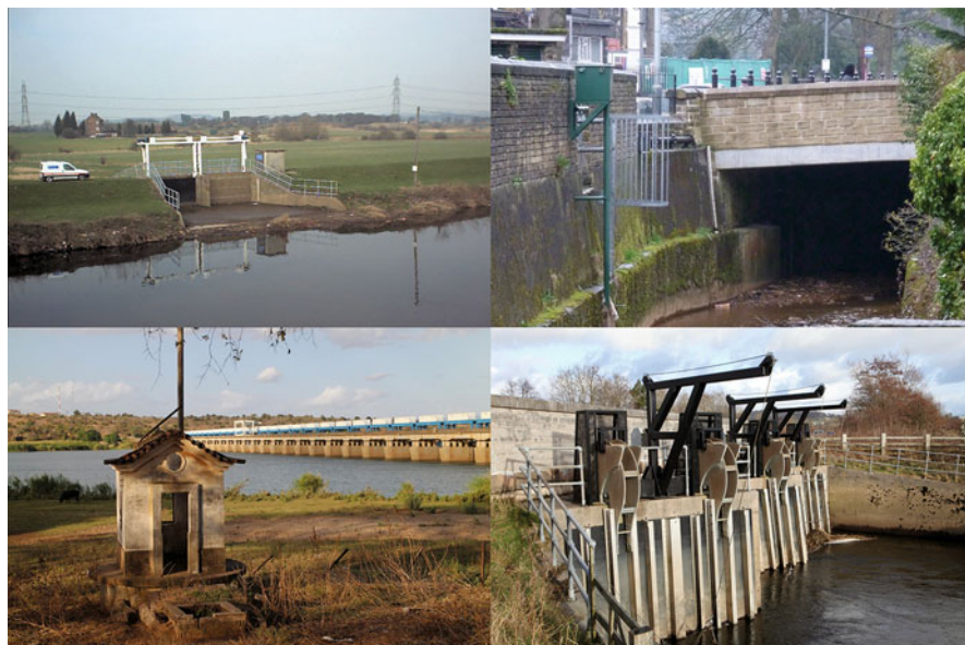
Fig. 11.1 Illustration of some types of hydraulic structures; clockwise from top left : (a) sluice gates at an off-line flood detention area, (b) culvert in urban area, (c) river tide gates, (d) irrigation-scheme barrage
