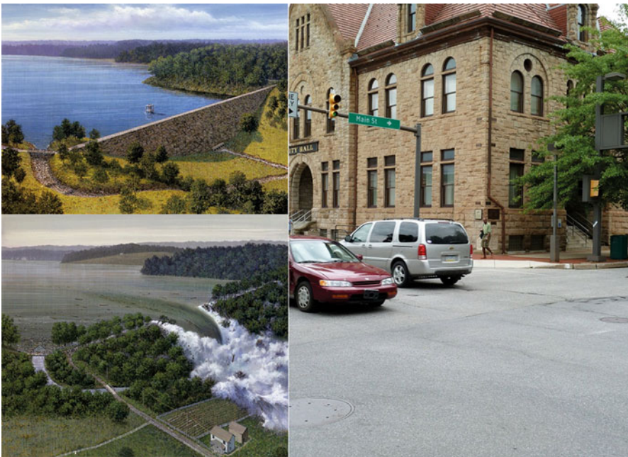
Fig. 9.14 Artists' impression of the South Fork Dam as it appeared when newly constructed and during the breach of 1889 ( left ); peak flood levels marked on a corner of the city hall in Johnstown; the highest mark (at 21 ft) was from the 1889 flood, whilst the lower marks relate to river floods ( right ) (Art by L. Kenneth Townsend, http://www.shadedrelief.com/ , Patterson 2005) (Adapted from Sene 2013)
