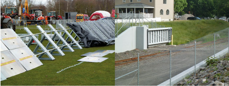
Fig. 9.3 Temporary barriers on display at an exhibition in the UK ( left ) and a flood closure gate in a levee system in the USA ( right ) (Adapted from Sene 2013)
