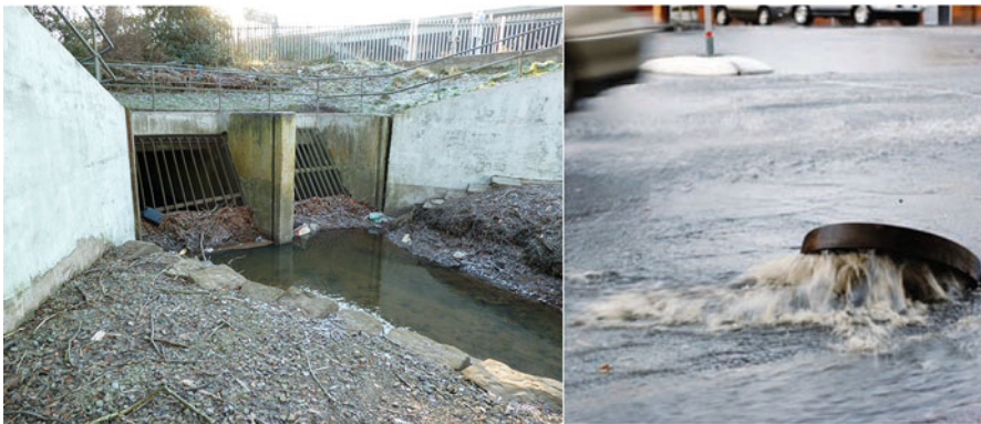
Fig. 9.8 Illustration of culvert inlet with trash screens to trap debris (Sene 2013) and outflows at a manhole cover (Defra 2010 © Crown Copyright 2010) (Adapted from Sene 2013)
