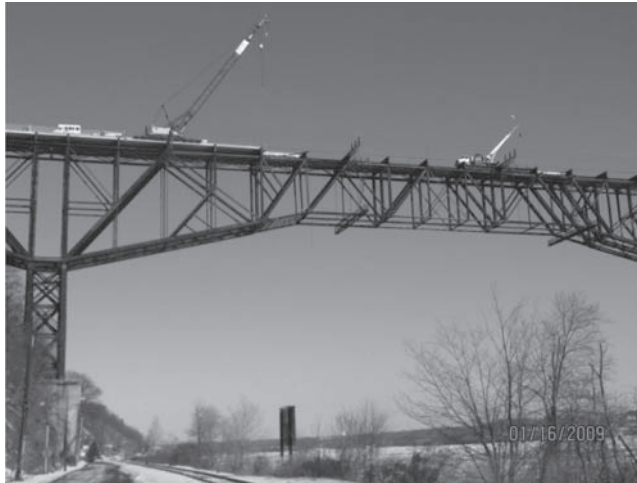
Figure 14. Steel crew (right), followed by panel installation crane (left).
