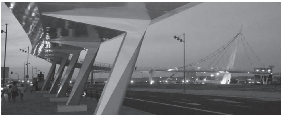
Figure 22. Image of the access ramp with the main span of the footbridge and the mast at the background.
