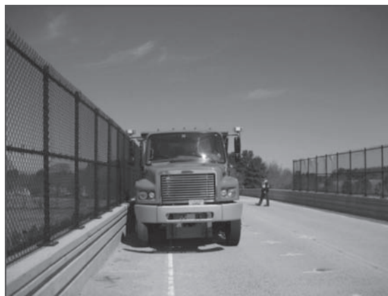
Figure 6. NHDOT sand truck as load application during April 2008 load test.
