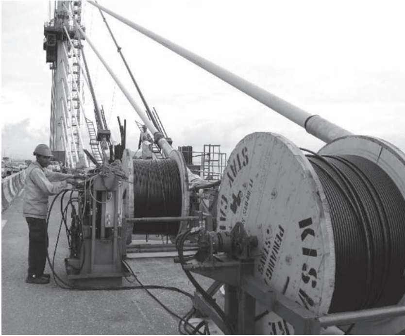
Figure 9. Parallel strand stay cable installation on a bridge under traffic.
