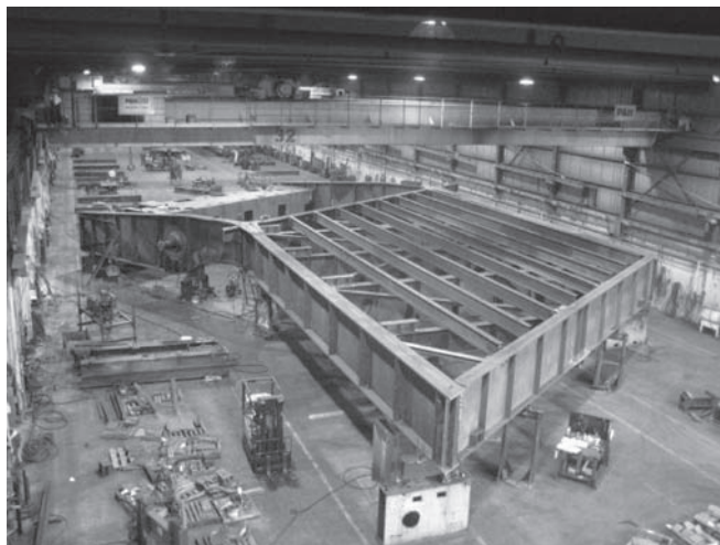
Figure 10. Shop assembly of west span.
