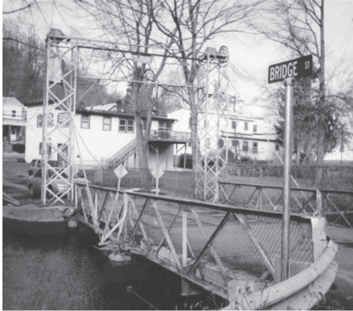
Figure 1. Bridge Street Bridge prior to rehabilitation.
