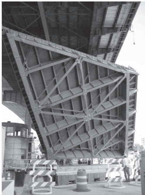
Figure 6. New east span-gowanus expressway above.
