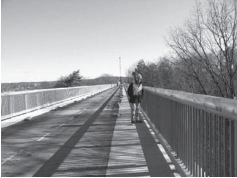
Figure 20. New deck and railing in early 2009 (at west abutment looking East).
