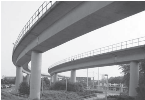
Figure 2. Dual elevated metro track structure near Ronald Reagan Washington National Airport.
