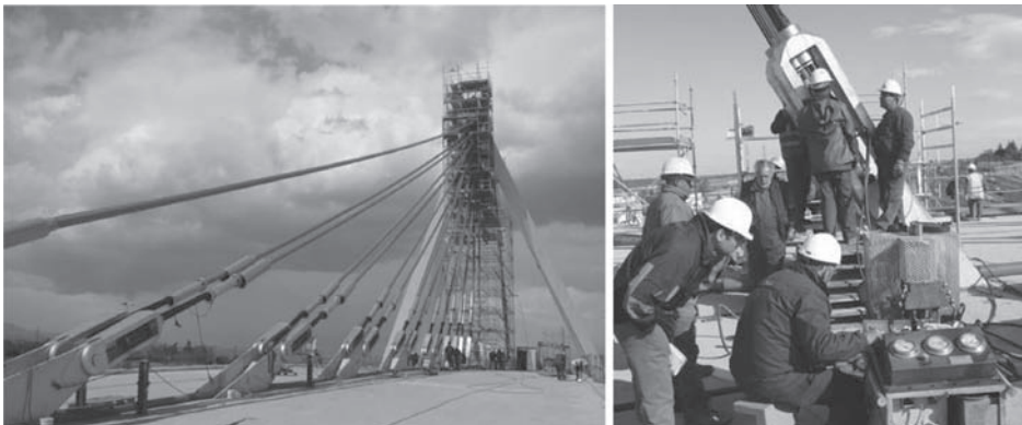
Figure 6. Tensioning of the stays using isotension system.
