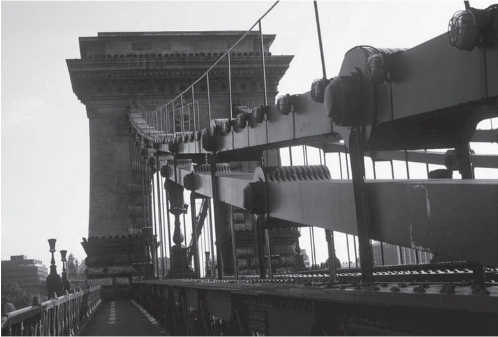
Figure 3. Eyebars of the Budapest Chain Bridge.
