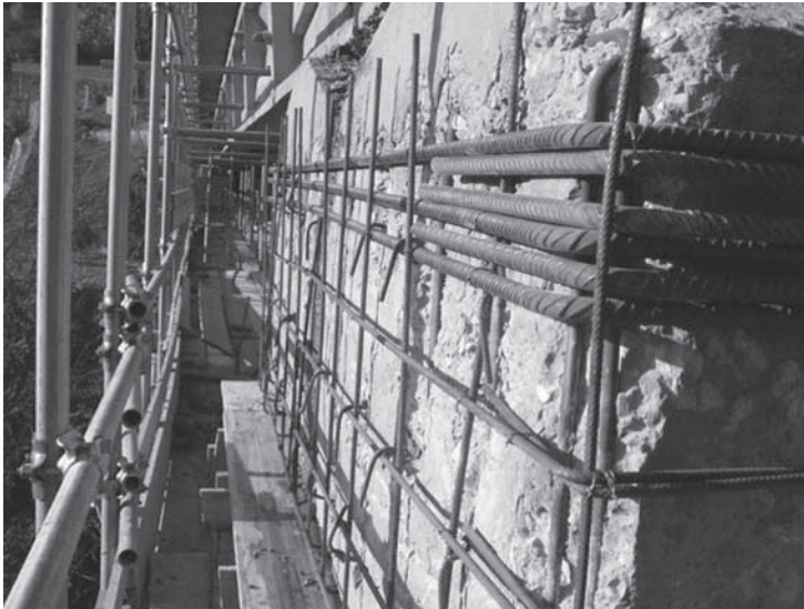
Figure 14. Abutment reinforcing.
