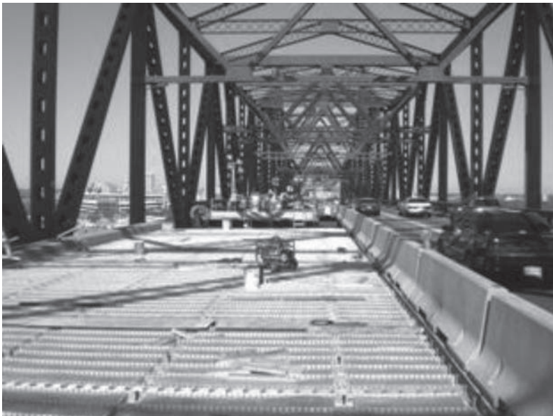
Figure 5. Bare Exodermic™ panels placed on Mathews Bridge (Photograph courtesy of RS&H).
