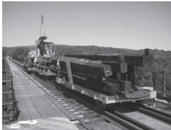
Figure 10. Demolition of rail ties.
