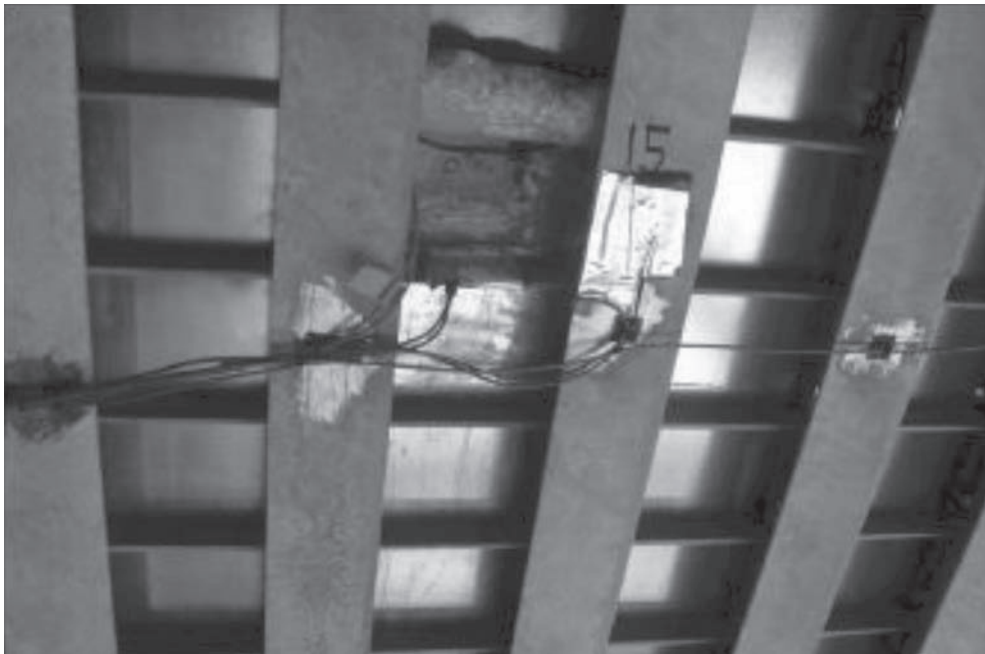
Figure 10. Strain gauge placement.
