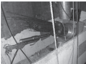
Figure 14. Freyssinet stay cables.
