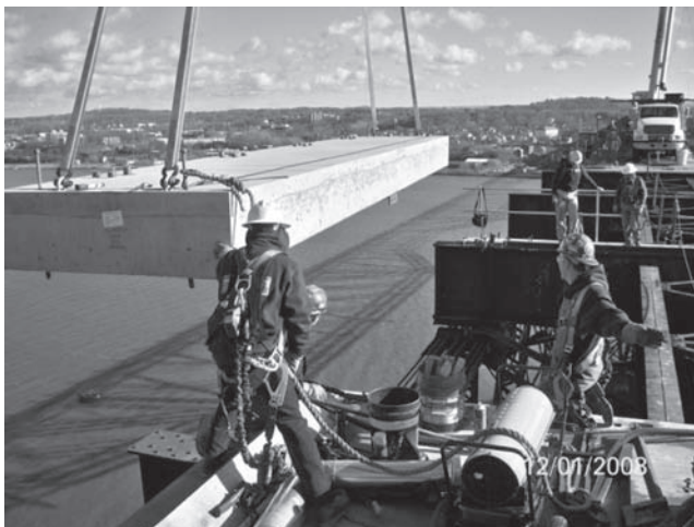
Figure 13. Panel installation on Main Span (looking East).
