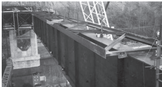
Figure 9. Example of a compression flange stiffening truss.
