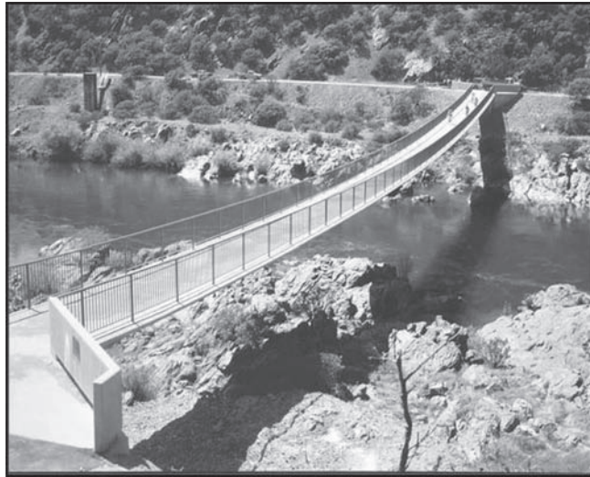
Figure 11. Sacramento River Trail Bridge, CA.
