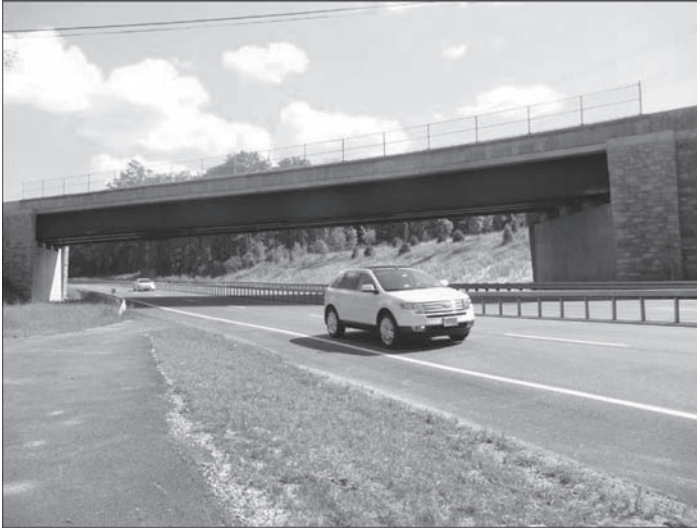
Figure 9. View of completed bridge.
