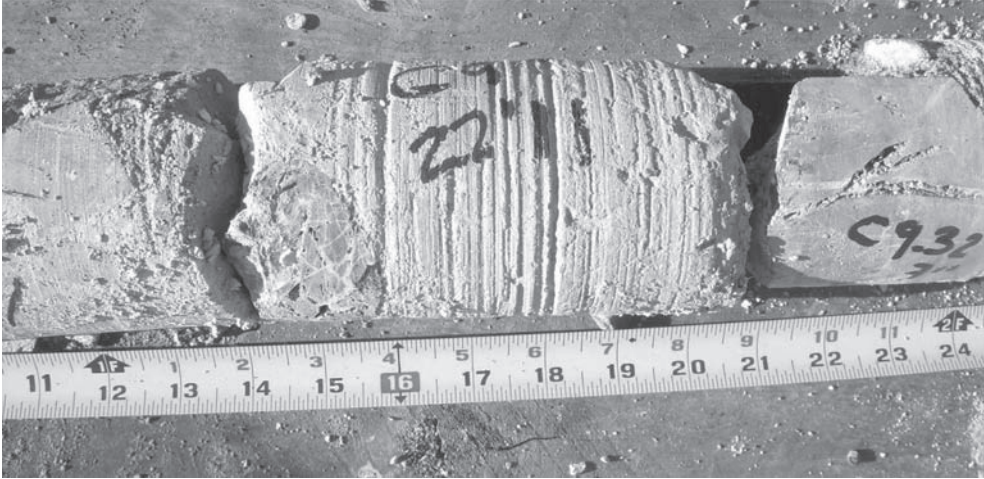
Figure 14. Concrete sample showing high level of cement paste.
