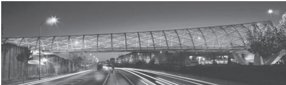
Figure 12. Elevation view of the finished footbridge.
