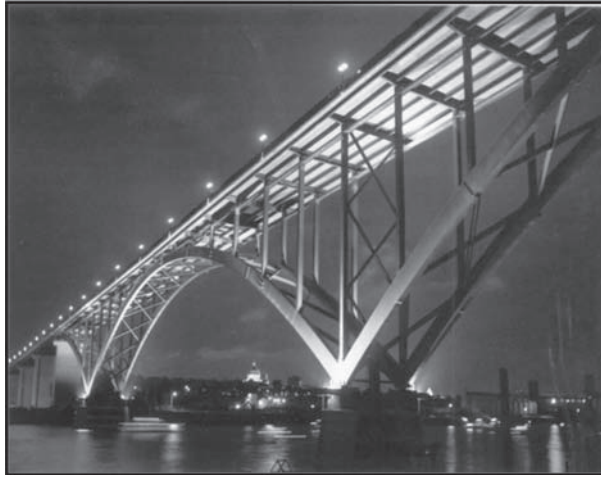
Figure 9. High Bridge, MN.
