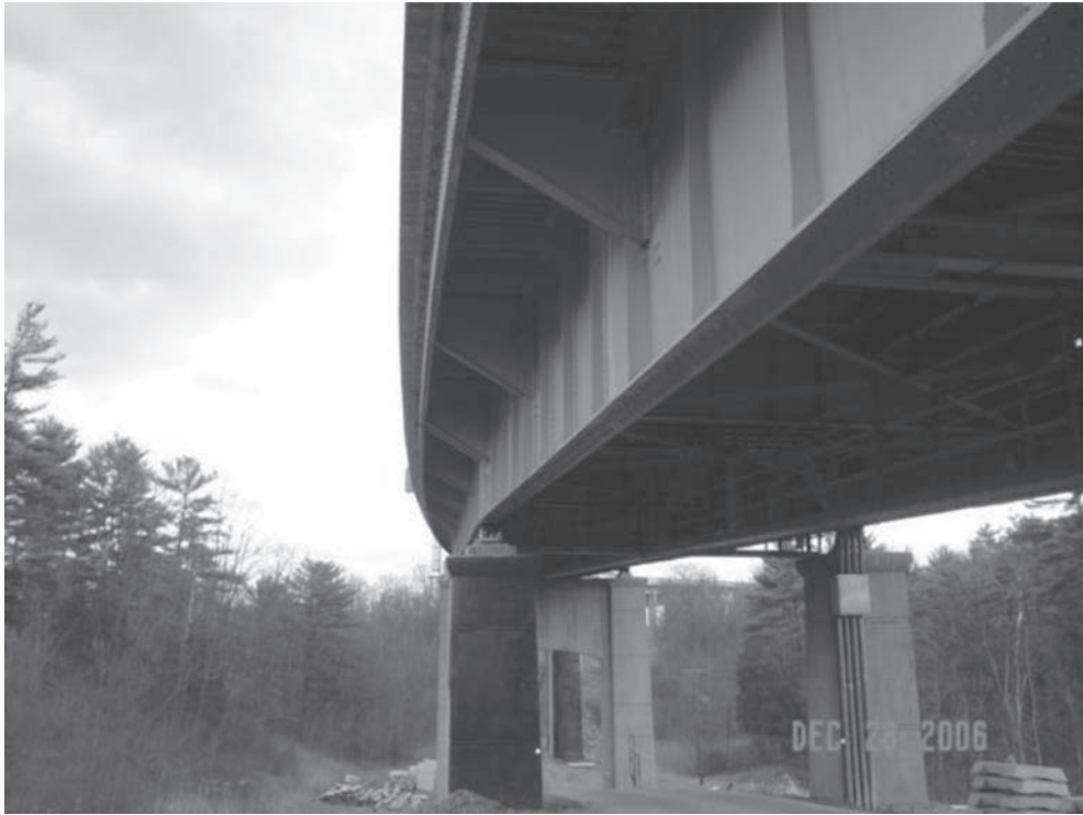
Figure 4. West approach girder spans.
