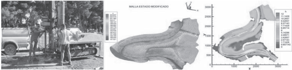
Figure 13. Additional geotechnical drilling campaign during construction (left) and hydraulic model to characterize the meander response during construction and after the bridge finishing (center and right).
