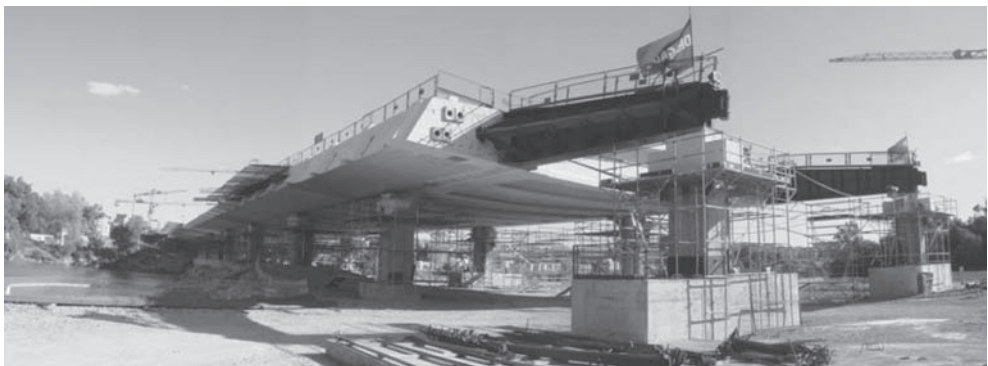
Figure 19. Launching of the deck over temporary piers.
