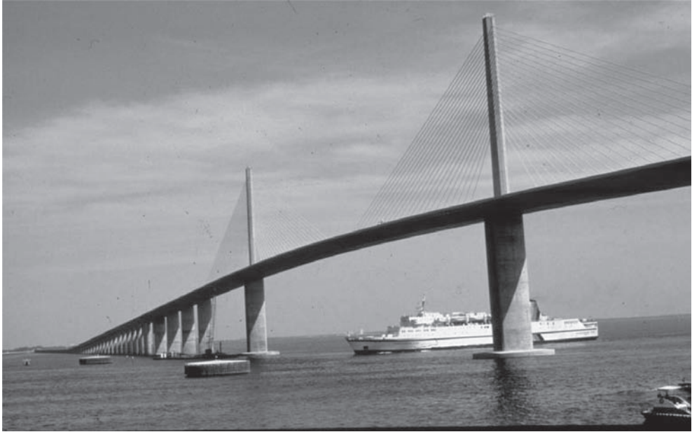
Figure 5. Sunshine Skyway Bridge, Florida (photo courtesy of Figg Bridge).
