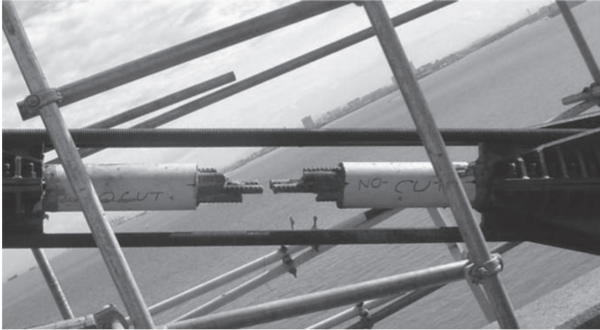
Figure 8. Controlled cable distressing in progress.
