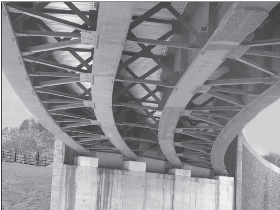
Figure 4. View bridge underside.
