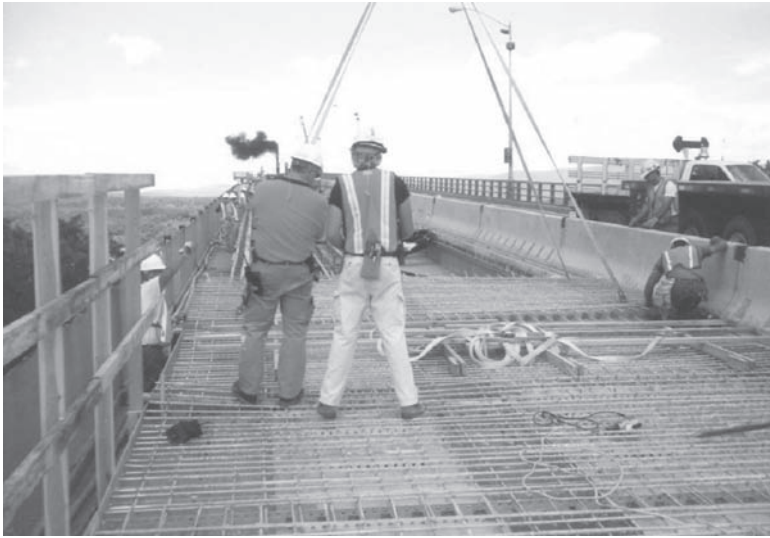
Figure 2. Placement of un-filled steel grid panels.
