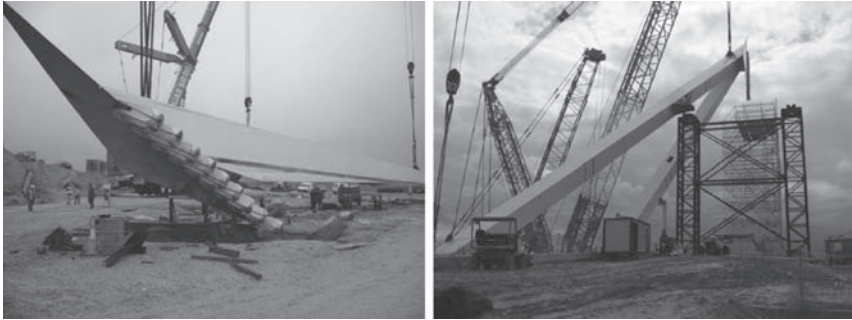
Figure 5. Erection of the mast using cranes with one temporary support.
