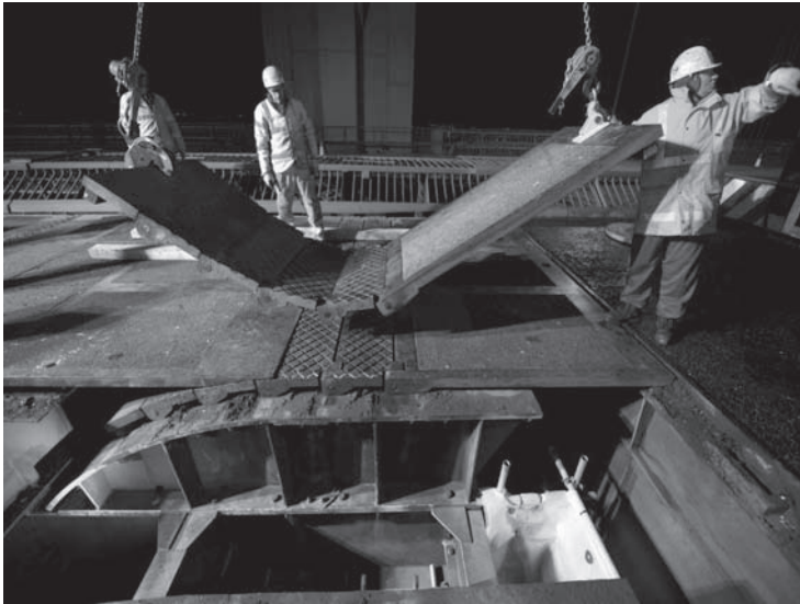
Figure 9. Plate train being removed.
