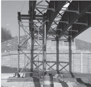
Figure 1. Temporary support structure under a single I-girder.
