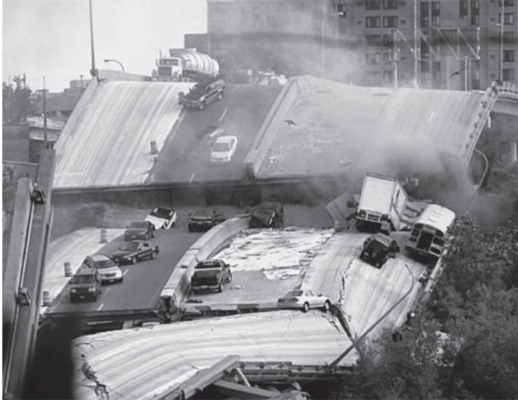
Figure 1. Collapse of the I-35W Bridge in Minneapolis.
