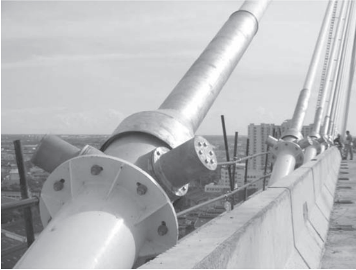
Figure 8. Hydraulic dampers.
