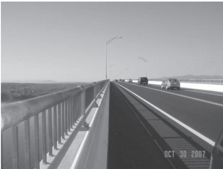
Figure 15. Kingston-Rhinecliff Deck with Nova-Chip Overlay.
