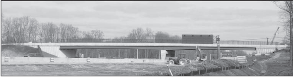
Figure 5. King Avenue over I-95, Maryland.
