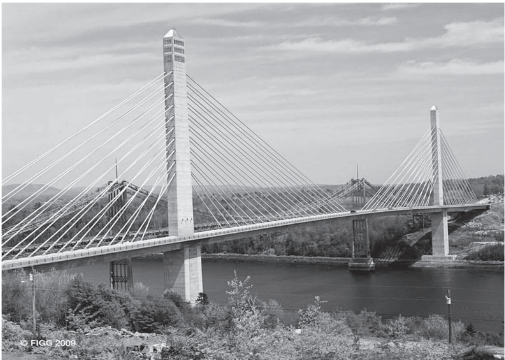
Figure 6. Penobscot Narrows Bridge, Maine (photo courtesy of Figg Bridge).
