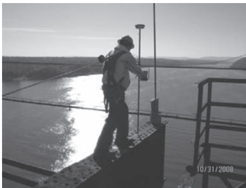
Figure 15. Existing steel survey (looking South).
