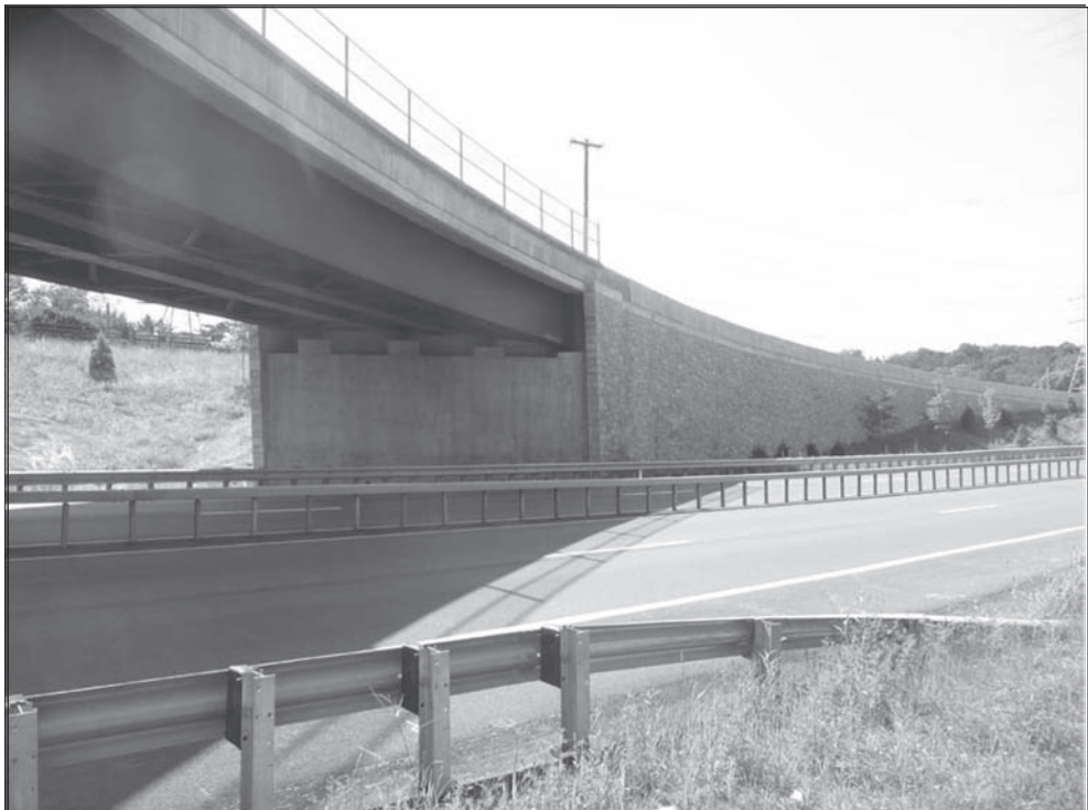
Figure 5. View of west abutment wingwall and approach retaining wall.
