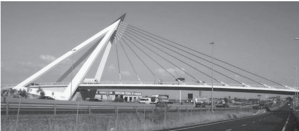
Figure 1. View of Las Rozas Bridge from the A-6 highway.
