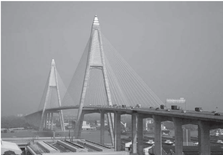
Figure 1. The Kanchanaphisek Bridge crossing the Chao Phraya River in Bangkok, Thailand.
