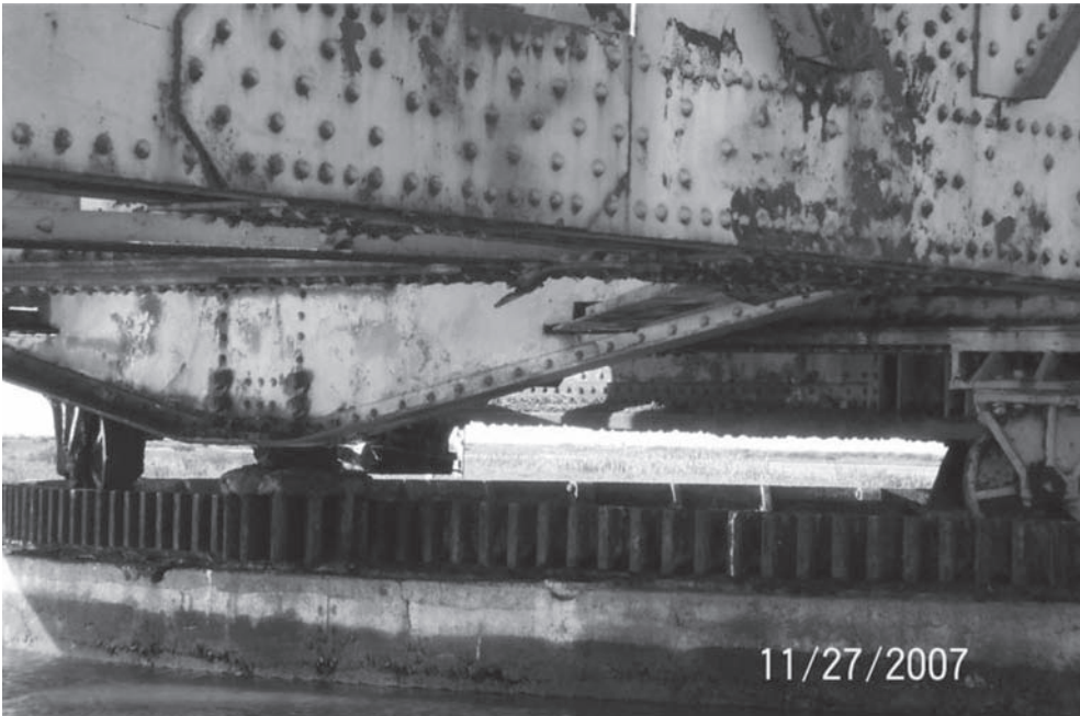
Figure 11. Newark swing span—view of floor beam and pier top.
