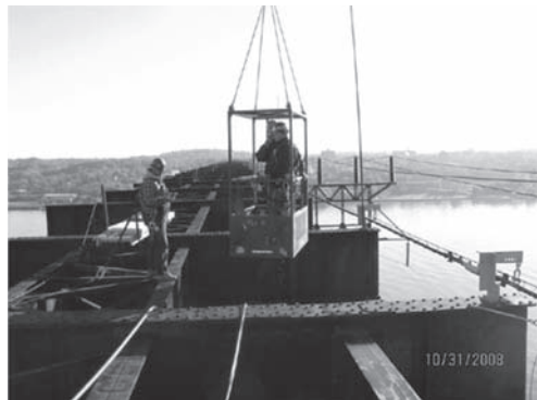
Figure 16. Structural steel repair crew (looking East).
