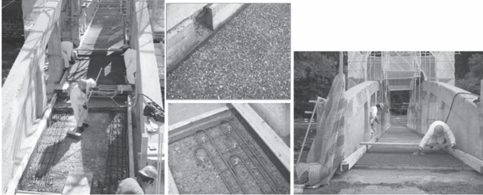
Figure 7. Rehabilitation and strengthening of a bridge deck slab with reinforced UHPFRC.
