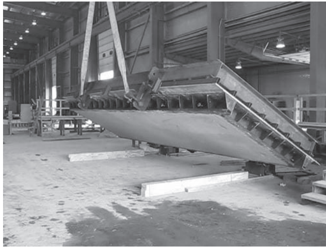
Figure 12. 25" by 6'-9" panel being rotated at the Fort Miller facility.
