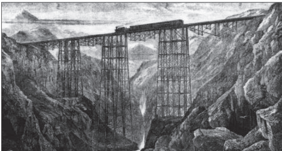
Figure 6. Rendering of completed Verrugas Viaduct.
