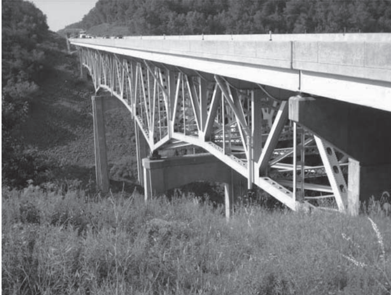
Figure 1. Elevation of the Hawk Falls Bridge.
