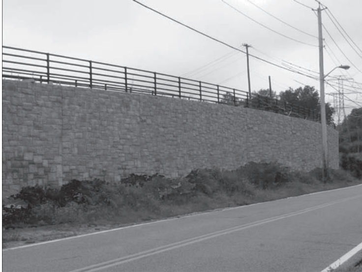
Figure 6. View of relocated bikepath retaining wall.
