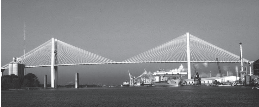
Figure 4. Cable-stayed bridge over the Savannah River.
