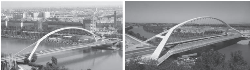
Figure 2. Barqueta bridge in Sevilla (left) and Third Millennium Bridge in Zaragoza (right).
