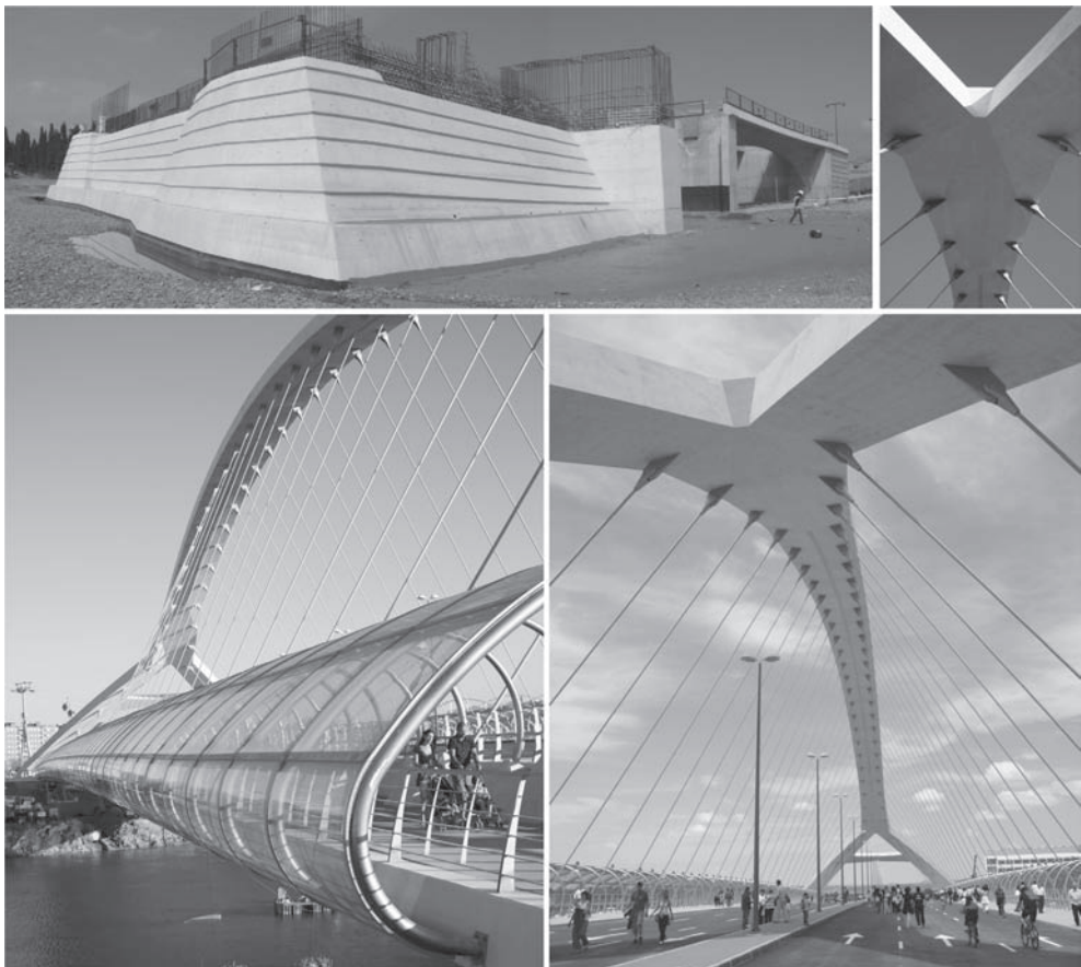
Figure 6. From left to right and from top to bottom, left bank abutment, detail of the transition between pure arch and inclined legs, one of the side glazed balconies and perspective of the three dimensional space inside the bridge.
