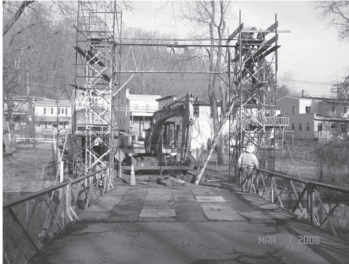
Figure 6. Demolition of steel towers.
