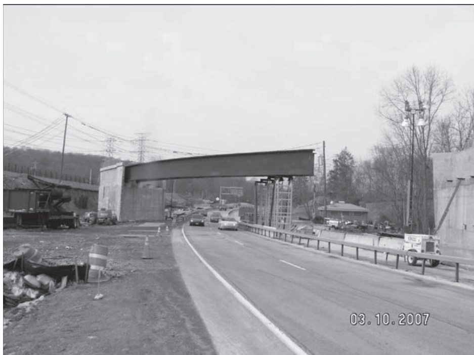
Figure 8. View of partially erected superstructure steel.
