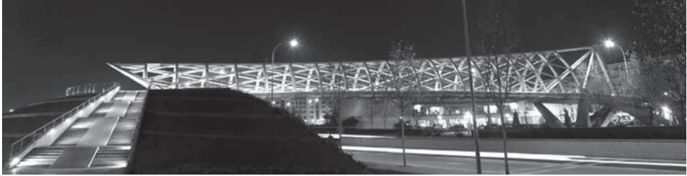
Figure 16. Night view of the access artificial hill in the south abutment.
