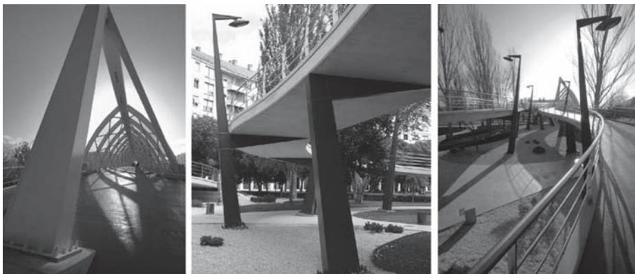
Figure 15. Access ramps and north abutment.
