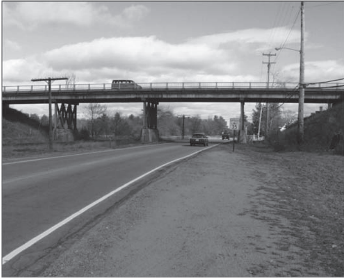
Figure 2. Rollins Road Bridge prior to new bridge construction (Bowman M.M., 2002).
