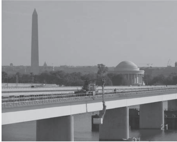
Figure 1. WMATA Bridge crossing the potomac river from Virginia into Washington, DC.
