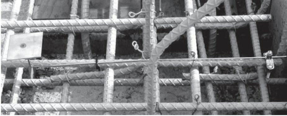
Figure 1. Stainless steel contact attachment to the rebar of bridge deck.
