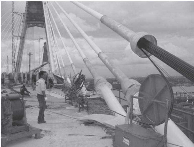
Figure 7. Stay cable strand is pulled into the PE pipe.
