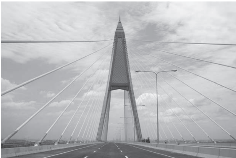
Figure 16. Elevation of the Completed Bridge.
