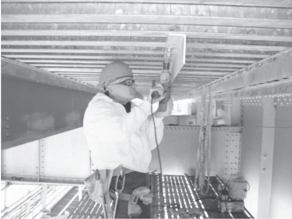
Figure 9. Retrofit L5 \times 3 \times \frac{5}{16} installation.
