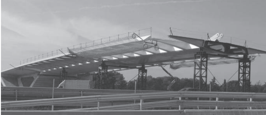
Figure 4. View of the steel deck during construction, and end abutment.
