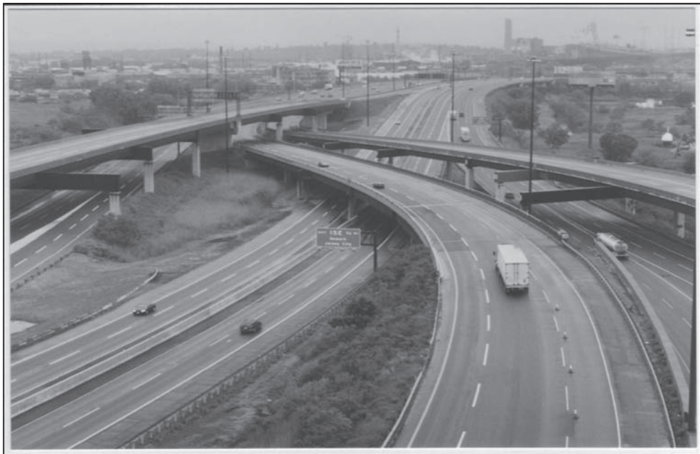
Figure 1. The New Jersey Turnpike varies from two 2-lane roadways to six 3-lane roadways by Newark Airport, with dual-dual roadways over a 32 mile length through the busiest zone.
