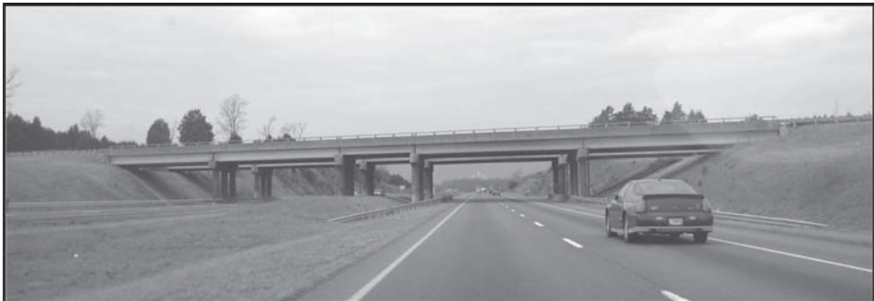
Figure 4. Typical “bottom line” overpass structure.
