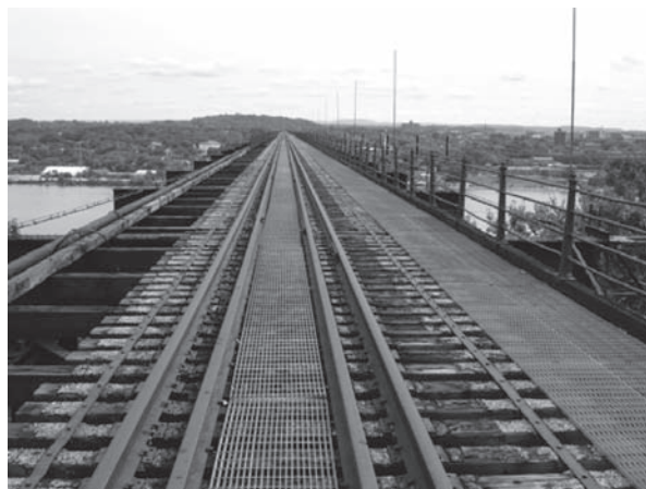
Figure 19. Existing bridge deck in 2007 (looking East).
