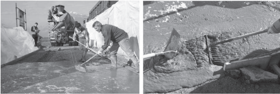
Figure 4. UHPFRC casting and handling of UHPFRC using simple tools.
