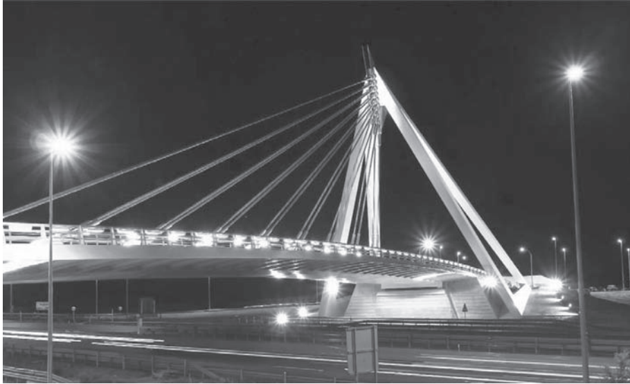
Figure 3. Night view of Las Rozas bridge.
