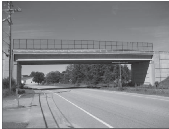
Figure 3. New Rollins Road Bridge, opened in 2000.
