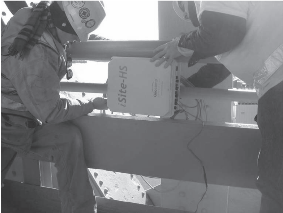
Figure 10. Installation of data loggers on the Little Mystic Span at connection L6.
