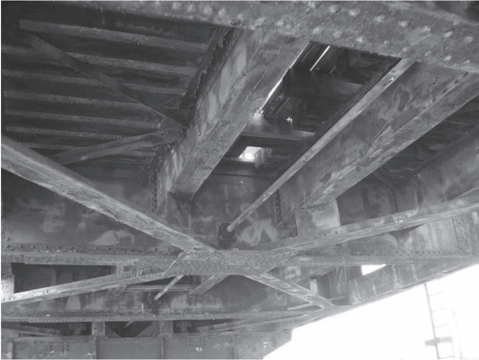
Figure 10. Dumbarton swing span—view of floor beam.
