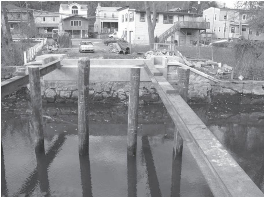
Figure 15. View looking north at piles for new timber pier.
