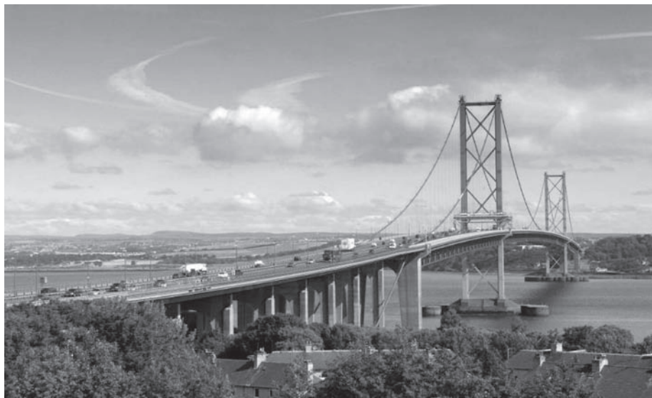
Figure 2. View of the bridge looking north.
