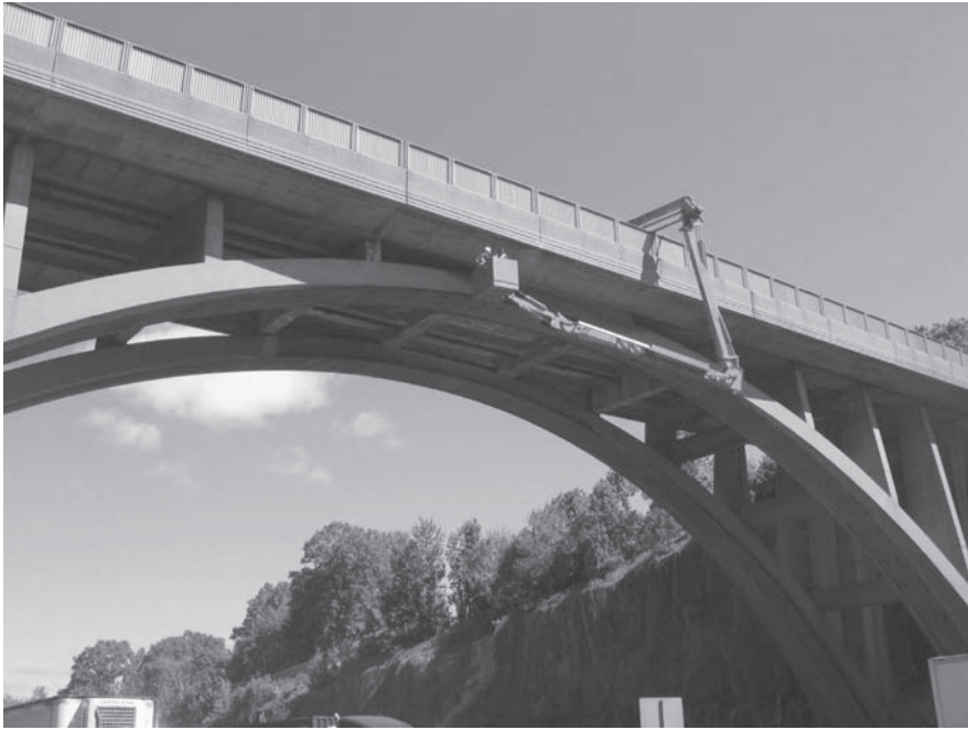
Figure 5. Inspection of an I-95 extension bridge included in the pilot program.
