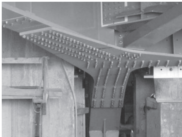
Figure 7. Interior knee joint connection.
