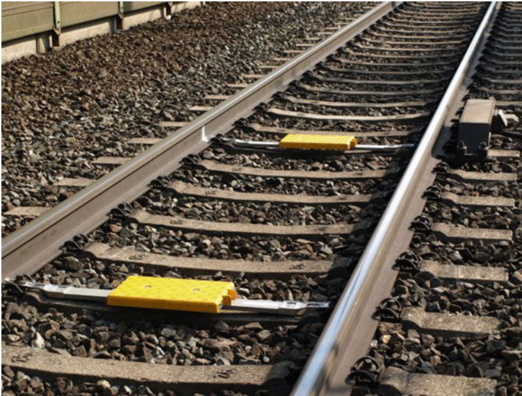
Fig. 6.14 Balise Group composed of two balises
