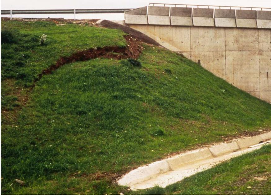
**Figure 3.2** Collapsed fill around a bridge abutment.
