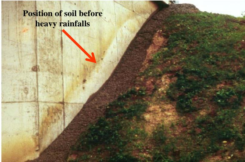
**Figure 3.4** Collapse of embankments after rainfall.
