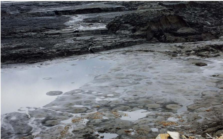
**Figure 6.3** Mud volcanoes observed a few hours after the failure on the surface of the depressed basin, upstream of the slid dam (Courtesy of J. M. Rodriguez Ortiz).
