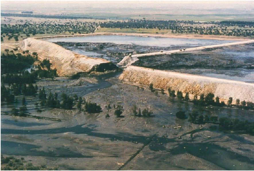
**Figure 4.3** Breach open in the dam. The foreground shows the valley of the Agrio river, covered by a thick deposit of mine waste (acid liquefied pyrites) (Alonso and Gens, 2006).
