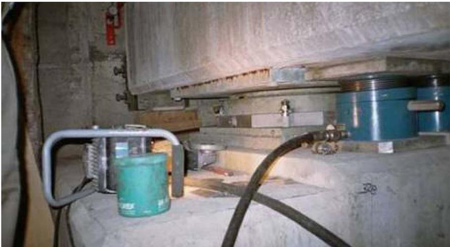
**Figure 1.15** The Leaning Tower: (a) new foundations; (b) the jacking-up procedure.
