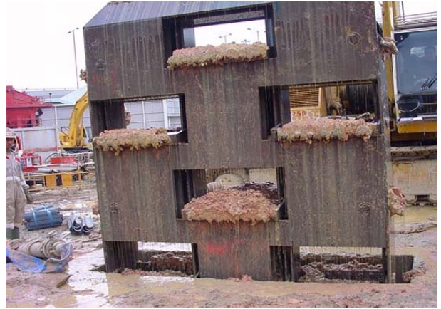
Plate 4.2 A Trench Scraping Unit in Barrette Construction
