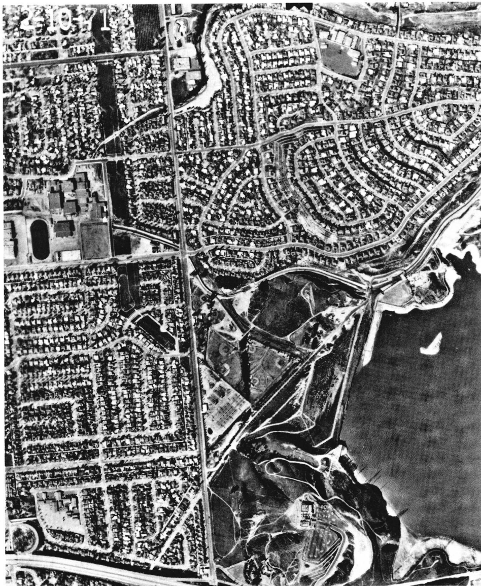
FIGURE 43. Damaged Lower San Fernando Dam one day after the February 9, 1971 San Fernando, California earthquake ( M_L = 6.4 ) and its relation to the densely built-up area downstream. The complex at the left edge of the photograph is a school. (National Aeronautics and Space Administration photograph; from Rush, M., Holguin, A., and Vernon, S., Potential Role of Remote Sensing in Disaster Relief Management , School of Public Health, University of Texas, Houston, no date, 49A. With permission.)
