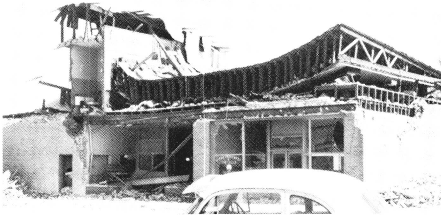
FIGURE 6. Unreinforced brick Lodge Hall in Tehachapi following the July 21, 1952 Kern County, California earthquake ( M_L = 7.7 ). Wood partition at left shows original roof height of this two-story structure. The roof collapsed after supporting walls failed. (Courtesy of National Oceanic and Atmospheric Administration, Environmental Data Service.)
