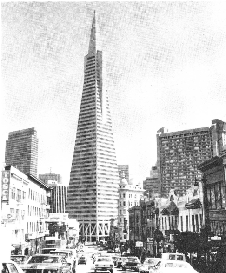
FIGURE 11. The 48-story (plus 65-m spire) Transamerica Pyramid in San Francisco. The establishment and distribution of lateral forces for this structural steel frame building were determined by dynamic analysis . The windowless protrusions rising from the 29th story house elevators on one side of the building and a stair well and smoke tower on the opposite side. (Courtesy of Dale Honeycut, Northern Arizona University.)
