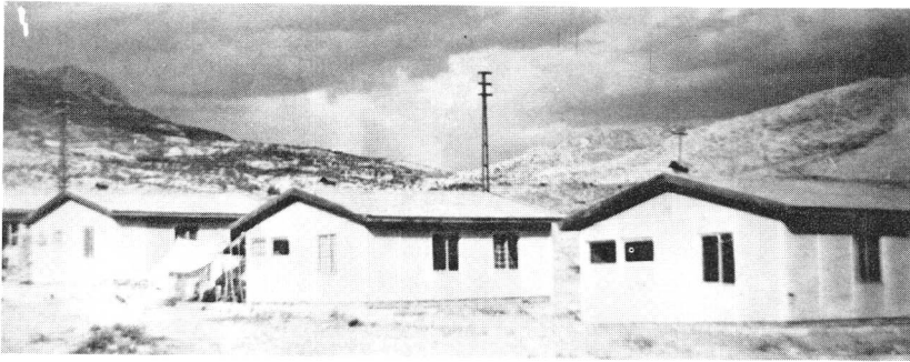
FIGURE 40. Undamaged earthquake-resistant dwellings in Hani following the September 6, 1975 Lice, Turkey earthquake ( M_s = 6.7 ). (Courtesy of Peter I. Yanev; URS/John A. Blume & Associates, San Francisco.)
