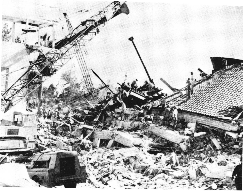
FIGURE 16. Rescue operations at the San Fernando Veterans Administration Hospital complex following the February 9, 1971 San Fernando earthquake ( M_L = 6.4 ). The collapse of four pre-1933 unreinforced masonry buildings was responsible for 44 deaths. Newer buildings and additions in the complex that were designed and constructed in accordance with earthquake-resistant provisions did not collapse. (Los Angeles City Department of Building and Safety photograph. From Brugger, W., The San Fernando, California, Earthquake of February 9, 1971 , Geological Survey Professional Paper 733, U.S. Government Printing Office, Washington, D.C., 1971, 218.)
