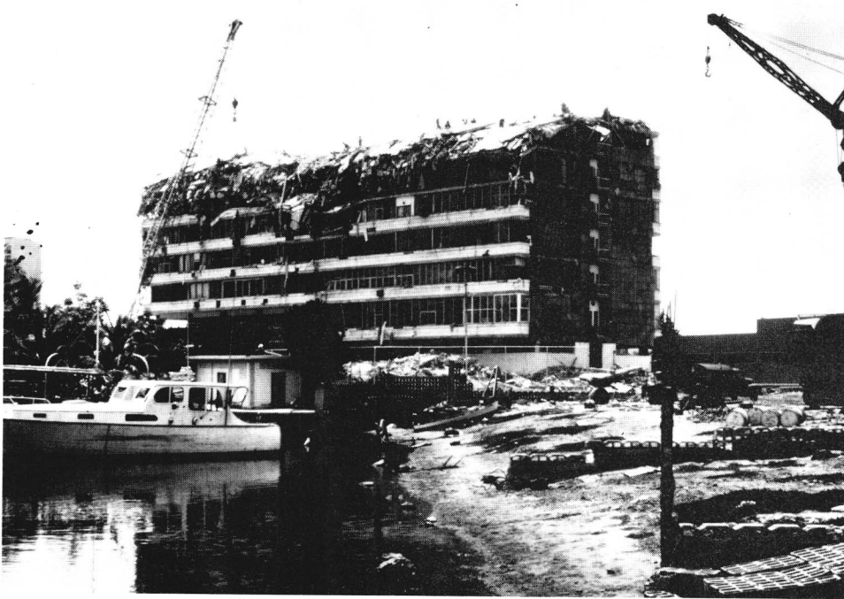
FIGURE 6. Reinforced concrete Mansion Charaima Apartment building in Caracas, Venezuela following the July 29, 1967 earthquake ( M_L = 6.5 ). The top four floors “pancaked” causing 42 deaths. 933 (Courtesy of the National Oceanic and Atmospheric Administration, Environmental Data Service.)
