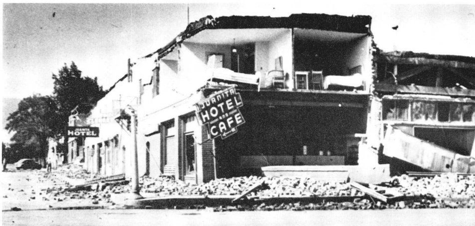
FIGURE 7. Collapsed unreinforced brick bearing wall of the Juanita Hotel in Tehachapi following the July 21, 1952 Kern County, California earthquake ( M_L = 7.7 ). Note support given by the nonstructural wood partitions after collapse of exterior bearing walls. (University of California, Berkeley, photograph; courtesy of National Oceanic and Atmospheric Administration, Environmental Data Service.)
