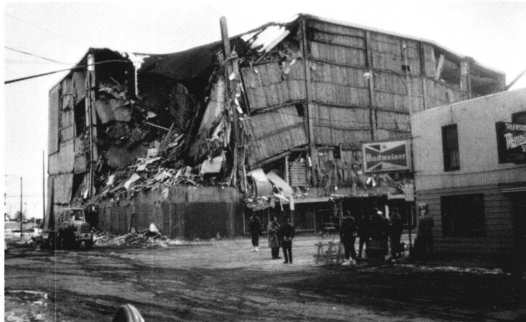
FIGURE 8. Northeast corner of the five-story reinforced concrete J.C. Penney building in Anchorage following the March 27, 1964 Alaskan earthquake ( M_s = 8.5 ). Most of the rubble has been cleared from the streets. (Courtesy of George Plafker, U.S. Geological Survey.)
