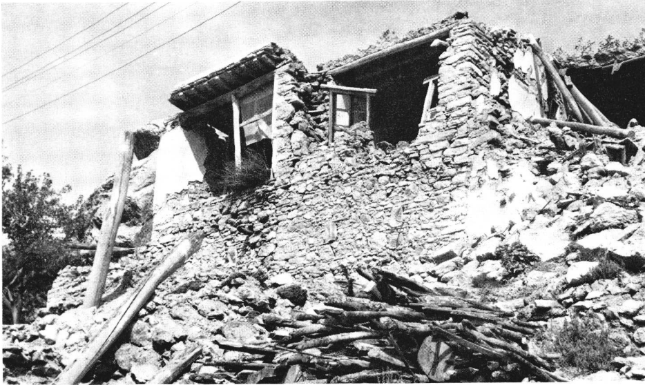
FIGURE 39. View of a traditional stone dwelling in Lice following the September 6, 1975 Lice, Turkey earthquake ( M_s = 6.7 ). Total roof collapse is evident at photo (right); note pile of roof support timbers. (Courtesy of Peter I. Yanev; URS/John A. Blume & Associates, San Francisco.)
