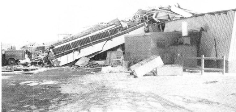
FIGURE 10. Collapsed six-story reinforced concrete control tower at Anchorage International Airport following the March 27, 1964 Alaskan earthquake ( M_s = 8.5 ). (Courtesy of George Plafker, U.S. Geological Survey.)
