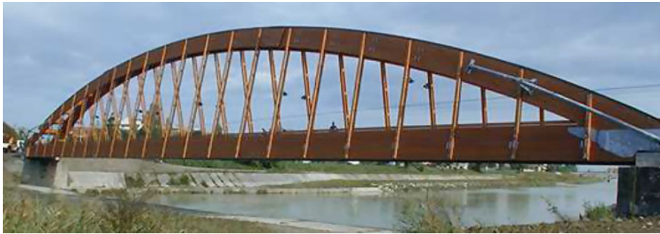
Fig. 26.1 Overview of the Marecchia River bridge
