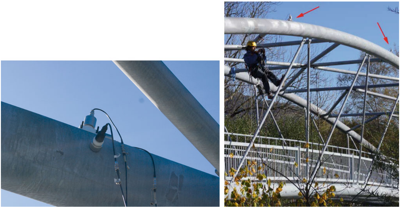
Fig. 27.3 Attaching sensors to the top chord
