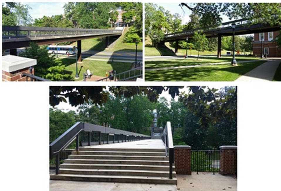
Fig. 17.1 Views of the bridge from each side and then from the deck
