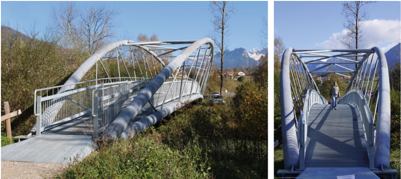
Fig. 27.1 Footbridge on the Sarine River at Broc, Switzerland
