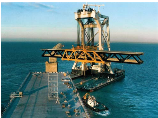
Figure 10.12 Øresund Bridge, approach span erection using the heavy-lift vessel “Svanen.”
