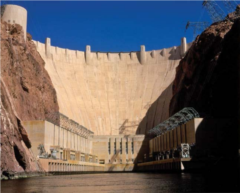
Figure 1.5 The Hoover Dam on the Colorado River, then the largest concrete structure in the world, requiring 2,480,000 m 3 of concrete, constructed from 1931 to 1936. (Courtesy of the United States Bureau of Reclamation.)
