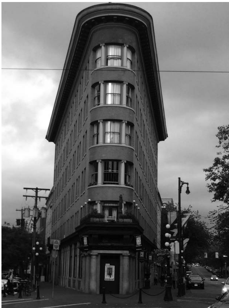
Figure 1.4 The Hotel Europe, Vancouver, the first reinforced concrete structure in Canada, 1908–1909. (Courtesy of Katherine Mindess.)
