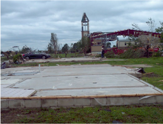
Fig. 7 Demolished home located within the tornado damage path in Joplin. Note the lack of underground access
