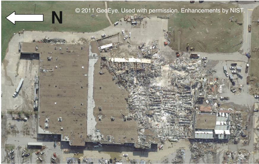
Fig. 6 Aerial photo of the tornado-damaged Walmart Store #59, showing the collapsed south half and uncollapsed north half of the building.
