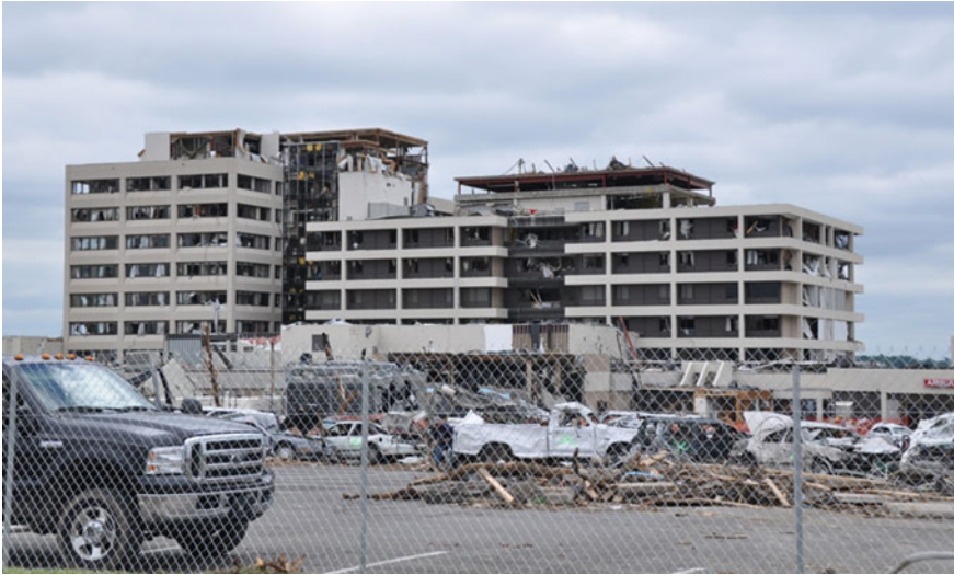
Fig. 5 Damage to the towers of the SJRMC due to the tornado (West Tower on the right )
