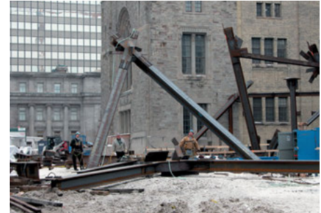
Ironworkers on the Royal Ontario Museum are preassembling members prior to erection. This procedure was critical to the success of the project because of the highly heterogeneous nature of the assemblies and lifts. Combinations of nodes and diagrid members would have been too large to be transported to the site as units.
