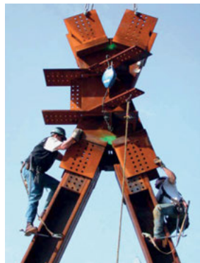
The prefabricated node for the Swiss Re Tower (30 St. Mary Axe) in London, England, designed by Foster + Partners and engineered by Arup, provides four identical attaching points for the incoming diagrid members and an alternate system to connect the bracing hoops, which in this case are acting in tension.
