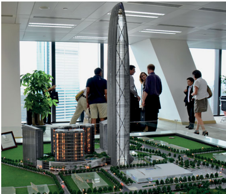
This site model for the KK100 Tower in Shenzhen, China, designed by TFP Architects with Arup, shows the use of a diagonalized core on a Supertall building. The photo was taken inside KK100 in the presentation center. The actual size of a diagonal can be seen in the background.
