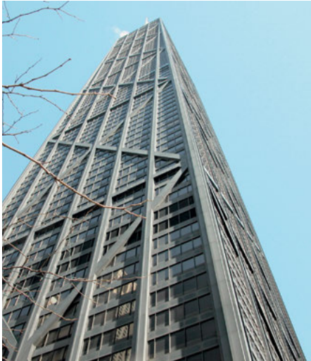
The diagonal braces of the John Hancock Center in Chicago, IL, USA, designed by SOM and completed in 1969, clearly express the lateral bracing system as part of the aesthetic of the façade.
