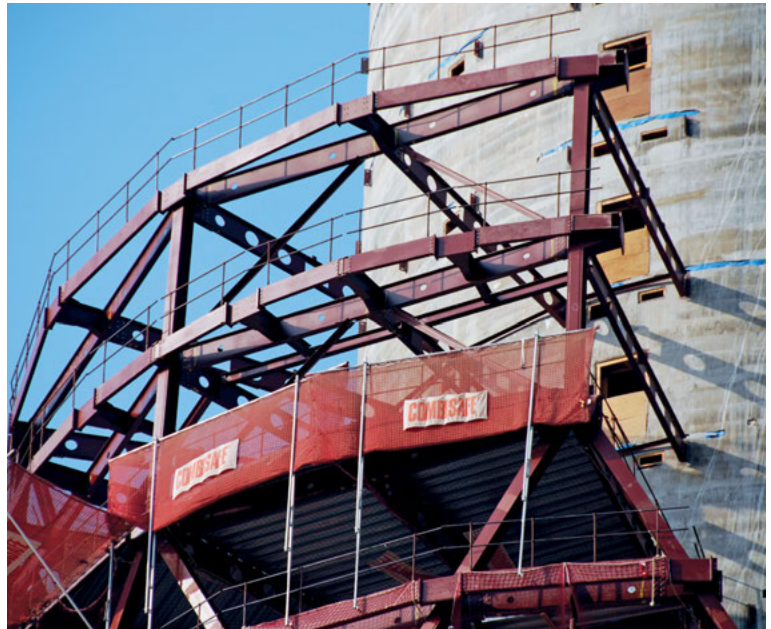
The attaching plates for the steel beams that will clear span from the concrete core to the perimeter framing must be carefully integrated into the casting of the concrete core as it proceeds. Here you can see that the round shape of the Al Bahar Tower is created through faceting rather than bending the steel. Steel fabrication and erection by William Hare Limited.
