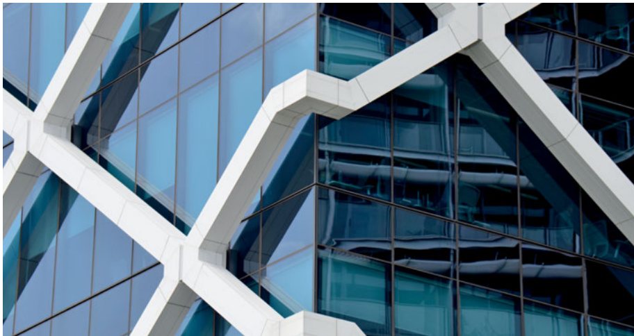
The exterior diagrid at One Shelley Street in Sydney, Australia, designed by Fitzpatrick + Partners with Arup, permits the use of a rectilinear curtain wall system and standard window shades on the interior.
