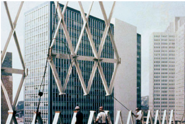
The diagrid for the IBM Building was prefabricated into modules for ease of site assembly, with primary structural connections occurring at the mid-points between the floor levels.
