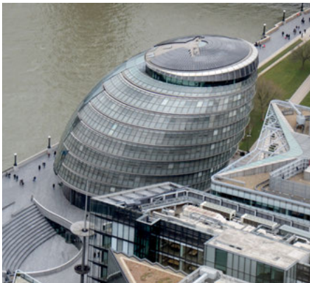
London City Hall in London, England, designed by Foster + Partners with Arup and completed in 2002. The structure leans away from the water to form a stepped façade on the south side to create sustainable self-shading.
