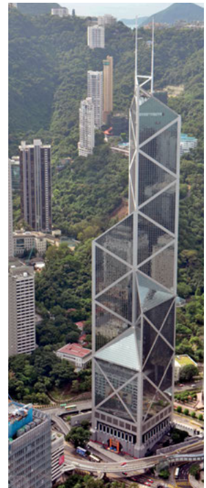
The Bank of China Tower in Hong Kong, China, designed by I.M. Pei and engineered by Leslie E. Robertson Associates, completed in 1990, uses the structure and lines of the diagonal bracing system to support changes in the form of the building.
