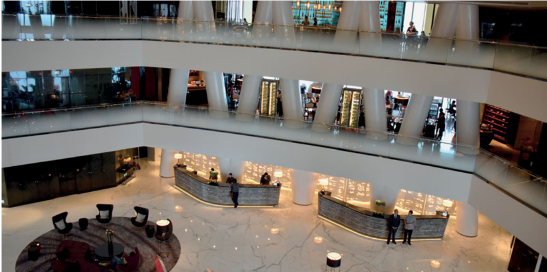
At the upper level of the Guangzhou IFC, the central core splits and the elevators and staircases move to the sides to make room for a large atrium.
