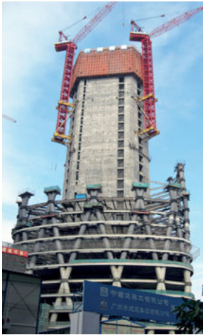
A building of the height of the Guangzhou IFC uses a combination of a perimeter diagrid and a reinforced concrete core to resist lateral loads. The selection of reinforced concrete for the core also works toward the fire engineering strategies of the building.
