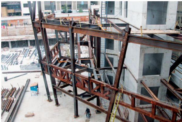
The Royal Ontario Museum by Daniel Libeskind incorporated a concrete core into the building. Although the initial diagrid elements used the core for stability during construction, much of the completed complex structure did not rely on the core to assist with overall stability.
