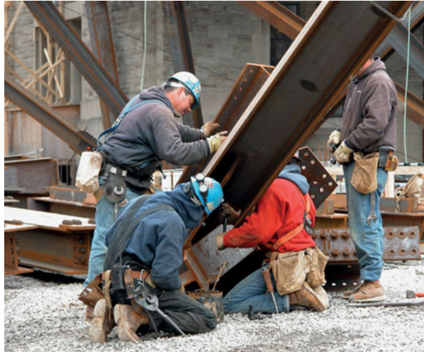
Ironworkers on the Royal Ontario Museum are preassembling members prior to erection. This procedure was critical to the success of the project because of the highly heterogeneous nature of the assemblies and lifts. Combinations of nodes and diagrid members would have been too large to be transported to the site as units.
