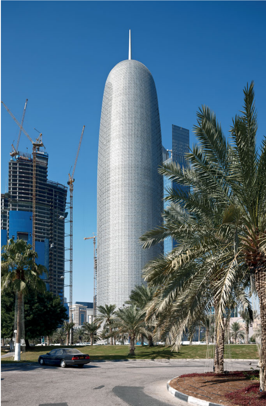
South façade of the Doha Tower showing the highly detailed outer skin of the double façade. The mashrabiya is more dense on this façade to limit solar penetration.
