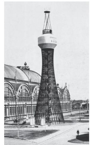
First diagrid tower designed by Vladimir Shukhov in 1896.
