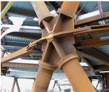
The prefabricated node for the Swiss Re Tower (30 St. Mary Axe) in London, England, designed by Foster + Partners and engineered by Arup, provides four identical attaching points for the incoming diagrid members and an alternate system to connect the bracing hoops, which in this case are acting in tension.
