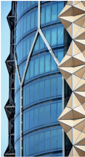
The Al Bahar Towers in Abu Dhabi, UAE, designed by Aedas Architects with engineering by Arup, use a light-responsive mashrabiya shading system to create what is essentially a second façade on all but the north façade, which is left exposed.
