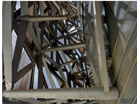
This view of the mashrabiya panels in their fully open position (top left) was taken prior to commissioning of the building. The intelligent system results in highly uniform, automated opening and closing of the screen as a function of the time of day and light conditions.
