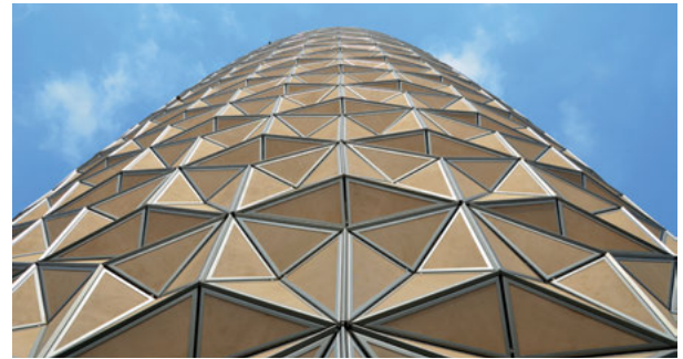
This view of the mashrabiya panels in their fully open position (top left) was taken prior to commissioning of the building. The intelligent system results in highly uniform, automated opening and closing of the screen as a function of the time of day and light conditions.
