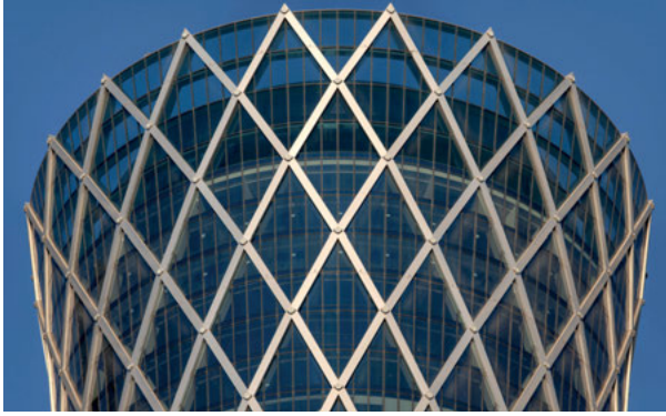
The Tornado Tower in Doha, Qatar, designed by CICO Consulting Architects and Engineers, uses an expressed system to highlight the diagonals, but not the horizontal bands of its diagrid structure, with LED lights installed at the nodal points for night lighting of the structure. A rectilinear glazing system has been used that runs continuously behind the diagonal bands.
