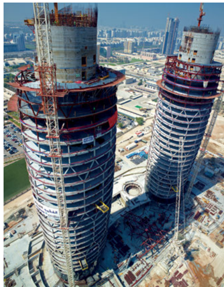
The attaching plates for the steel beams that will clear span from the concrete core to the perimeter framing must be carefully integrated into the casting of the concrete core as it proceeds. Here you can see that the round shape of the Al Bahar Tower is created through faceting rather than bending the steel. Steel fabrication and erection by William Hare Limited.
