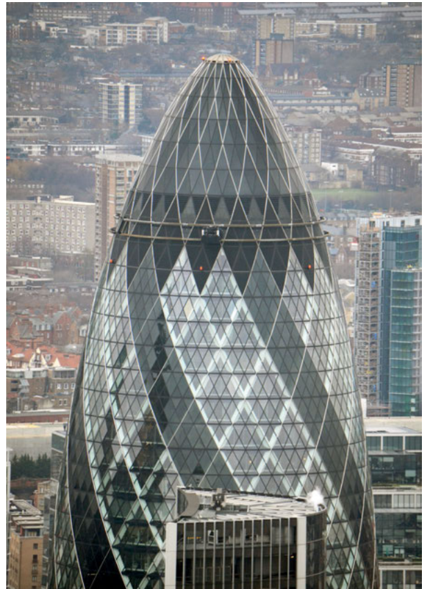
Swiss Re Tower (also called 30 St. Mary Axe) in London, England, designed by Foster + Partners and engineered by Arup, completed in 2004, was the most unique tower on the Central London skyline for several years. Its height was recently surpassed by The Shard (from where this photo was taken). The Leadenhall Building by Rogers Stirk Harbour + Partners (see Project Profile , page 148) is encroaching on Swiss Re’s spot on the London skyline.
