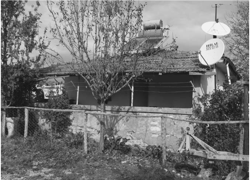
Figure 10.6 View of the lean-to roof.
