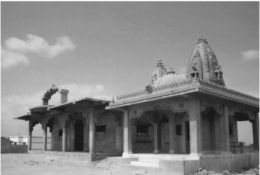
Figure 3.8 New temples in Chandrani. Due to widespread post-earthquake fear of the use of stones, replicas of traditional stone temples built with concrete can be seen in Chandrani village, Gujarat.
