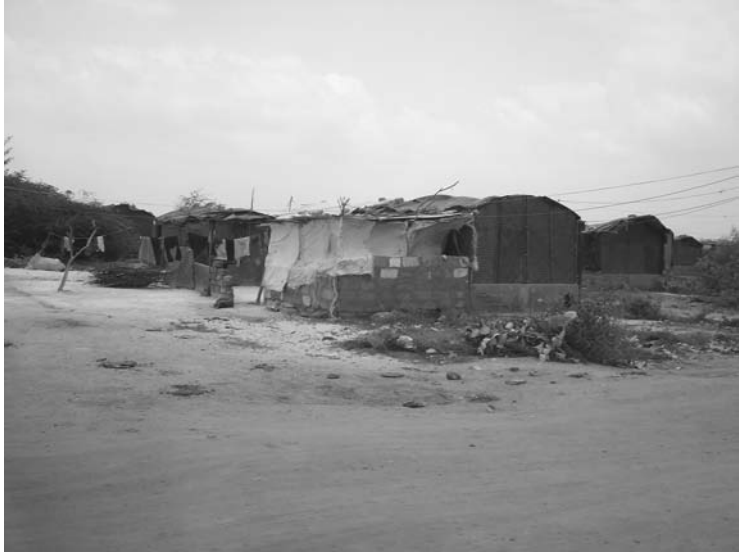
Figure 3.10 Temporary structures in Bhuj. Urban poor in Bhuj are still residing in temporary structures, even after seven years. The additions have subsequently been made using a variety of materials.
