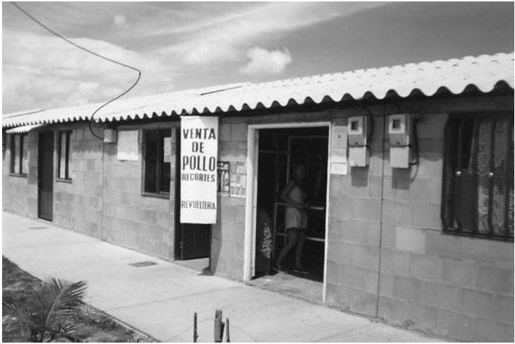
Figure 1.4 Post-disaster houses in Colombia. Domestic and income-generation activities often merge in low-cost housing in developing countries. Top: Having the option of deciding how to invest their own subsidies, beneficiaries of this rural reconstruction project in the coffee-growing area of Colombia decided to build infrastructure for coffee production (as in this picture), in this way boosting their economic recovery. Bottom: Thanks to proper public services, informal commerce quickly appeared in post-disaster urban residential projects in Colombia after the 1999 earthquake, demonstrating the crucial links between income generation and domestic activities (the sign reads “chicken for sale”).
