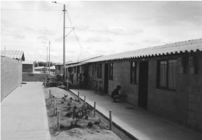
Figure 2.3 Formal and informal houses-in-progress. Top: Informal settlement in Bogotá showing four different stages in the housing evolution process: from a shack made of scrap wood to a three-storey unit made of concrete and masonry. Bottom: One-storey units in El Cantarito. Although higher densities were obtained by adopting the row-house approach and infrastructure could be provided, a few months after the project was finished, users had already modified the rigorously standardized façades to personalize them with colours and finishes.
