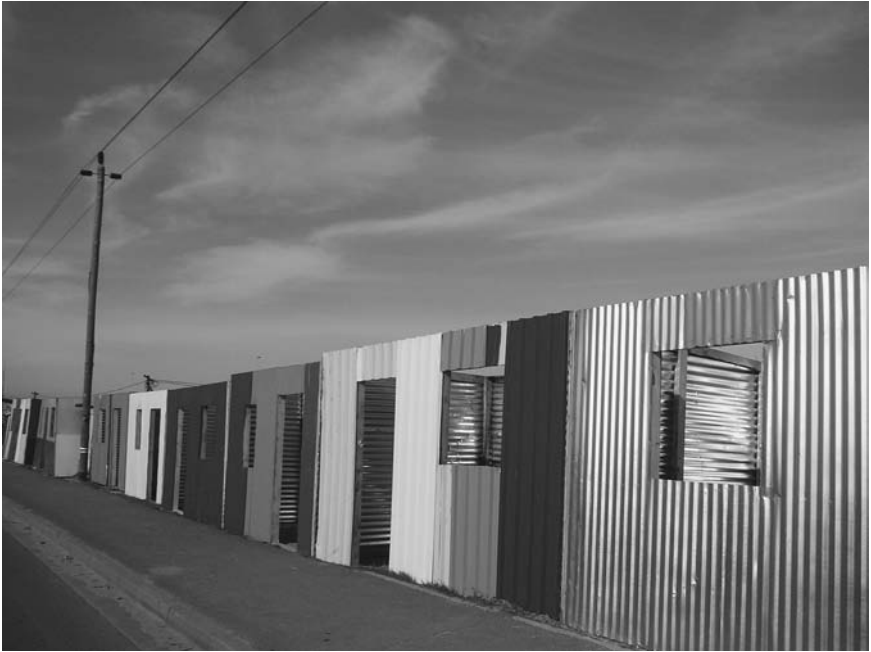
Figure 1.5 Prefabricated informal housing. Architects and urban planners interested in reconstruction have much to learn from the way in which the informal sector produces buildings for the poor. This informal sale of prefabricated shacks in the townships of South Africa delivers prefabricated housing solutions that can be customized and installed in 30 minutes. Using recycled materials and a simple technology, these solutions are well adapted to the needs of a sector of the population for which no architect has been able to produce a viable, large-scale solution.
