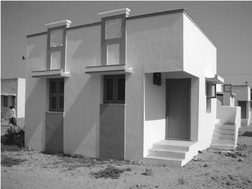
Figure 8.6 Post-tsunami houses in Tamil Nadu.
