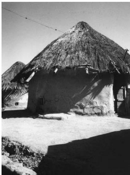
Figure 3.7 Traditional bhungas of Kutch. The traditional bhungas performed well against earthquake because of their circular form and wattle-and-daub construction.
