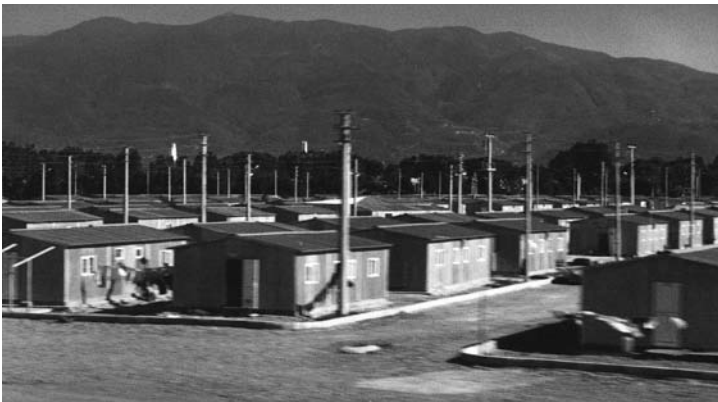
Figure 4.4 Temporary housing units. Top: Basic temporary housing units made of wood. Bottom: More elaborate prefabricated units. Düzce province, Turkey.
