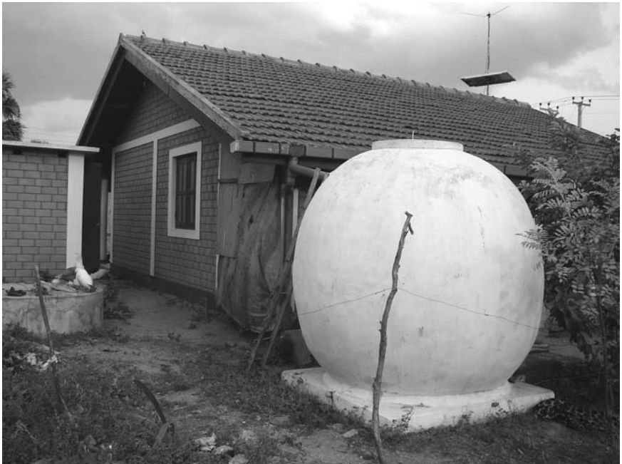
Figure 11.2 Designing layouts in relation to infrastructure needs – domestic water supply. Top: Kolavil resettlement scheme in Thirukkovil, Sri Lanka. Bottom: Thirukkovil resettlement scheme in Sri Lanka.
