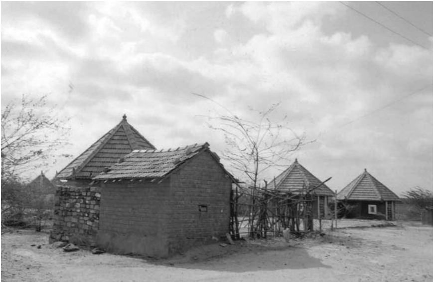
Figure 3.3 Bhungas reconstructed by an NGO after the earthquake. These bhungas are now being extended using stones and soil blocks, thereby increasing their vulnerability.
