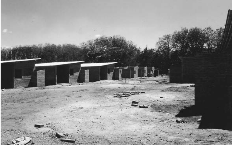
Figure 9.1 General view of La Hermandad under construction.
