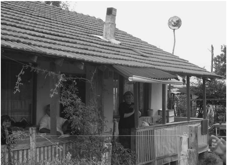
Figure 4.6 Core house. A shipping container was used as a temporary house and then additions were built around it to make a permanent house. Top: Side view of house showing shipping container. Bottom: Front view of house. Düzce, Turkey.
