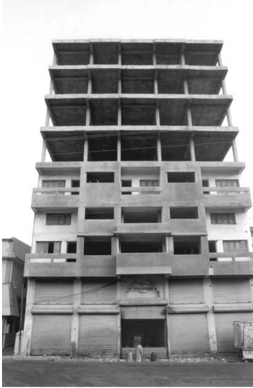
Figure 3.9 A multi-storeyed concrete-framed building in Bhuj. Due to widespread fear, a multi-storeyed concrete-framed building constructed just before the earthquake is lying abandoned in Bhuj, even though it did not sustain any damage from the earthquake.
