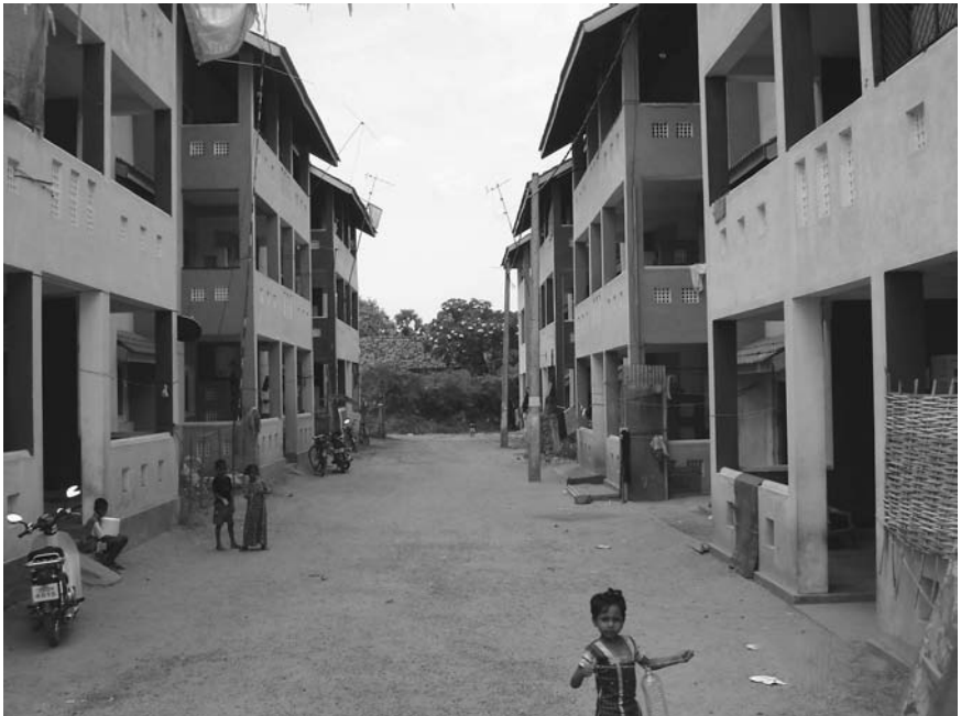
Figure 11.8 The design constraints imposed by poor site selection and land shortages. Top: Periyaneelavanai resettlement sites in Kalmunai, Sri Lanka. Bottom: Islamabath resettlement sites in Kalmunai, Sri Lanka.
