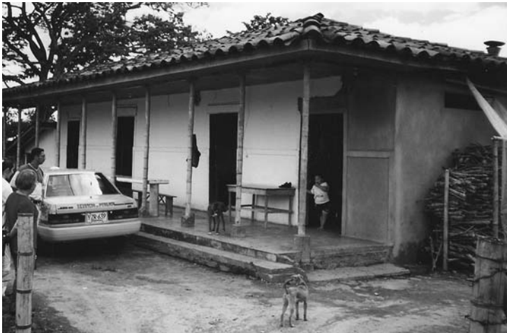
Figure 2.6 Reconstructed house in rural Colombia. The beneficiaries optimized the resources and subsidies to develop their customized projects (here a storage room was rebuilt in a partially affected house).
