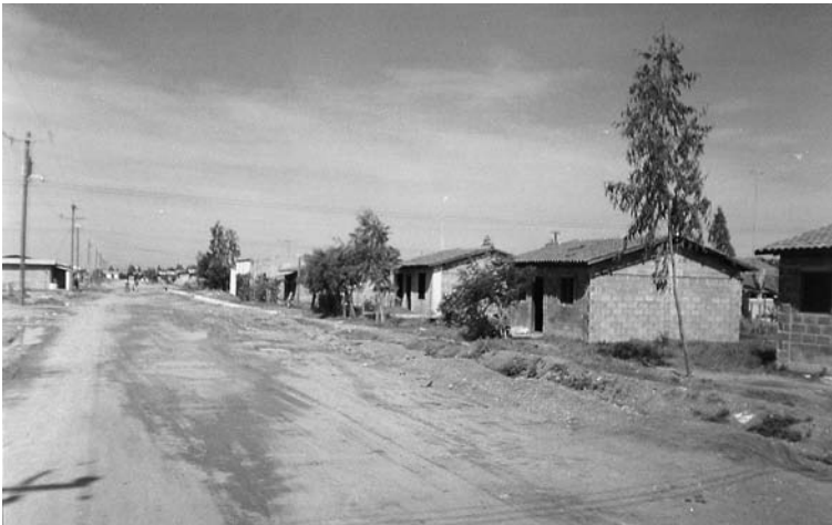
Figure 1.3 Post-disaster houses in Honduras. Houses that are ill-adapted to local needs and lifestyles represent a second disaster (sometimes as dangerous as the original one). Top: Beneficiaries dismantled the roof, doors and windows and abandoned this house built as part of a post-Mitch reconstruction initiative in Nueva Choluteca (Honduras). Bottom: Without proper infrastructure and with little sensitivity for lifestyles in hot weather, this housing settlement in Nueva Choluteca had a low economic recovery and led to increased criminality and major public-health problems.
