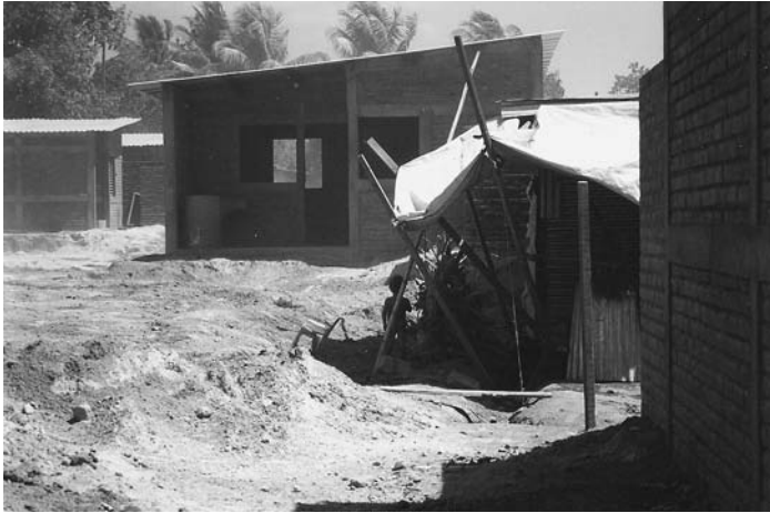
Figure 9.2 Houses under construction and temporary shelters.
