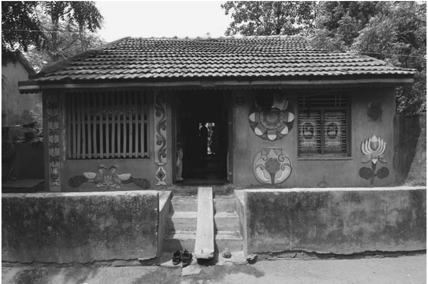
Figure 8.4 Traditional houses with tiled roofs.
