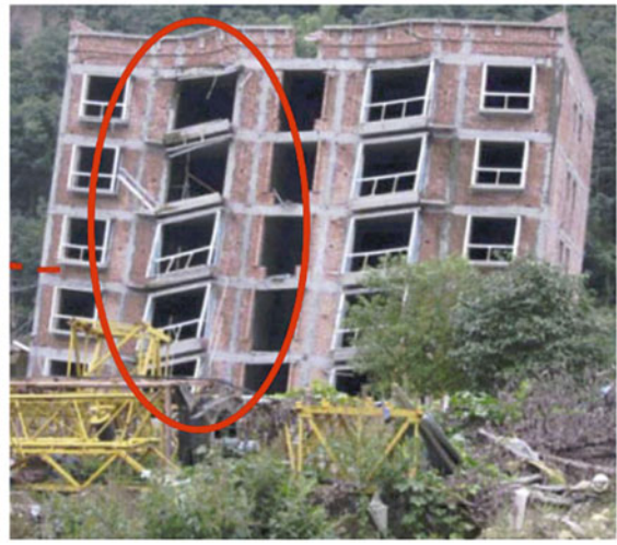
Fig. 2.13 Moment frames: unfavourable "storey mechanism" to be avoided (left) and favourable "beam mechanism" (right)
