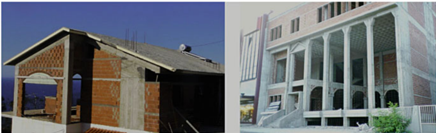
Fig. 2.29 Inclined diaphragm (left), partial diaphragm (right)
