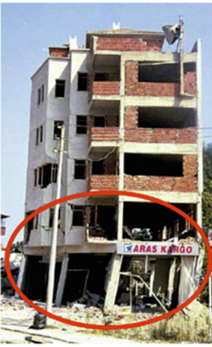
Fig. 2.13 Moment frames: unfavourable "storey mechanism" to be avoided (left) and favourable "beam mechanism" (right)
