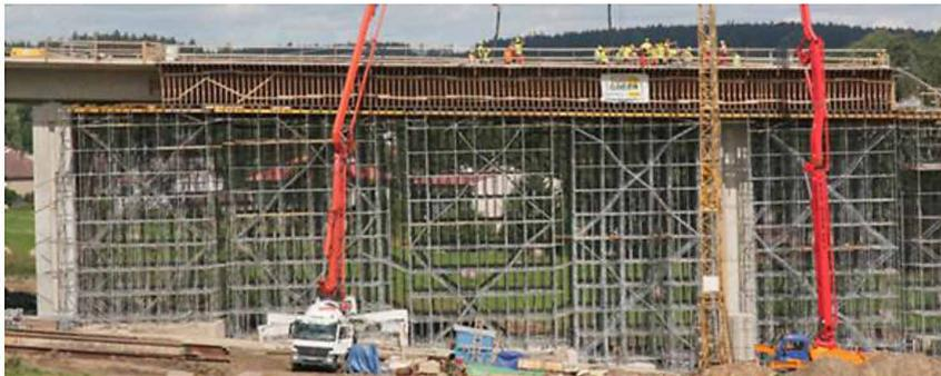
*Figure 7. Falsework heavy-duty tower system. ©2016 RMD Kwikform. Used with permission*
