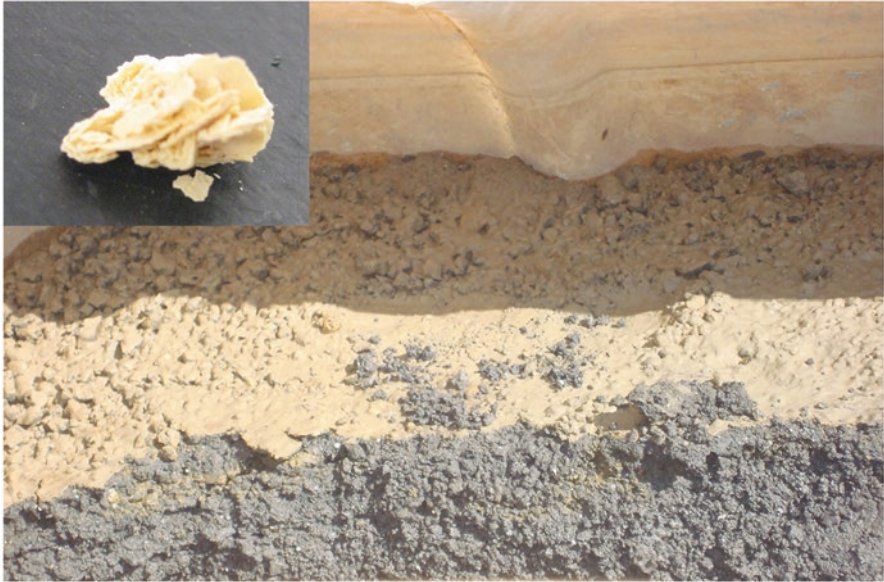
Fig. 4.15 Cutaway of a clogged PSM bed that consisted of un-sieved electric arc furnace steel slag. The brown-orange precipitant at the surface and in the pore space are precipitated Ca carbonate, sulfate, and silicate minerals that formed and ultimately restricted all flow after about 100 h of flow through the PSM bed. The inset photograph shows a solid piece of the precipitant that formed in the drainage pipe of the P removal structure. For this reason, steel slag should always be screened to remove the fine particles prior to use in a P removal structure
