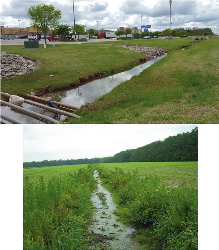
Fig. 3.3 Drainage ditches in agricultural or urban environments can serve as an ideal intercession point for the construction of a P removal structure if the dissolved P concentrations are high. Photo credits— upper : Joshua Bradley, Oklahoma State University; lower : Gene Hahn, University of Kentucky
