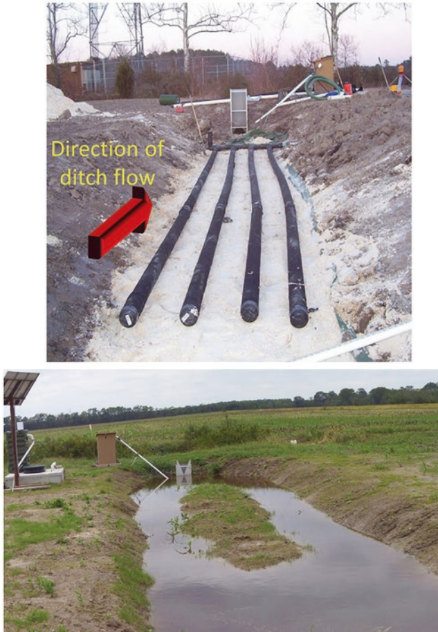
Fig. 3.9 A “ditch-filter” style of P removal structure. The upper and lower photos show the ditch-filter during and after construction, respectively. A flow control structure is used to maintain hydraulic head on the PSMs in the ditch, and water is forced to drain through the bed of PSMs into a series of buried perforated pipe that transfers the treated water to another drainage ditch in the rear. For this type of structure, it is very important to consider the loss of ditch flow capacity by placing PSMs into the ditch. Photo credit: Josh McGrath, University of Kentucky
