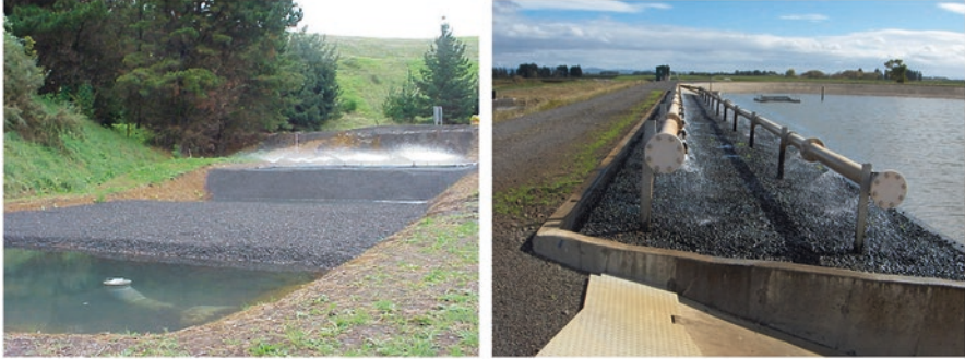
Fig. 3.21 Phosphorus removal structures used to treat municipal wastewater at wastewater treatment plants located in New Zealand. Both P removal structures utilize steel slag. Photo credit: Harsco Metals and Minerals
