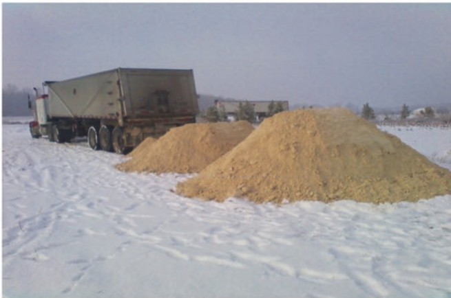
Fig. 4.4 Upper: schematic of the steam generating process for coal-fired power plants and the resulting waste products of bottom ash, fly ash, and flue gas desulfurization (FGD) gypsum. Lower: photograph of several tons of FGD gypsum to be placed into a ditch-style P removal structure on the Eastern Shore of Maryland. Photograph courtesy of Gene Hahn
