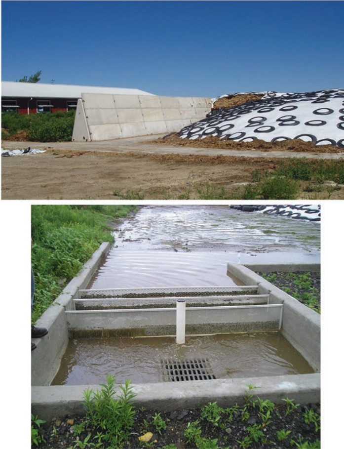
Fig. 3.23 Silage storage bunkers ( upper photo ) are capable of releasing a large load of dissolved P into the environment. In some silage storage bunkers, runoff is channeled through a series of screens to remove solid particle to prevent particulate P transport ( lower photo ), and then the water is typically discharged to a vegetated treatment area to promote infiltration of the water. A P removal structure could be configured to this system to remove dissolved P after the particulate P has been removed. Photos courtesy of Erie County, NY NRCS
