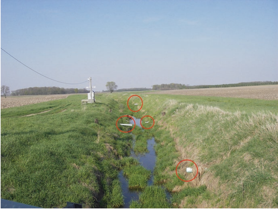
Fig. 3.7 Typical tile drain outlets into ditches for farms in the upper mid-western U.S. A single ditch on one farm can have many subsurface drainage outlets. In choosing a location for a P removal structure, one should choose to treat the subsurface drains that have the highest dissolved P concentrations. If all of the subsurface drainage is elevated in dissolved P, then the entire ditch can serve as a location for a ditch-filter. Photo credit: Stan Livingston, USDA-ARS.
