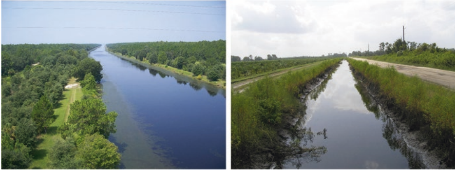
Fig. 3.6 Example drainage canal ( left ) and on-farm drainage ditch ( right ) found in Florida. Low-flow drainage water with high P concentrations are more efficient locations for removing dissolved P with a P removal structure compared to high-flow drainage where dissolved P has already been mostly diluted. Left photograph: Wikimedia Commons, “Cross Fla Barge Canal SR19W-01.jpg. Right photograph is courtesy of Bill Frank, www.jaxshells.org
