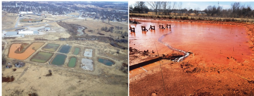
Fig. 4.3 Left: aerial view of an acid mine drainage treatment facility for treating drainage from Tar Creek, located near Miami, Oklahoma. Right: close up photograph of a passive acid mine drainage treatment pond. Photographs courtesy of Dr. Bob Nairn, University of Oklahoma
