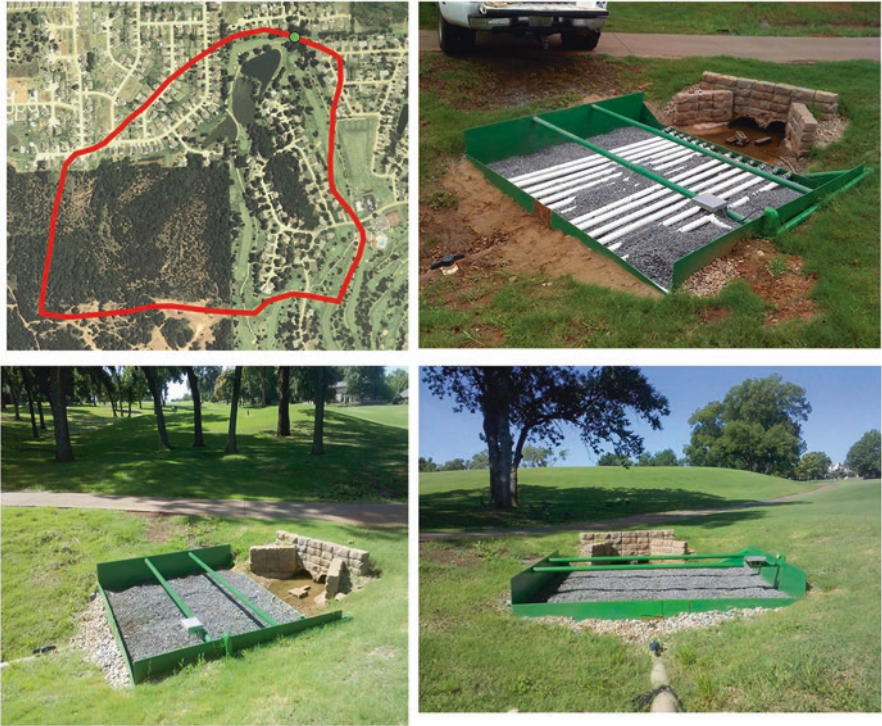
Fig. 3.10 A “confined bed” style P removal structure located on a golf course. Upper left photo shows the 150 acre watershed that drains into the confined bed of PSMs (green dot). Upper right photo shows the manifold of perforated pipe that evenly distributes water over the bed of PSMs before draining into the outlet pipe. Lower photos show the completed structure. Photo credit: Chad Penn, USDA-ARS
