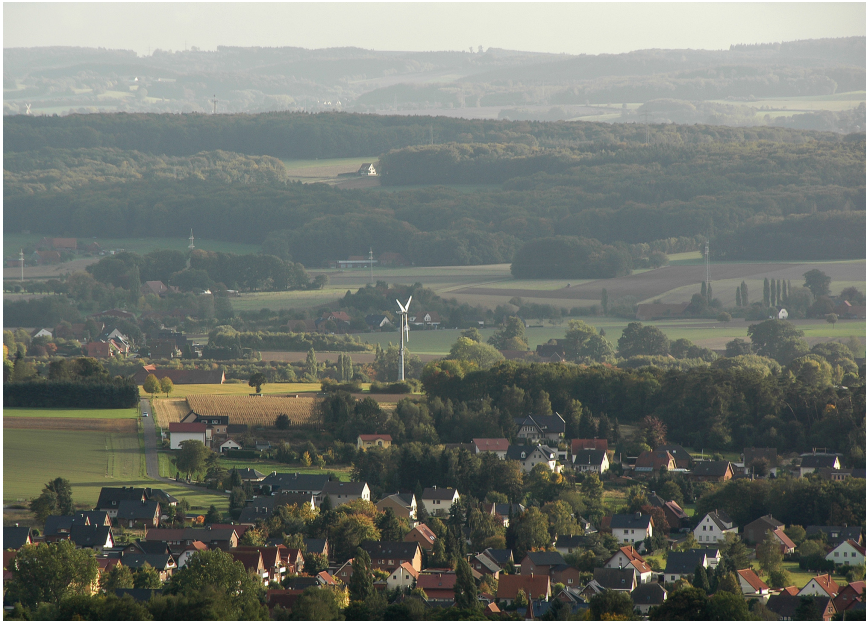
Fig. 11.2 Example of a community based wind turbine in a German village
