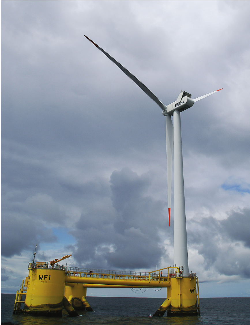
Fig. 8.2 The introduction of floating turbines poses even more challenges than current offshore turbines
