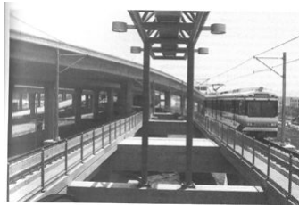
Figure 3.19: Light Rail Transit
