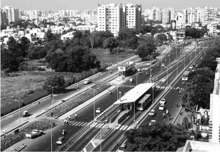
Figure 7.10 Median bus lane in Ahmedabad (Janmarg)
