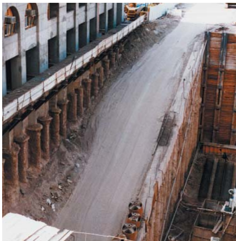
Fig 12.1 Example of an access ramp
