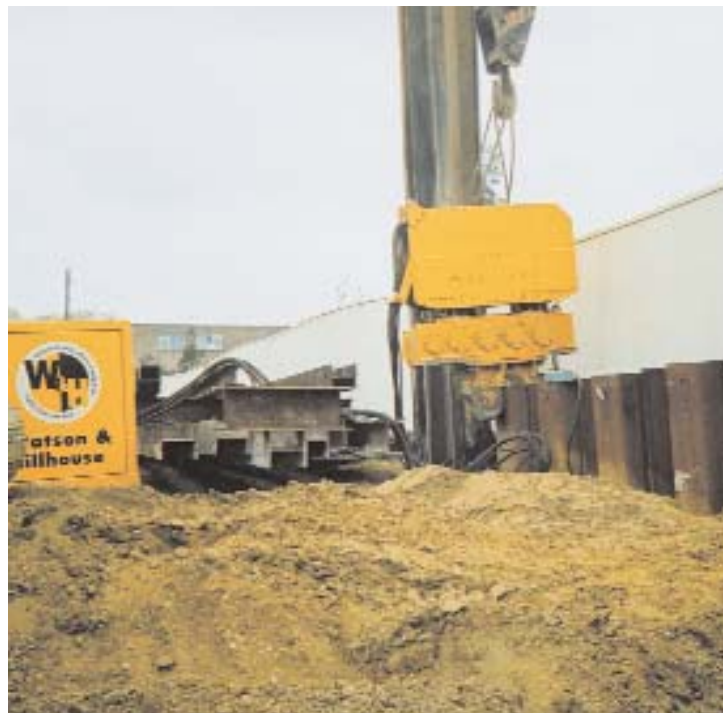
Fig 4.12 Sheet pile installation by high frequency vibrator
