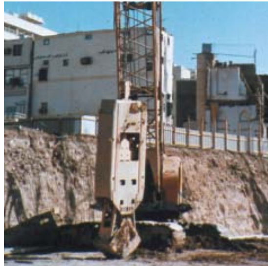
Fig 4.17 Grab excavation equipment for diaphragm walls
