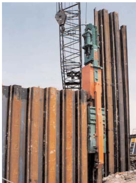
Fig 4.13 Sheet pile installation by hydraulic hammer © BSP International Foundations Limited
