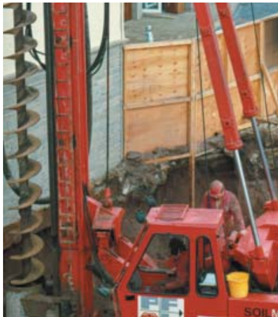
Fig 4.15 Continuous flight auger (cfa) rig
