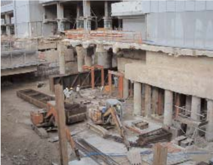
Fig 10.5 Changi Airport Station: underpinning transfer beams being inserted © Benaim
