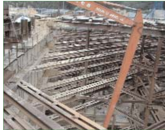
Fig 9.1 Changi Airport: excavation by long-reach/dipper excavator © Benaim
