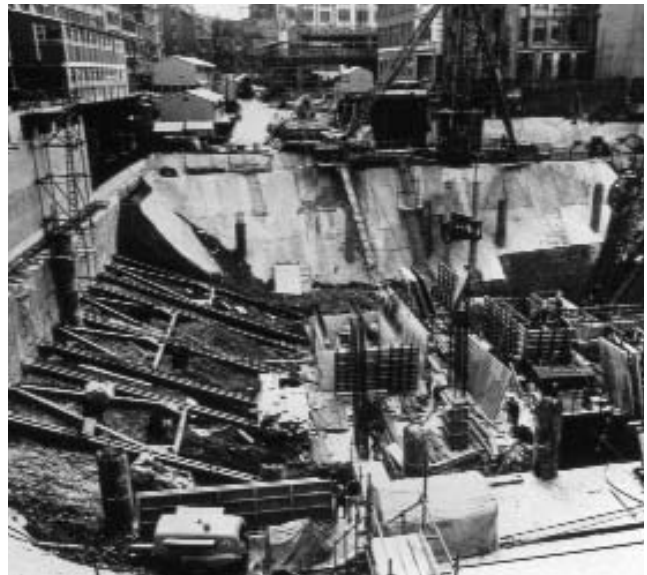
Fig 4.10 Britannic House, London: Showing top struts positioned and preloaded
