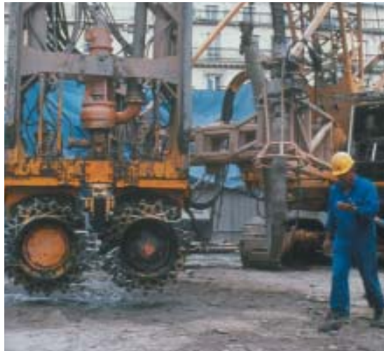
Fig 4.20 Cutters of mini-rig for restricted urban sites © Bauer Spezialtiefbau
