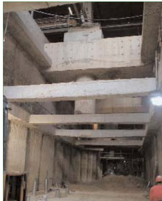
Fig 10.2 Changi Airport Station: pile underpinned by transfer beams and amputated
