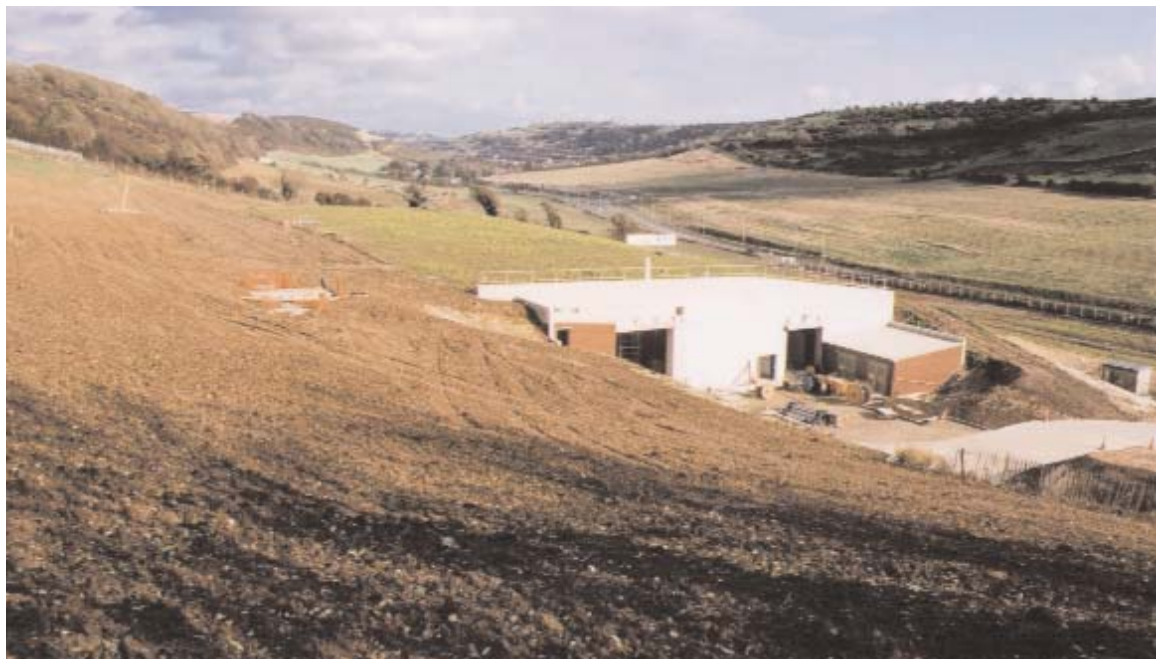
Fig 1.7 Broomfield Bank WWTW, Dover: buried in hillside © AMEC
