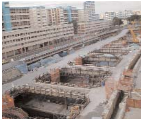
Fig 4.5a Semi top-down construction, Singapore M.R.T, C705 Boon Keng Station © Benaim
