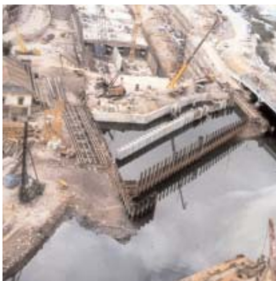
Fig 11.2 Central Expressway II: phased passage under River Singapore in cofferdam © Benaim
