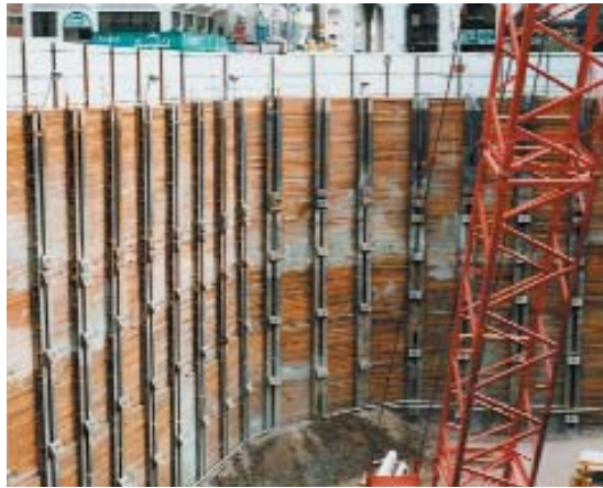
Fig 4.14 King post wall construction, Medinah, Saudi Arabia
