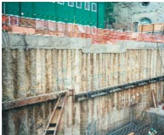
Fig 4.16 Hard-soft secant wall construction, Carlton Gardens, London
