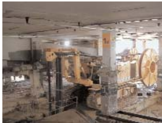
Fig 4.18 A cutter rig working in low headroom © Benaim
