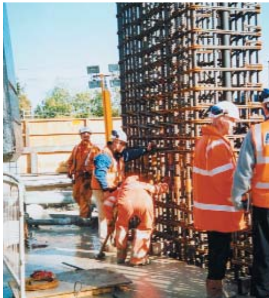
Fig 4.21 Diaphragm wall cage during insertion into a slurry filled trench
