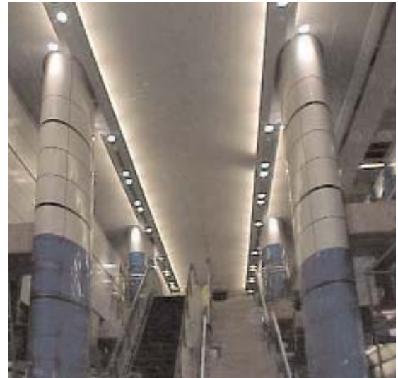
Fig 1.9 Boon Keng Station, Singapore: double storey height free of struts © Benaim
