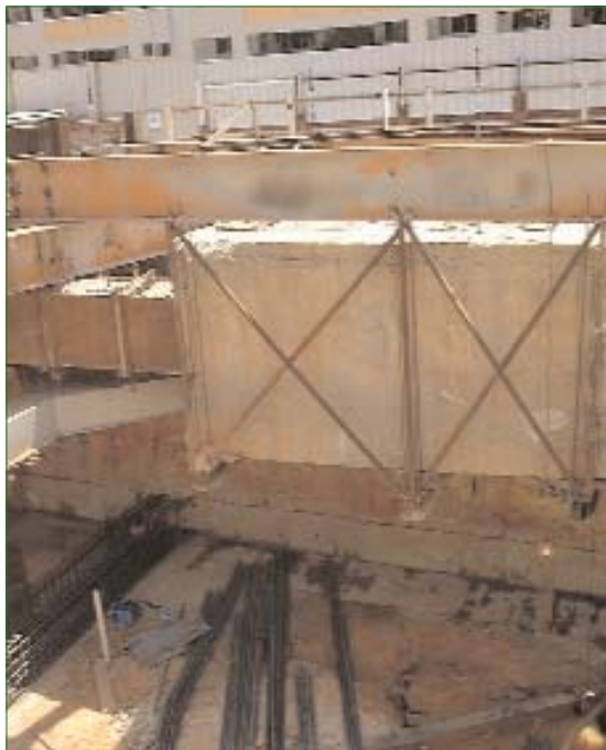
Fig 10.1 Potong Pasir Crossover, Singapore: support of existing manhole
