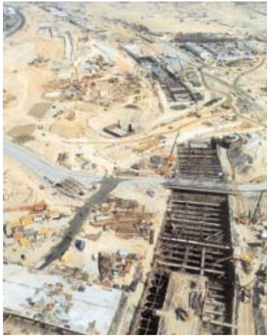
Fig 1.6 Airport Express Tunnel, Hong Kong © Aoki Corporation
