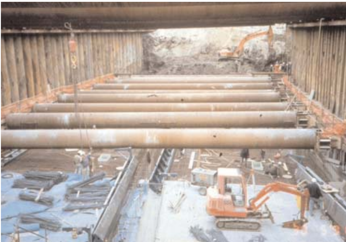
Fig 4.22 Construction proceeding below heavy temporary steel tubular struts
