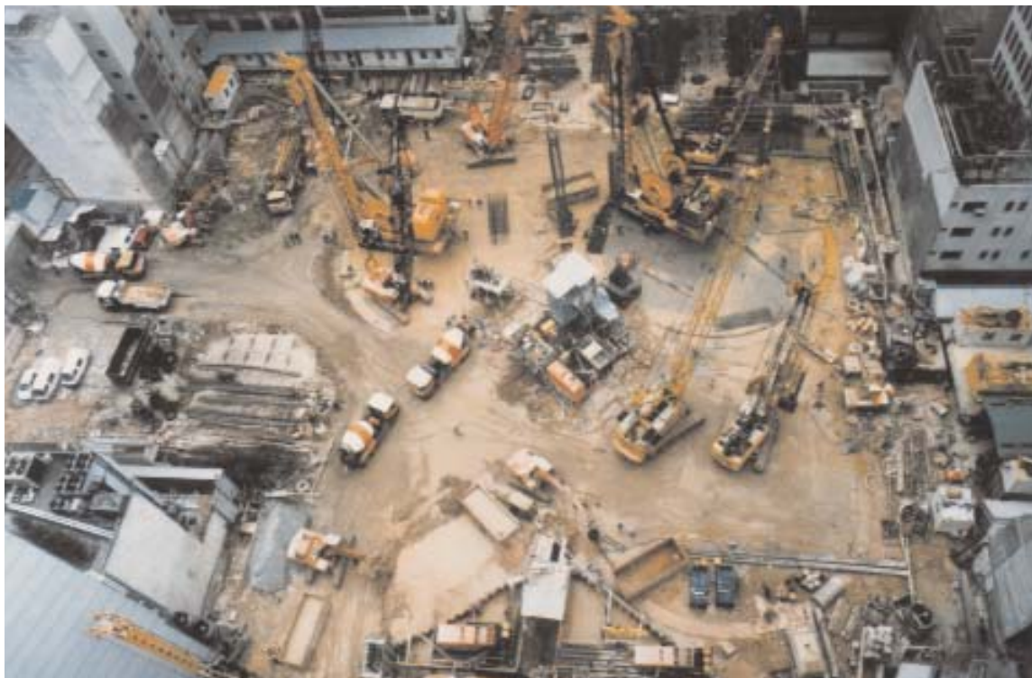
Fig 12.2 Example of a congested site © Paul Y. Foundation Limited
