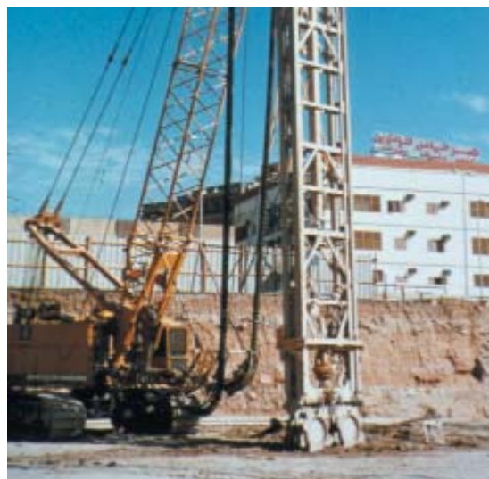
Fig 4.19 Reverse circulation cutter for diaphragm walls
