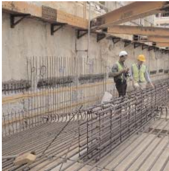
Fig 11.4 Boon Keng Station, Singapore: couplers in diaphragm walls for crack control © Benaim
