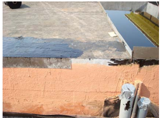
Figure 2.1-J Slab Foundation Example 1 Photograph copyright Liberty Building Forensics Group®.
