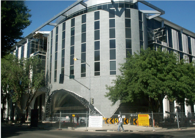
Figure 5.1-B Capitol Area East End Complex Photograph courtesy of Leon Alevantis.
