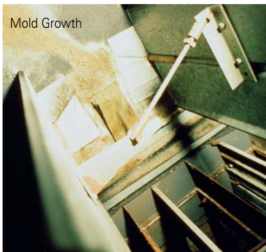
Figure 4.1-C Porous Airstream Surface Heavily Colonized by Visible Mold Growth Photograph courtesy of Phil Morey.
