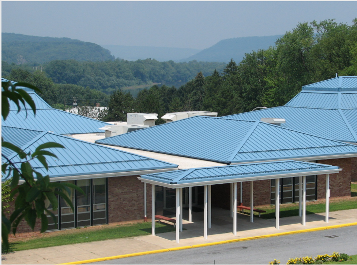
Figure 8.1-C Junior High School in Pennsylvania (Roof-Mounted DX DOAS Visible)
