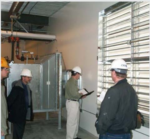
Figure 7.2-B Minimum Outdoor Air Fan and Main Outdoor Air Dampers
