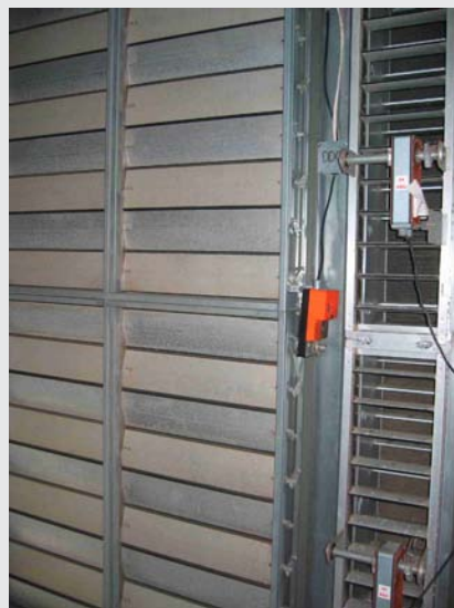
Figure 7.2-G Downstream View of Intake as in Figure 7.2-F
