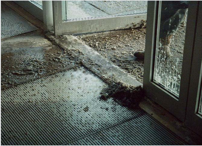
Figure 2.5-A Inadequate Track-Off Design for Local Conditions Photograph courtesy of Hal Levin.
