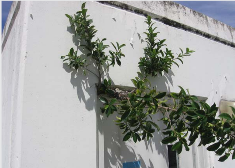
Figure 2.6-A Tree Sapling Growing from Upper Portion of Window Photograph courtesy of Phil Morey.
