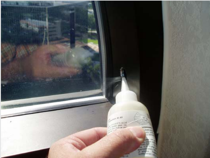
Figure 2.3-A “Smoke” Test Demonstrating the Building was Negatively Pressurized in Reference to the Exterior
