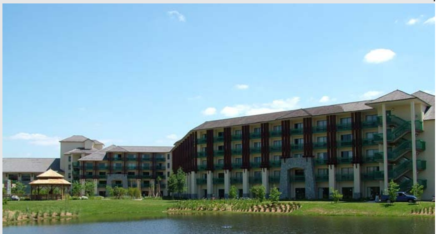
Figure 1.2-G Completed Project Photograph courtesy of Dave MacPhaul; copyright CH2M HILL.
