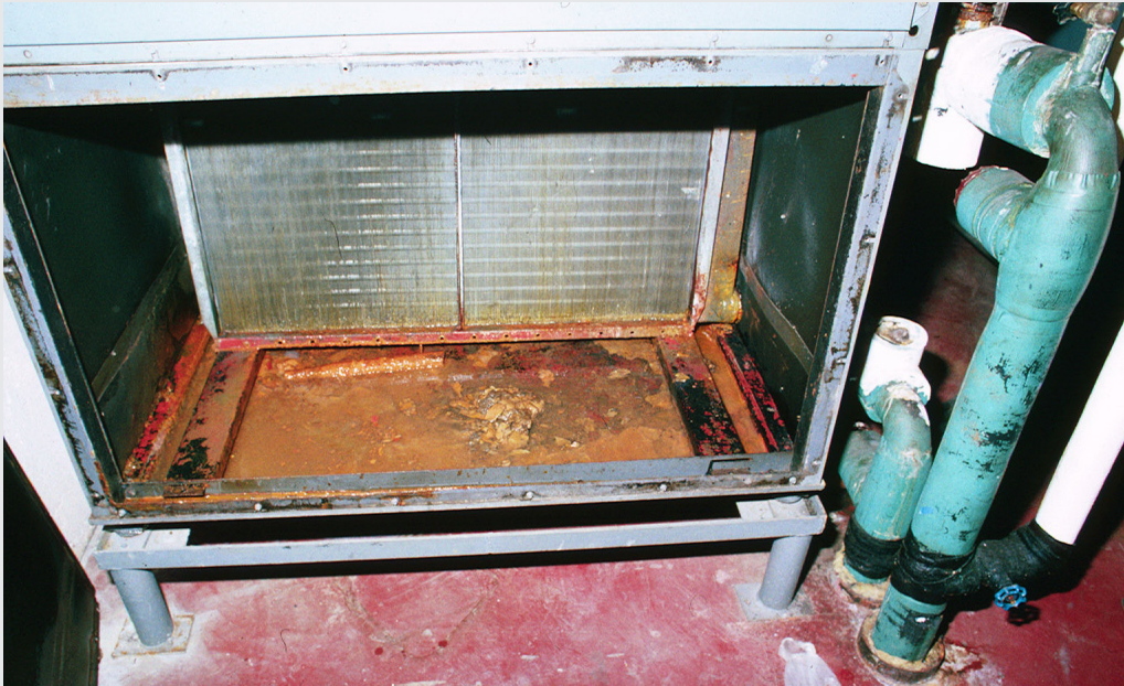
Figure 4.1-A Drain Pan that was Poorly Designed and Maintained Photograph courtesy of Phil Morey.
