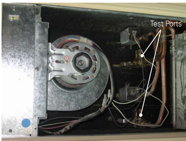
Figure 4.3-G Inaccessible Test Ports due to Balancing Valve Installation Photograph courtesy of Jim Hall.
