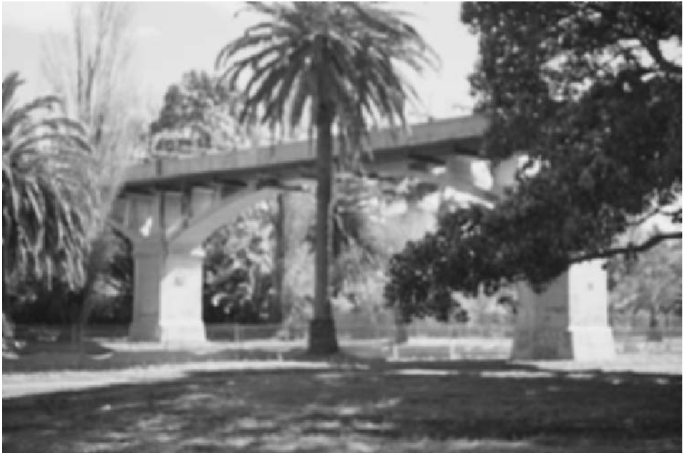
Fig. 8.3 Johnstone's Creek aqueduct after repair (photo: Susan Macdonald).
