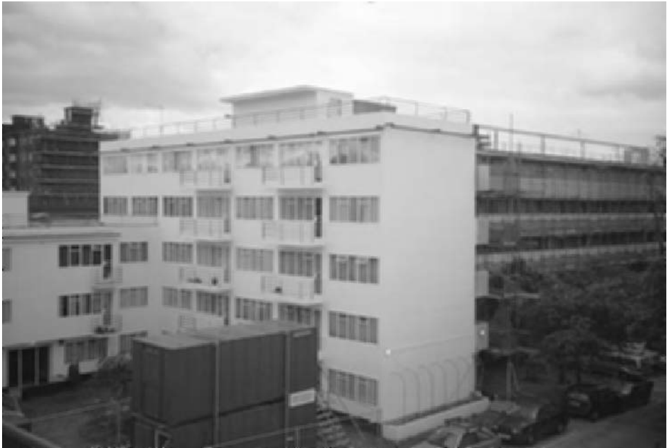
Fig. 5.4 Pullman Court, Streatham Hill, London, designed by Sir Frederick Gibberd, 1936. The concrete was repaired by patching, followed by the application of an anti-carbonation coating to reduce the progress of carbonation (photo Susan Macdonald).
