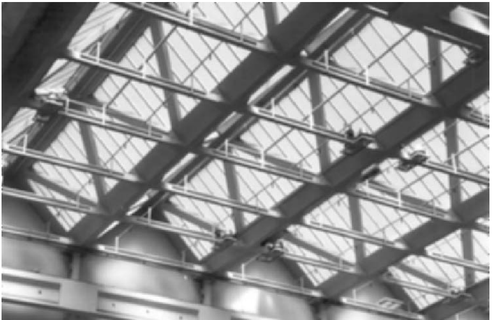
Fig. 2.33 Roof detail on BOAC maintenance headquarters hangar, Heathrow Airport, west London, 1950–1955. Engineer and architect Owen Williams (photo Bill Addis).
