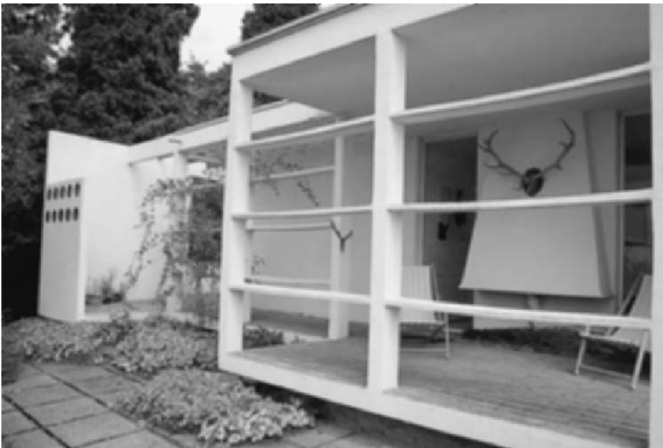
Fig. 1.3 The Loggia, Bungalow 'A', Whipsnade, Buckinghamshire, 1933–1936, designed by Berthold Lubetkin. The thin-walled construction of the architect's own house has suffered problems typical of its era and construction type. The slender precast-concrete members of the loggia and fenestration have sagged. Despite the thin-walled construction, with its minimal cover to the reinforcing steel, the concrete is of a high quality and has therefore survived relatively well. The building was to be repaired using a fairly minimal approach.
