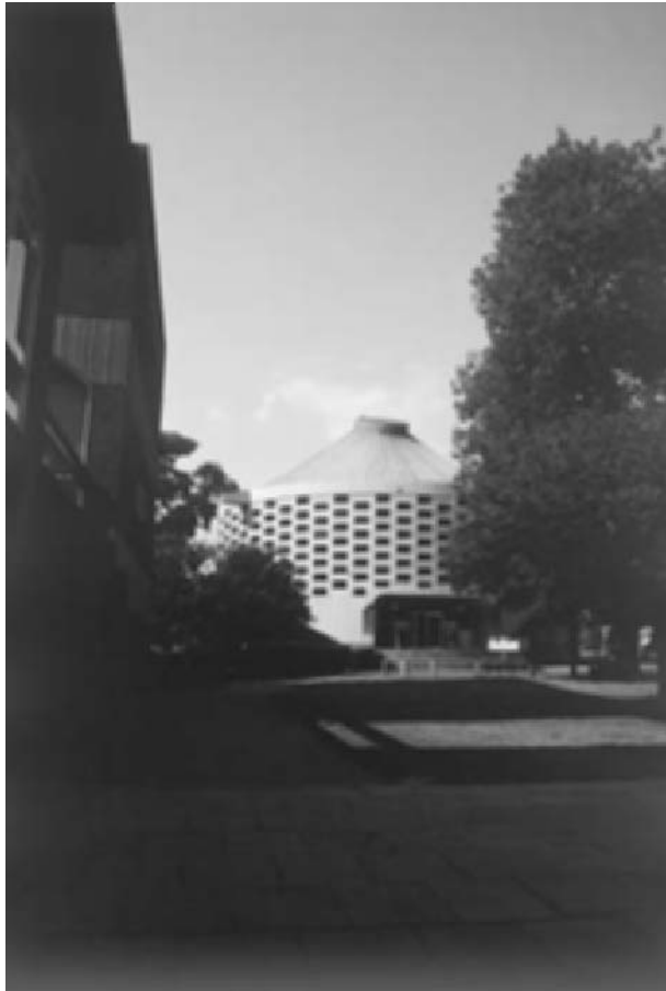
Fig. 8.15 The Meeting House at the University of Sussex following its repair 2 years earlier in 1992. The building was coated with an anti-carbonation coating. Although this attempts to replicate the colour of the concrete, the finish gives a plastic shiny appearance and some of the texture of the board-marking has been lost.
