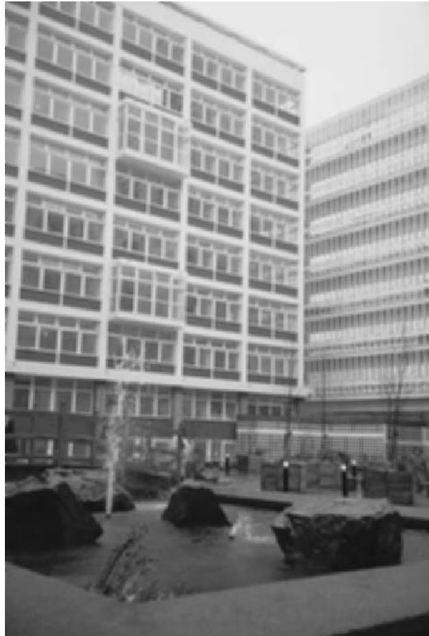
Fig. 6.5 The former Department of National Health building Alexander Fleming House, London (designed by Ernő Goldfinger 1959–1966), after repair and re-use as an apartment block. The repairs included the application of an elastomeric coating over the previously unpainted concrete. The decision to paint the building was the result of a combination of factors: the large number of patch repairs required, the extent of the micro-cracking and an argument that painting would improve the building's appearance (photo Susan Macdonald).
