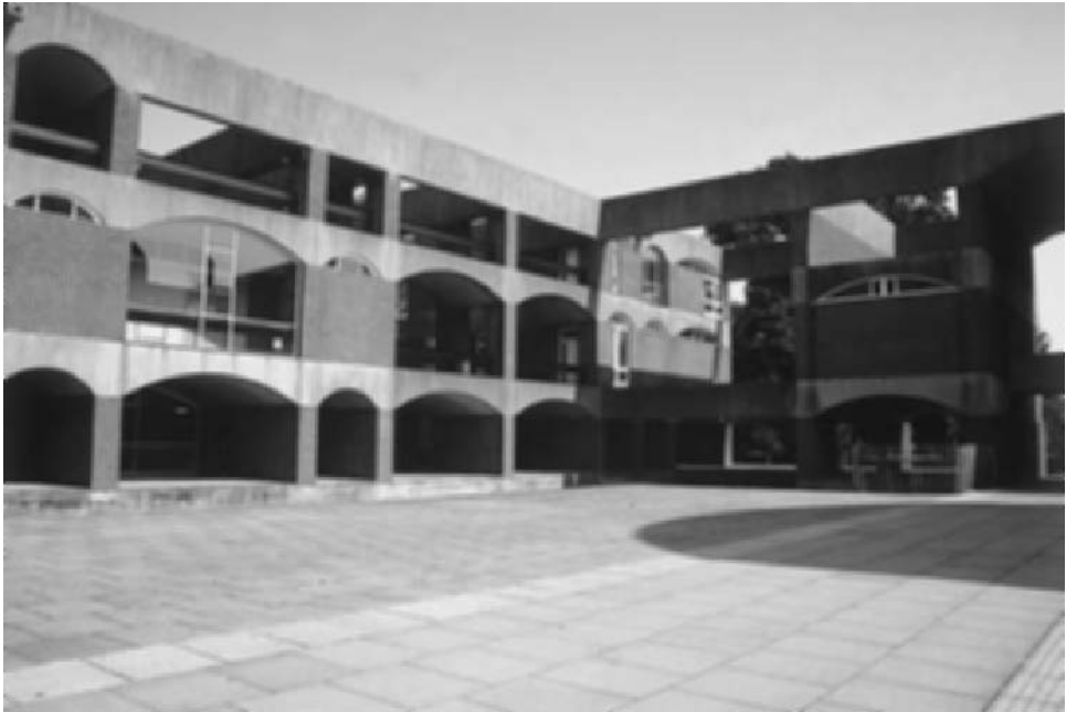
Fig. 3.1 Falmer House, University of Sussex, designed by Sir Basil Spence 1960–1961, is a listed Grade 1 building. Testing can be an invasive process, and when dealing with a listed building special care must be taken to design the testing so that it minimises the effect on the building. In some cases, statutory consent may be required (photo Susan Macdonald).
