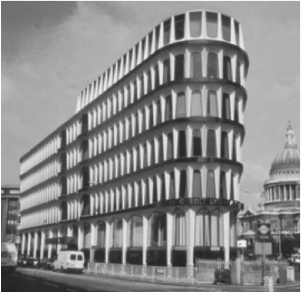
Fig. 2.46 Glass-reinforced cement cladding on the Crédit Lyonnais building in Queen Victoria Street, City of London (courtesy Ove Arup & Partners; photo Mike Taylor).
