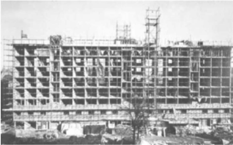
Fig. 2.24 Spa Green Estate, Finsbury, London, 1949, seen under construction (photograph Sydney Newbery, courtesy Ove Arup Partnership).
