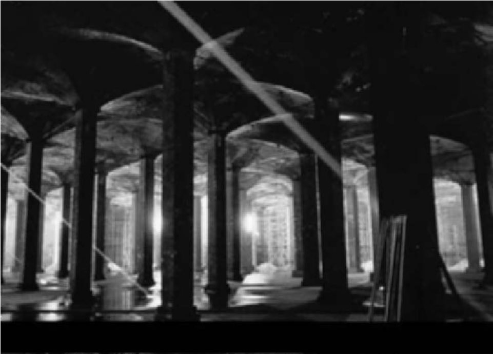
Fig. 8.4 Centennial Park reservoir, showing mass concrete groined arches and brick columns (photo Sydney Water).
