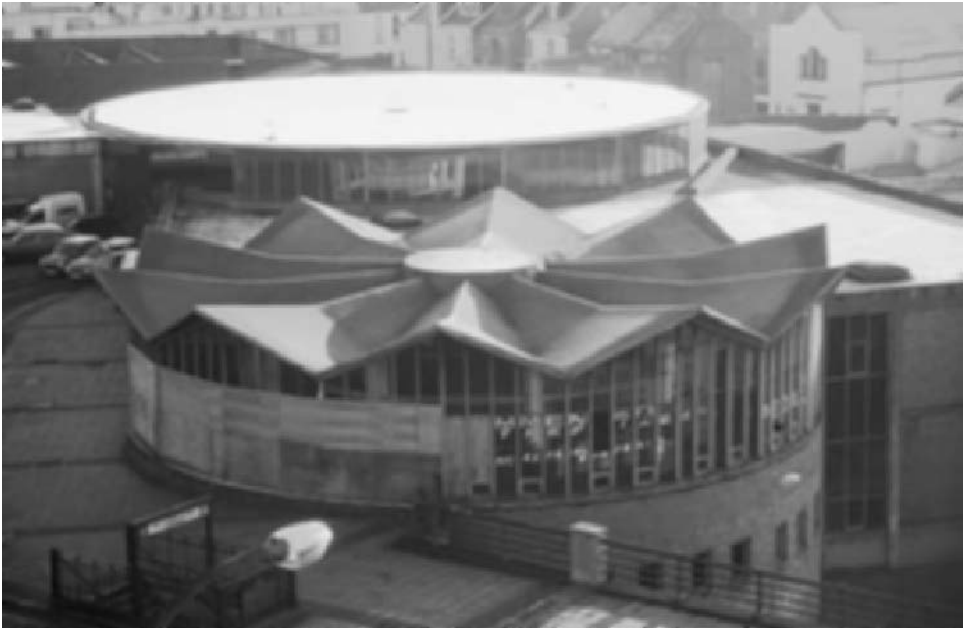
Fig. 2.31 Folded plate roof over car showroom, Turnbull's Garage, Plymouth, 1960. The folded plate roof is supported on ten columns beneath the valley points. The adjacent flat circular roof covered the filling station area of the garage, which was the first self-service filling station in Britain (photo Bill Addis).
