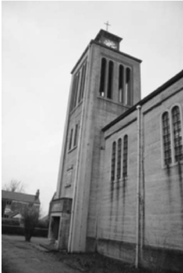
Fig. 1.1 St John and St Mary Magdalene, Goldthorpe, South Yorkshire, 1914–1916, designed by A. Nutt. The problems associated with the reinforced concrete decay in this church are a result of the particular way it was constructed, and are different from problems that have occurred in the building shown in Fig. 1.3.
