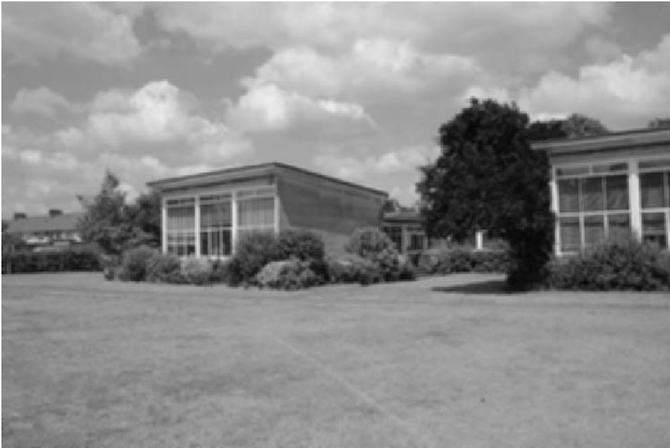
Fig. 8.12 Burleigh School, Hertfordshire, 1947, one of the schools designed by the Hertfordshire County Council Architect's Department, with a design based around child-like proportions. A modular prefabricated construction method was developed to provide this series of small-scale buildings (photo Susan Macdonald).
