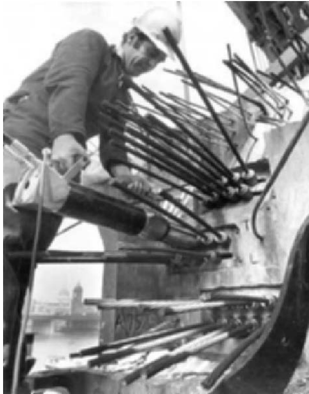
Fig. 2.40 Post-tensioning and fixing cables in a long-span beam (British Cement Association).
