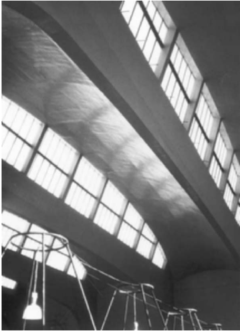
Fig. 2.30 Pannier Market, Plymouth, interior view (photo Bill Addis).
