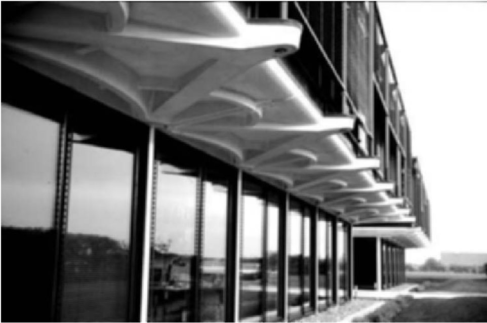
Fig. 2.53 Exterior of the Schlumberger Research Headquarters, Cambridge (Architects Michael Hopkins & Partners; Engineers Buro Happold; photo Bill Addis).
