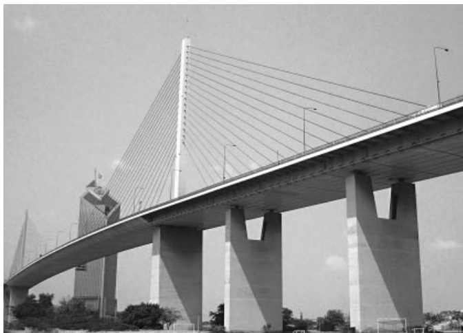
Figure 1.71 The Rama IX Bridge in Bangkok (Thailand)
