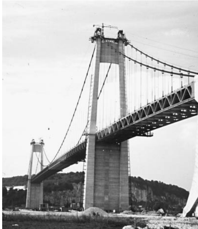
Figure 1.30 Tancarville Bridge across the Seine (France)
