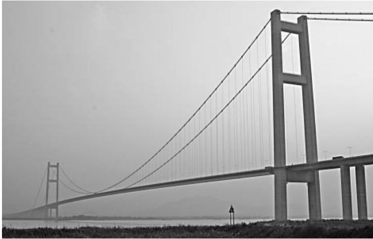
Figure 1.108 Runyang Suspension Bridge (China)
