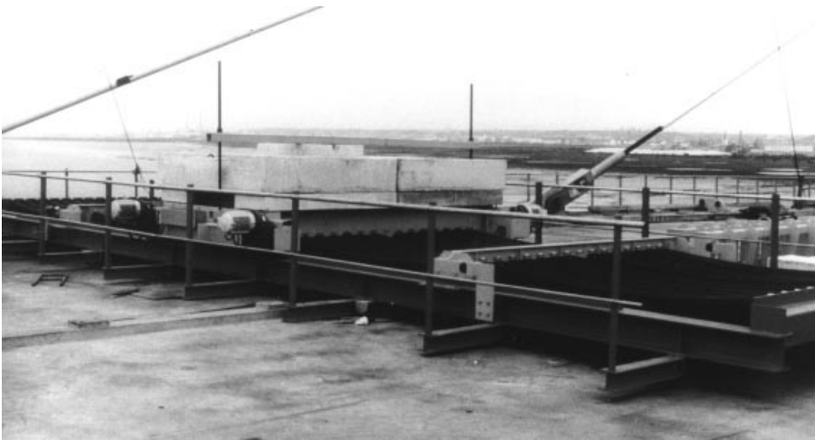
Figure 7.75 Tuned mass dampers on the deck of the Normandy Bridge
