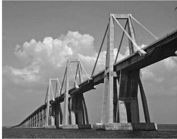
Figure 1.33 Maracaibo Bridge (Venezuela)
