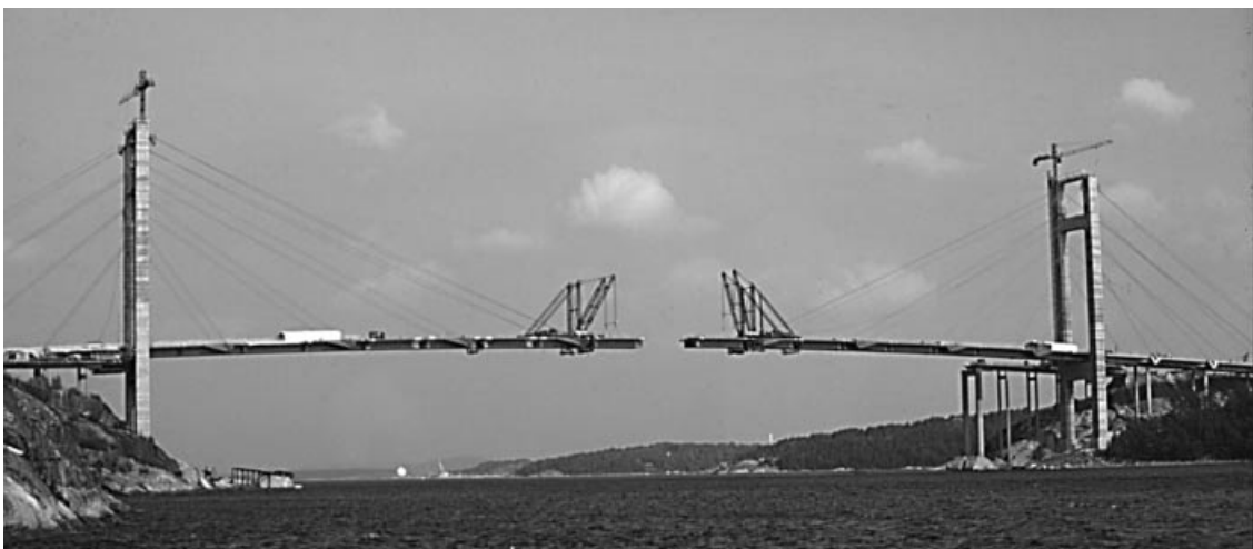
Figure 1.62 The second Tjörn Bridge under construction in 1981 (Sweden)
