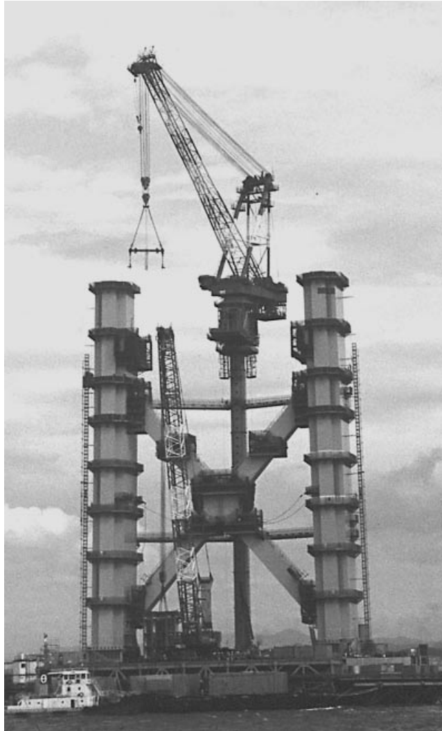
Figure 7.5 The Akashi Kaikyo Bridge pylon during erection
