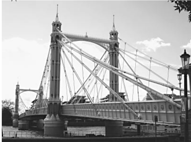
Figure 1.3 Albert Bridge across the Thames (UK)
