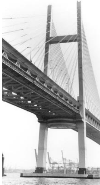
Figure 5.54 Pylon of the Yokohama Bay Bridge
