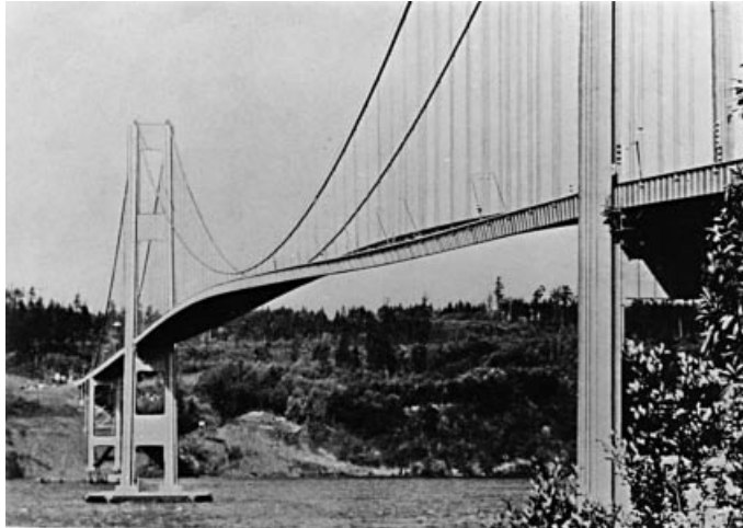
Figure 1.17 The fatal twisting oscillation of the First Tacoma Bridge
