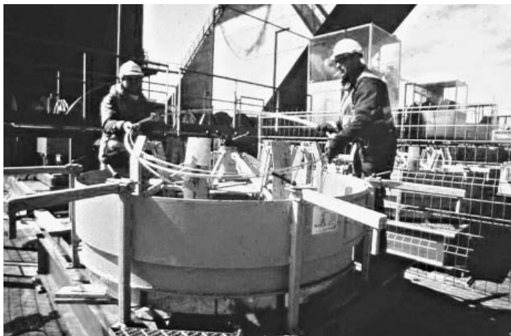
Figure 7.20 Loading swift at the Storebælt Bridge site
