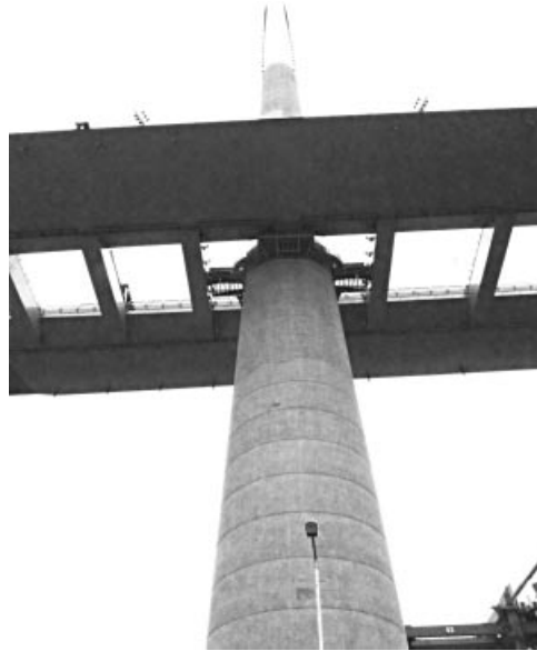
Figure 5.25 Pylon of the Stonecutters Bridge
