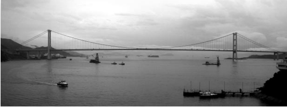
Figure 3.41 Tsing Ma Bridge
