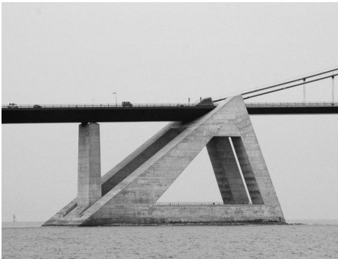
Figure 6.85 The Storebælt East Bridge anchor block
