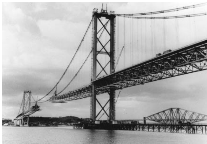
Figure 7.49 Firth of Forth Road Bridge during erection. Note the derrick cranes at the tips of the stiffening truss
