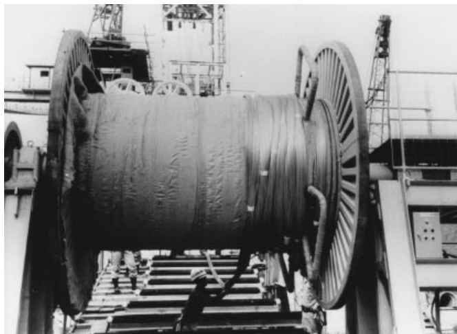
Figure 7.29 Unreeling machine for the PPWS of the Akashi Kaikyo Bridge
