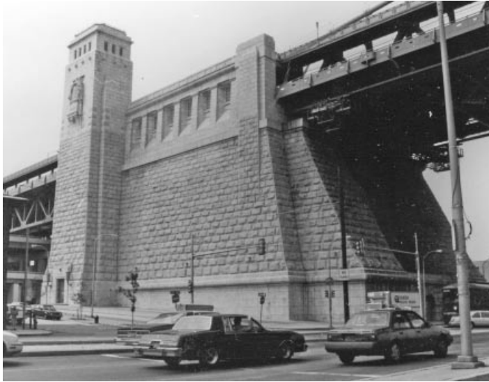
Figure 6.81 Anchor block of the Benjamin Franklin Bridge
