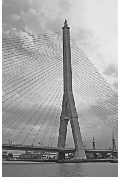
Figure 5.73 Pylon of the Rama VIII Bridge in Bangkok
