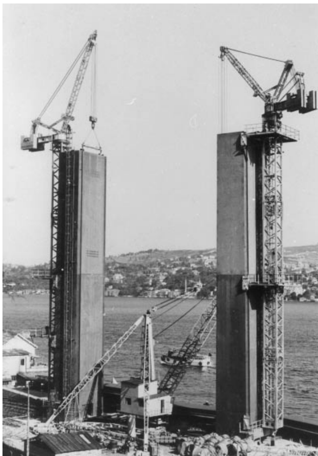
Figure 7.4 Erection of the Bosphorus Bridge pylon by twin tower cranes
