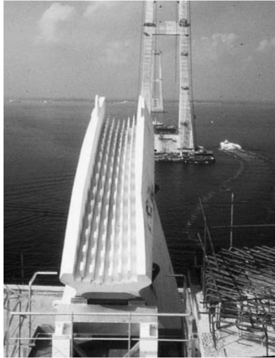
Figure 6.76 Splay saddle at the anchor block of the Storebælt East Bridge
