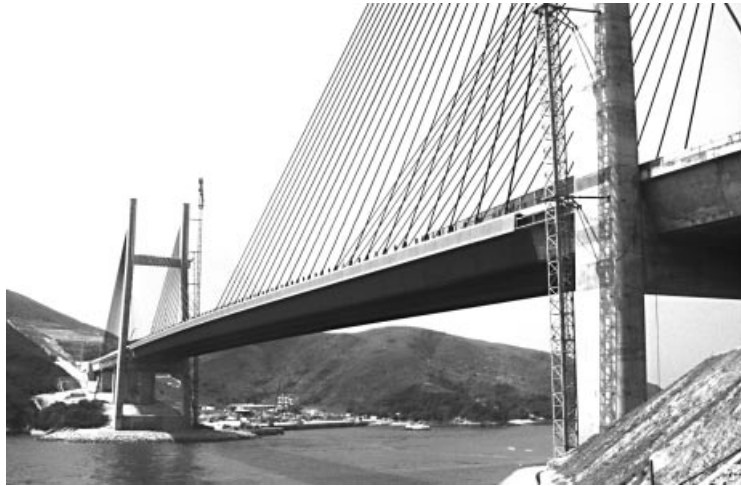
Figure 1.94 Kap Shui Mun Bridge (Hong Kong SAR)
