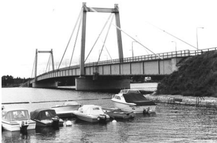
Figure 1.26 Strömsund Bridge (Sweden)
