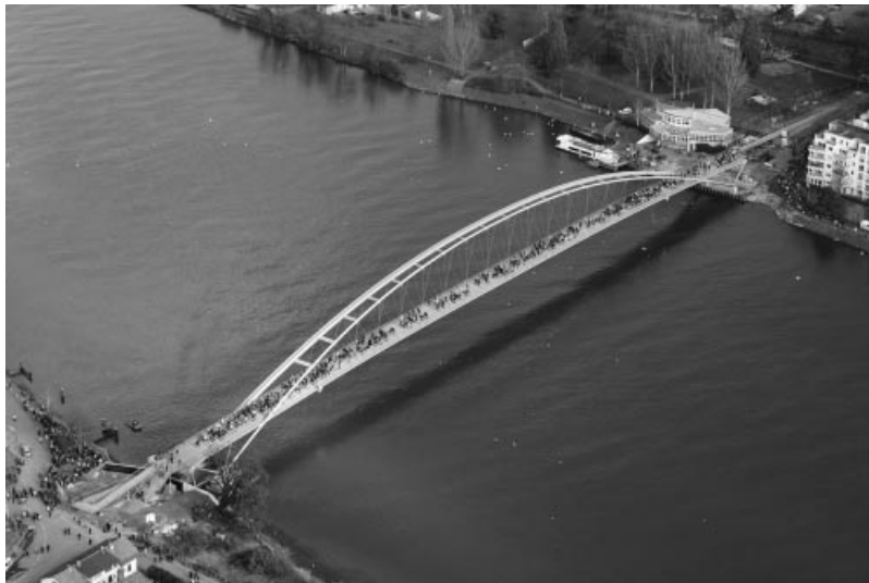
Figure 9.7 Tri-Countries Bridge pedestrian-induced vibration testing (Courtesy of Leonhardt, Andrä und Partners)
