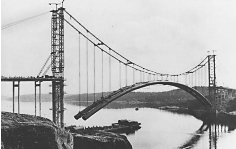
Figure 1.61 The first Tjörn Bridge under construction in 1959 (Sweden)
