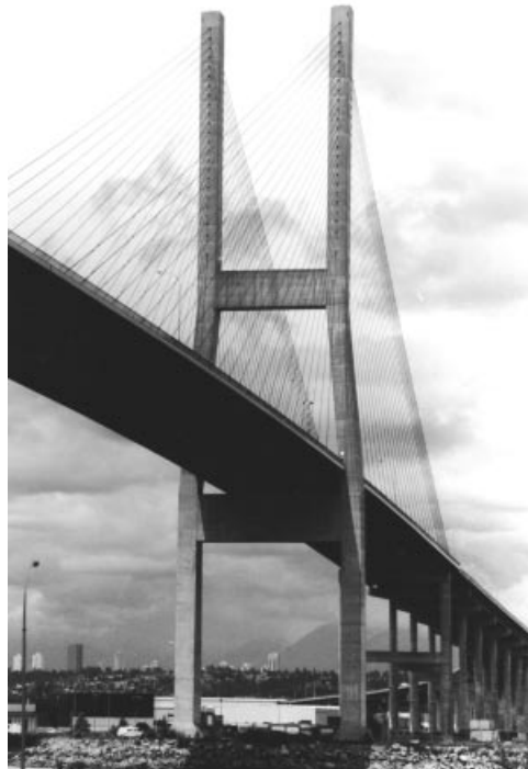
Figure 5.53 Pylon of the Alex Fraser Bridge
