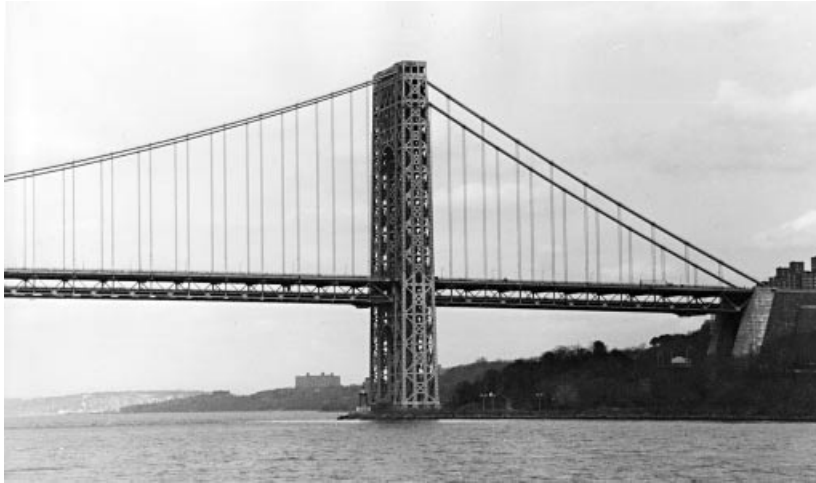
Figure 1.32 George Washington Bridge after addition of the lower deck (USA)
