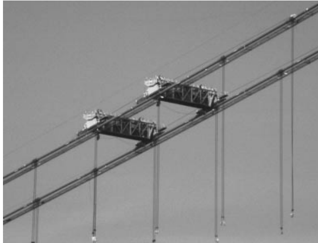
Figure 7.56 Gantry cranes on the Storebælt Bridge main cables
