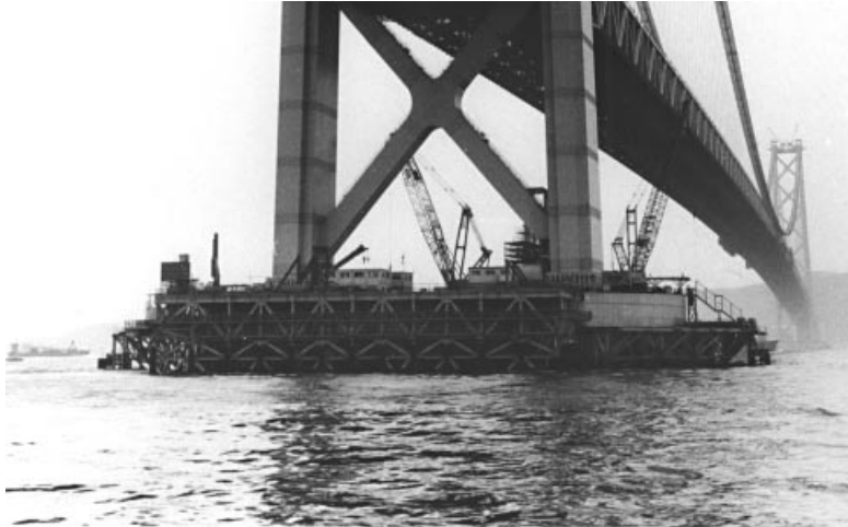
Figure 7.50 Temporary work site at the pylon pier (Akashi Kaikyo Bridge)
