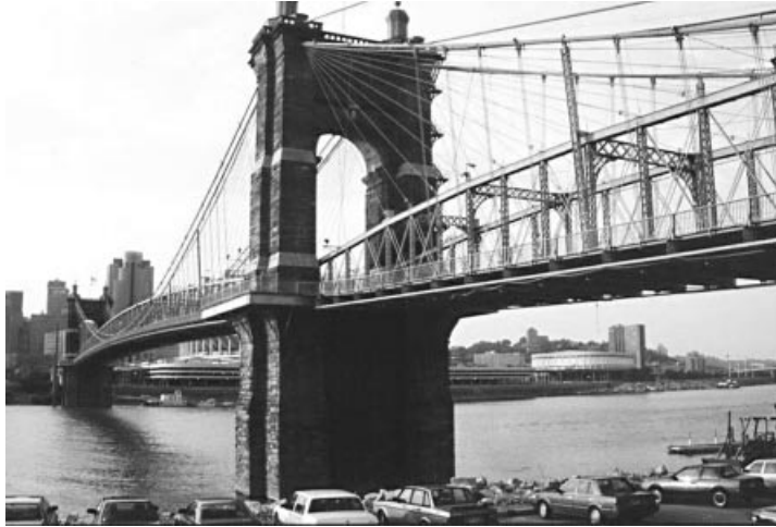
Figure 1.5 The suspension bridge across the Ohio River between Cincinnati and Covington (USA)
