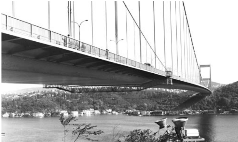
Figure 1.77 Fatih Sultan Mehmet Bridge (Second Bosphorus Bridge) (Turkey)
