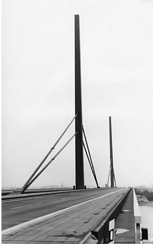
Figure 1.34 Norderelbe Bridge in its initial form (Germany)
