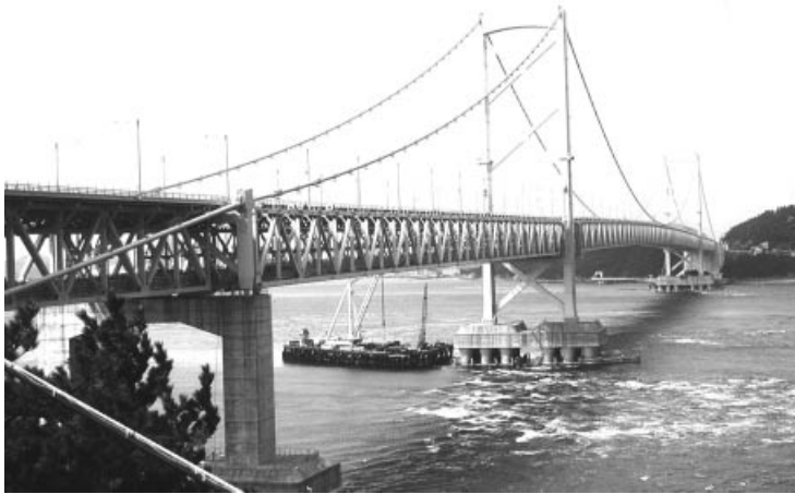
Figure 1.65 Ohnaruto Bridge (Japan)
