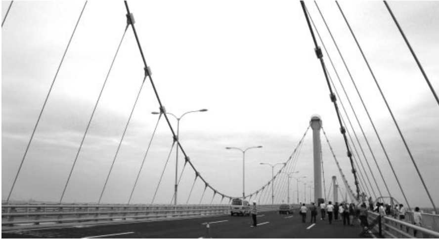
Figure 1.111 Jiangdong Bridge (China)
