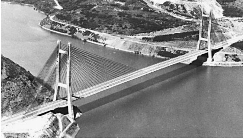
Figure 1.64 Barrios de Luna Bridge (Spain)
