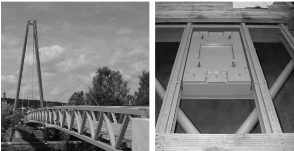
Figure 9.8 Forchheim Bridge TMD (Courtesy of Maurer Söhne)
