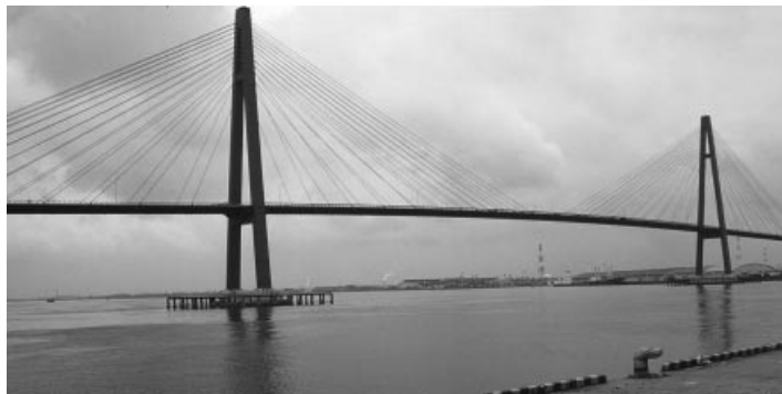
Figure 1.66 Meiko Nishi Bridge at Nagoya (Japan)
