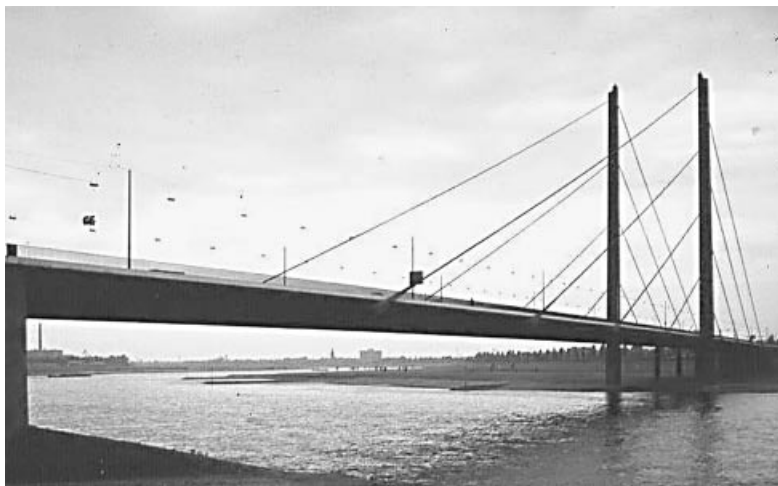
Figure 3.119 Knie Bridge at Düsseldorf
