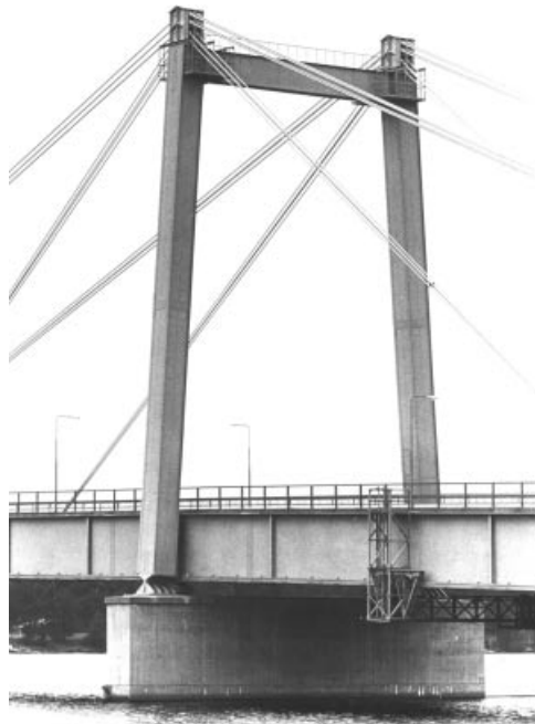
Figure 5.10 Pylon of the Strömsund Bridge
