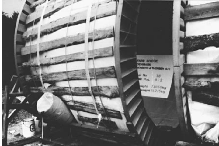
Figure 2.32 PWS with PE tube reeled for transportation (Farø Bridge)
