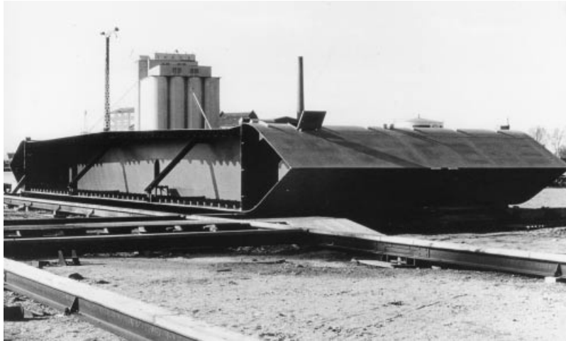
Figure 7.57 Fabrication unit for the deck of the Lillebælt Bridge
