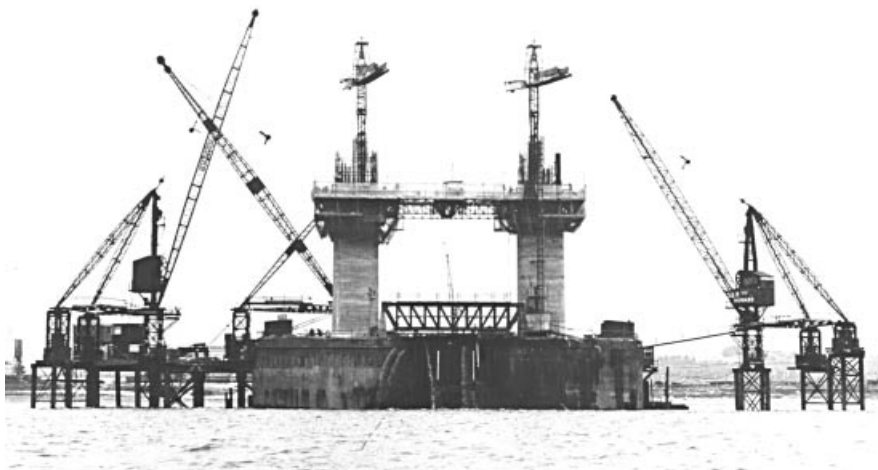
Figure 7.6 Slip forming of the Humber Bridge pylon
