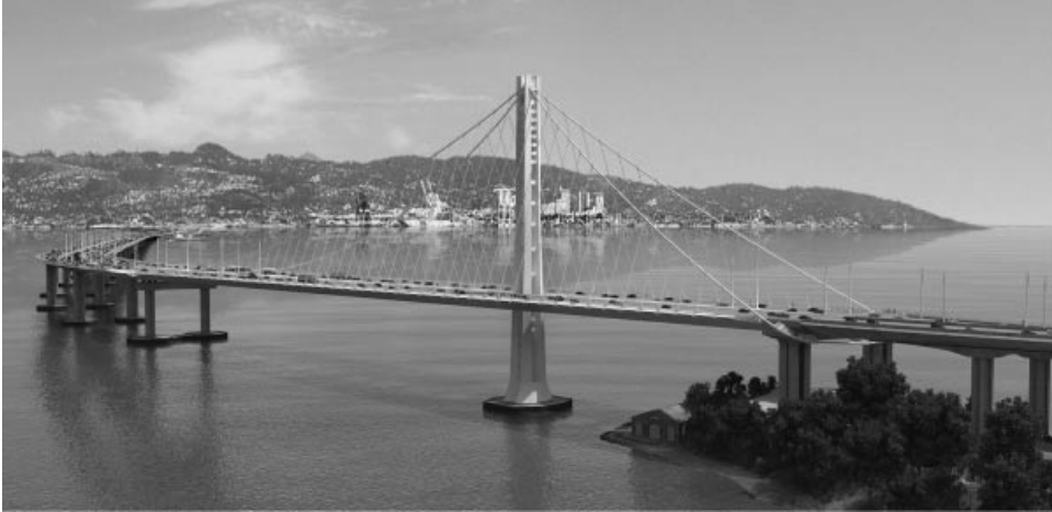
Figure 9.11 New Oakland Bay Suspension Bridge (Copyright Caltrans)
