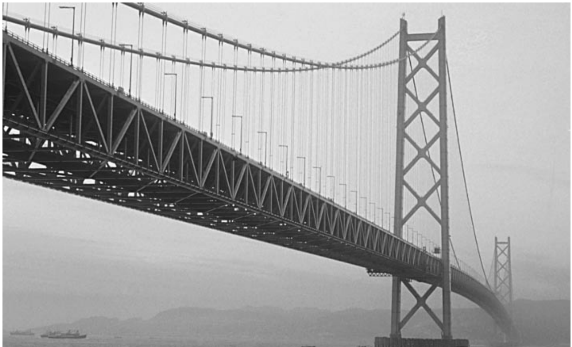
Figure 1.95 Akashi Kaiko Bridge (Japan)
