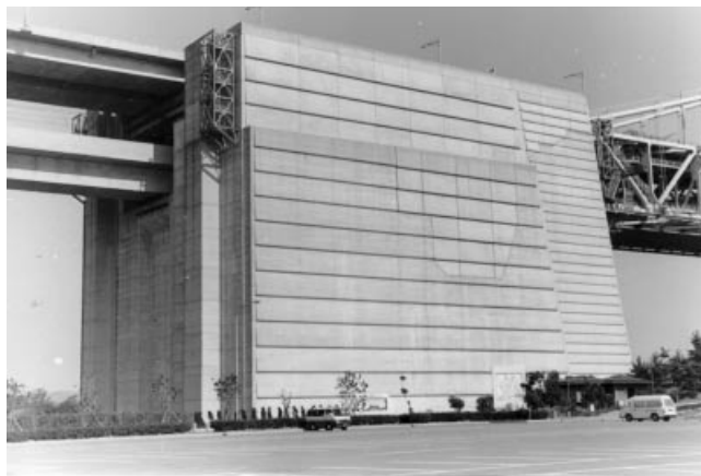
Figure 6.84 Anchor block of the Bisan Seto Bridges
