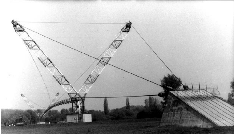
Figure 3.181 Pipeline bridge across the Danube River at Barbara
