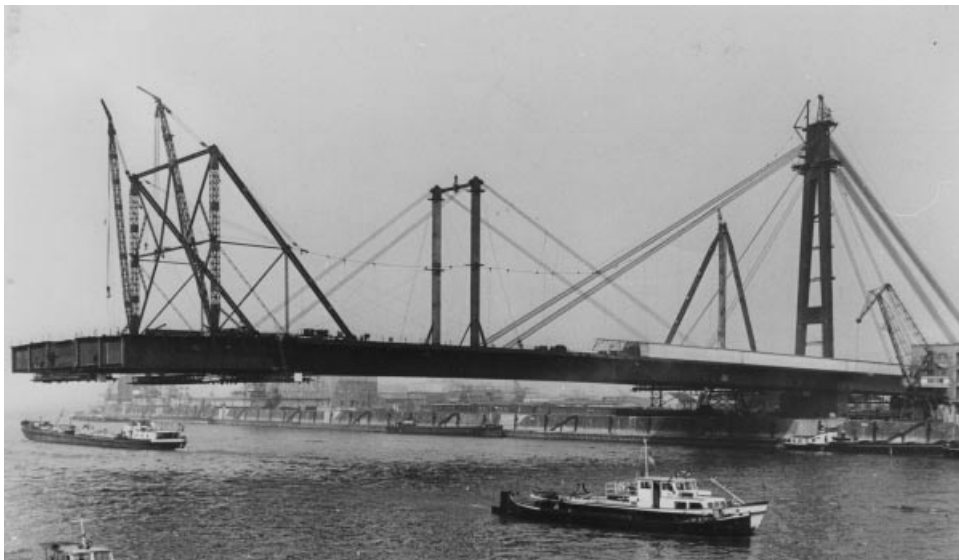
Figure 7.86 The Rhine Bridge between Mannheim and Ludwigshafen during erection
