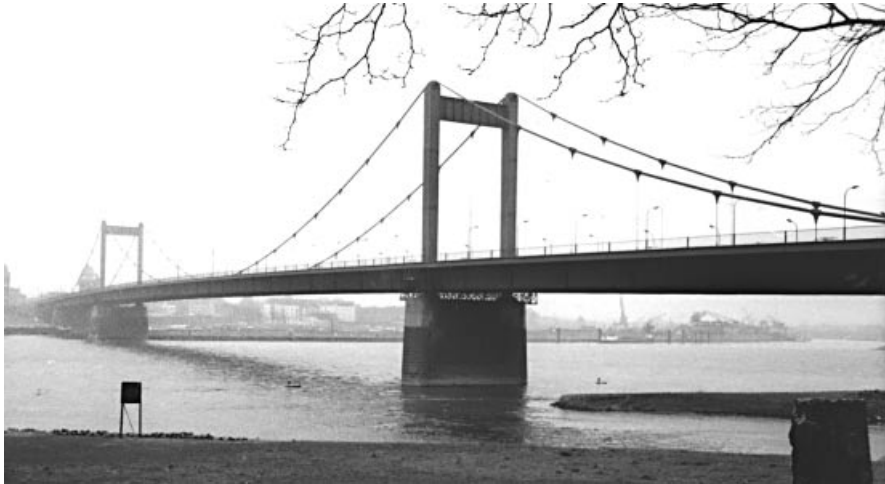
Figure 1.27 Duisburg–Ruhrort Bridge across the Rhine (Germany)
