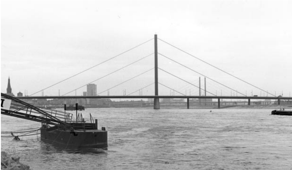
Figure 3.19 Oberkasseler Bridge in Düsseldorf (harp system with intermediate supports in the side span)
