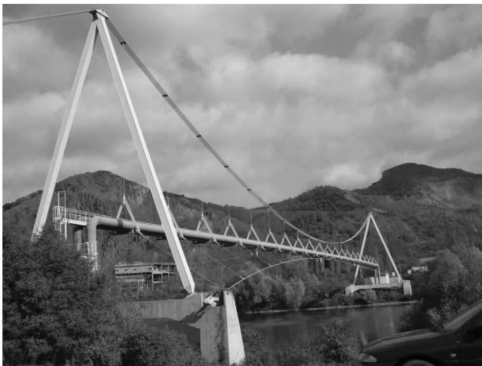
Figure 3.180 Pipeline bridge across the Labe River in the Czech Republic
