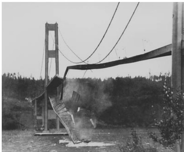
Figure 8.3 Tacoma Narrows Bridge at the moment of girder failure. (Reproduced with permission from University of Washington Press)
