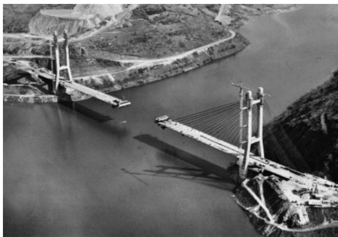
Figure 7.83 The Barrios de Luna Bridge during construction
