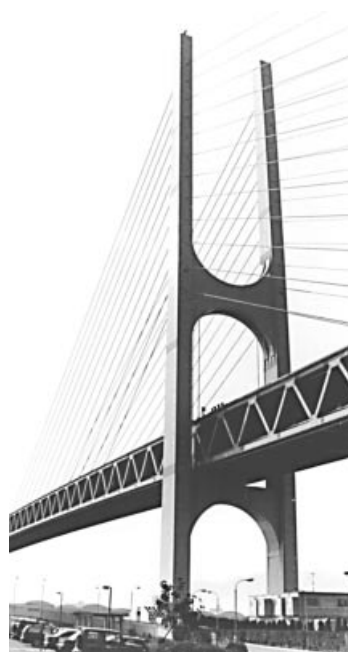
Figure 5.55 Pylon of the Higashi Kobe Bridge
