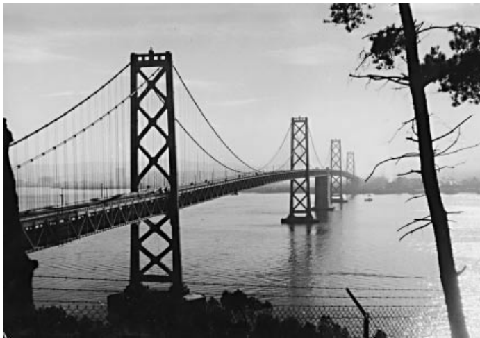
Figure 1.14 The West Bay crossing of the San Francisco–Oakland Bay Bridge (USA)
