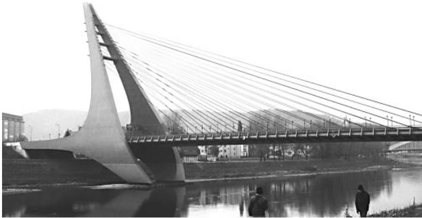
Figure 1.97 Mariánský Bridge (Czech Republic)
