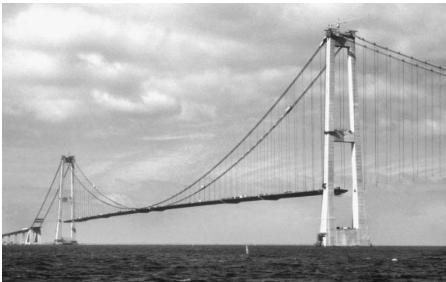
Figure 7.46 The Storebælt East Bridge after erection of the main span deck
