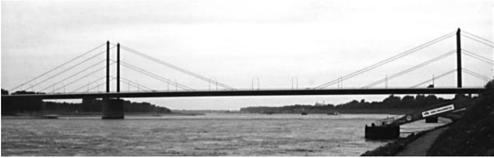
Figure 1.29 Theodor Heuss Bridge across the Rhine at Düsseldorf (Germany)
