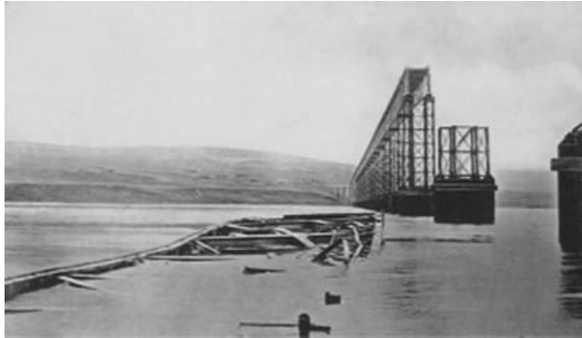
Figure 8.2 Tay Bridge after its collapse in 1879
