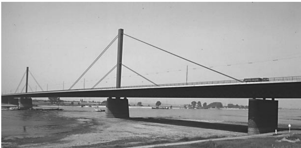
Figure 1.38 The bridge across the Rhine at Leverkusen (Germany)
