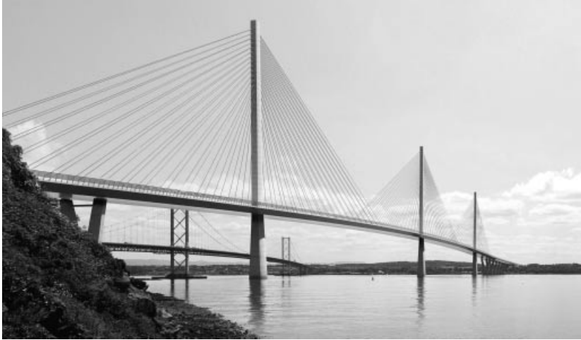
Figure 1.115 Third Bridge across the Firth of Forth in Scotland (visualisation by Dissing+Weitling Architecture)
