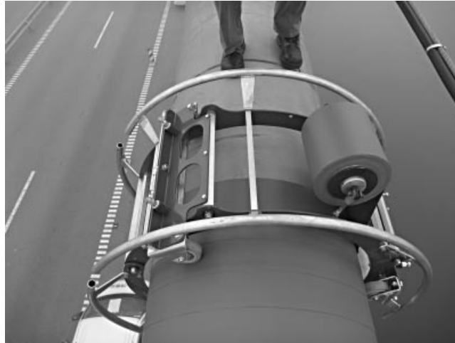
Figure 2.30 Wrapping with polyethylene strips to achieve air tightness (Photo credit: Ove Sørensen, COWI)
