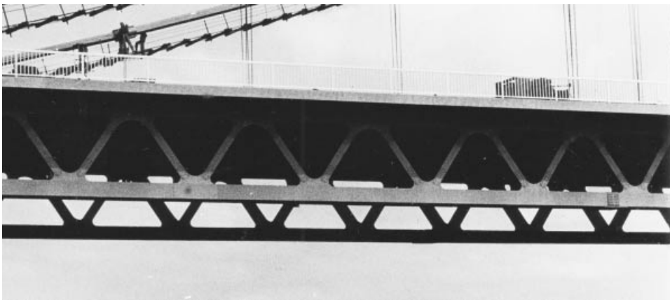
Figure 4.91 Stiffening truss of the Emmerich Bridge
