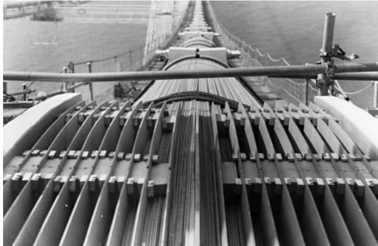
Figure 7.32 Cable saddle with spacer plates
