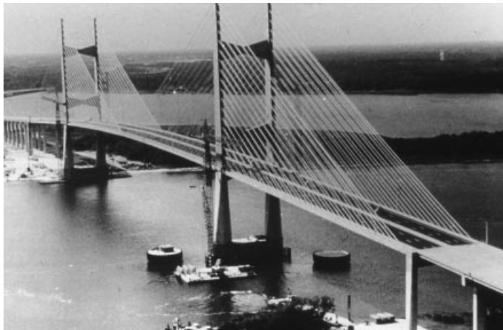
Figure 3.121 Napoleon Bonaparte Broward Bridge (Dames Point Bridge)
