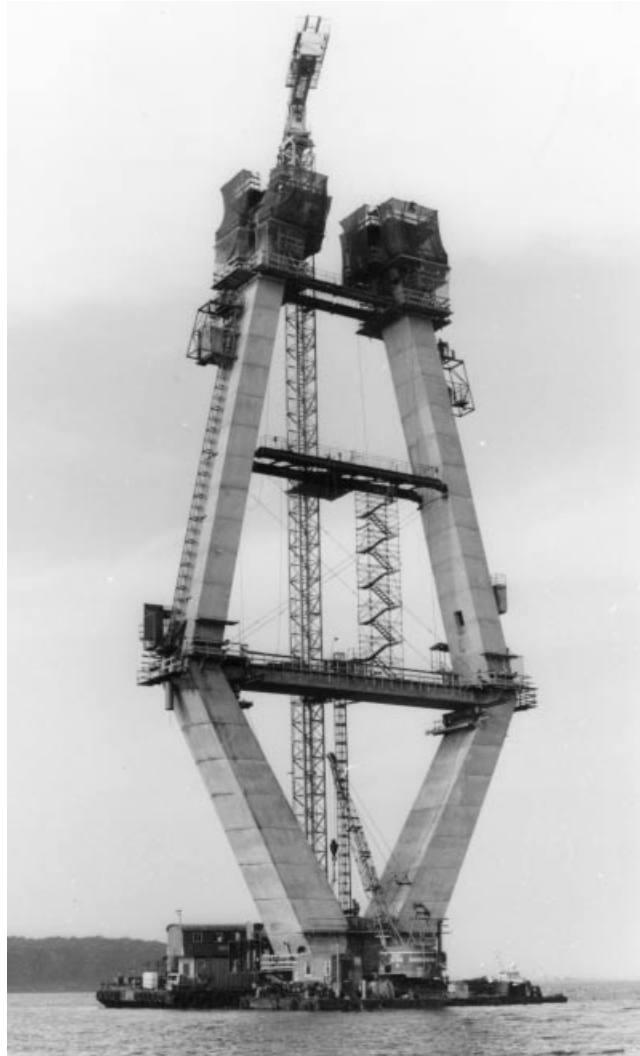
Figure 7.9 Pylon of the Farø Bridge during construction
