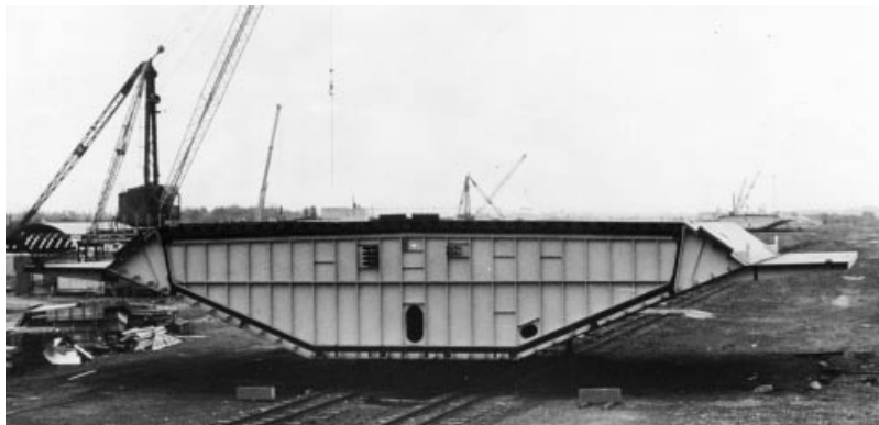
Figure 4.68 Erection unit for the Humber Bridge
