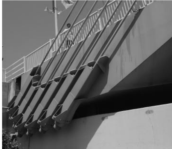
Figure 3.91 Anchor cable composed of six individual strands (Jindo Bridge)
