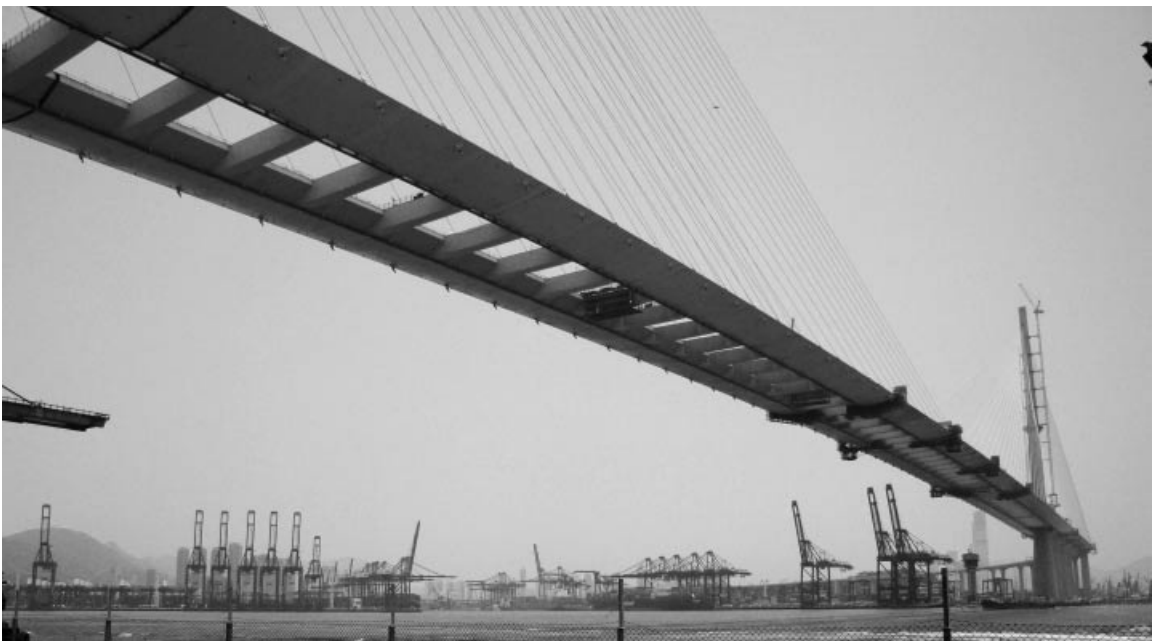
Figure 1.112 Stonecutters Bridge (Hong Kong SAR)
