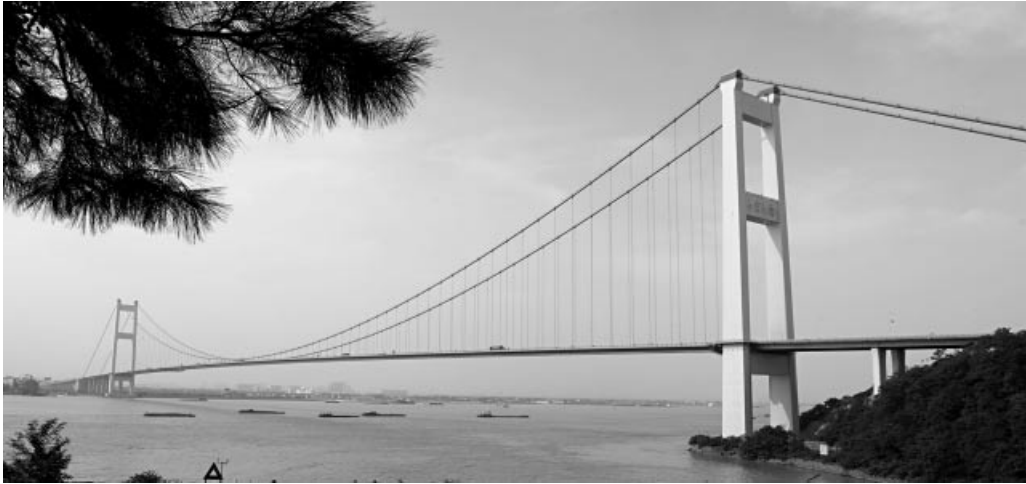
Figure 1.99 Jiangyin Bridge across Yangtze River (China). (Courtesy of Bridge Magazine)
