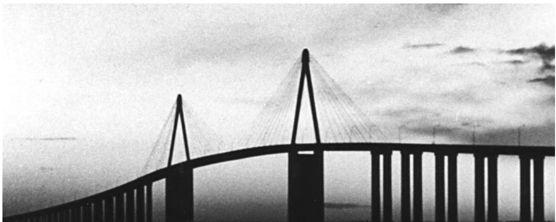
Figure 1.53 Saint Nazaire Bridge with a 404 m long main span across the Loire (France)
