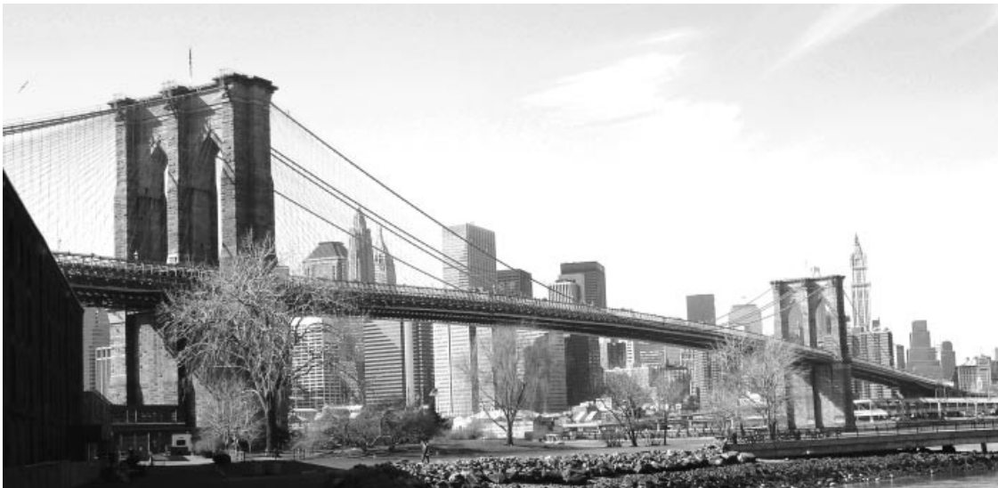
Figure 1.6 Brooklyn Bridge across the East River in New York (USA)
