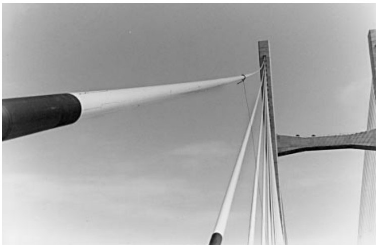
Figure 2.35 Parallel-strand cable of the Second Severn Bridge with plastic cover
