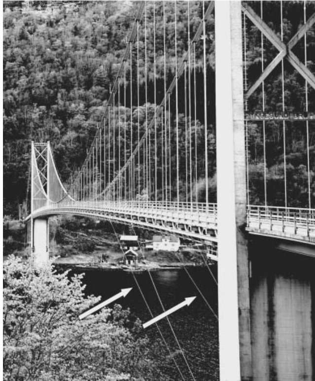
Figure 8.4 Fyksesund Bridge, Norway (1937). Note girder ties
