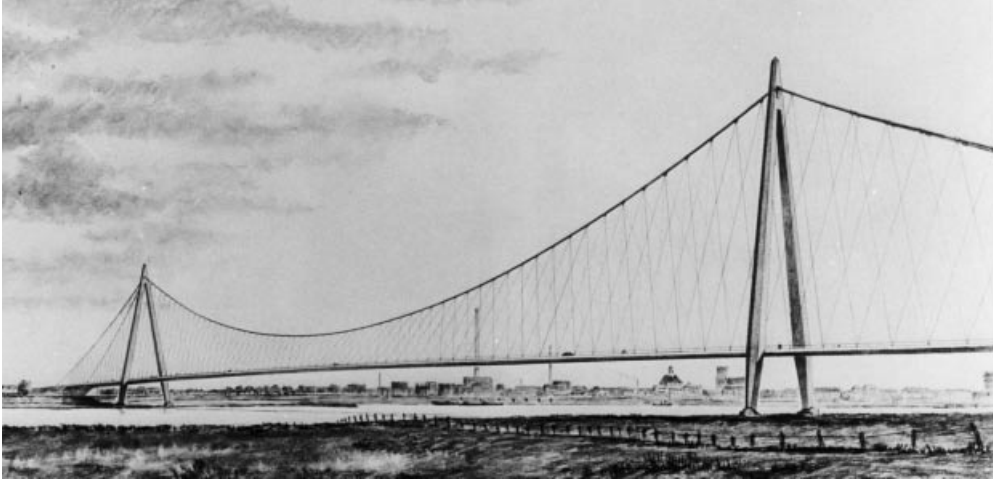
Figure 3.60 Mono-cable bridge proposed in the early 1960s by F. Leonhardt for the Emmerich Bridge across the Rhine
