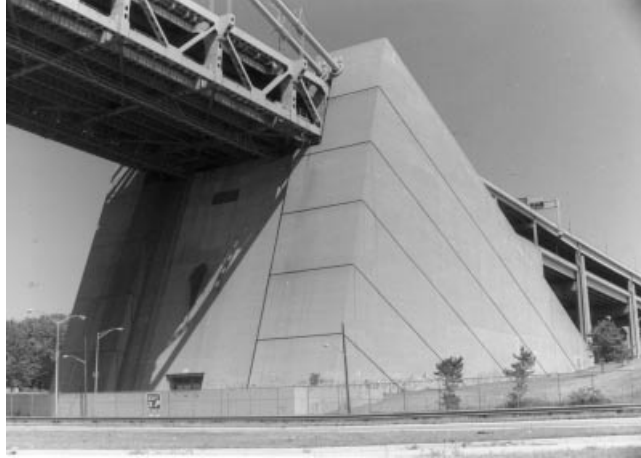
Figure 6.83 Anchor block of the Verrazano Narrows Bridge
