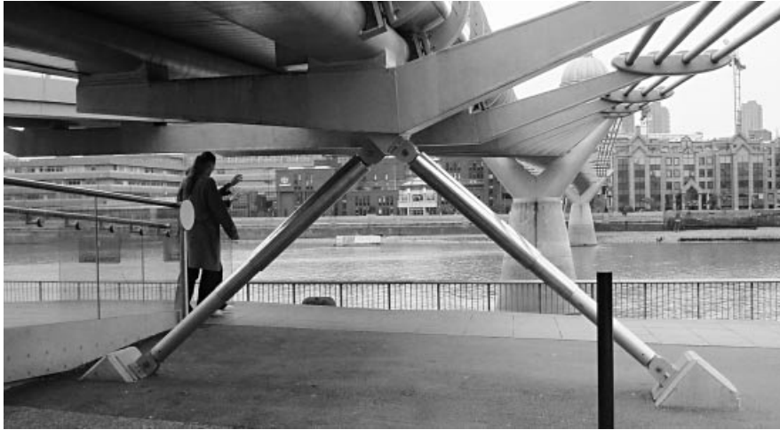
Figure 1.105 London Millennium Bridge with dampers
