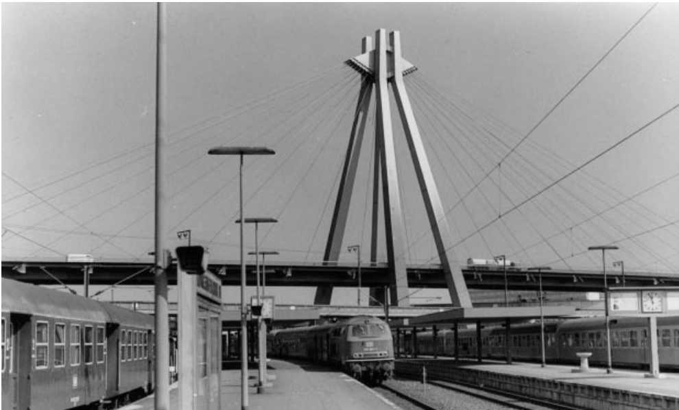
Figure 3.21 Two-span cable stayed bridge in Ludwigshafen, Germany
