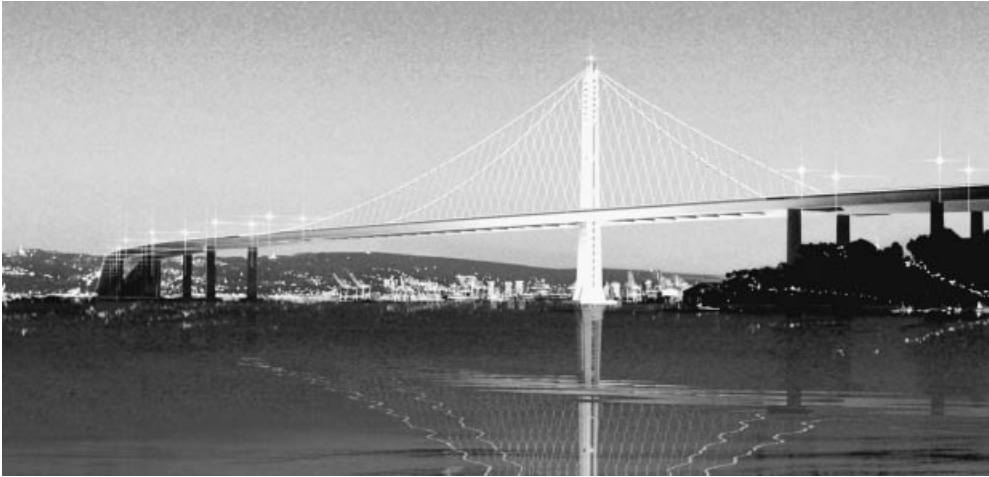
Figure 4.81 The self anchored suspension bridge of the new East Bay Crossing at San Francisco (Image © Caltrans)
