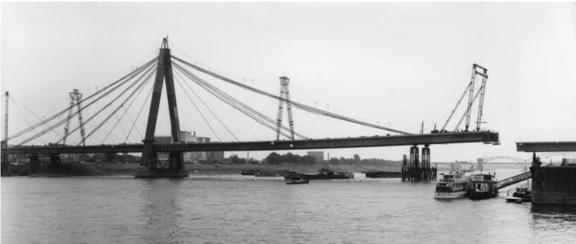
Figure 7.73 The Severins Bridge under construction in 1959
