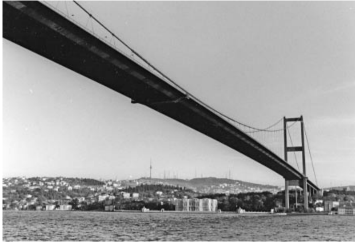
Figure 1.50 First Bosphorus Bridge at Istanbul (Turkey)
