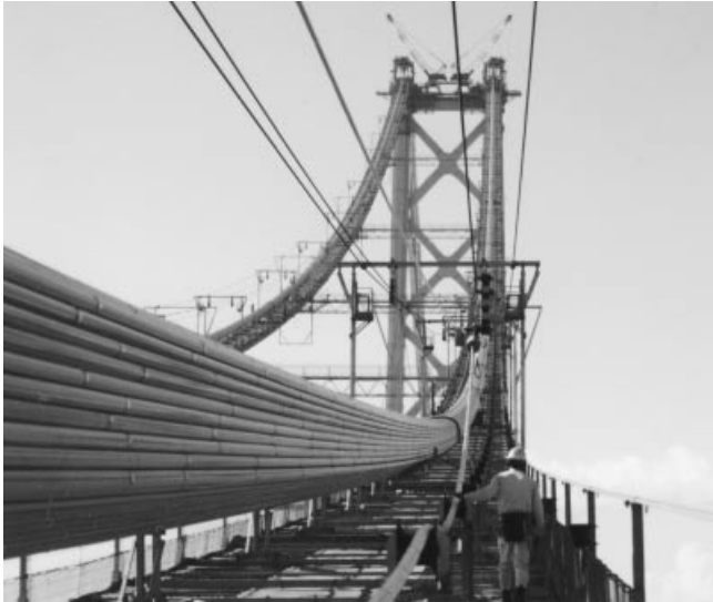
Figure 7.30 PPWS in the process of being pulled across on the catwalk
