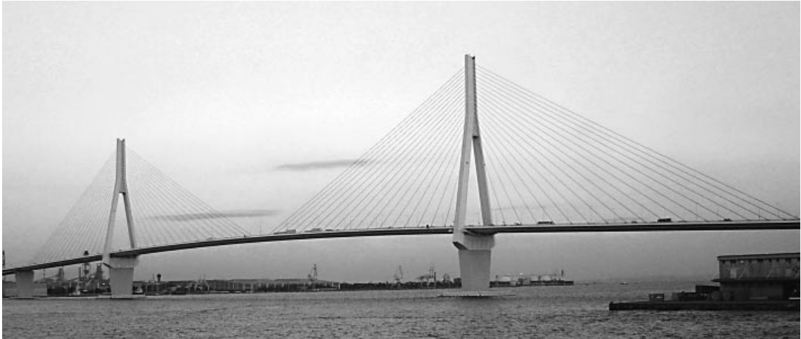
Figure 1.85 Tsurumi Tsubasa Bridge (Japan)
