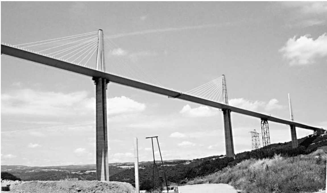
Figure 1.109 Millau Viaduct (France)
