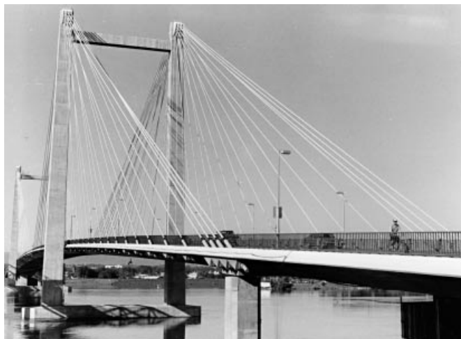
Figure 1.57 Pasco–Kennewick Bridge across the Columbia River (USA)
