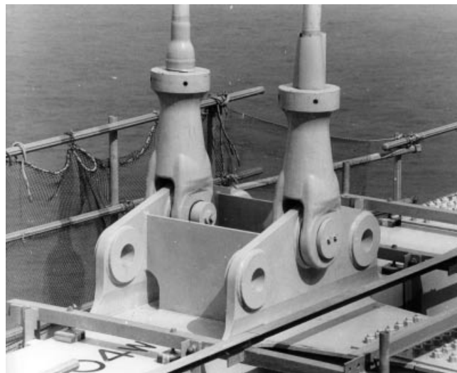
Figure 6.15 Fork sockets on the hangers of the Akashi Kaikyo Bridge
