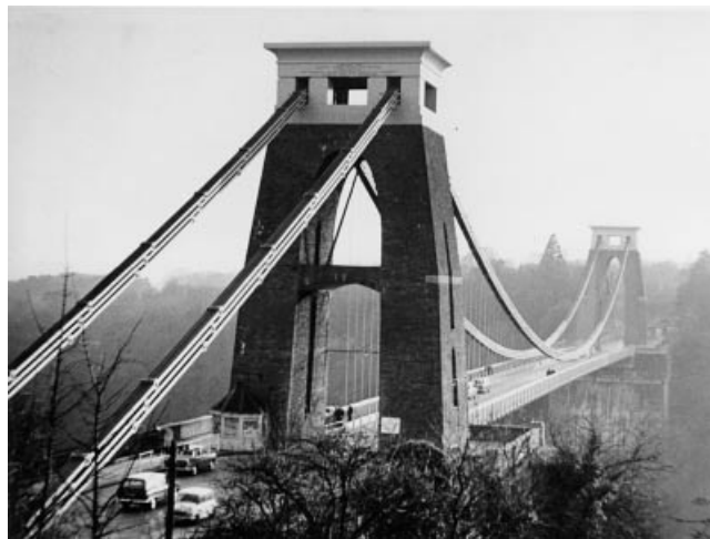
Figure 1.2 Clifton Suspension Bridge (UK)
