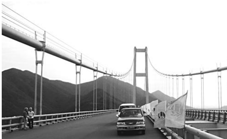
Figure 1.114 Xihoumen Bridge (China)
