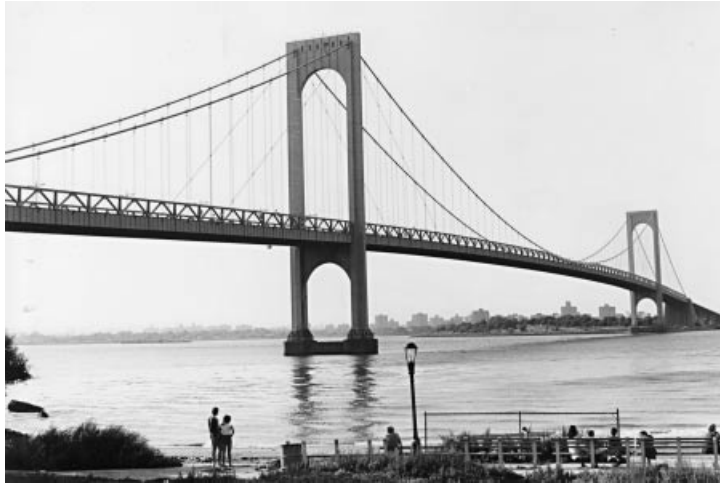
Figure 1.18 Bronx–Whitestone Bridge after the first strengthening to improve the aerodynamic stability (USA)
