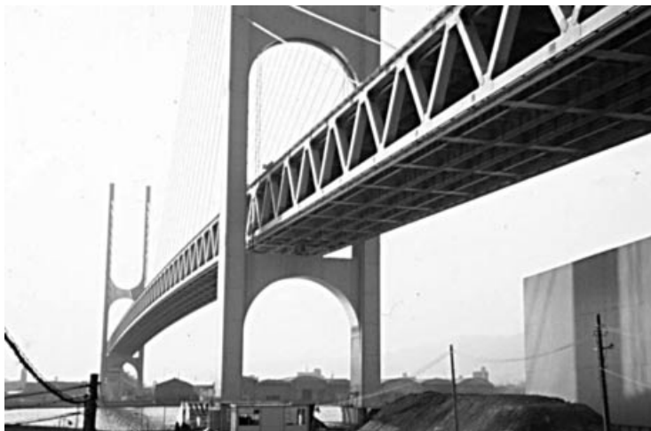
Figure 1.84 Higashi Kobe Bridge (Japan)
