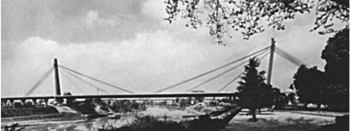
Figure 1.56 Indiano Bridge across the Arno near Firenze. First major cable-stayed bridge with an earth anchored cable system (Italy)
