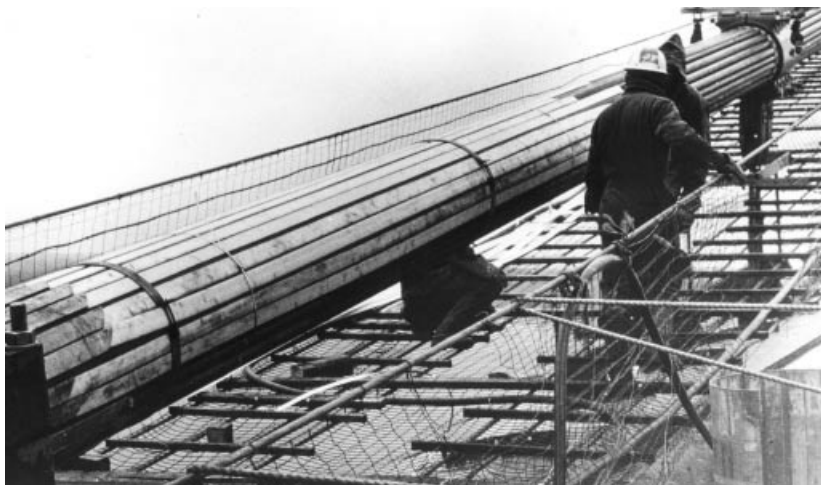
Figure 2.19 Lillebælt Bridge main cable with polyethylene fillers to achieve a circular shape
