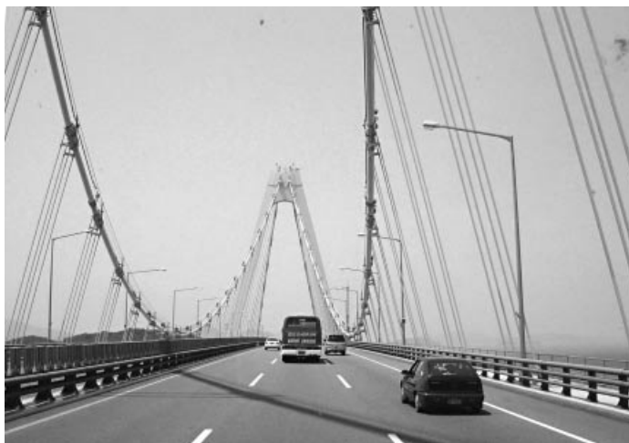
Figure 1.103 Youngjong Bridge (Korea)
