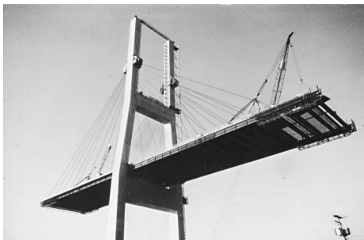
Figure 7.67 The Alex Fraser Bridge during erection
