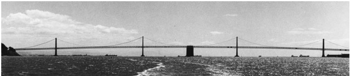
Figure 3.134 West Bay crossing of the San Francisco–Oakland Bay Bridge comprising two consecutive three-span suspension bridges
