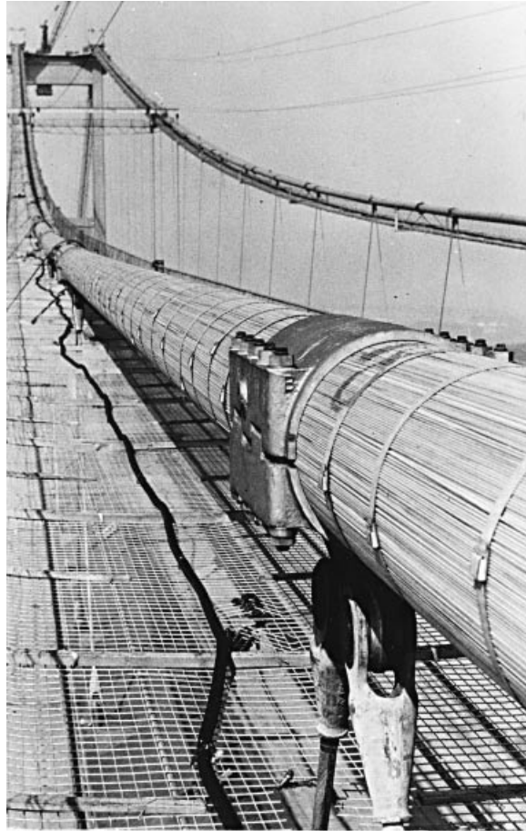
Figure 2.22 Main cable of the Severn Bridge after compaction
