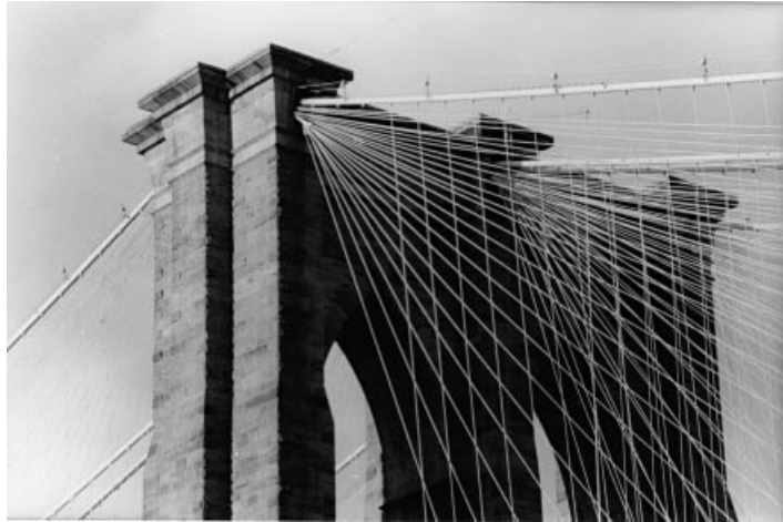
Figure 1.7 The cable system of the Brooklyn Bridge at the pylon (USA)
