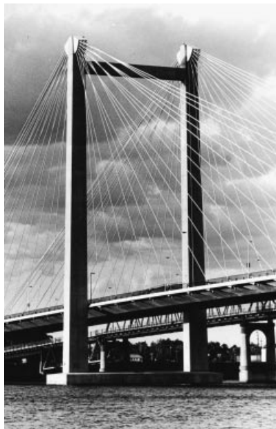
Figure 5.37 Pylon of the Pasco–Kennewick Bridge
