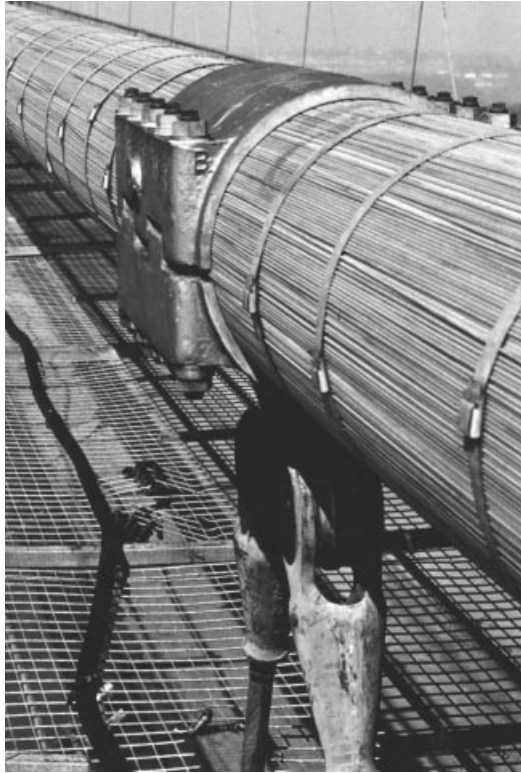
Figure 6.53 Cable clamp in the Severn Bridge
