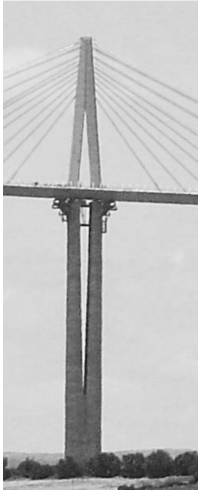
Figure 5.78 Pylon of the Millau Viaduct
