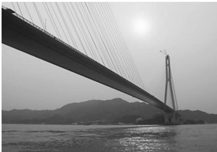
Figure 1.100 Tatara Bridge (Japan)
