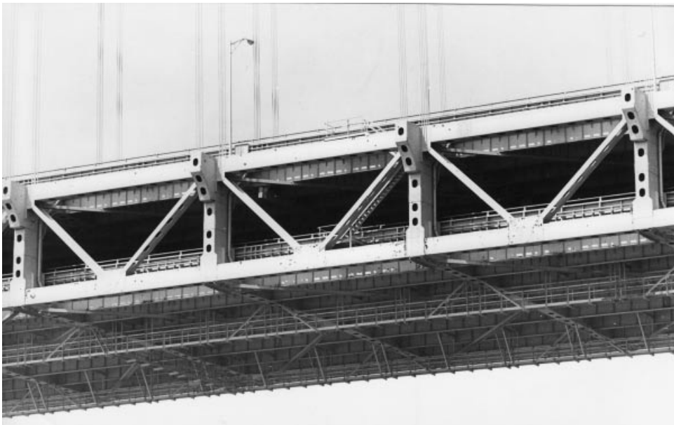
Figure 4.89 Truss of the Verrazano Narrows Bridge
