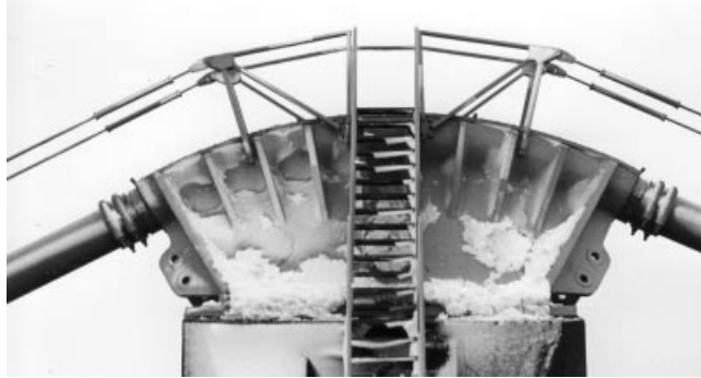
Figure 6.68 Cable saddle of the Lillebælt Bridge in the final condition
