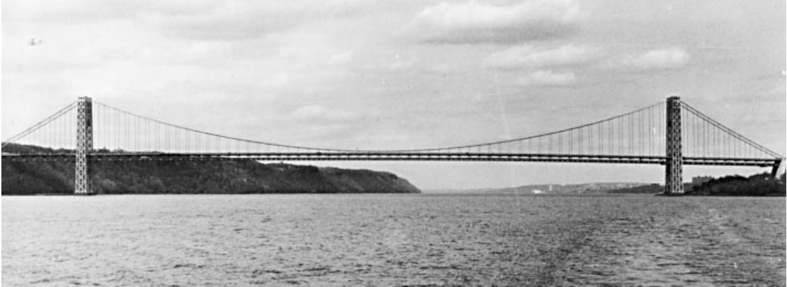
Figure 3.36 George Washington Bridge
