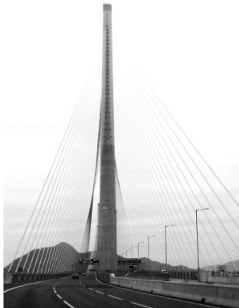
Figure 5.57 Pylon of the Stonecutters Bridge
