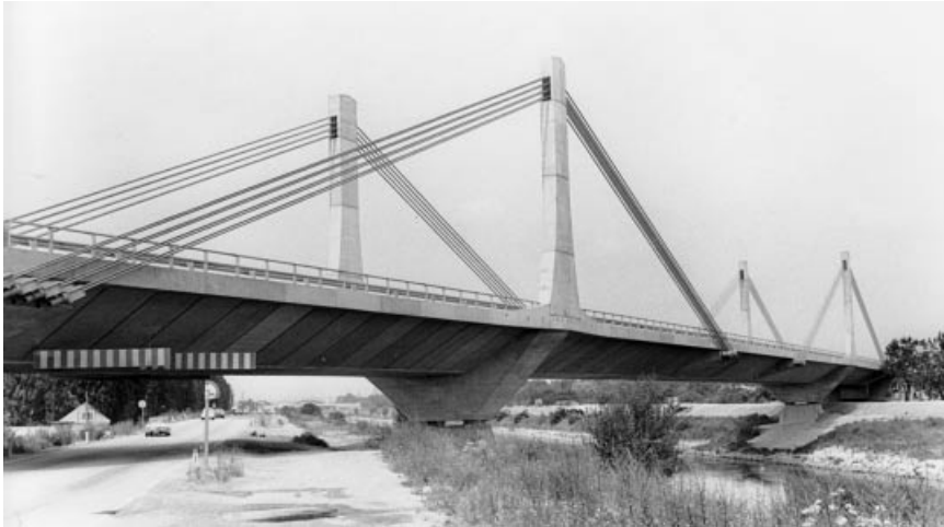
Figure 1.43 Danube Canal Bridge in Vienna (Austria)
