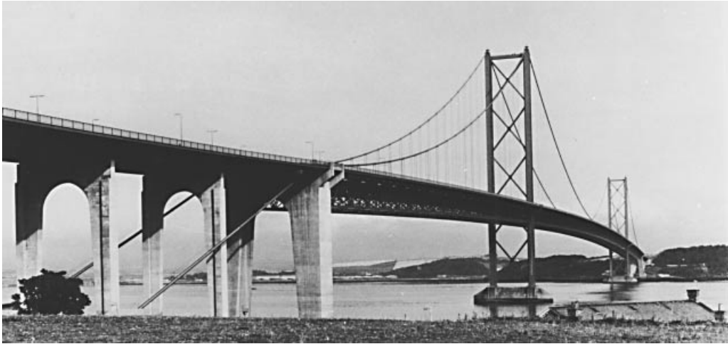
Figure 1.37 Firth of Forth Road Bridge in Scotland (UK)
