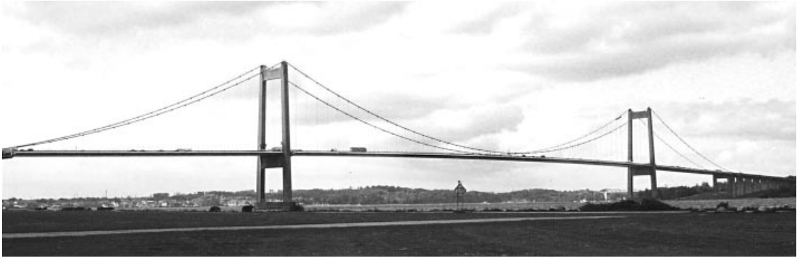
Figure 1.47 Lillebælt Suspension Bridge (Denmark)
