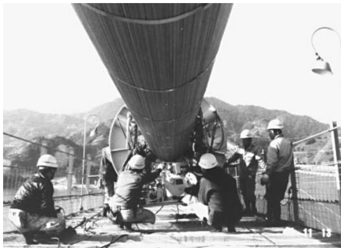
Figure 7.33 Compaction of the main cable in the Innoshima Bridge
