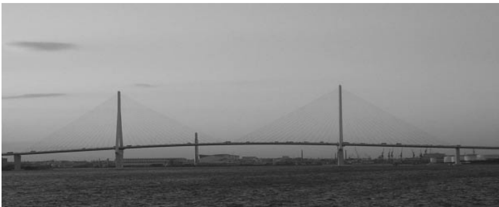
Figure 3.94 The Turumi Tsubasa Bridge in Japan
