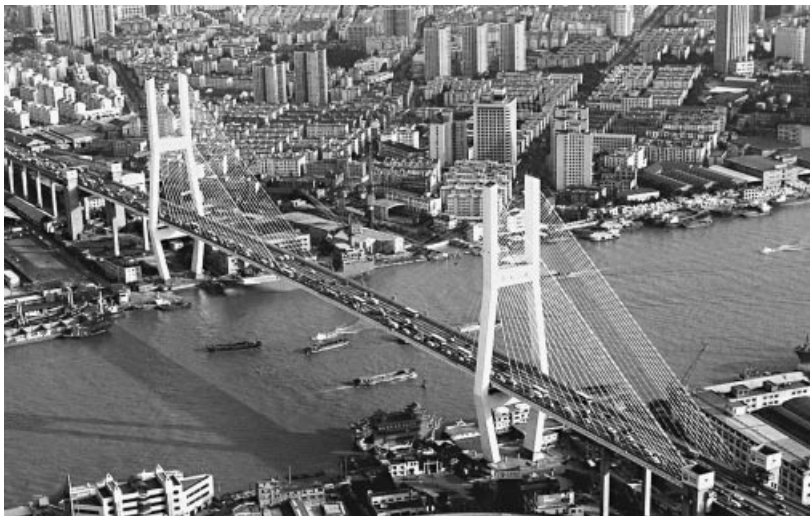
Figure 1.80 Nanpu Bridge in Shanghai (China). (Courtesy of Bridge Magazine)
