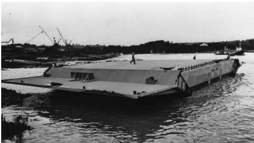
Figure 7.58 Self-floating erection unit for the deck of the Severn Bridge
