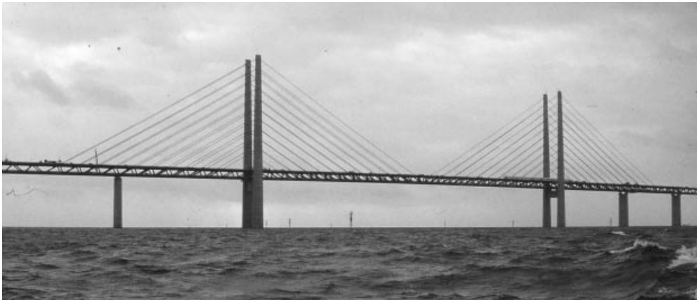
Figure 3.126 The main span of the Øresund Bridge
