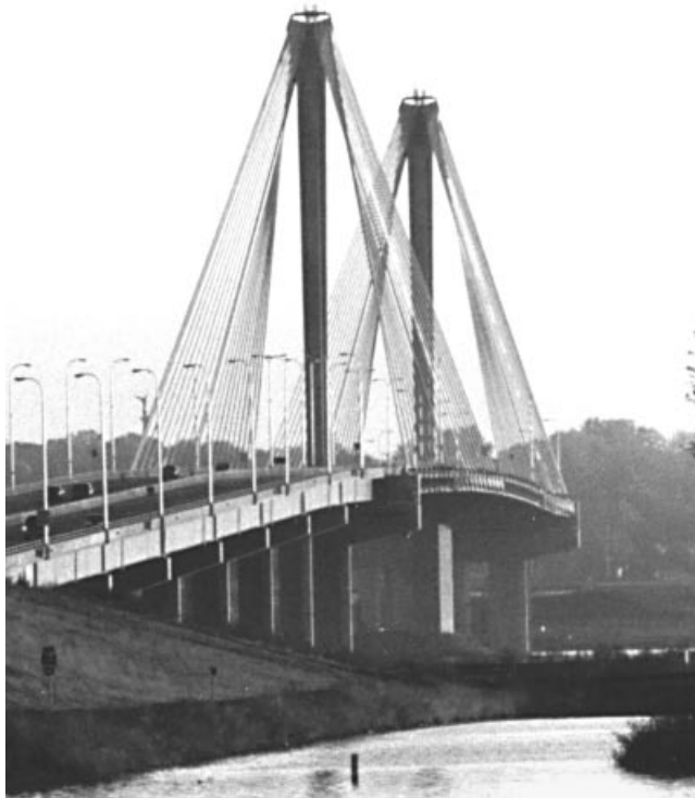
Figure 1.86 Clark Bridge across the Mississippi (USA)
