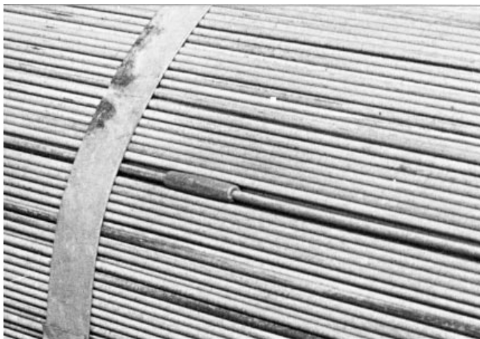
Figure 7.22 Splice in a wire of a suspension bridge main cable
