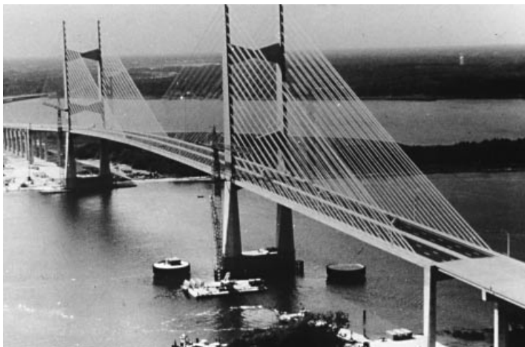
Figure 1.79 Napoleon Bonaparte Broward Bridge (Dames Point Bridge) at Jacksonville in Florida (USA)
