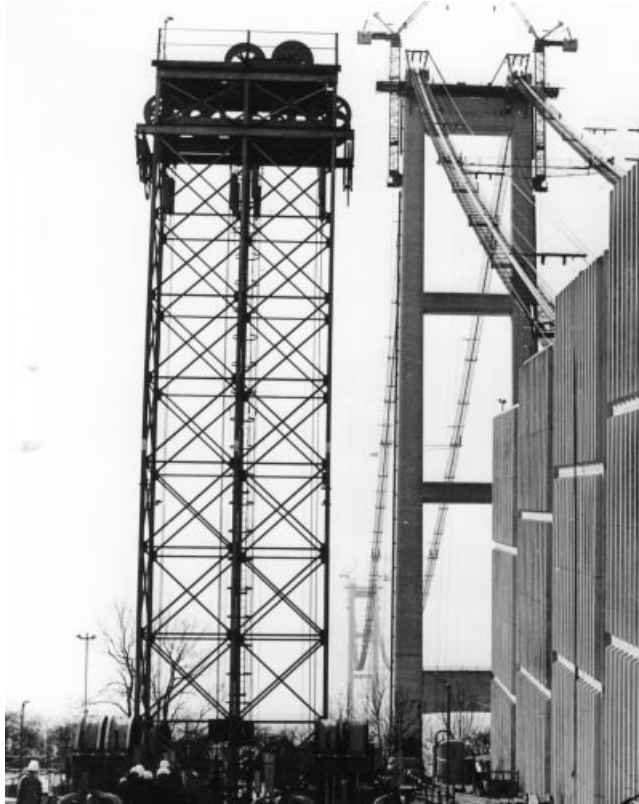
Figure 7.23 Counterweight tower at the anchor block of the Humber Bridge
