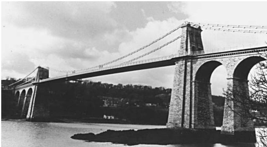
Figure 1.1 The suspension bridge across the Menai Strait (UK)
