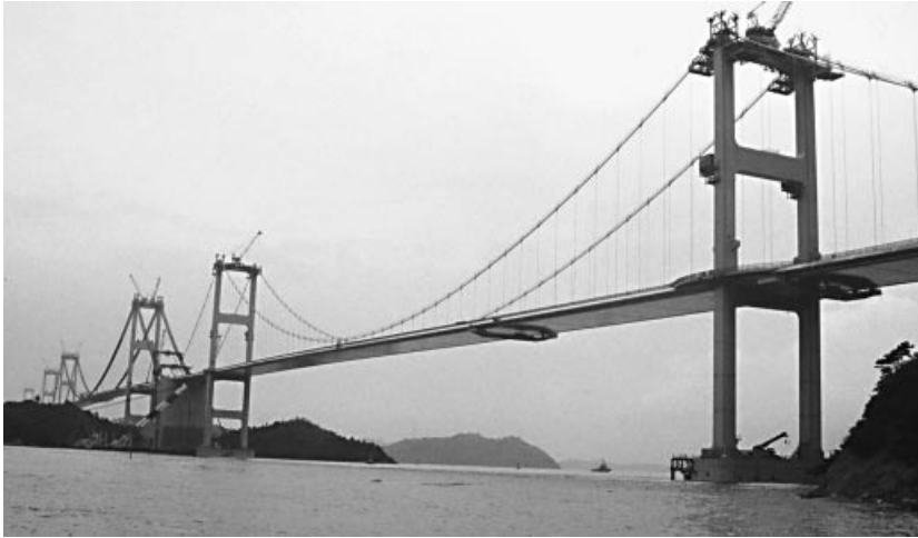
Figure 1.101 Kurushima Kaikyo Bridges in the final construction phase (Japan)
