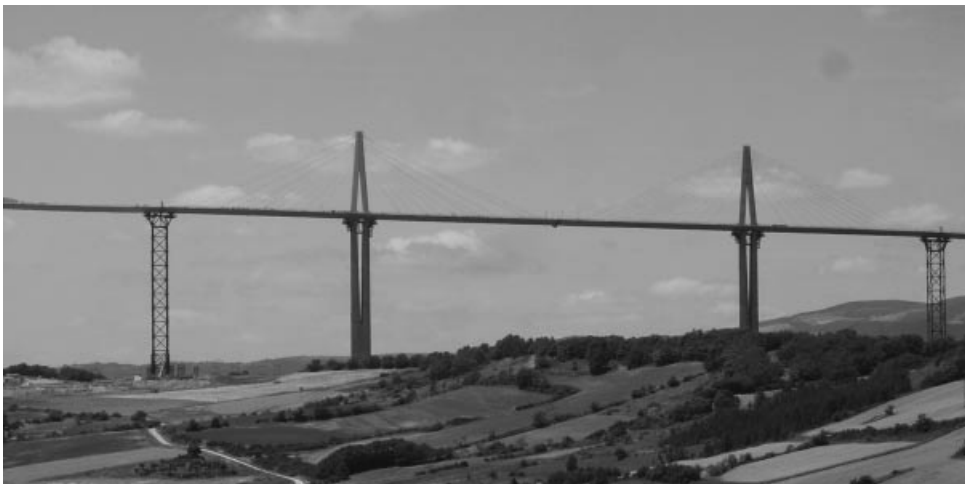
Figure 7.88 The Millau Viaduct after completion of the launching. The deck is still partly supported by the temporary supports until the remaining pylons and cable systems will be added
