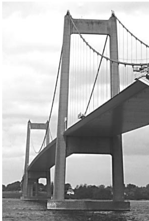
Figure 5.49 Pylon of the Lillebælt Bridge
