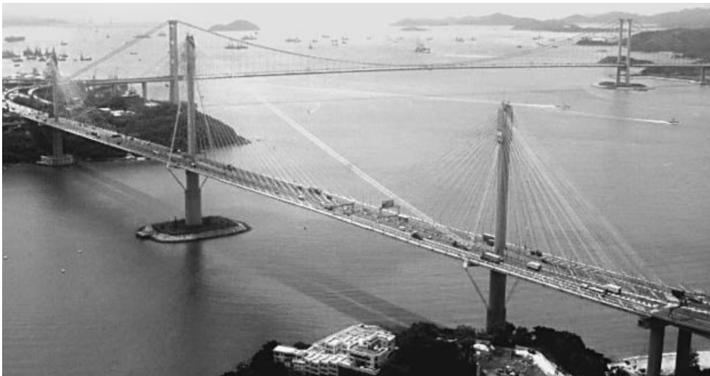
Figure 3.140 The Ting Kau Bridge in Hong Kong
