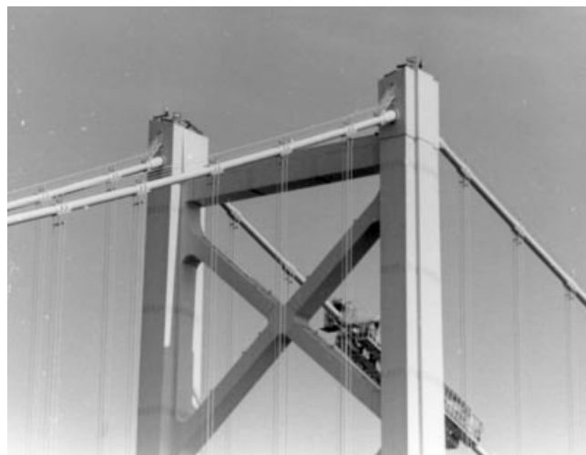
Figure 6.74 Pylon top of the Bisan Seto Bridges
