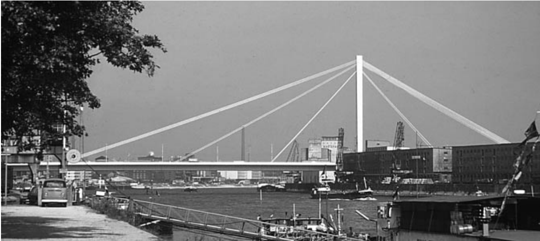
Figure 1.49 The cable-stayed bridge across the Rhine between Mannheim and Ludwigshafen (Germany)
