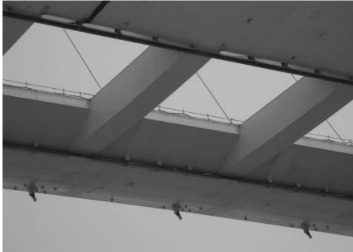
Figure 6.23 The deck of the Stonecutters Bridge as viewed from below
