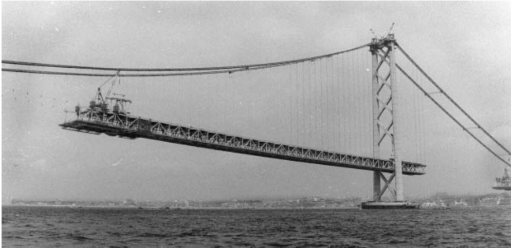
Figure 7.48 The Akashi Kaikyo Bridge during erection
