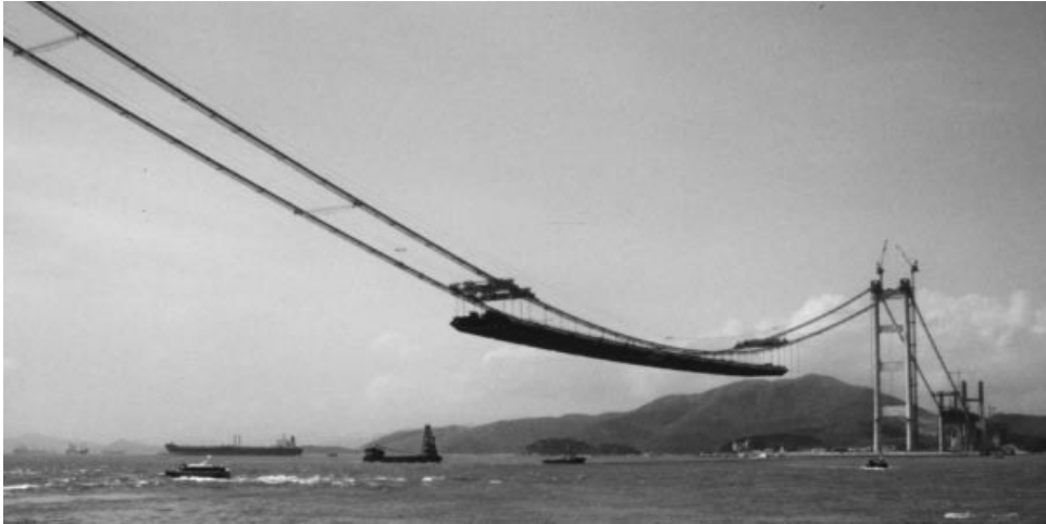
Figure 7.43 The Tsing Ma Bridge during erection
