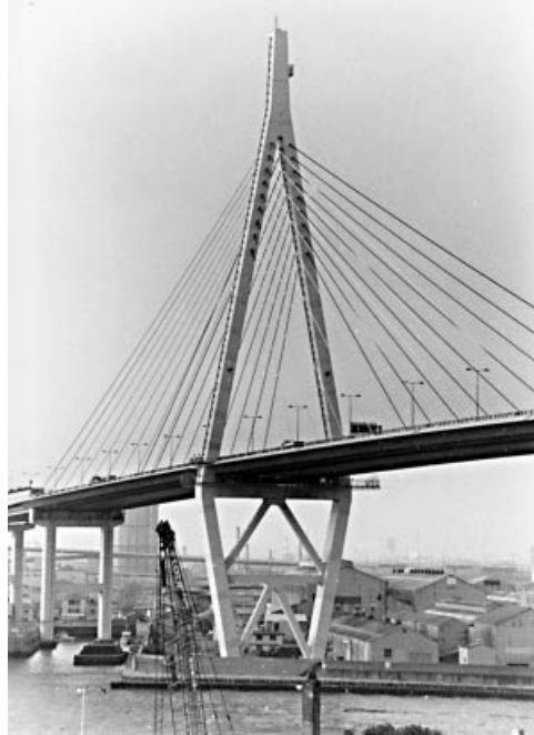
Figure 5.70 Pylon of the Tempozan Bridge
