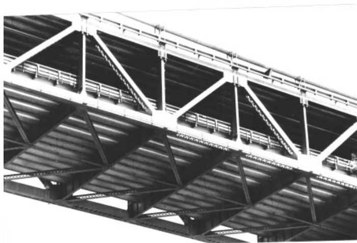
Figure 4.87 Truss of the San Francisco–Oakland Bay Bridge
