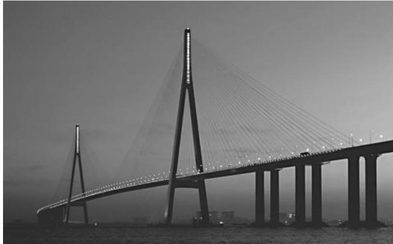
Figure 1.110 Sutong Bridge across the Yangtze River (China). (Courtesy of Bridge Magazine)
