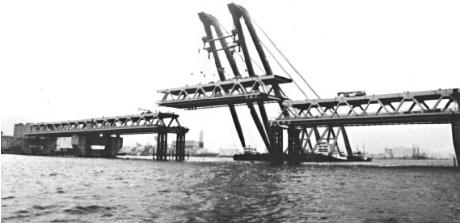
Figure 7.64 The Rokko Bridge under construction
