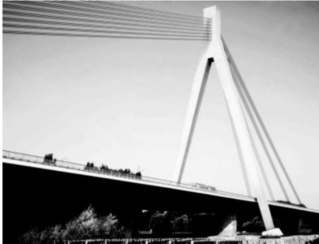
Figure 5.27 Pylon of the Rhine Bridge at Speyer
