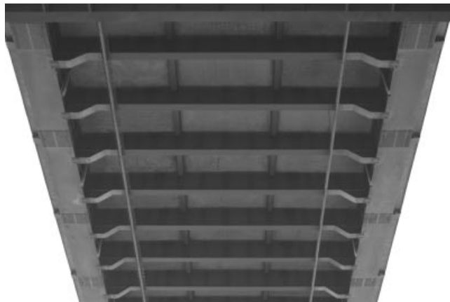
Figure 4.46 Ladder deck seen from below (Yangpu Bridge)
