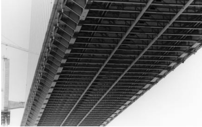
Figure 4.47 The deck of the Second Severn Bridge as seen from below
