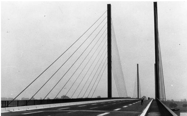
Figure 1.42 Rees Kalkar Bridge (Germany)
