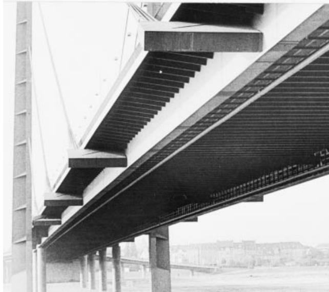
Figure 4.44 Inclined anchor girders of the Knie Bridge
