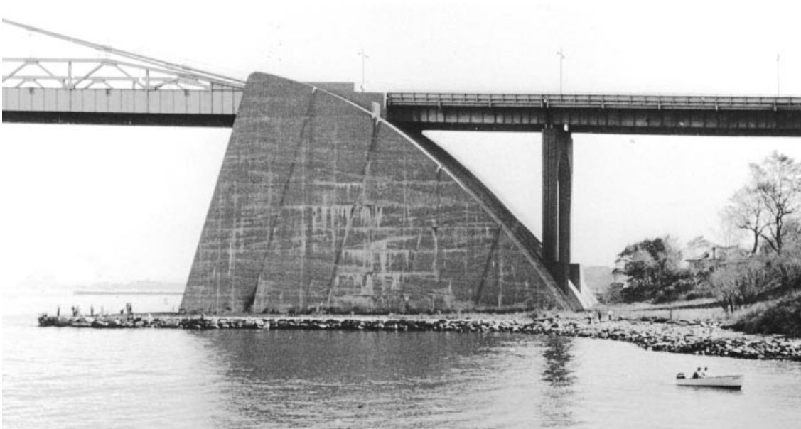
Figure 6.82 Anchor block of the Bronx Whitestone Bridge
