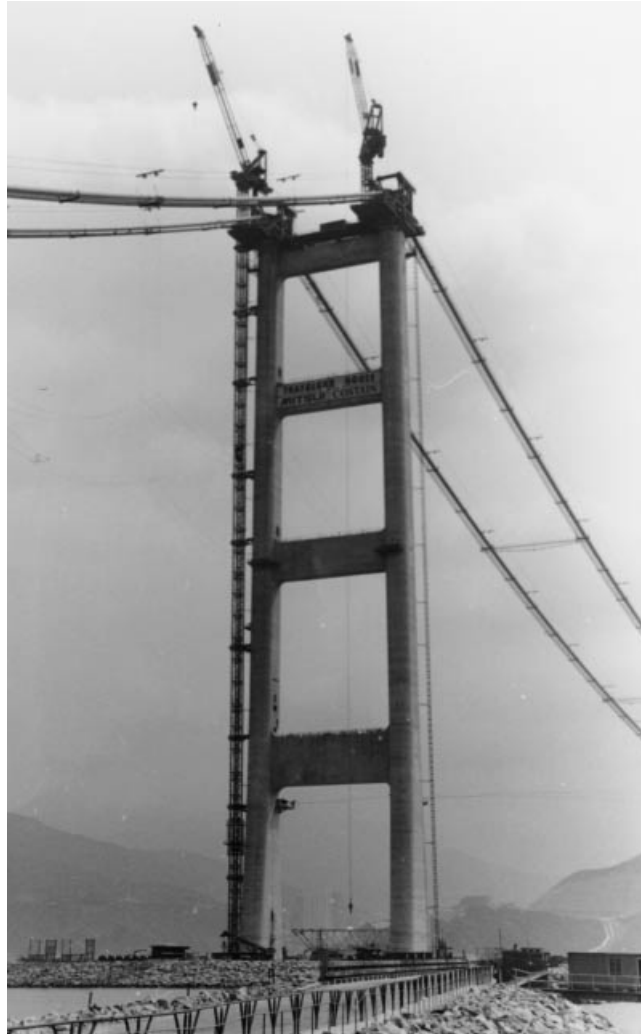
Figure 5.51 Pylon of the Tsing Ma Bridge
