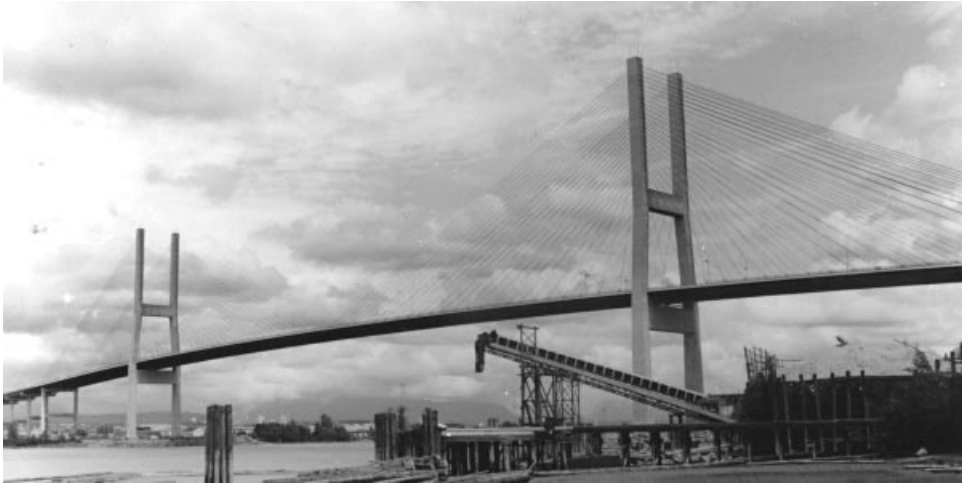
Figure 1.69 Alex Fraser Bridge in Vancouver (Canada)
