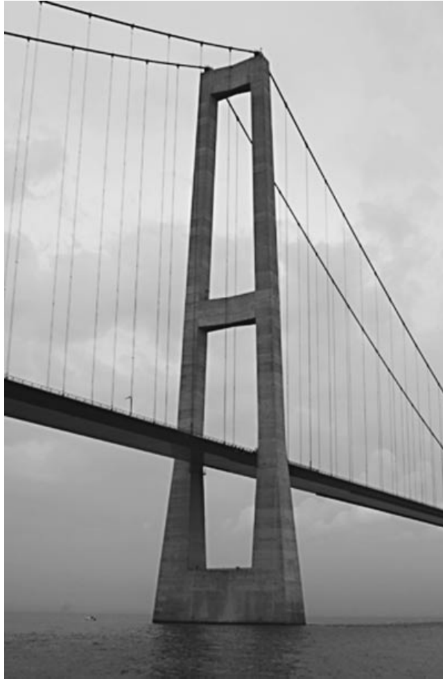
Figure 5.50 Pylon of the Storebælt East Bridge
