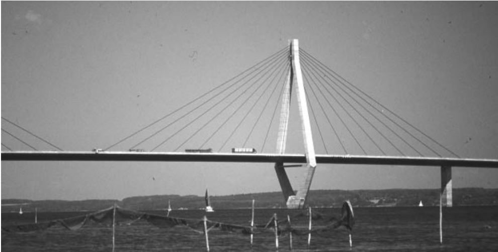
Figure 3.93 Cable system of the Farø Bridge in Denmark
