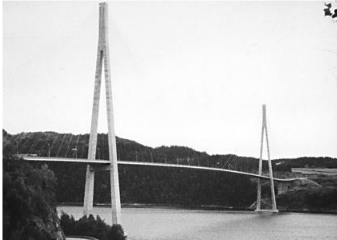
Figure 1.81 Kvarnsund Bridge at Trondheim (Norway)
