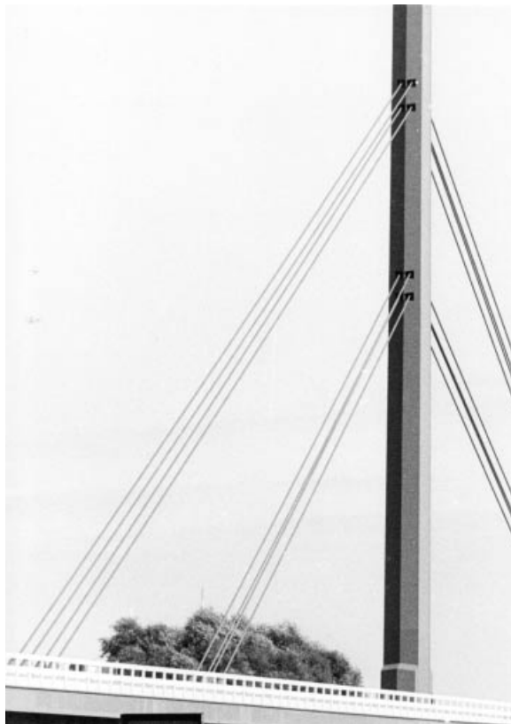
Figure 2.20 Stay cables composed of individual locked-coil strands (renovated Norderelbe Bridge)
