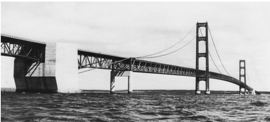
Figure 1.23 Mackinac Bridge in Michigan (USA)
