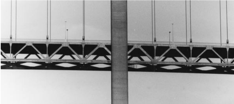
Figure 4.88 Truss of the Tancarville Bridge
