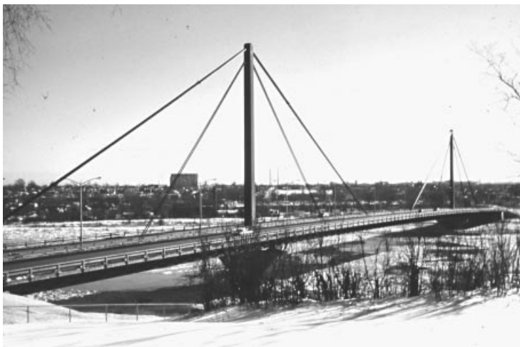
Figure 1.46 Papineau Bridge at Montreal (Canada)
