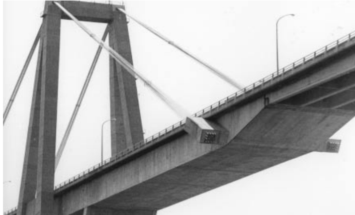
Figure 4.59 Stays anchored to an inclined anchor girder (Maracaibo Bridge)
