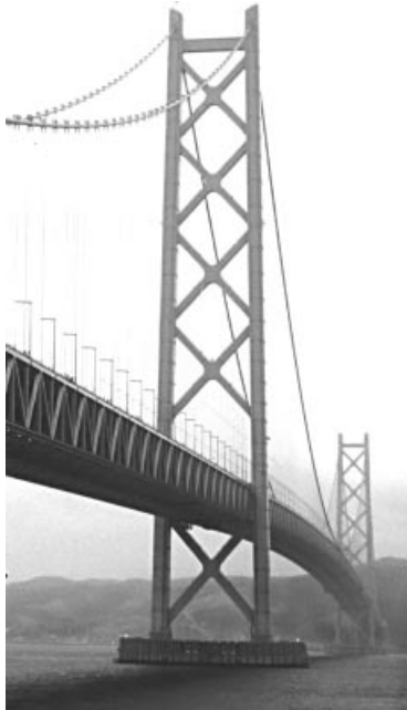
Figure 5.44 Pylon of the Akashi Kaikyo Bridge
