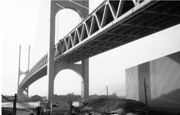
Figure 3.125 The Higashi Kobe Bridge in Kobe
