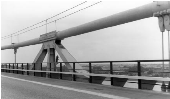
Figure 3.52 Central clamp in the Lillebælt Bridge
