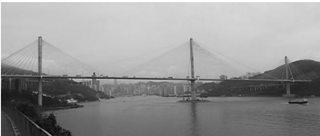
Figure 1.98 Ting Kau Bridge (Hong Kong SAR)
