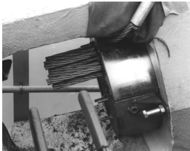
Figure 6.17 Anchorage block with partially installed seven-wire strands in a Freyssinet anchor (Normandy Bridge)
