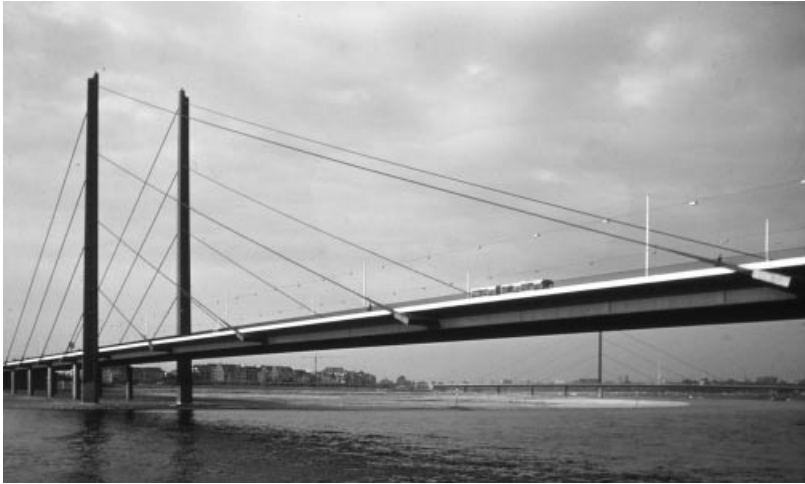
Figure 1.45 Knie Bridge across the Rhine at Düsseldorf (Germany)
