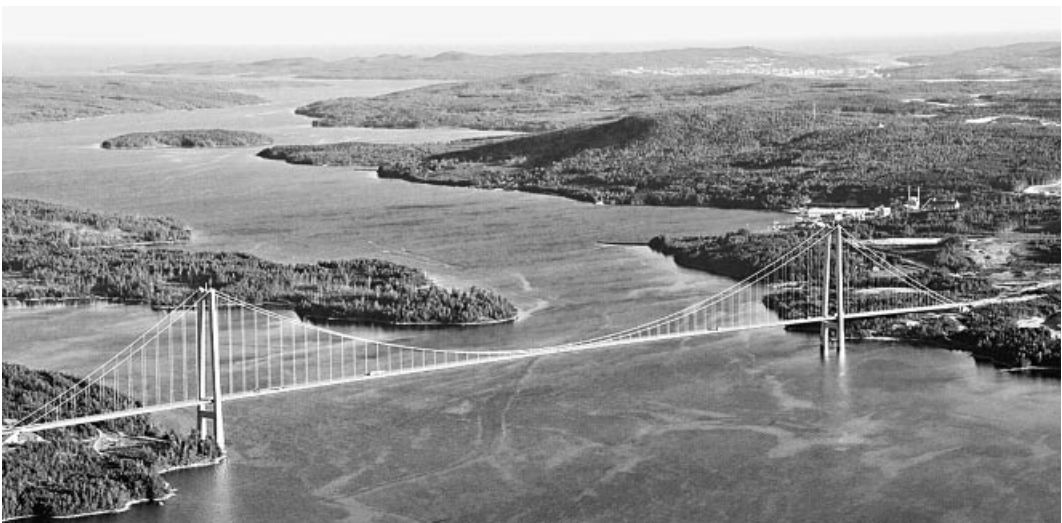
Figure 1.92 Höga Kusten Bridge. (Photo credit: Staffan Gillusson, Swedish Road Administration)
