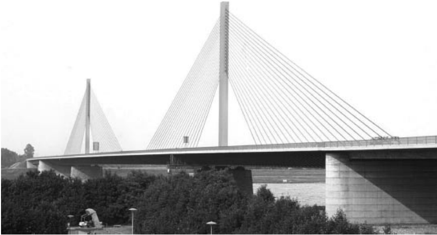
Figure 1.41 Friedrich Ebert Bridge across the Rhine at Bonn (Germany)
