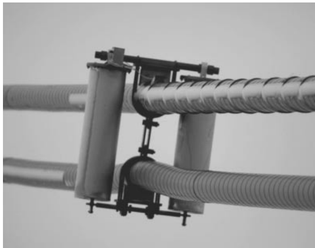
Figure 8.44 Øresund Bridge anchorage viscous radial dampers (top) and tuned mass dampers (bottom) (Courtesy of Øresund Bridge A/S. Photo credit Lennart Emanuelsson)
