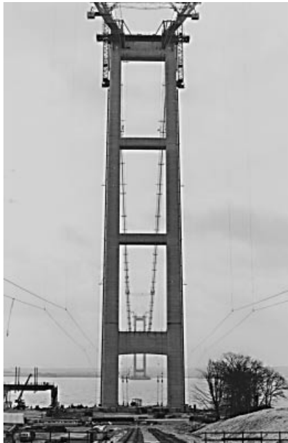
Figure 5.42 Pylon of the Humber Bridge
