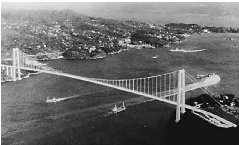
Figure 1.82 Askøy Bridge at Bergen (Norway)
