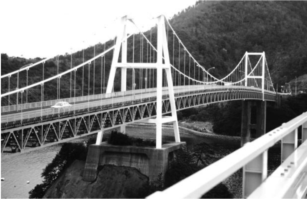
Figure 3.160 Konaruto Bridge with two consecutive 160 m main spans
