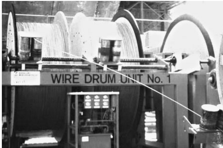
Figure 7.21 Wire drums on the reel stand at the Storebælt Bridge site
