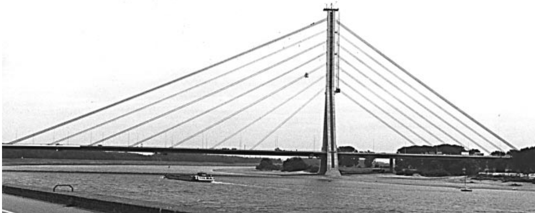
Figure 3.124 Rhine Bridge at Flehe
