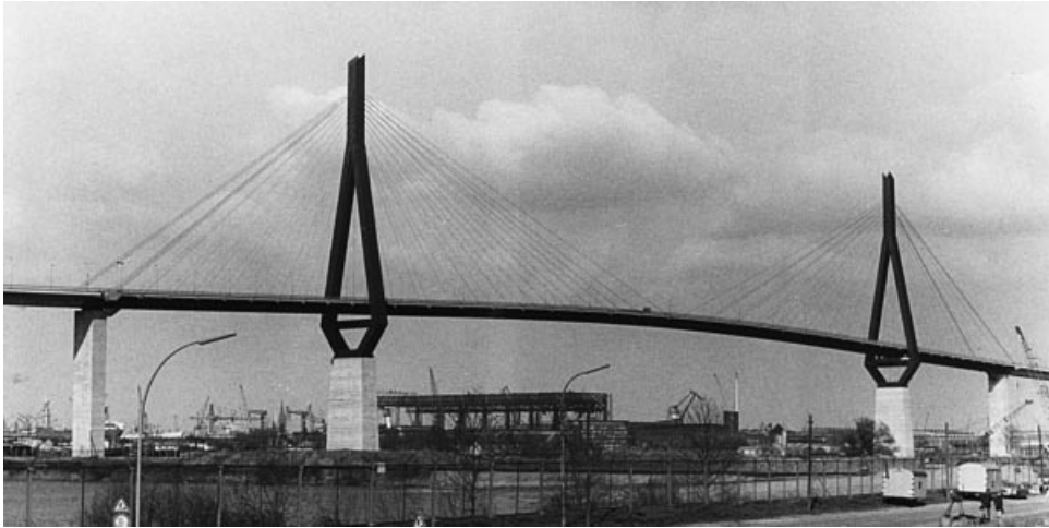
Figure 1.52 Köhlbrand Bridge in the port of Hamburg (Germany)
