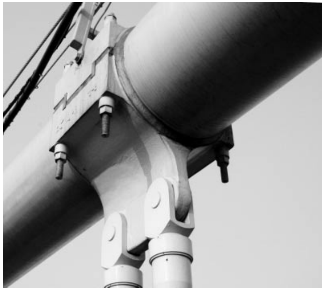
Figure 6.52 Cable clamps for the Runyang Bridge
