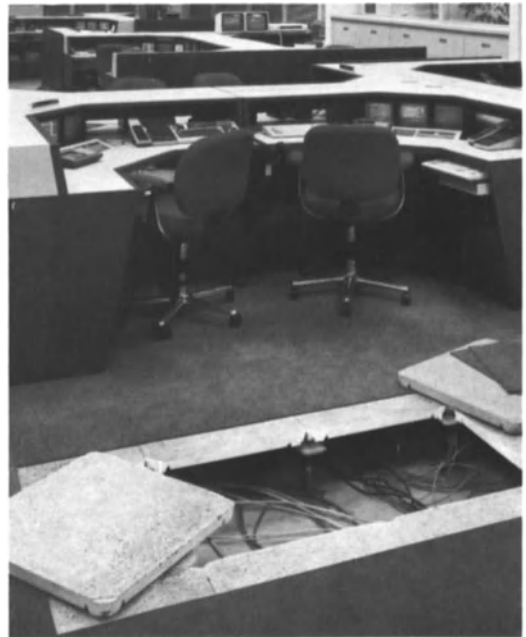
Fig. 16.12. Components and installation views for an access flooring system. Vertically adjustable pedestals support modular deck units that are readily removable for access to wiring or other services. (Courtesy Innocrete Systems, Inc.)
