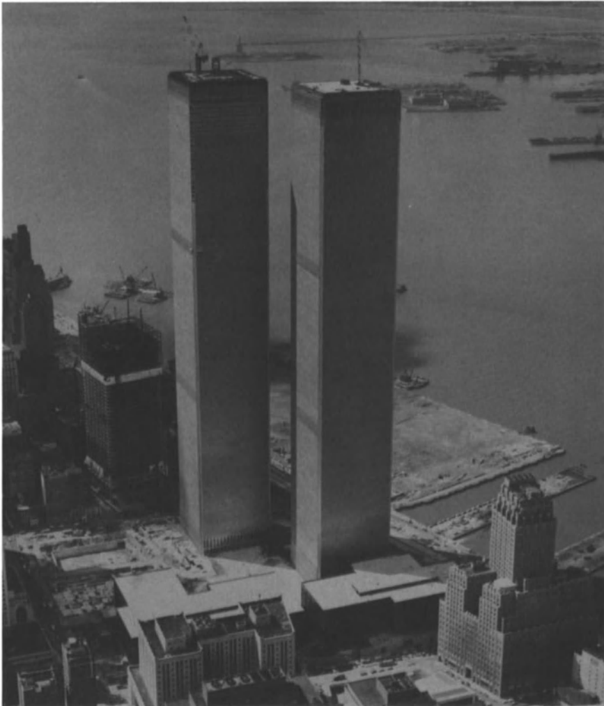
Fig. 8.73. Twin, 110-story towers of World Trade Center, New York City, with perforated-tube construction. (Courtesy Port Authority of New York and New Jersey.)
