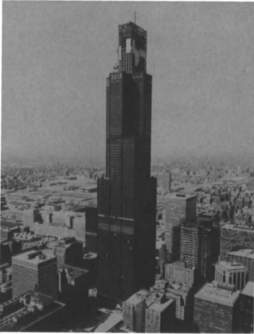
Fig. 8.74. Sears Tower, Chicago, 110 stories high, with bundled tube construction.
