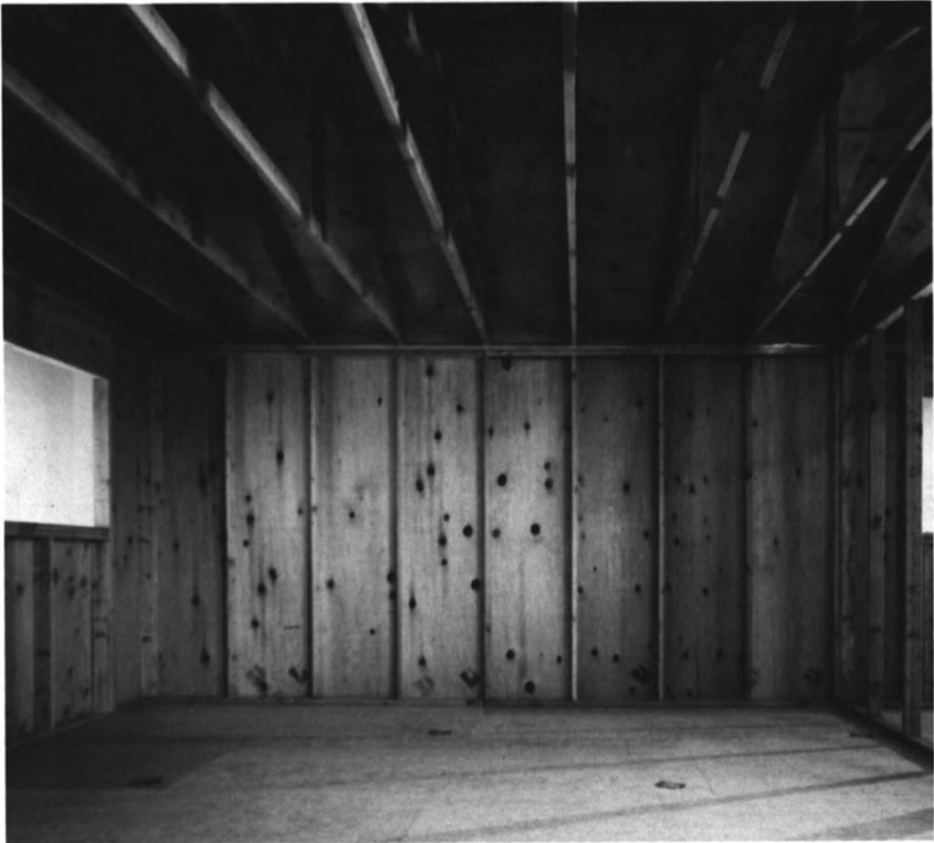
Fig. 2.7. Load-bearing wood-framed wall.
