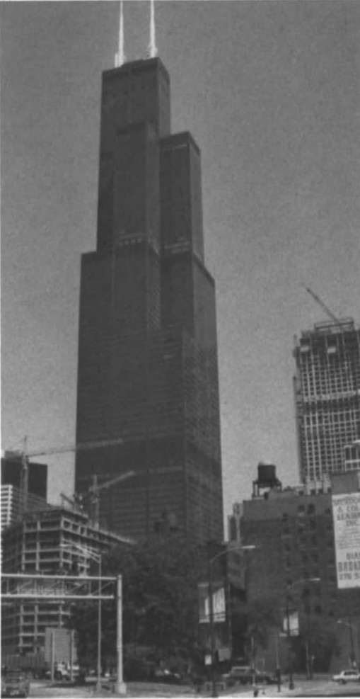
Fig. 1.4. Sears Tower (1974), Chicago, rises 110 stories, 1454 ft. Steel skeleton frame with bundled tube system for lateral load resistance.
