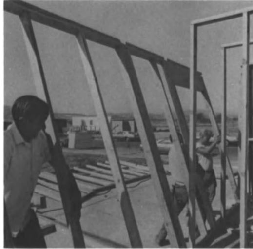
Fig. 8.67. Erection of a prefabricated wood-stud wall. (Courtesy Western Woods Products Association)
