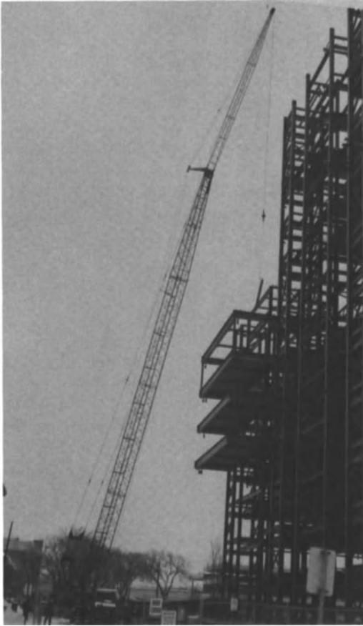
Fig. 8.11. Crane erecting structural steel. (Courtesy of American Hoist and Derrick Company)
