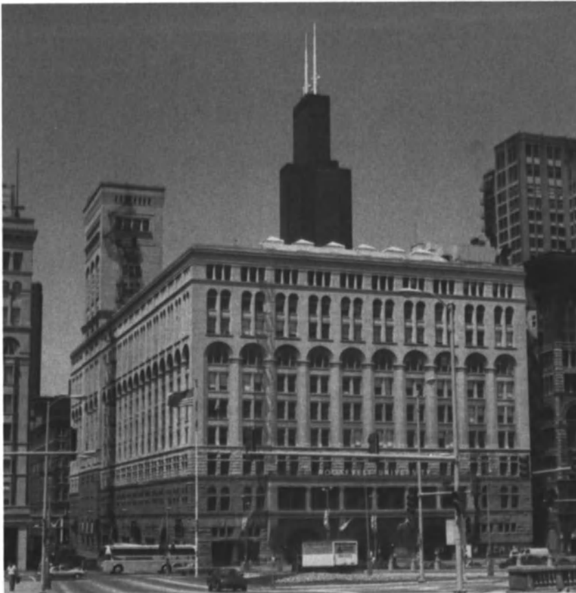
Fig. 1.3. Late 19th Century building, still expressing the basic forms of load-bearing wall construction, although its basic structure is steel framed. Auditorium Hotel, Chicago, by Adler and Sullivan. 80 years later, the worlds tallest steel frame structure, the Sears Tower, looms over it, clearly expressing the frame structure.
