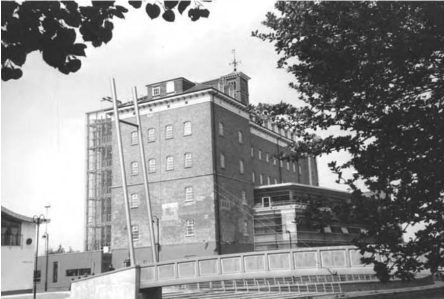
Figure 4.6 A former hosiery factory in Leicester, built as a six-storey worsted spinning mill c. 1844. Recently converted to office use as part of a City Challenge Scheme. To meet the requirements of the tenants, the Land Registry, an extension to the front, overlooking the Grand Union Canal, has been provided in a modern style. To the rear, glazed staircase/lift towers have been added
