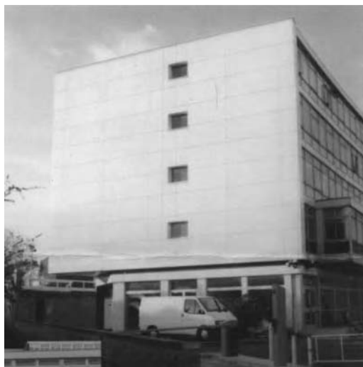
Figure 8.2 Recladding of an office block – before and after ( www.cape.co.uk/ )
