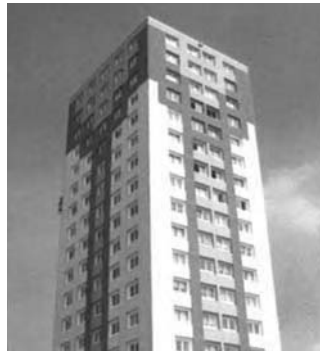
Figure 9.17 Photographs of typical overcladding systems to blocks of multi-storey flats ( www.cape.co.uk/ )
