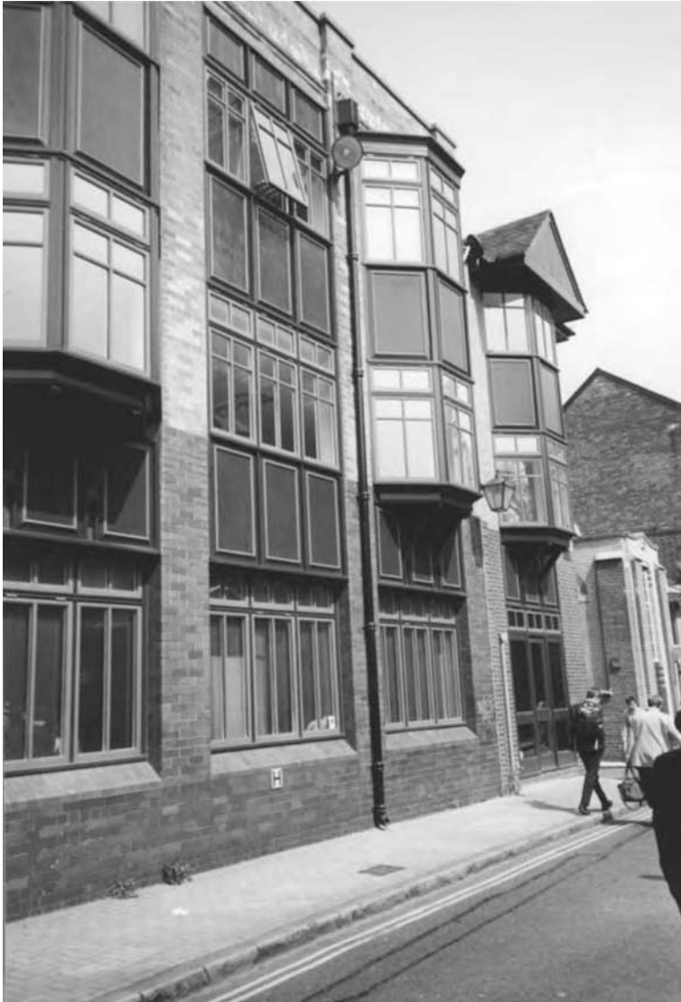
Figure 4.8 A former print works in Leicester adapted to office use. The fenestration has been remodelled and replaces a very bland façade of dull industrial windows
