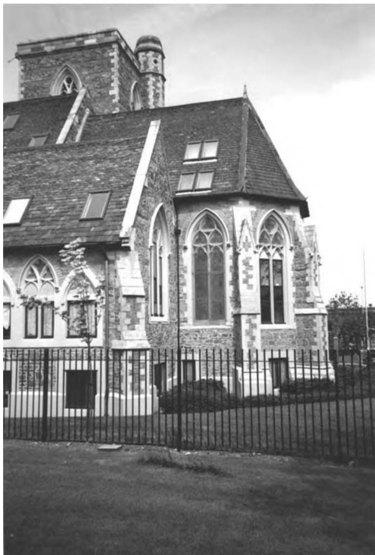
Figure 4.7 The former Anglican church of St John the Divine, Leicester 1853–1854 by G. G. Scott. After several years of being redundant the church has been converted to flats. Note how the building has been disfigured by the inclusion of roof lights and clumsy alterations to the windows
