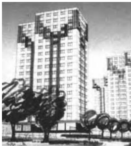
Figure 9.17 Photographs of typical overcladding systems to blocks of multi-storey flats ( www.cape.co.uk/ )
