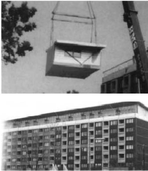
Communal space added to the roofs in Rodowa, Copenhagen
