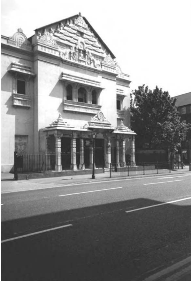
Figure 4.9 A former congregational chapel in Leicester dating from 1865 converted to a Jain temple in the 1980s. (Jainism is an ancient Indian religion which teaches love to all creatures and non-violence.) The interior has been remodelled and the exterior clad in marble and other stone sculpted in India
