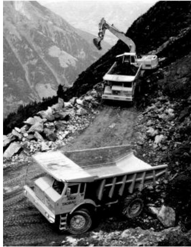
Fig. 1. A waiting queue in earth work.
