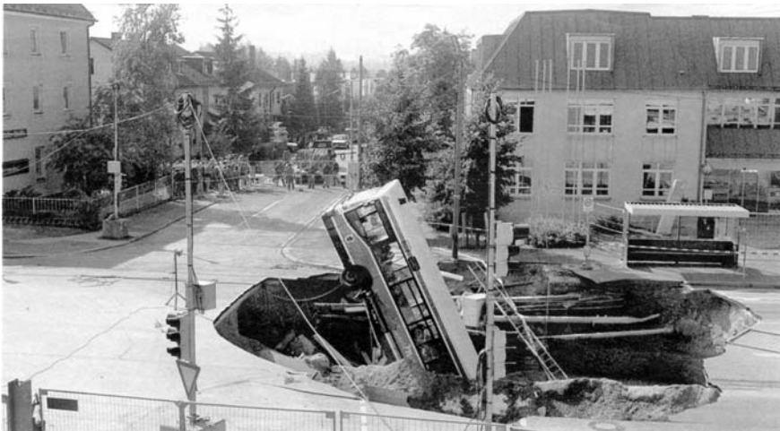
Fig. 1. Munich Trudering collapse, Subway line 2 - East Section 2 [9]
