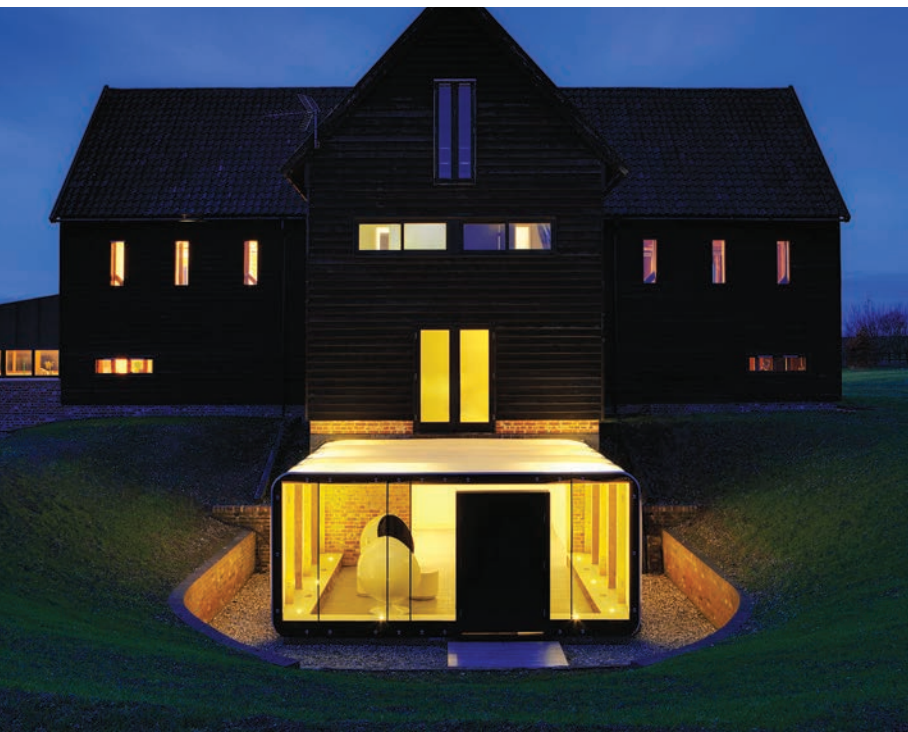
AirClad house extension structure with opaque PVC inflatable skin.
