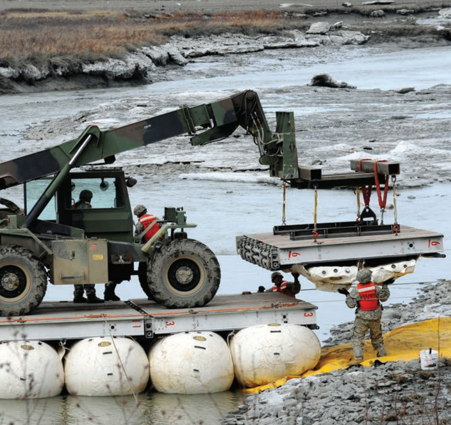
Lightweight Modular Causeway System during a trial assembly in Alaska.
