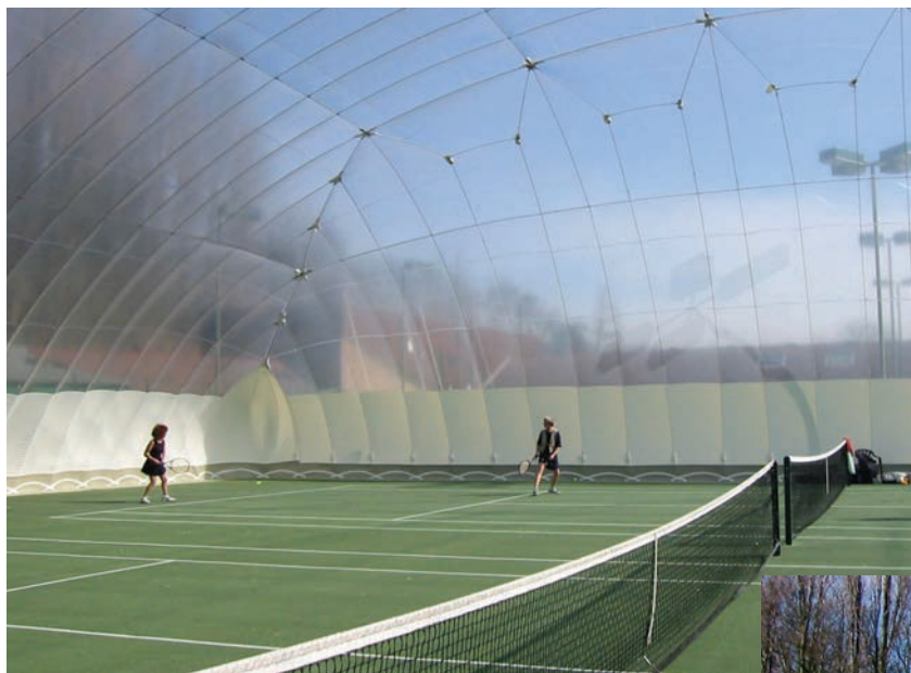
Interior photograph of the Airhall showing its 'net' of cables.
