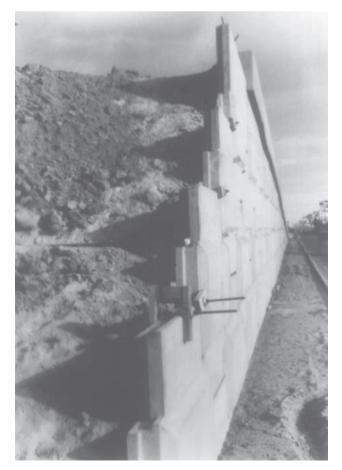
Figure 13.24 Reinforced-earth retaining wall (with metallic strip) under construction (Courtesy of Braja M. Das, Henderson, Nevada)
