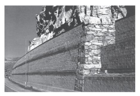
Figure 13.33 A completed geotextile-reinforced retaining wall in DeBeque Canyon, Colorado (Courtesy of Jonathan T. H. Wu, University of Colorado at Denver, Denver, Colorado)
