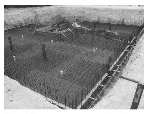
Figure 8.6 A flat plate mat foundation under construction (Courtesy of Dharma Shakya, Geotechnical Solutions, Inc., Irvine, California)
