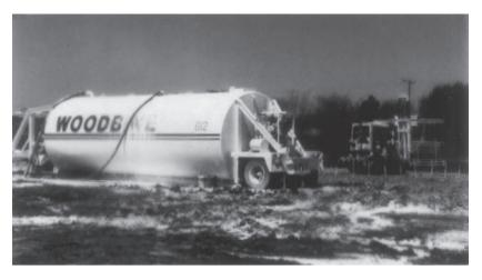
Figure 11.23 Pressure injection of lime slurry for a building pad (Courtesy of Hayward Baker Inc., Odenton, Maryland.)
