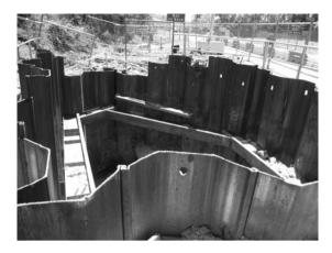
Figure 14.5 A small enclosure with steel sheet piles for an excavation work (Courtesy of N. Sivakugan, James Cook University, Australia)
