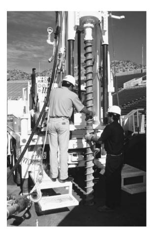
Figure 3.12 Drilling with continuous-flight augers (Danny R. Anderson, PE of Professional Service Industries, Inc, El Paso, Texas.)
