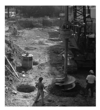
Figure 10.5 Drilled shaft construction using the dry method (Courtesy of Sanjeev Kumar, Southern Illinois University, Carbondale, Illinois)
