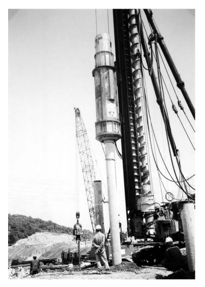
Figure 9.8 A pile-driving operation in the field (Courtesy of E. C. Shin, University of Incheon, Korea)
