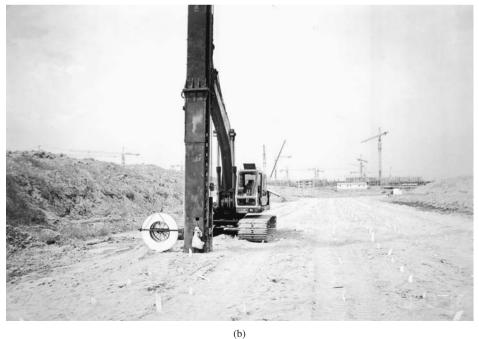
Figure 16.26 Installation of PVDs in the field [Note: (b) is a closeup view of (a)] (Courtesy of E. C. Shin, University of Incheon, Korea)
