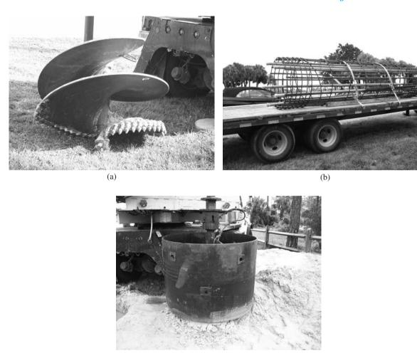
Figure 10.7 Drilled shaft construction: (a) A typical auger; (b) a reinforcement cage; (c) a cleanout bucket (Courtesy of Khaled Sobhan, Florida Atlantic University, Boca Raton, Florida)
