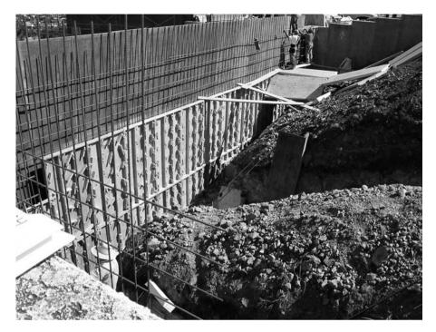
Figure 13.2 A cantilever retaining wall under construction (Courtesy of Dharma Shakya, Geotechnical Solutions, Inc., Irvine, California)
