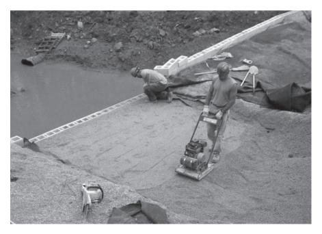
Figure 13.32 Construction of a geotextile-reinforced retaining wall (Courtesy of Jonathan T. H. Wu, University of Colorado at Denver, Denver, Colorado)
