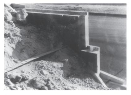
Figure 13.26 Metallic strip attachment to the precast concrete slab used as the skin (Courtesy of Braja M. Das, Henderson, Nevada)
