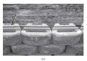
Figure 13.37 (a) HDPE geogridreinforced wall with precast concrete panel facing under construction; (b) mechanical splice between two pieces of geogrid in the working direction; (c) segmented concreteblock faced wall reinforced with uniaxial geogrid (Courtesy of Tensar International Corporation, Atlanta, Georgia)
