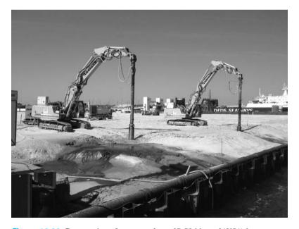
Figure 16.32 Construction of a stone column [DGI-Menard (USA).]
