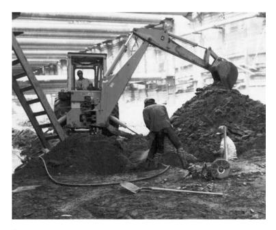
Figure 15.3 Braced cut in the construction of Washington, D.C. Metro, May 1974 (Courtesy of Ralph B. Peck)
