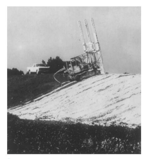
Figure 16.31 Pressure injection of lime slurry (Courtesy of Hayward Baker Inc., Odenton, Maryland)
