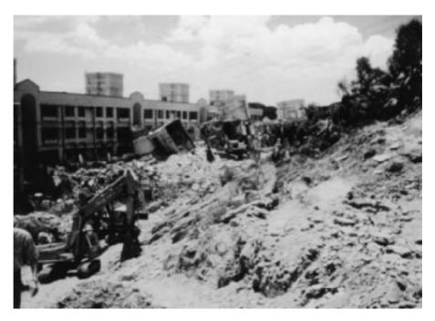
Figure 15.2 Soil and rock "fall" in a slope (Courtesy of E.C. Shin, University of Inchon, South Korea)
