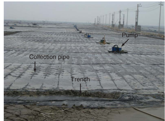
Figure 7.24 A vacuum preloading site with multiple vacuum pumps.
