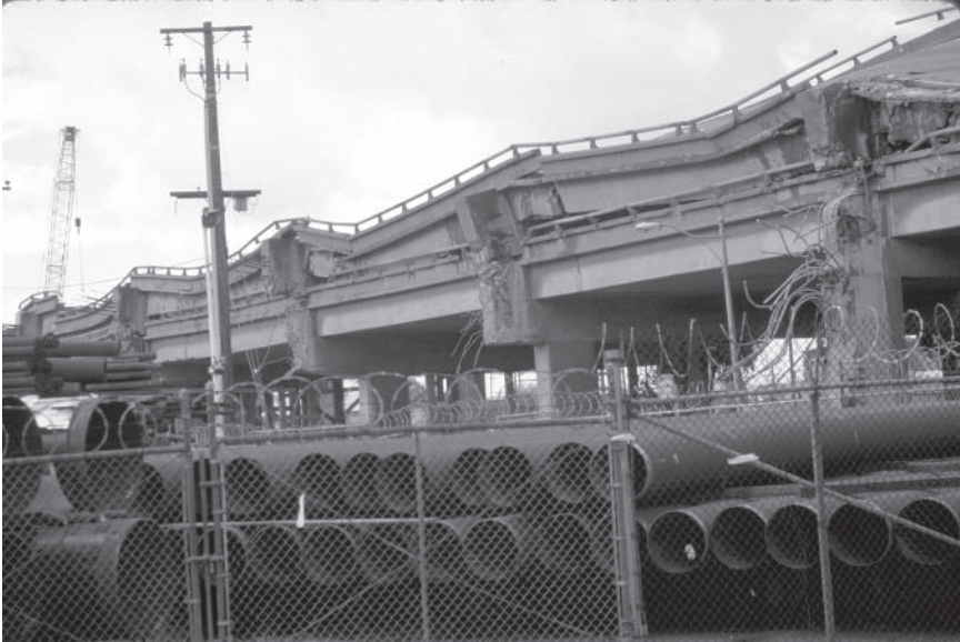
FIGURE 2.5 Collapse of the Cypress Avenue Freeway, 1989 Loma Prieta, California, earthquake. Reproduced courtesy of the National Information Service for Earthquake Engineering, University of California, Berkeley.
