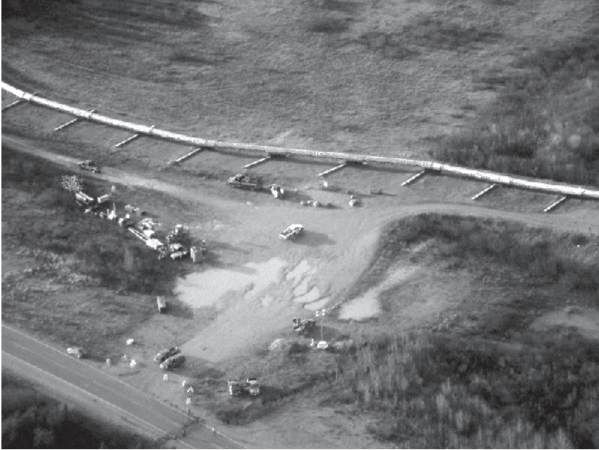
FIGURE 1.1 An aerial photo of the Trans-Alaska Pipeline System (TAPS) line near the Denali fault, looking west. SOURCE: Alaska Department of Natural Resources. Photo by Rod Combellick, Division of Geological and Geophysical Surveys.
