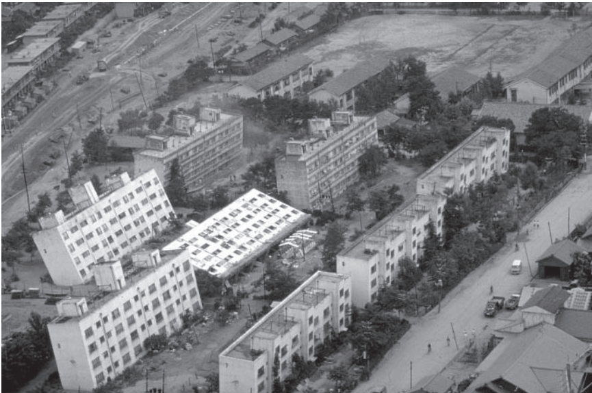
FIGURE 2.3 Foundation failures resulting from liquefaction, 1964 Niigata, Japan, earthquake. Reproduced courtesy of the National Information Service for Earthquake Engineering, University of California, Berkeley.
