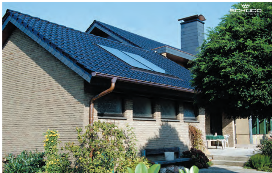
Figure 4.27. Example of in-roof installation. Source: Schüco, Bielefeld
