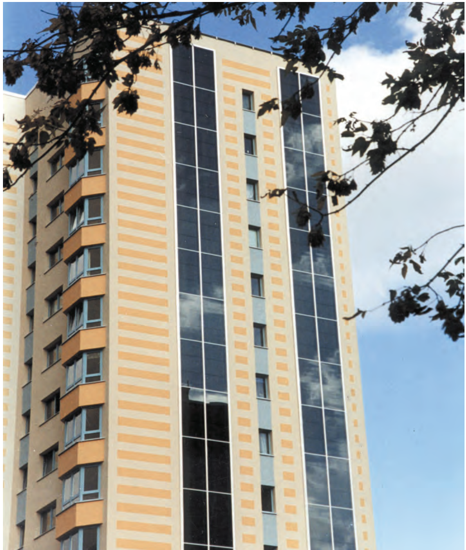
Figure 8.32. Solar air system at Breite Strasse, Potsdam. Source: DGS
