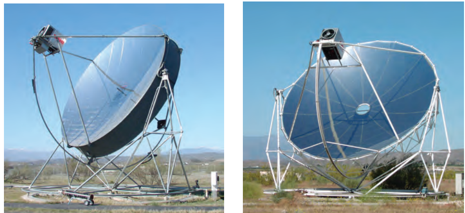
Figure 6.15. Dish/Stirling demonstration systems in Almería, Southern Spain. Source: Volker Quaschnig
