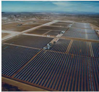
Figure 6.7. Parabolic trough power plants in California. Source: KJC
