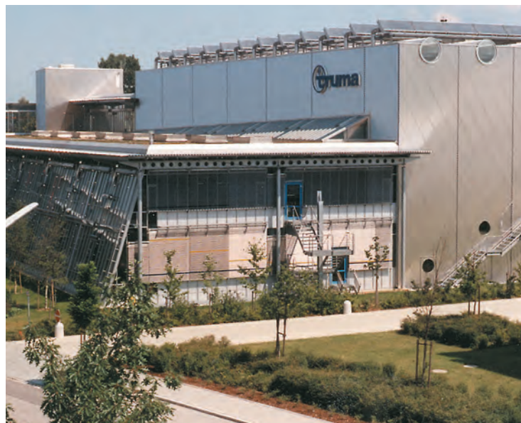
Figure 8.5. Air collectors placed on stands on the roof of a factory building. Source: Grammer, Amberg
