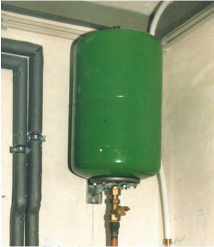
Figure 4.57 False expansion vessel connection from below
