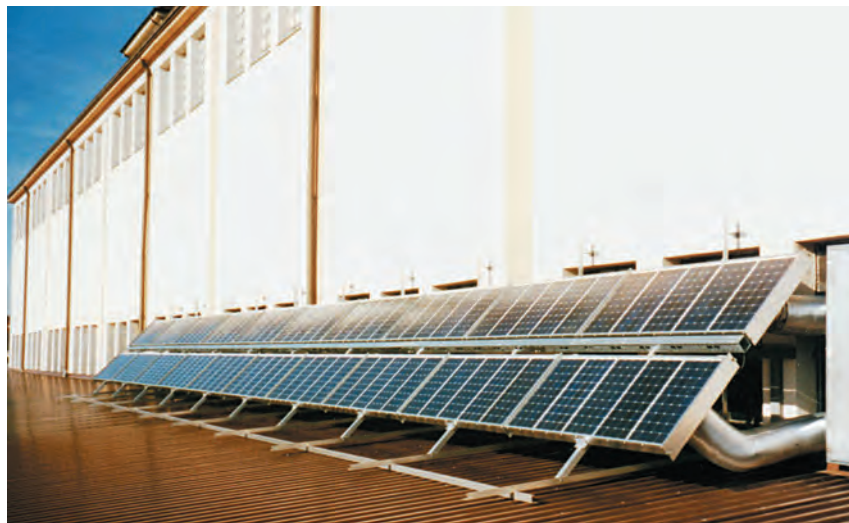
Figure 8.7. Hybrid collectors for solar air heating and generation of electricity for an automotive paint shop (Manufacturer: Grammer Solar+Bau GmbH, Amberg)
