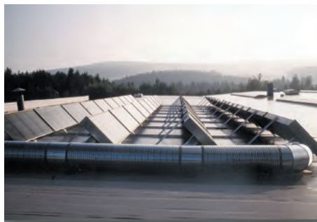
Figure 8.28. Stand-mounted solar air system on the roof of a hall. Source: Grammer, Amberg
