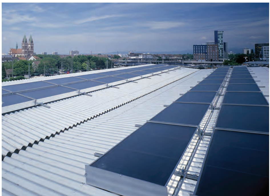
Figure 9.1. 100 m 2 collector system for a solar-powered air-conditioning system in Freiburg, Germany. Source: Fraunhofer ISE
