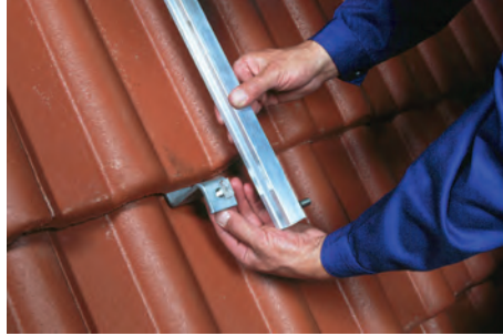
Figure 4.21. Example of on-roof installation Source: Wagner and Co., Cölbe
