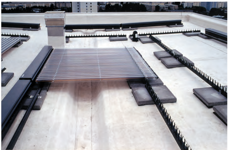
Figure 4.30. Direct flow-through evacuated tube collector on a flat roof. Source: Viessmann, Allendorf
