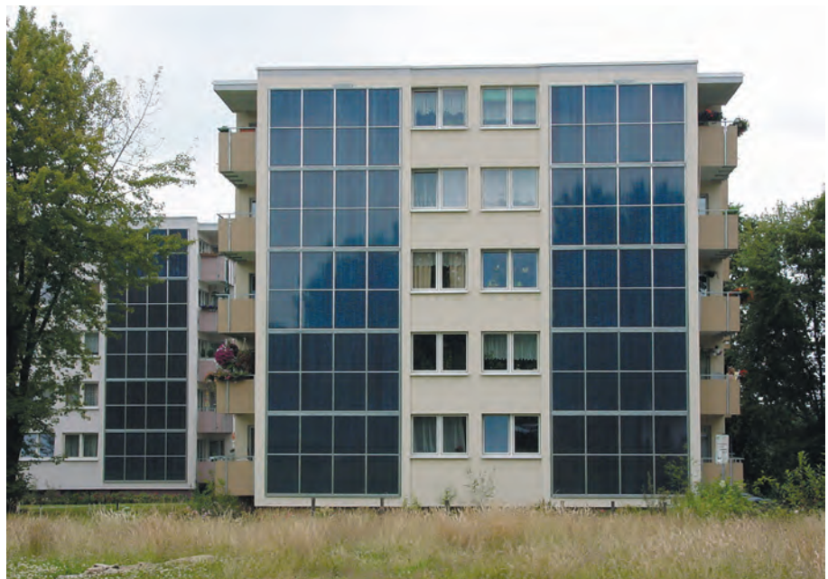
Figure 4.36. Façade installation of a large surface collector in Bielefeld. Source: Wagner & Co, Cölbe
