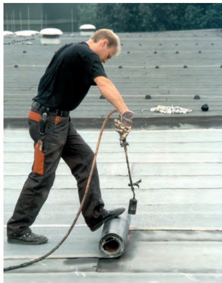
Figure 4.7. Left: welded sheet installation on flat roof 28 . Right: plastic roof sheeting 29
