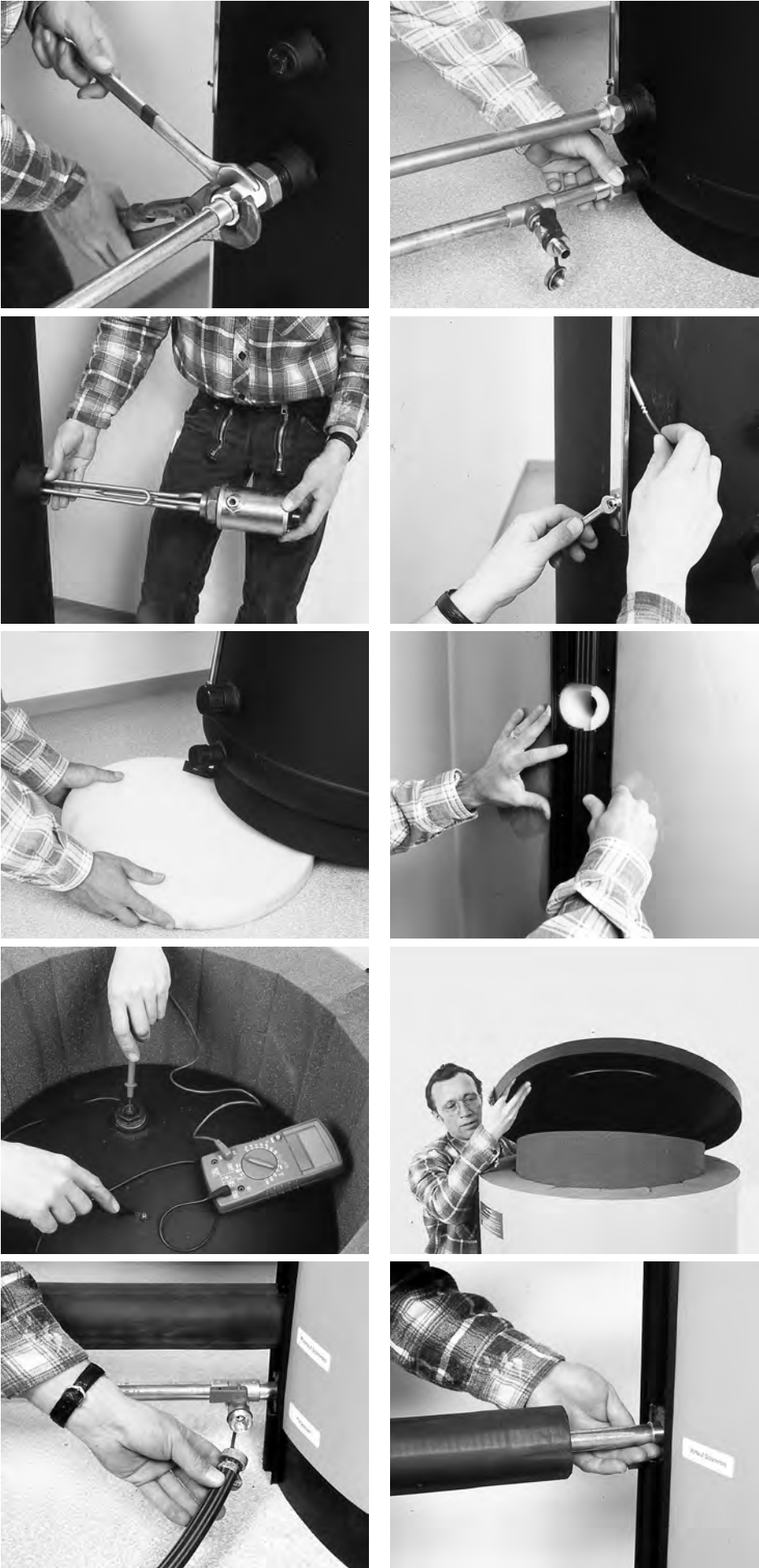
Figure 4.44. Connection and thermal insulation of a solar store Source: Wagner and Co., Cölbe
